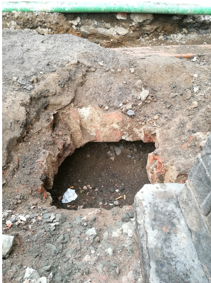
Plate 3 exposed cellar showing brick barrel roof and infill
