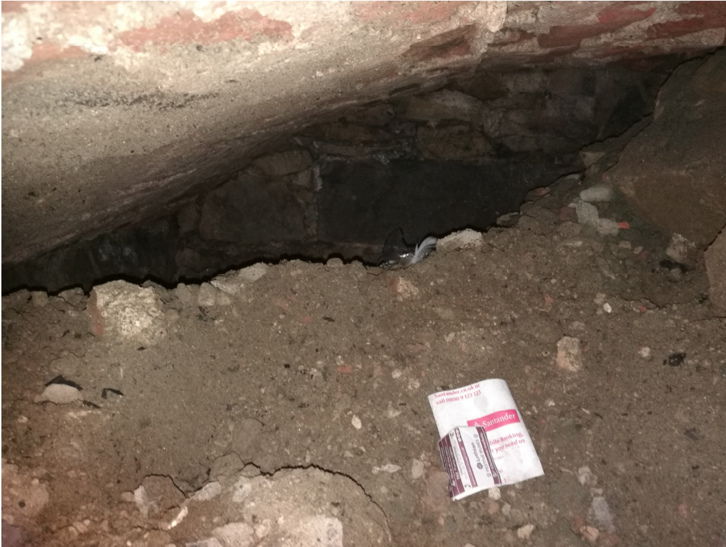
Plate 2 Interior of northern cellar showing probable door lintel
