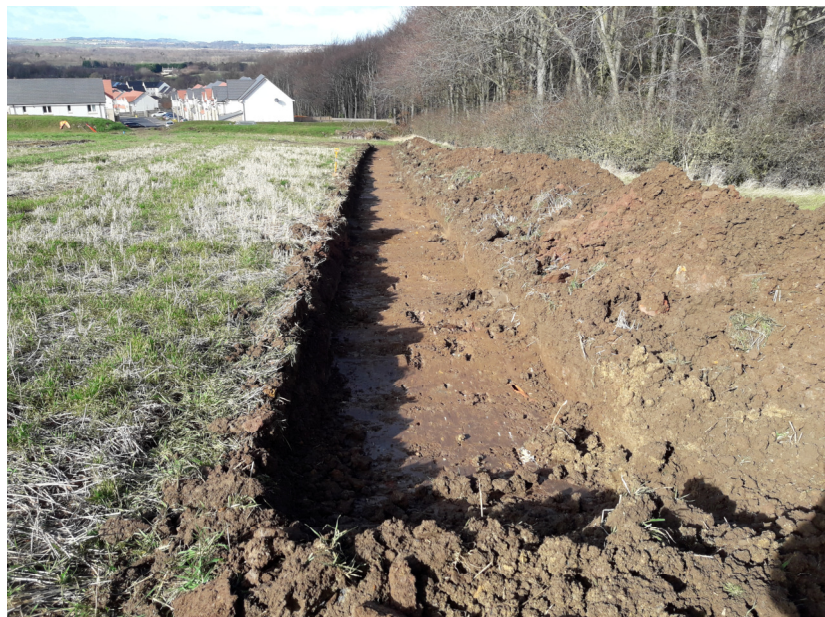
Plate 2: Trench 1 post excavation
