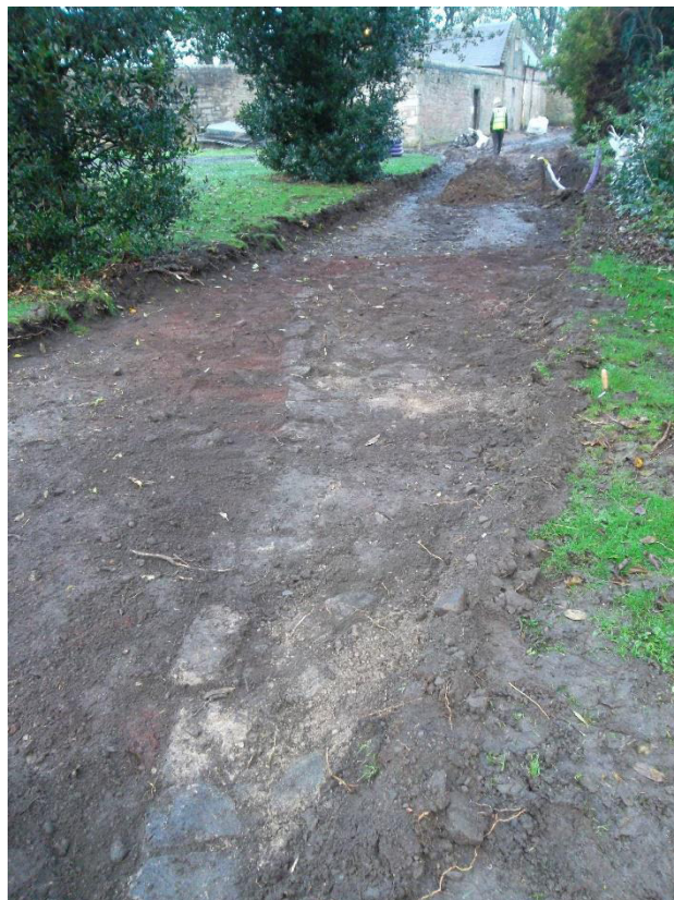
Plate 3: Surface [108] exposed NW of main excavation
