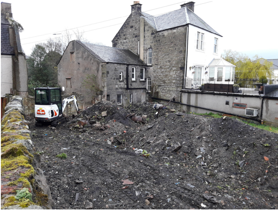
Plate 1 – General view of site showing excavated material
