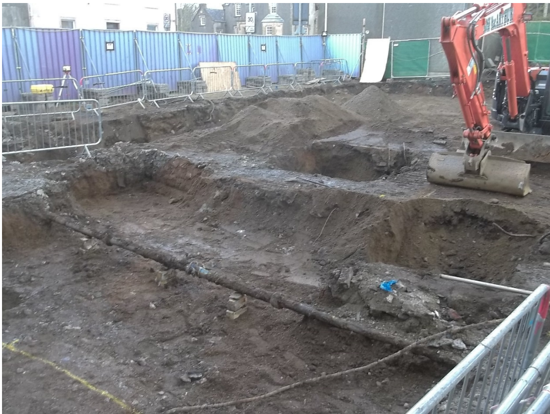
Plate 4: Stripping of area to formation level
