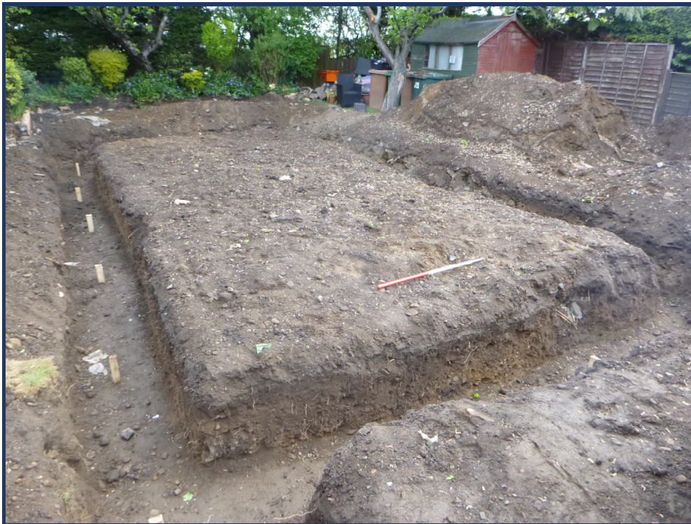
Plate 1: General shot of excavated foundation trench
