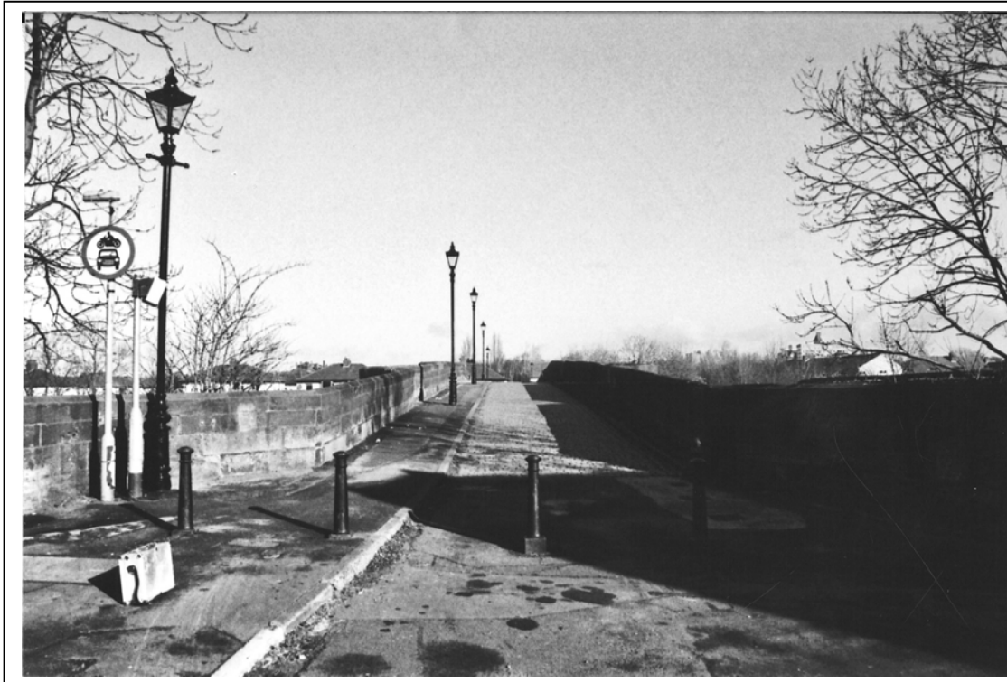
Figure 5: Penwortham Bridge from west following works
