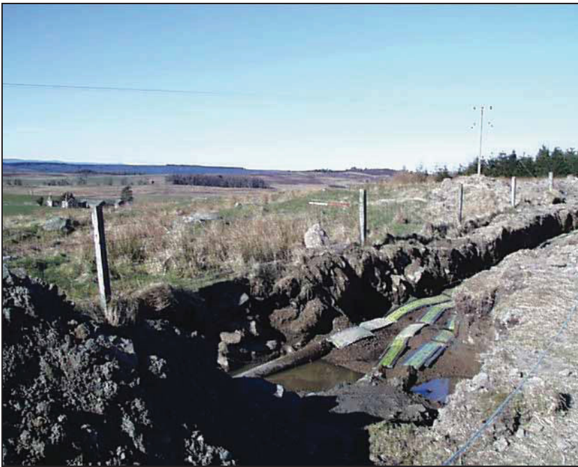
Plate 6 Watching brief area showing rectilinear structure
