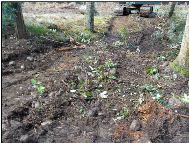
Plate 10: Post-removal of vegetation within access route to BTB4002 position
