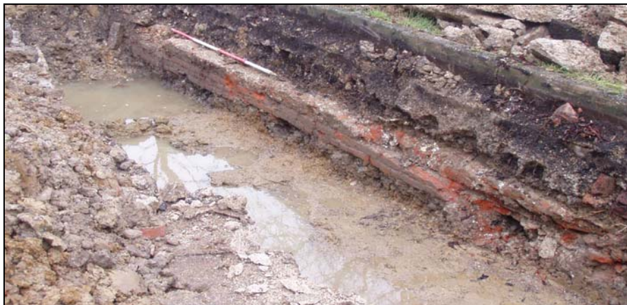
Plate 3. Brick building foundation [2/006].
