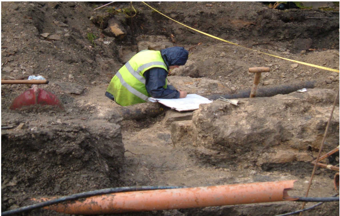
Plate 6: Culvert/Wall [028] & Wall [022] under excavation
