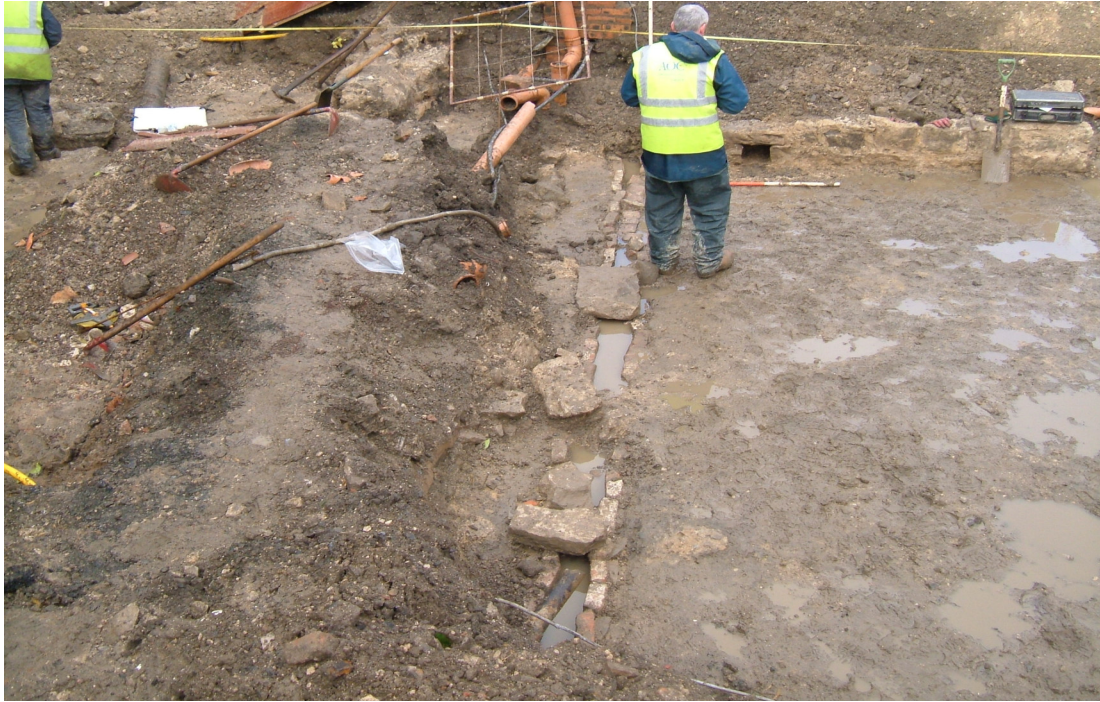
Plate 5: Brick Drain [010-012] under excavation
