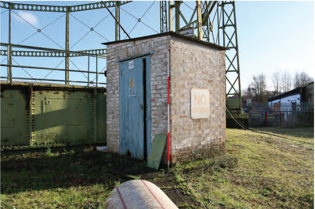
Plate 61: Gasholder No 1, general view of the anti-freeze room, from the north-west
