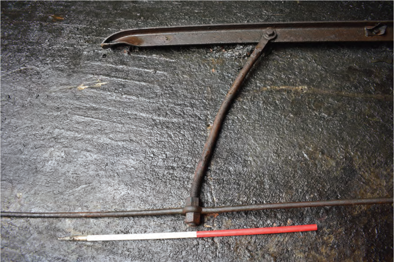
Plate 49: Gasholder No 1, detail view of bolted joint between T-section iron ribbon and iron bar
