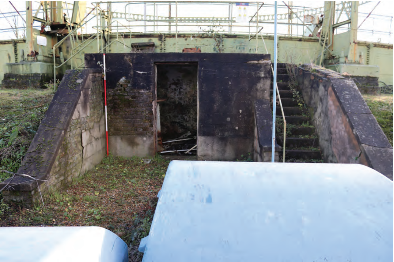
Plate 51: Gasholder No 1, general view of the inlet/outlet building exterior NNW side, from the NNW
