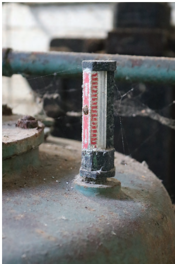
Plate 144: Structure N, detail view of gauge on the volumetric governor, from the west
