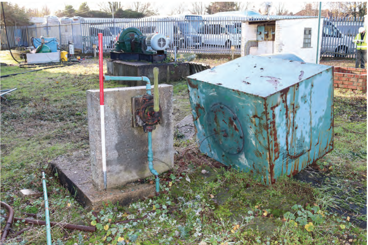
Plate 120: Structure E, general view of diesel tank setting remnants, from the NNE
