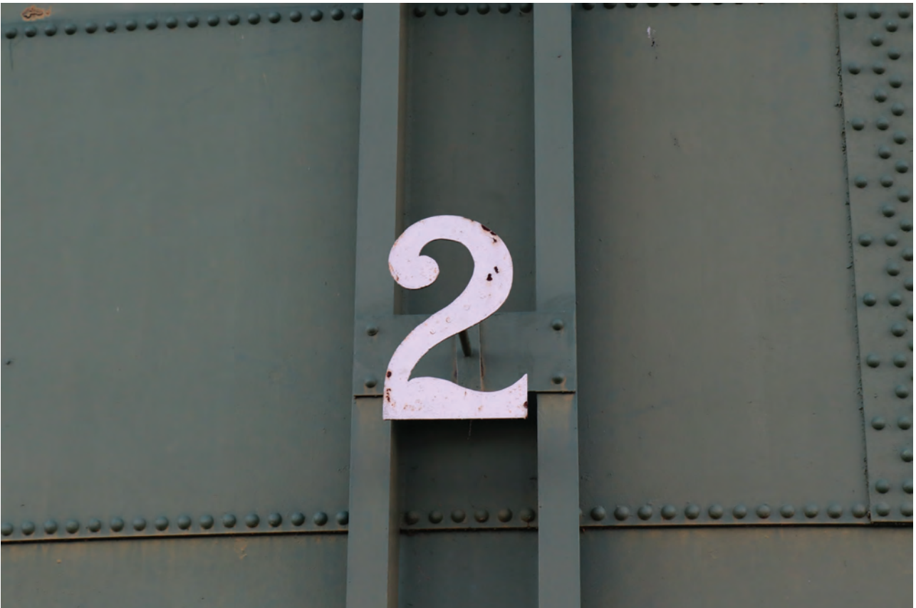
Plate 72: Gasholder No 2, detail view of '2' on the north-west side, from the north-west
