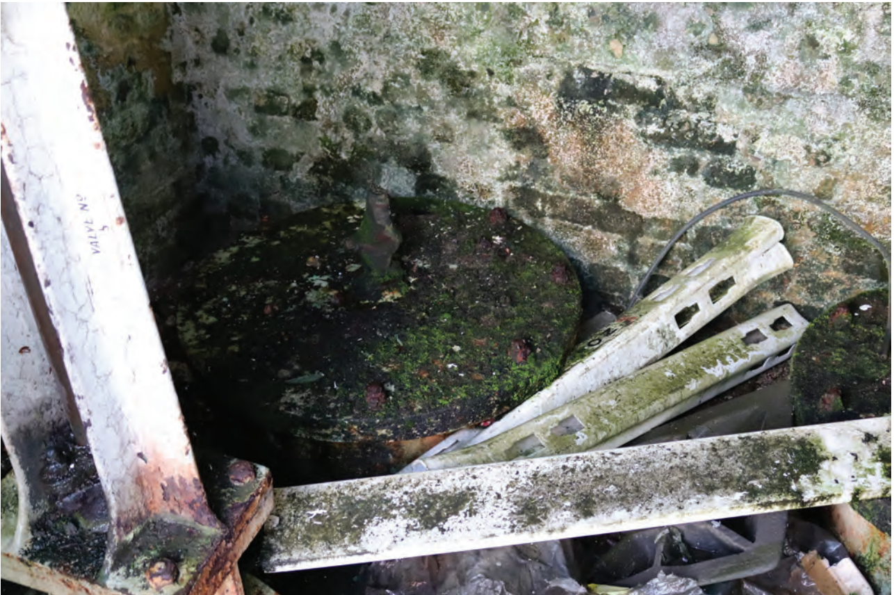
Plate 53: Gasholder No 1, detail view of northernmost inlet/outlet pipe, from the north-west
