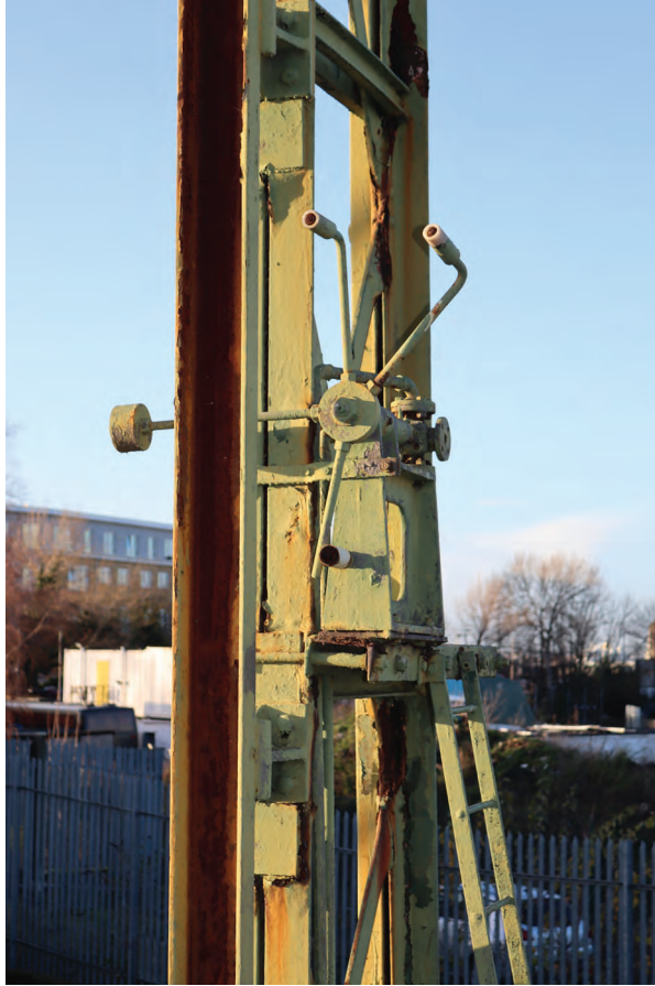
Plate 57: Gasholder No 1, detail view of gasmatic knock-off switch on the east side of standard 14, from the SSE
