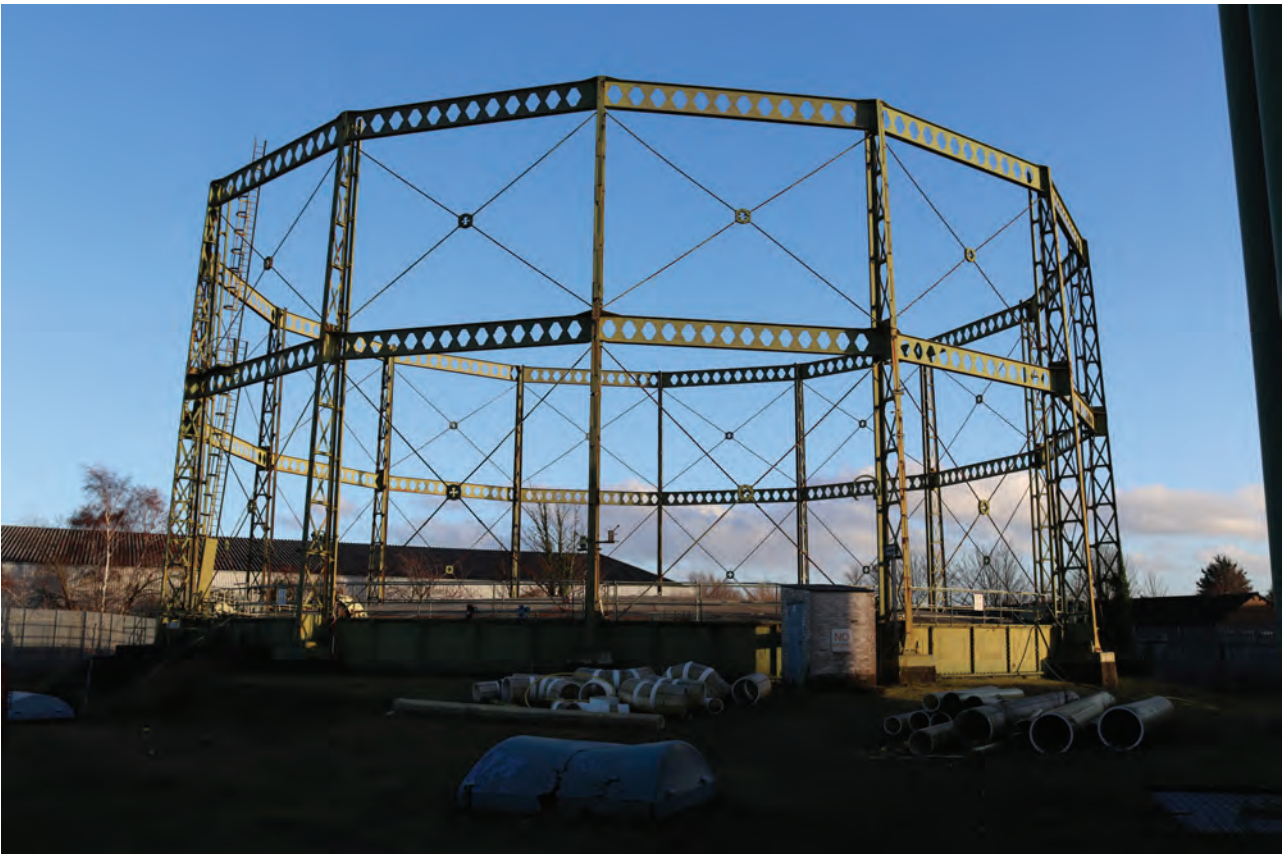
Plate 8: Gasholder No 1, general view of the north-west side, from the north-west
