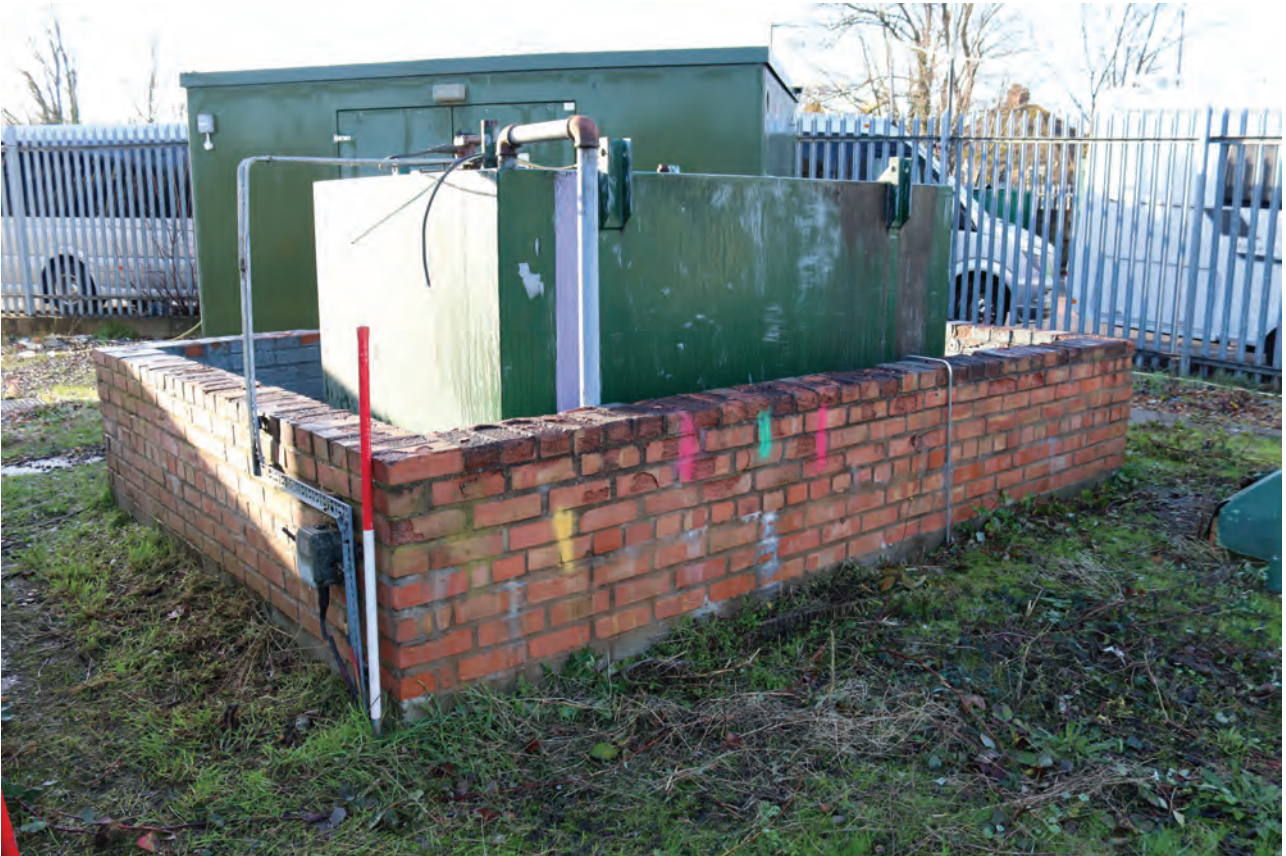
Plate 131: Structure I, general view of the meg tank, from the north-east
