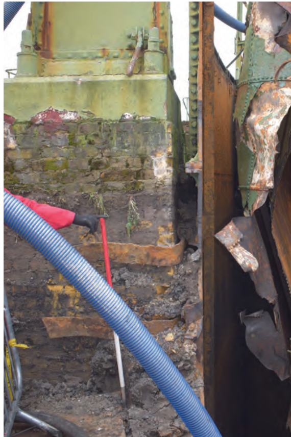
Plate 13: Gasholder No 1, detail view of section through tank showing below ground brick footing of standard 14, from the south-west
