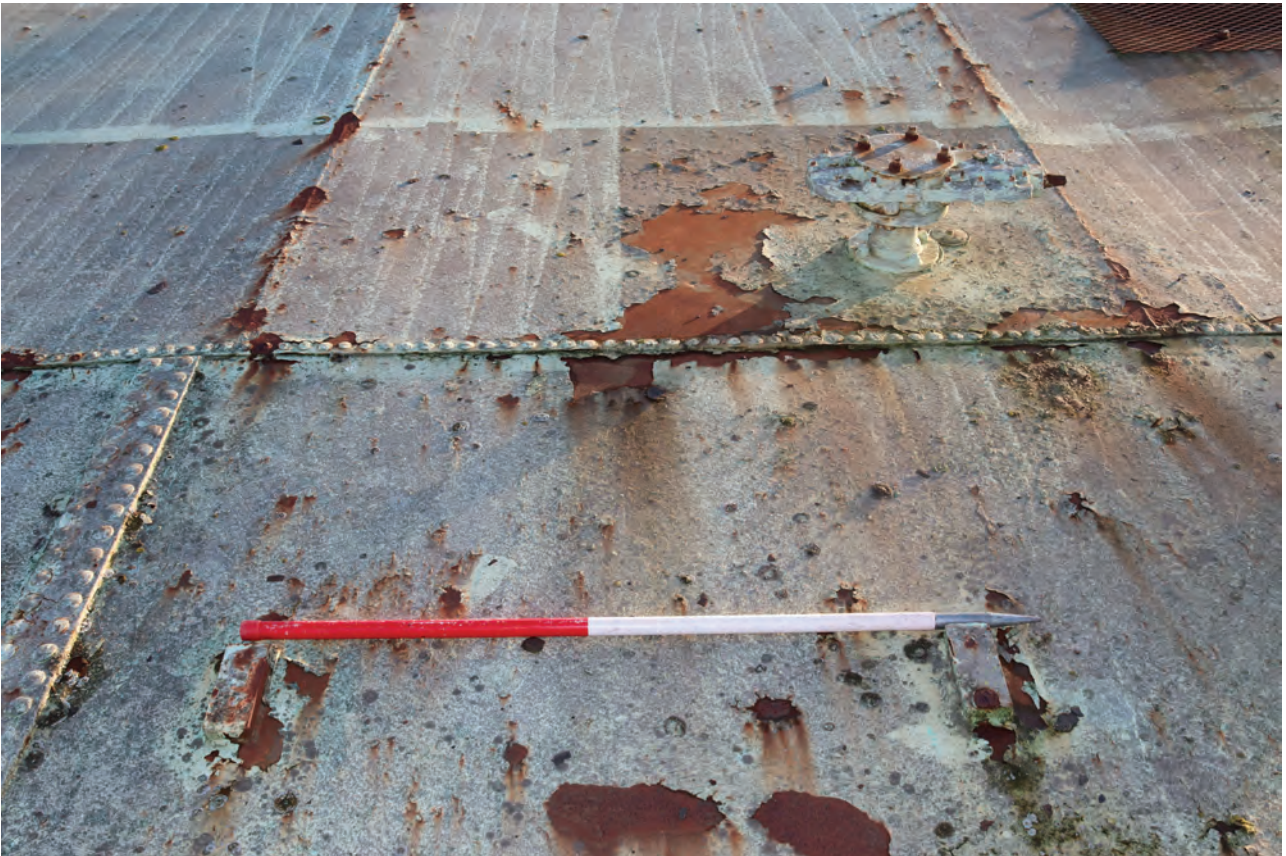
Plate 41: Gasholder No 1, detail view of crown vent and footings of previous handrail on the NNW, from the NNW
