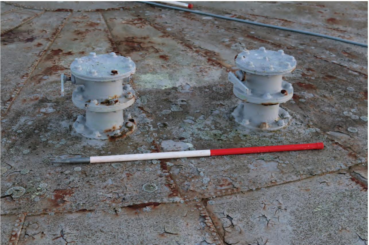
Plate 88: Gasholder No 2, detail view of two crown vents on the north-west side of the crown centre, from the north-west
