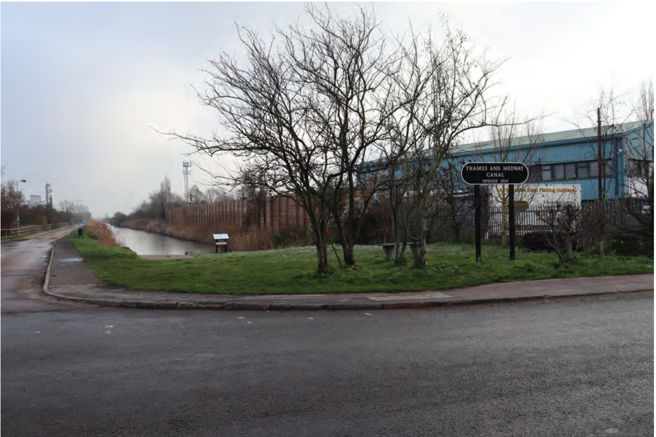
Plate 5: General view of the Thames and Medway Canal west end, from the west
