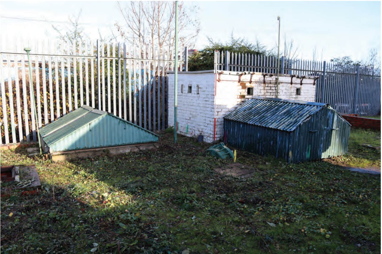
Plate 137: Structures M-O, general view, from the south-west
