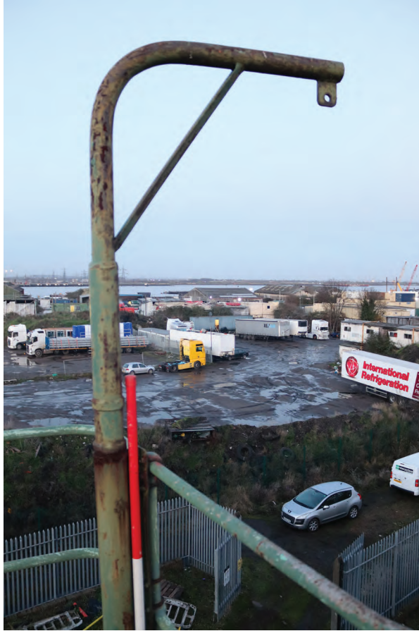
Plate 107: Gasholder No 2, detail view of winch support post, from the SSW
