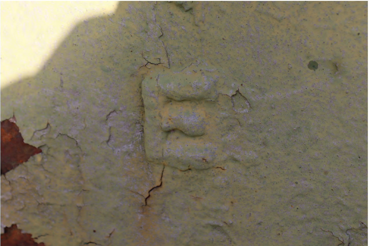
Plate 25: Gasholder No 1, detail view of embossed 'E' near the base of each tank panel
