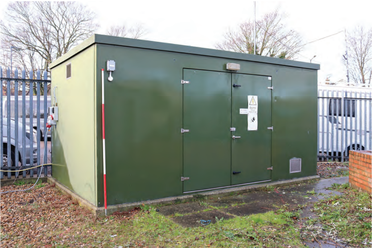
Plate 108: Gasholder No 2 & Structure A, general view of Structure A exterior north-east wall, from the ENE
