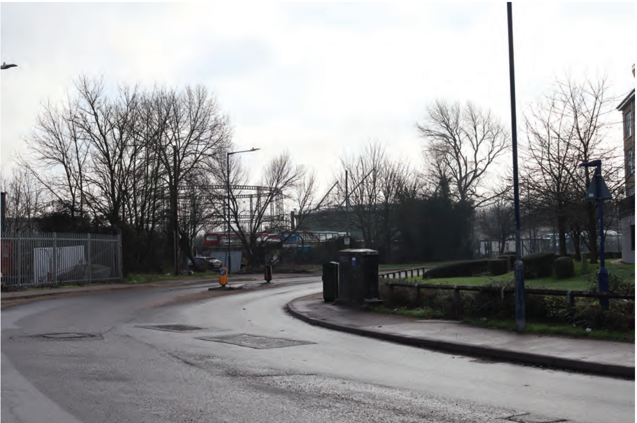
Plate 2: Gasholders Nos 1 & 2, obscured from view by trees in the flat landscape, from the north-west
