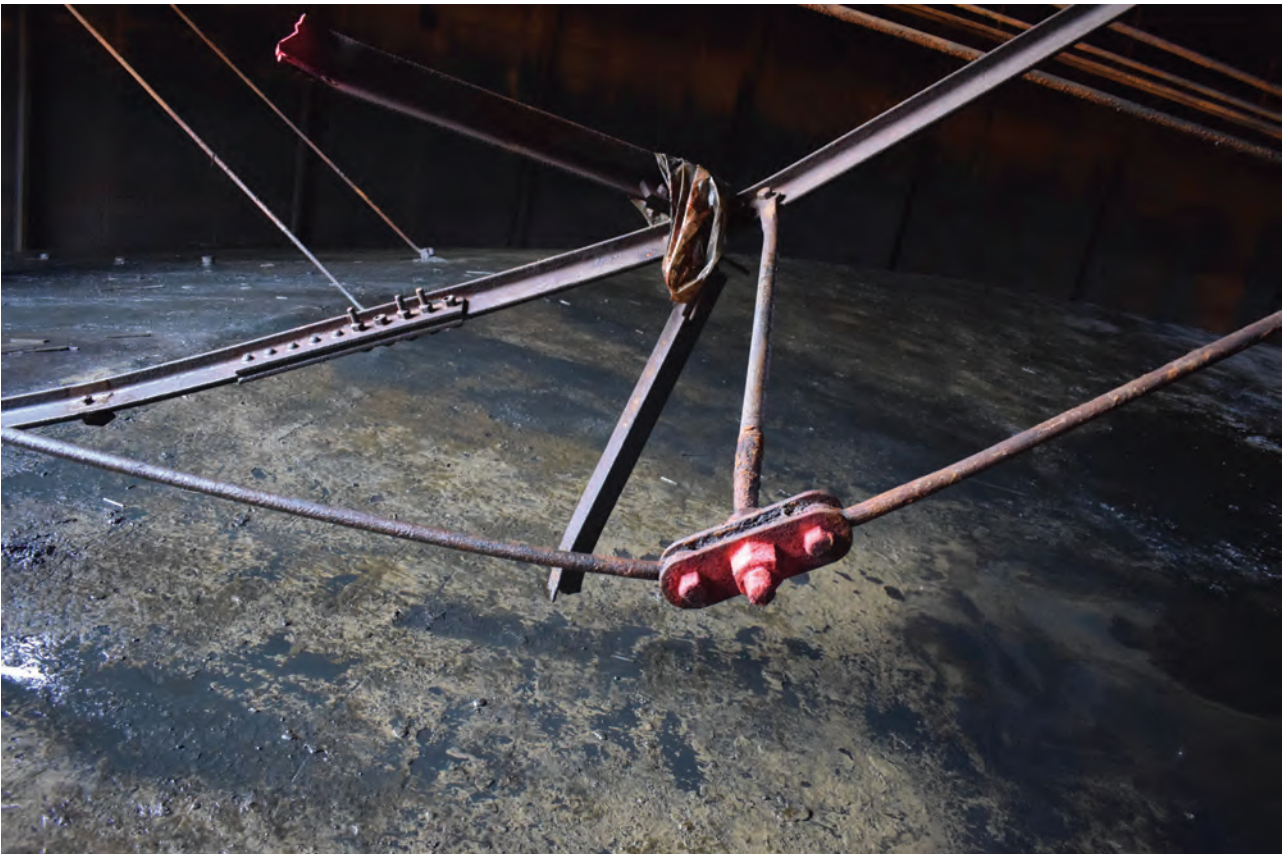
Plate 50: Gasholder No 1, detail view of various bolted joint designs on the truss frame
