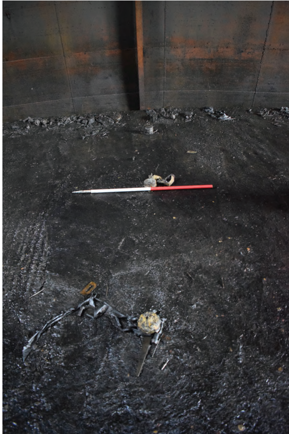
Plate 27: Gasholder No 1, general view of the metal cap line, from the east
