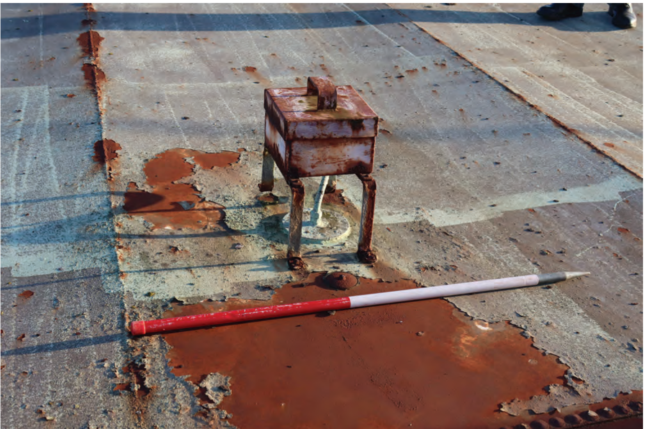
Plate 42: Gasholder No 1, detail view of the glycol pot on the WNW, from the WNW
