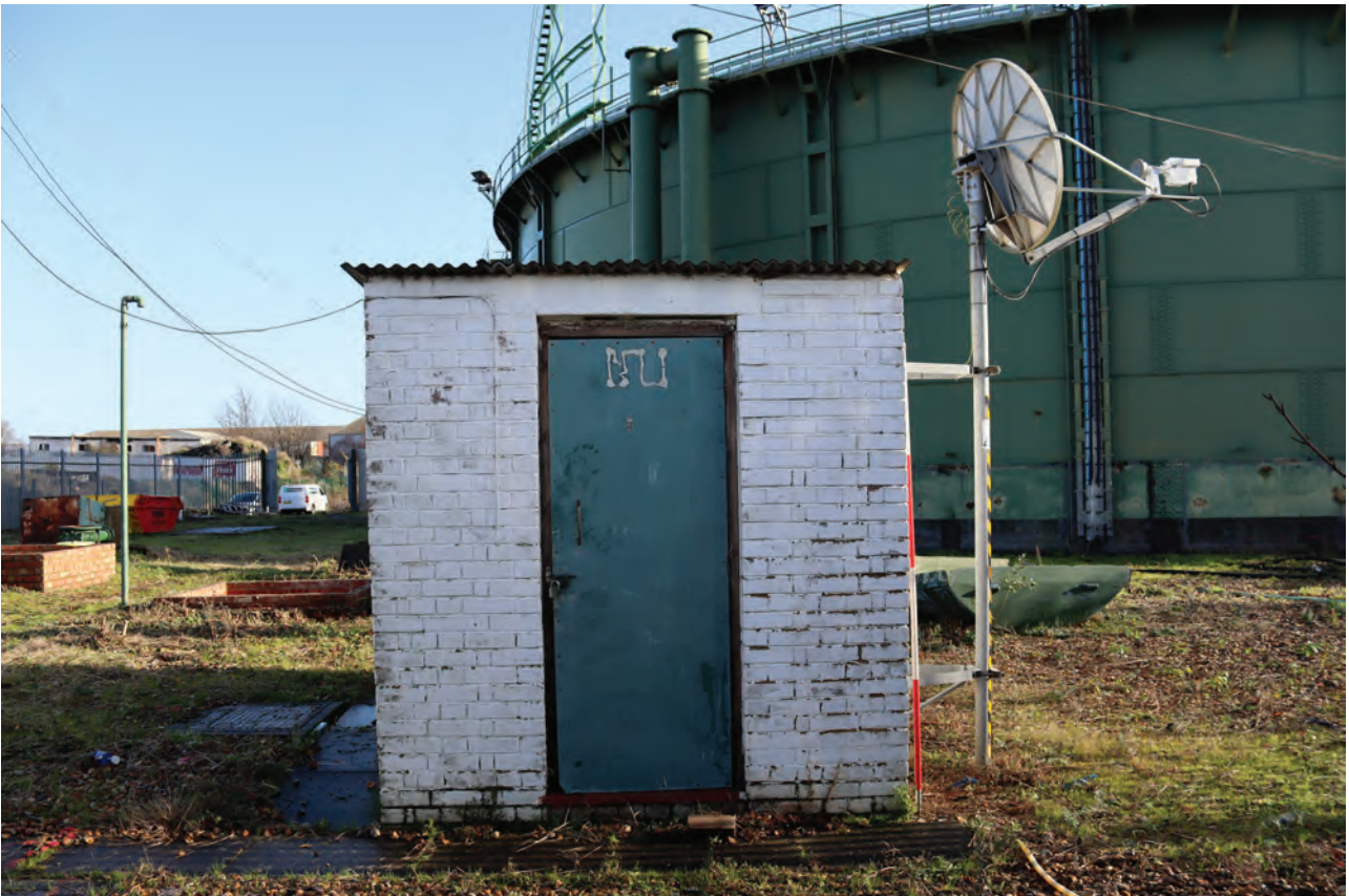
Plate 112: Structure B, general view of the exterior west wall showing entrance door and satellite dish attached to the south wall, from the west
