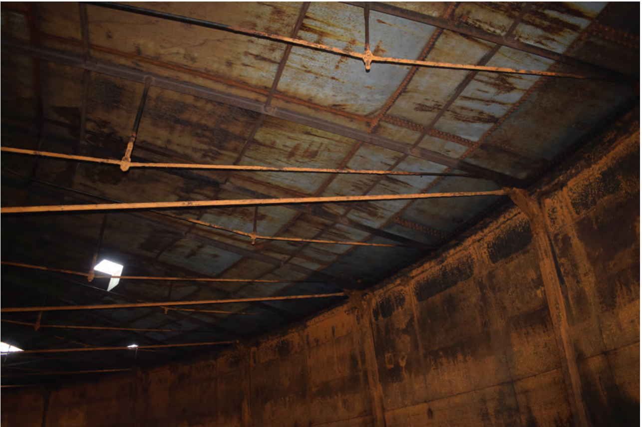
Plate 47: Gasholder No 1, detail view of truss, from the north
