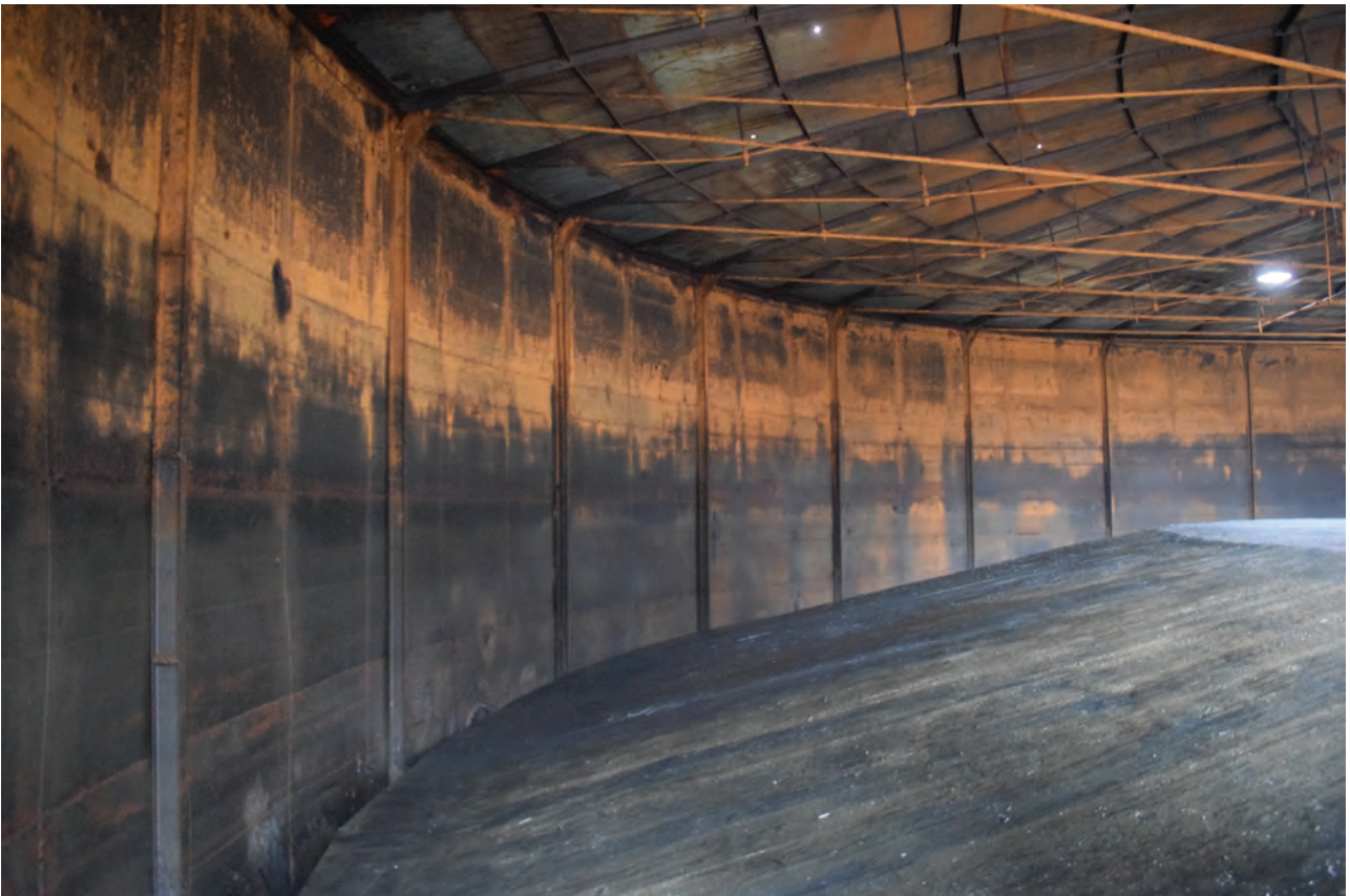
Plate 26: Gasholder No 1, general view of sloped dumpling, from the west
