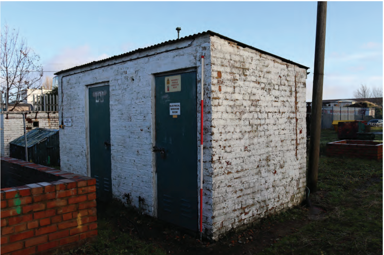
Plate 126: Structure H, general view of the exterior west wall showing entrance doors, from the south-west
