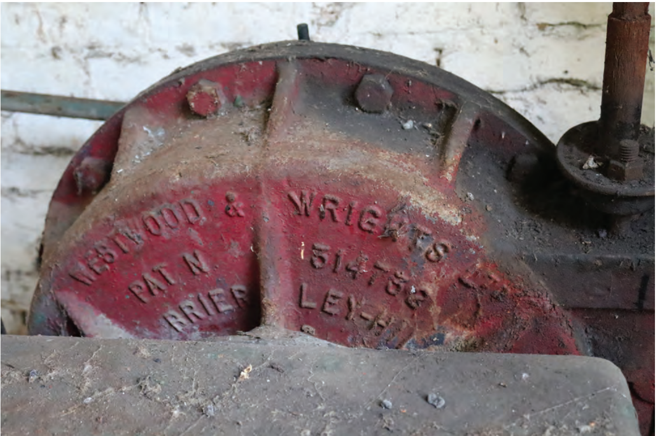
Plate 146: Structure N, detail view of 'WESTWOOD & WRIGHTS LTD' maker's mark on the valve at the west end of the volumetric governor house, from the east
