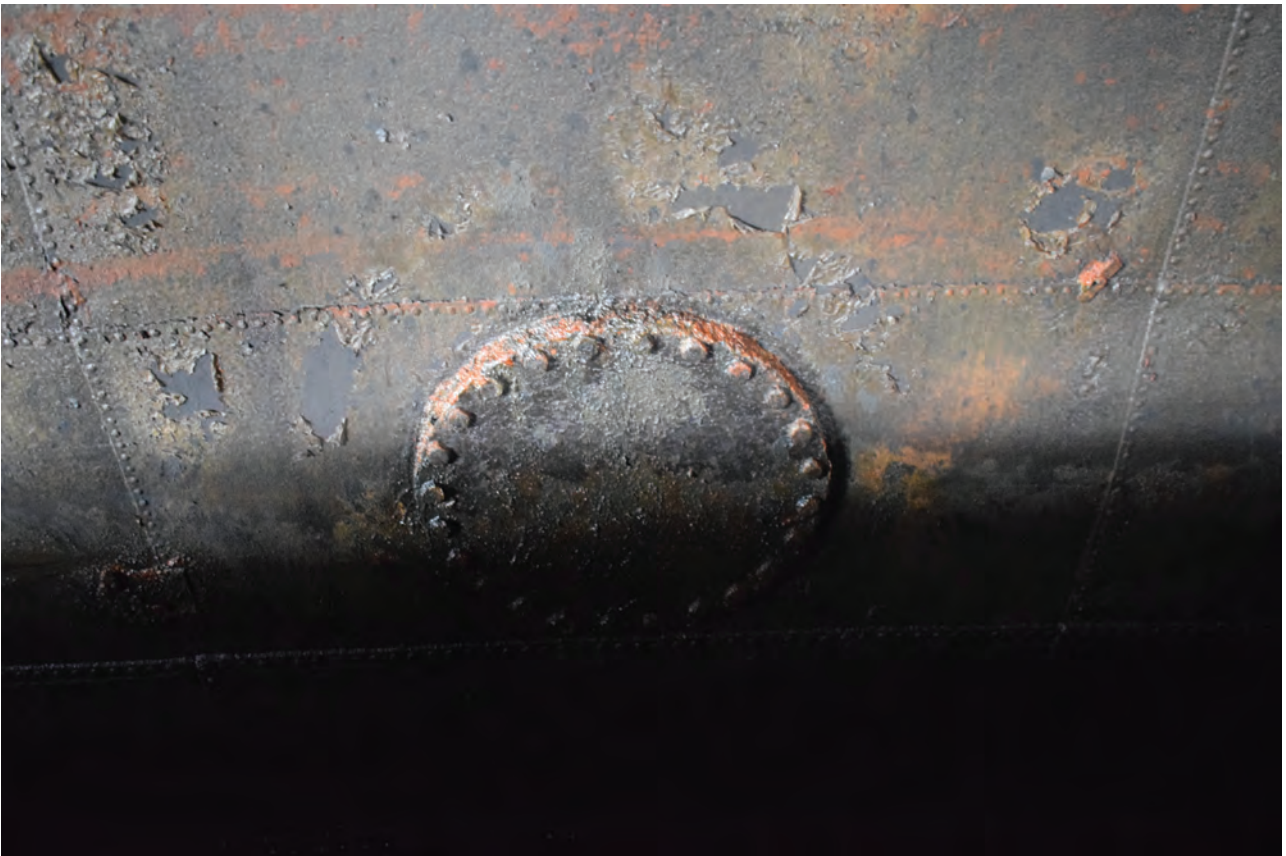
Plate 32: Gasholder No 1, detail view of cotter plate on the north-east side of the top lift wall interior, from the south-west
