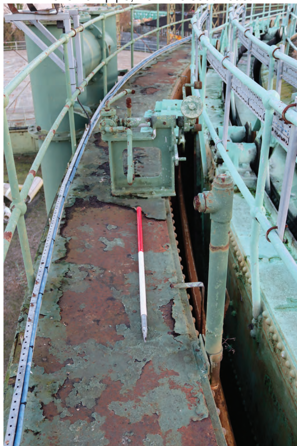
Plate 106: Gasholder No 2, detail view of oil pipe, from the west
