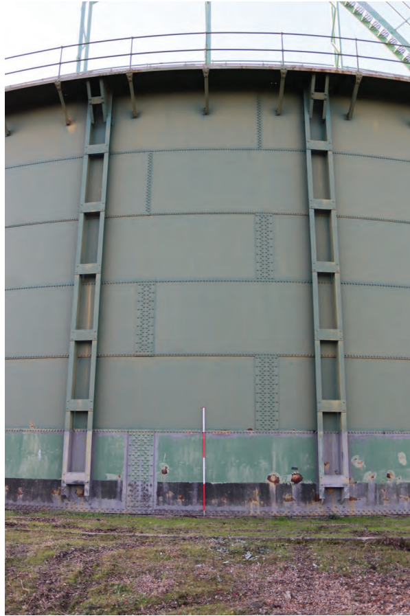
Plate 73: Gasholder No 2, detail view of tank sheet construction, from the east
