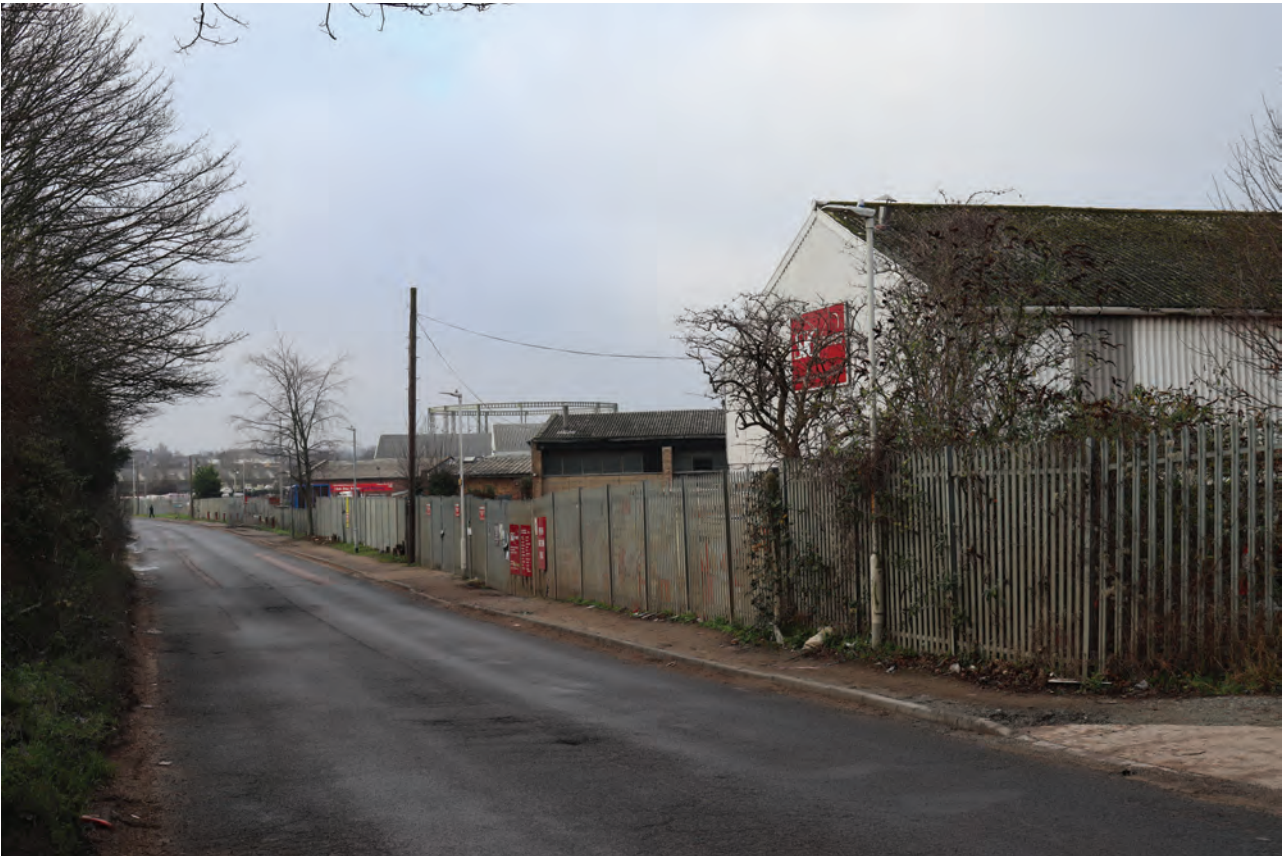
Plate 3: Gasholder No 1, unobtrusive in the flat landscape due to large, light industrial buildings, from the ESE
