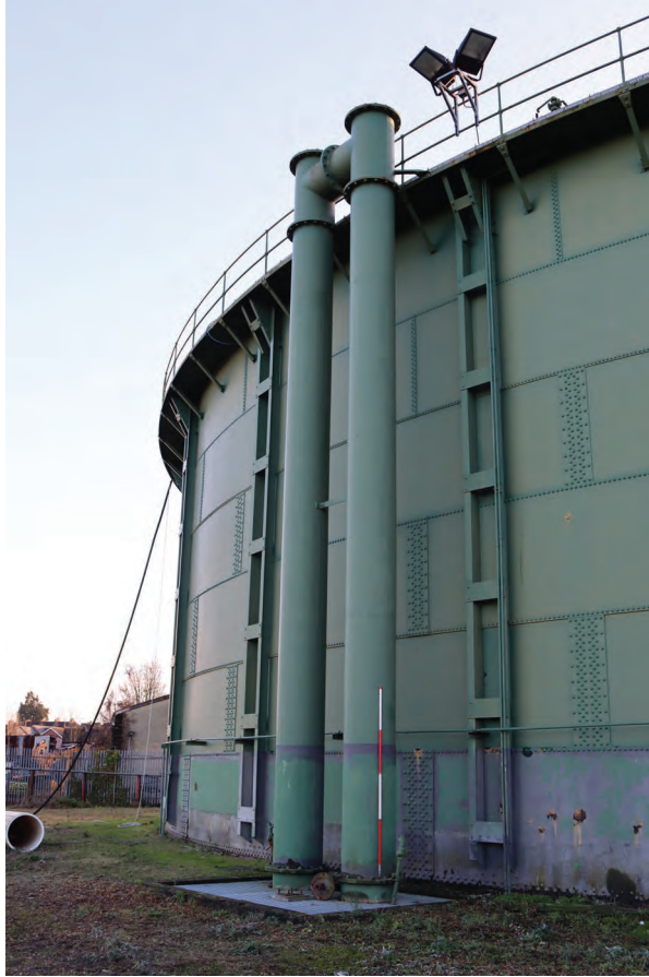
Plate 91: Gasholder No 2, general view of the gas outlet pipe on the north-east side of the holder, from the north-west
