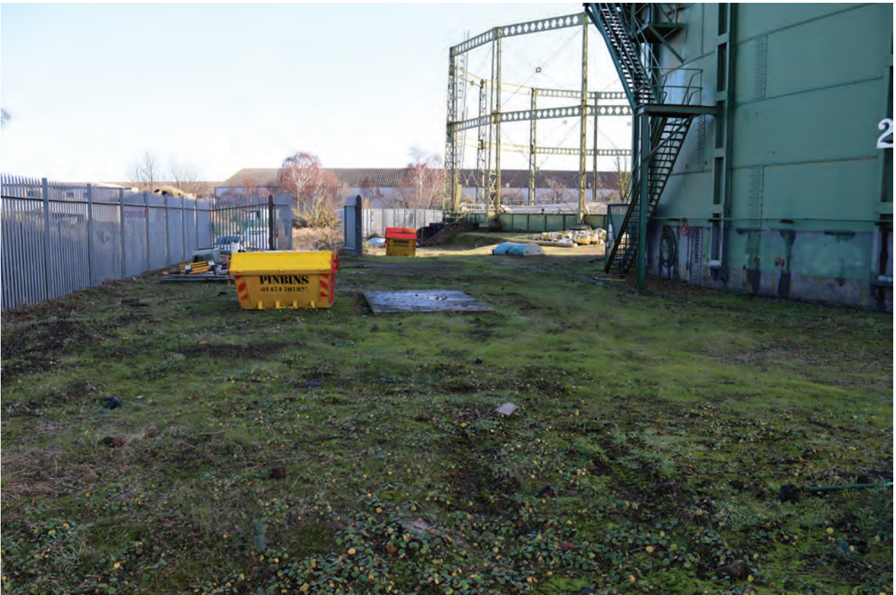
Plate 150: Structure R, general view of the open area in the north of the site with concrete platform Structure R in the centre, from the west
