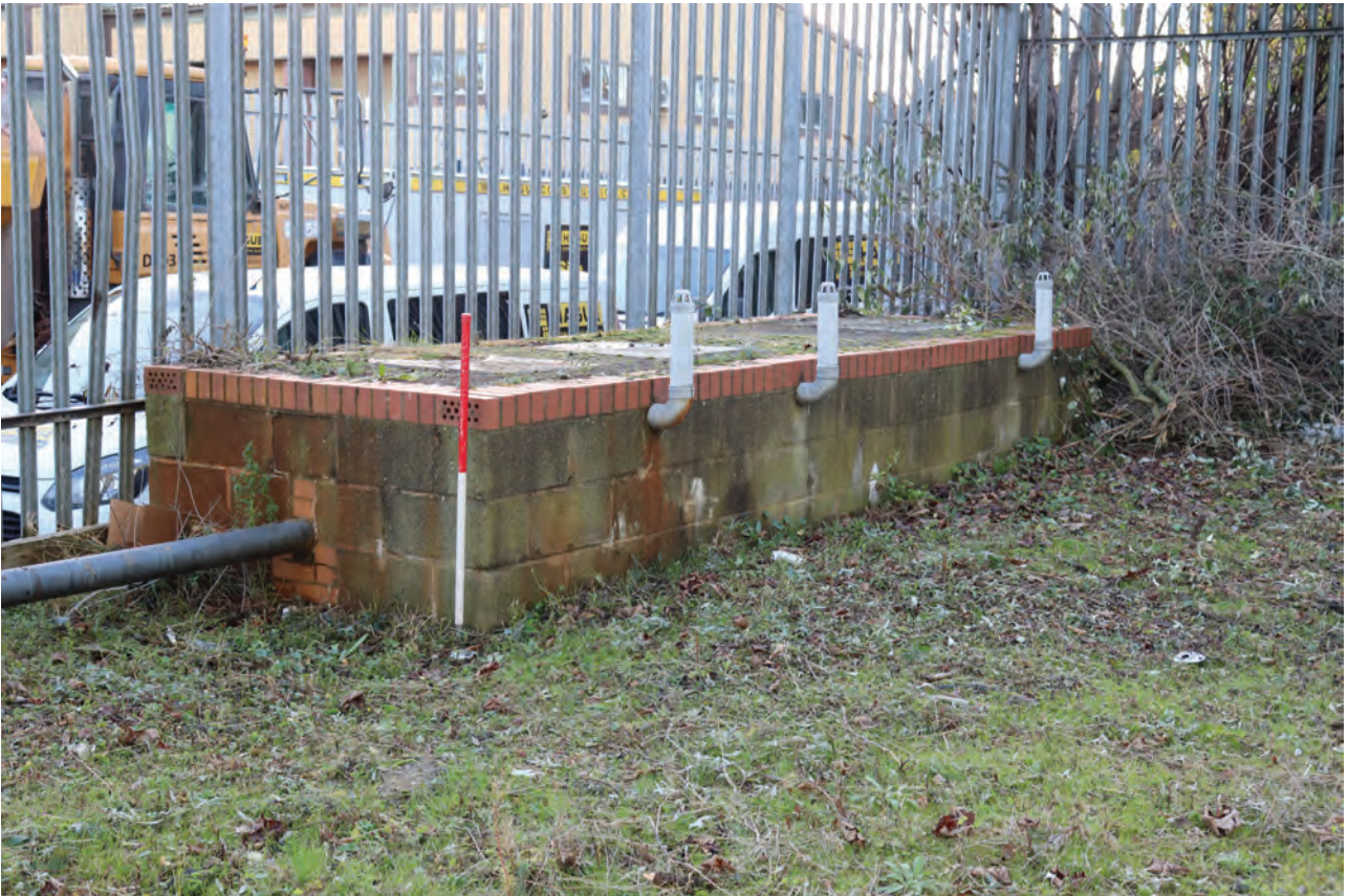
Plate 67: Gasholders Nos 1 & 2, general view of the interceptor tank, from the north-east
