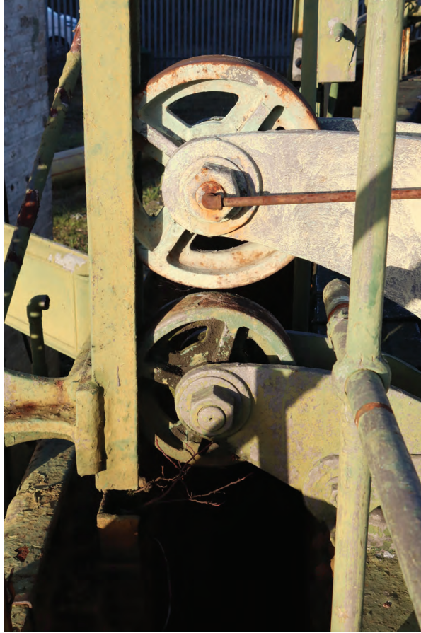
Plate 35: Gasholder No 1, detail view of guide rollers at standard 12, from the south
