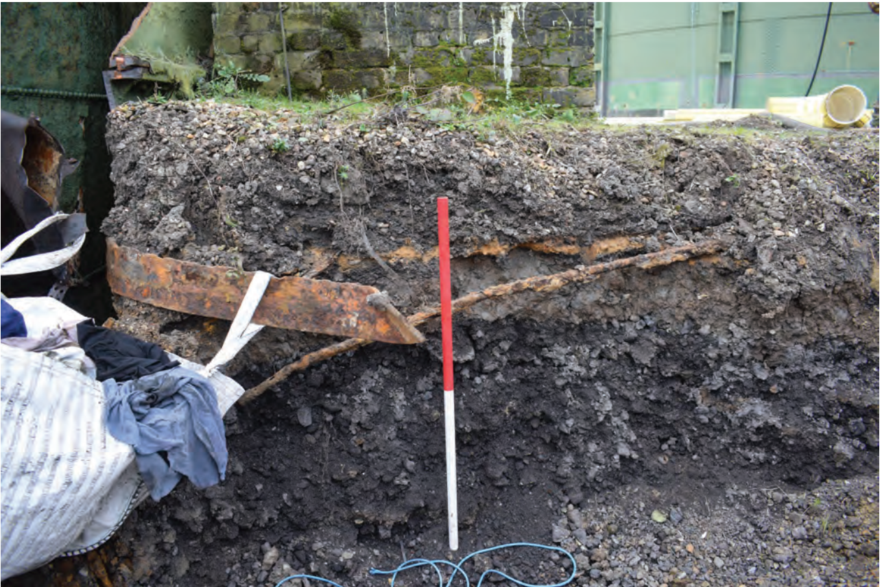
Plate 23: Gasholder No 1, detail view of section through made-ground showing broken wrought iron bands helping secure the tank, from the north-east
