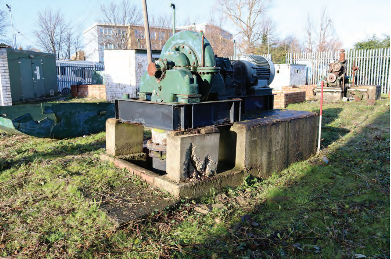
Plate 117: Structure C, general view of booster motor, from the south-east
