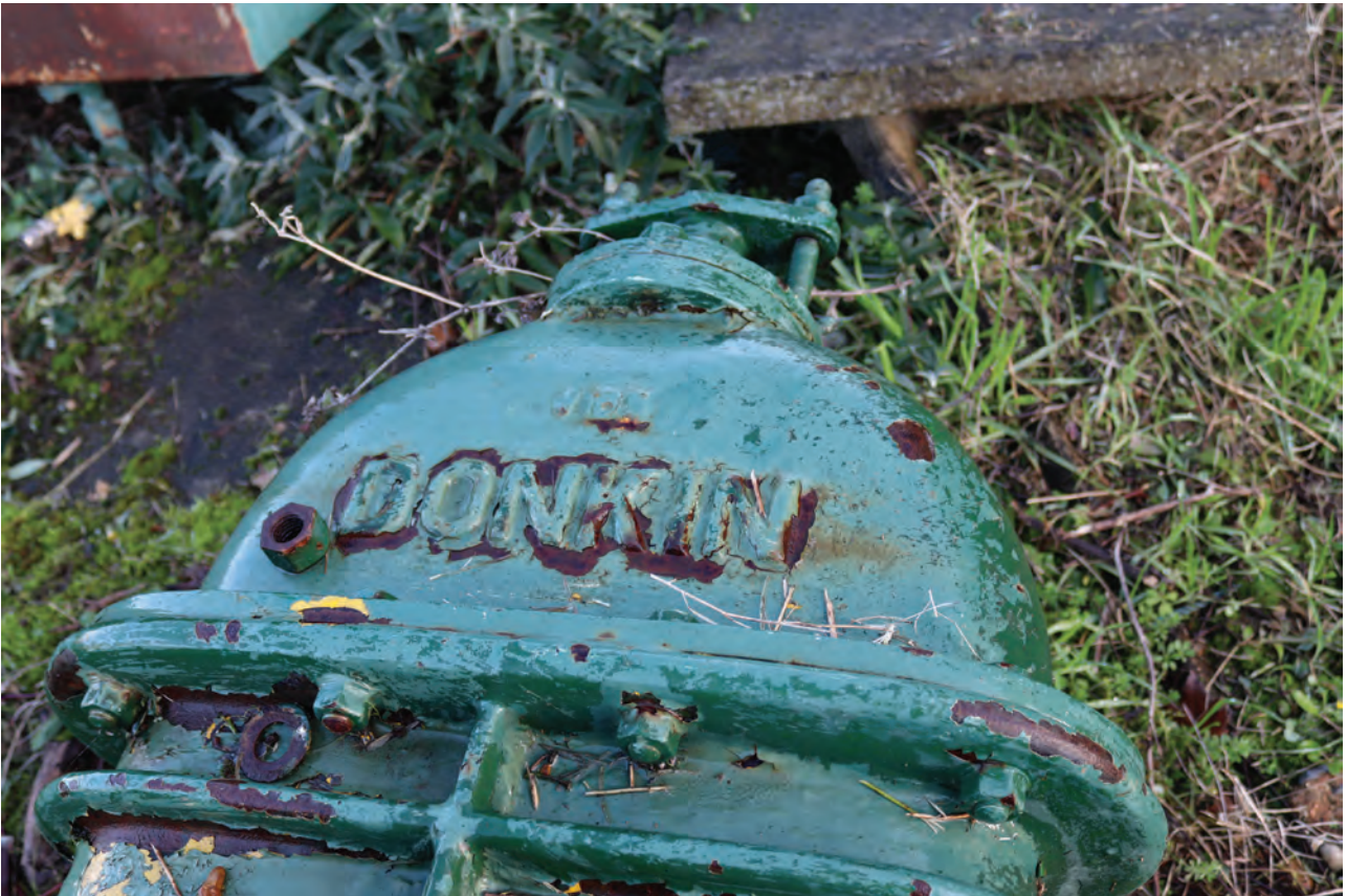
Plate 149: Structure Q, detail view of 'DONKIN' maker's mark on the gate valve, from the WSW
