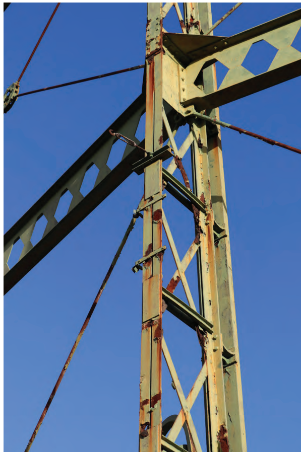
Plate 70: Gasholder No 1, detail view of hook as part of a winch system on standard 12, from the WSW
