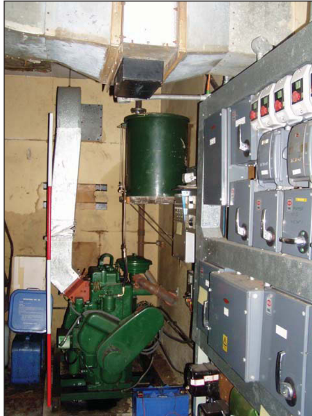
Plate 3: Plant Room 3, Diesel generator
