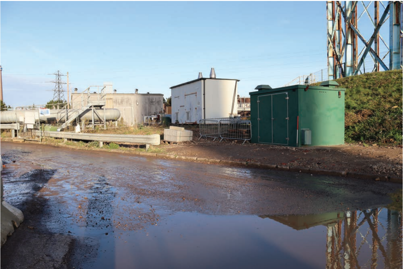
Plate 11: General view of structures in the centre of the site to the south of Gasholder No 5, from the south-east
