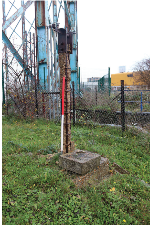
Plate 155: Gasholder No 5, detail view of removed equipment setting, from the south-west
