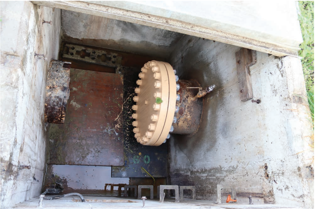
Plate 209: Valve pits, detail view of blanked pipe, from the WNW
