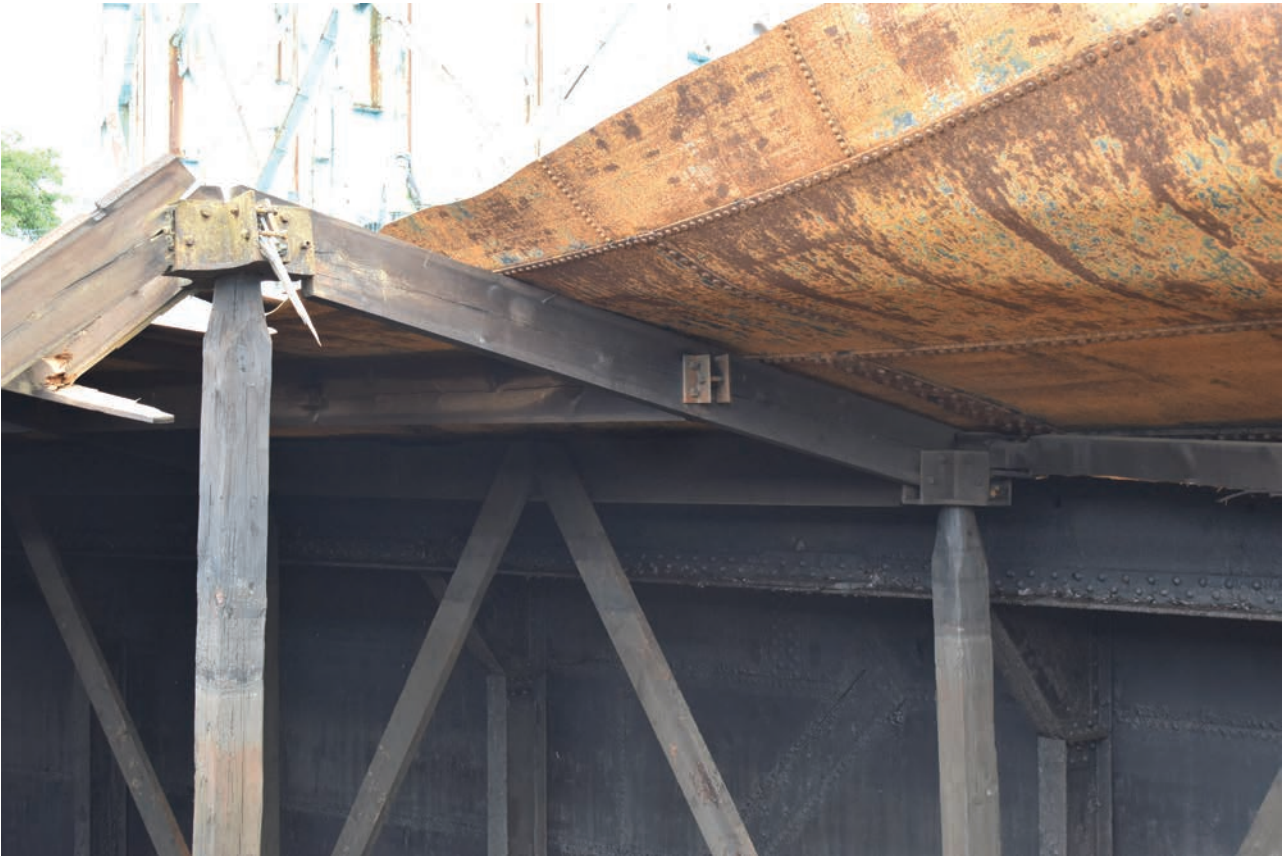
Plate 29: Gasholder No 4, detail view of pointed post tops slotted into cross-shaped fixtures, from the south-east
