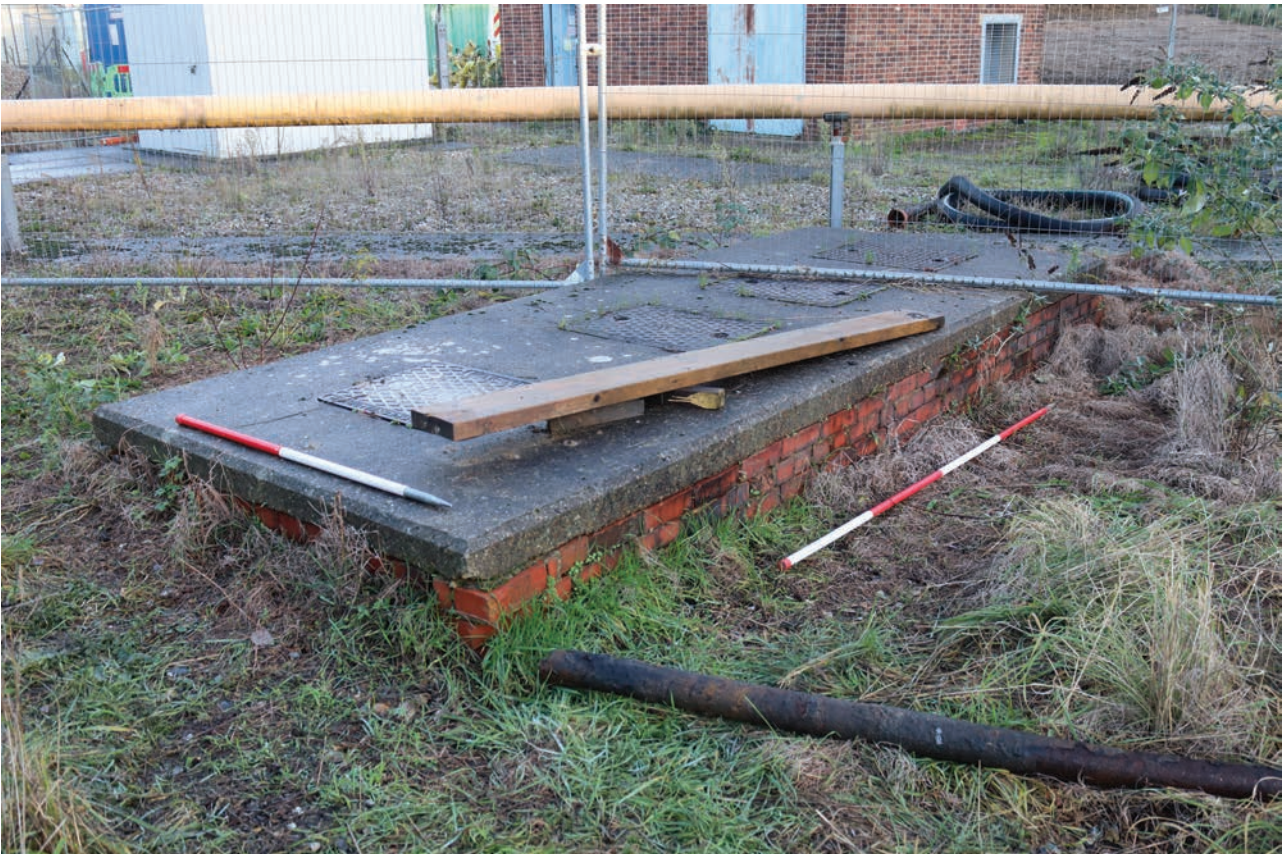
Plate 212: Interceptor tank, general view, from the south-east
