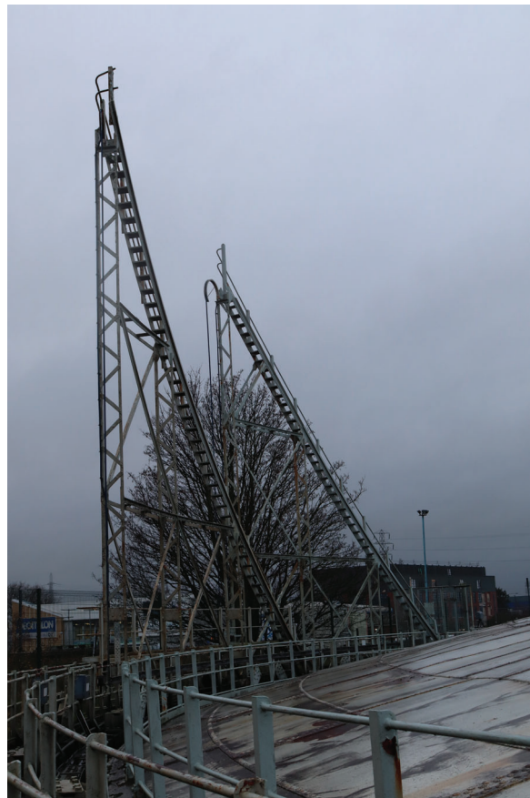
Plate 44: Gasholder No 4, general view of the guide rail and stair structures on the south-west side of the holder, from the east
