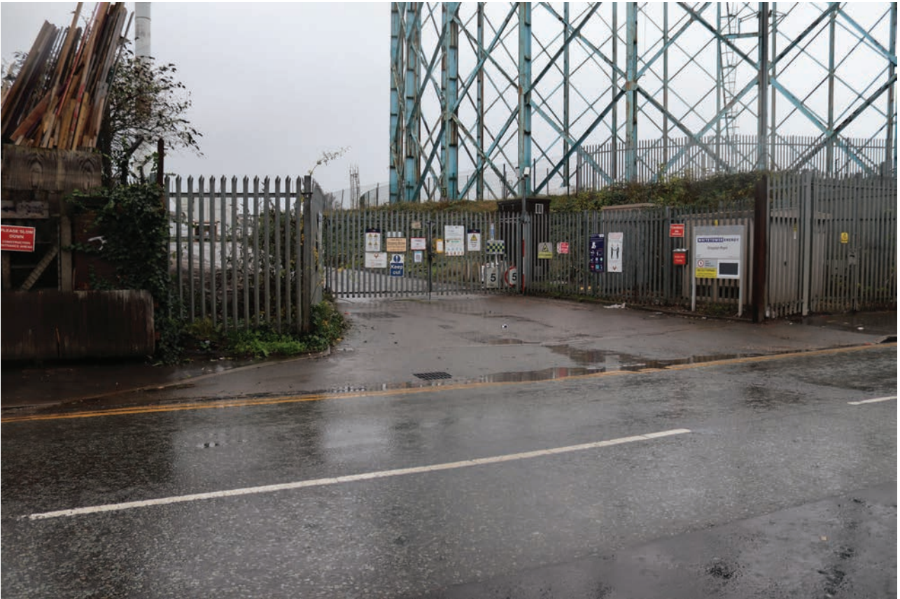
Plate 7: General view of the compound entrance on Factory Lane, from the north-east
