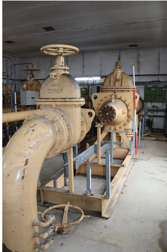
Plate 161: Structure 1, blanked pipework within the District Governor House, from the north-east
