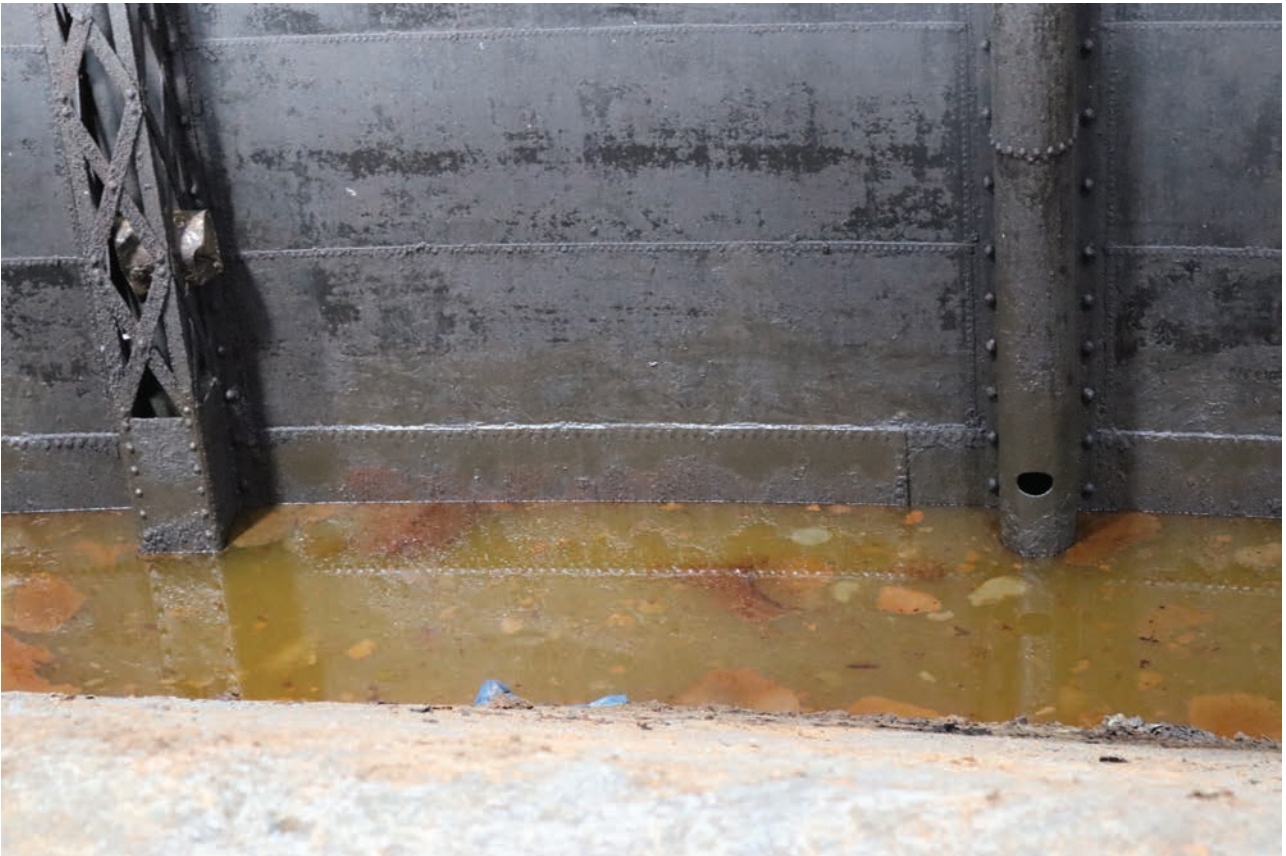
Plate 115: Gasholder No 5, detail view of latticework design and hole in the column support for releasing tank water easily, from the north-east
