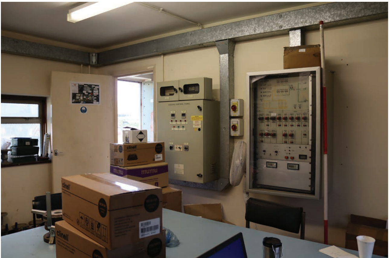
Plate 172: Structure 3, general view of monitoring and control panels including for the fogger system within the Control Room, from the east
