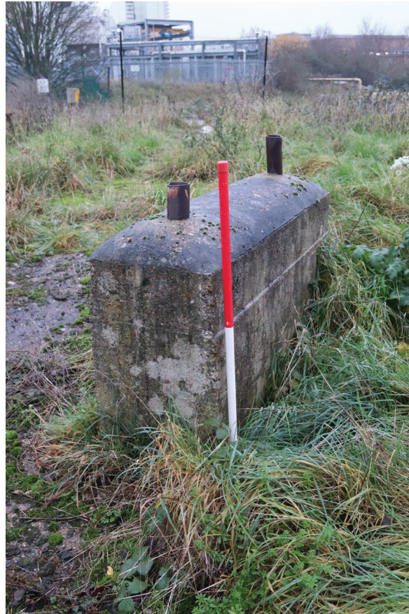
Plate 157: Gasholder No 5, detail view of cut-off steel bars, from the north
