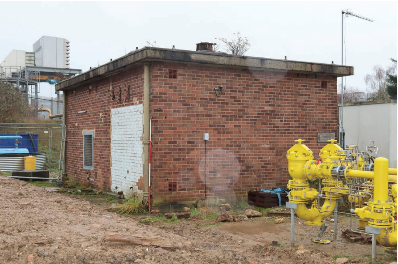
Plate 174: Structure 4, general view of the Switch Room exterior, from the north
