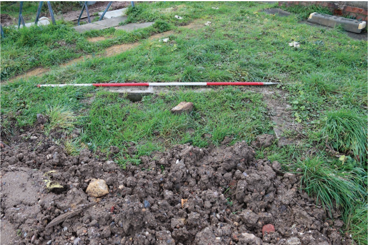
Plate 206: Valve pits, detail view of previously filled in pit, from the ENE
