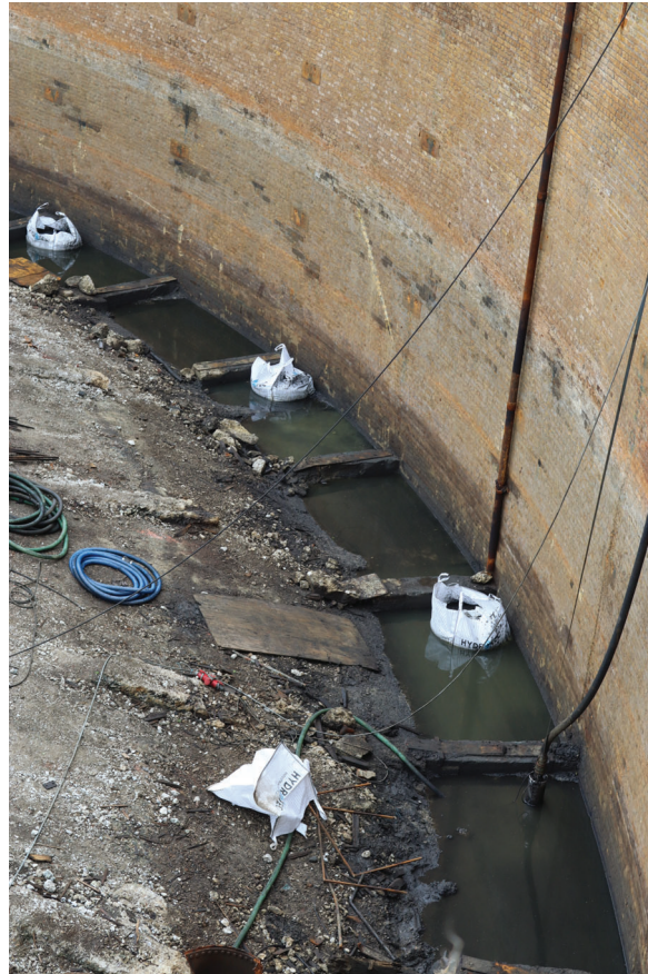
Plate 21: Gasholder No 4, detail view of the concrete blocks supporting the lift grips, from the WNW
