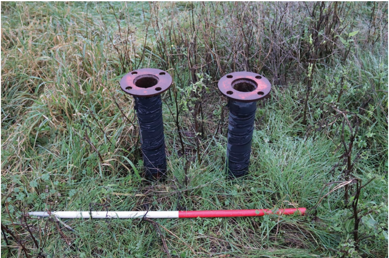
Plate 156: Gasholder No 5, detail view of removed equipment setting, from the north
