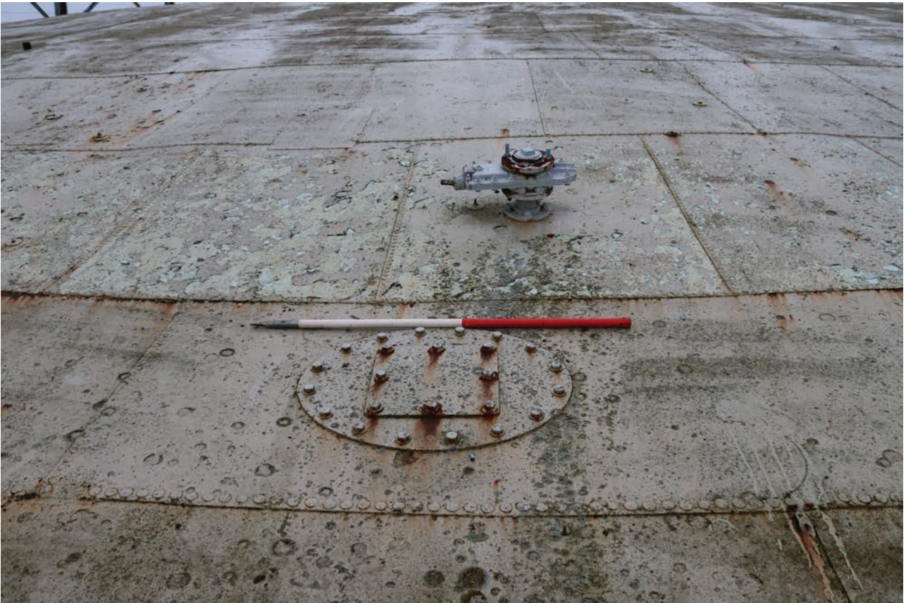
Plate 127: Gasholder No 5, detail view of crown vent and cotter plate on the south-west edge of the crown, from the south-west
