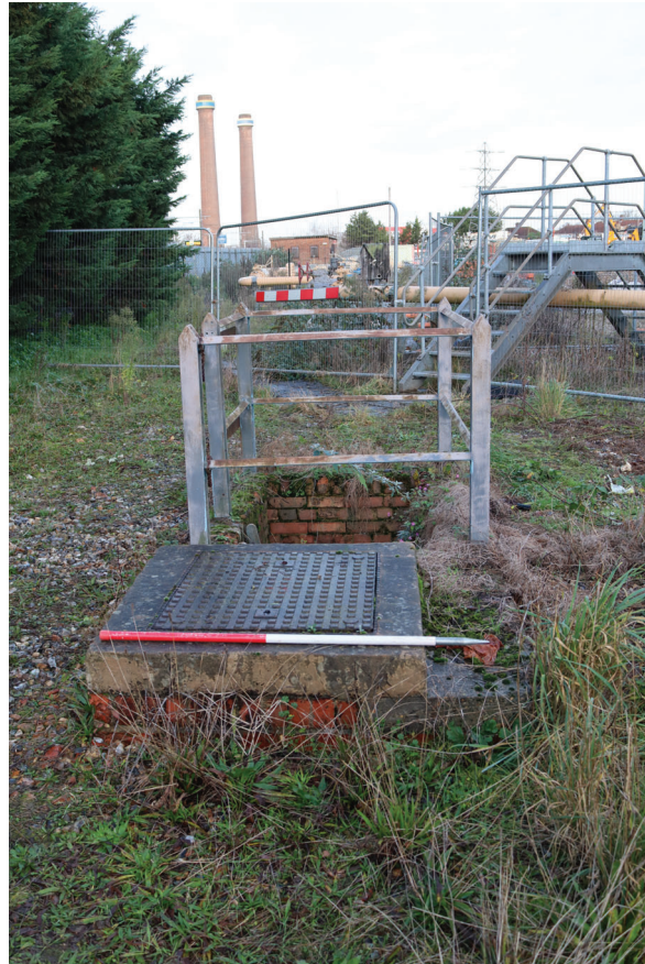
Plate 213: Interceptor tank, general view, from the south-east
