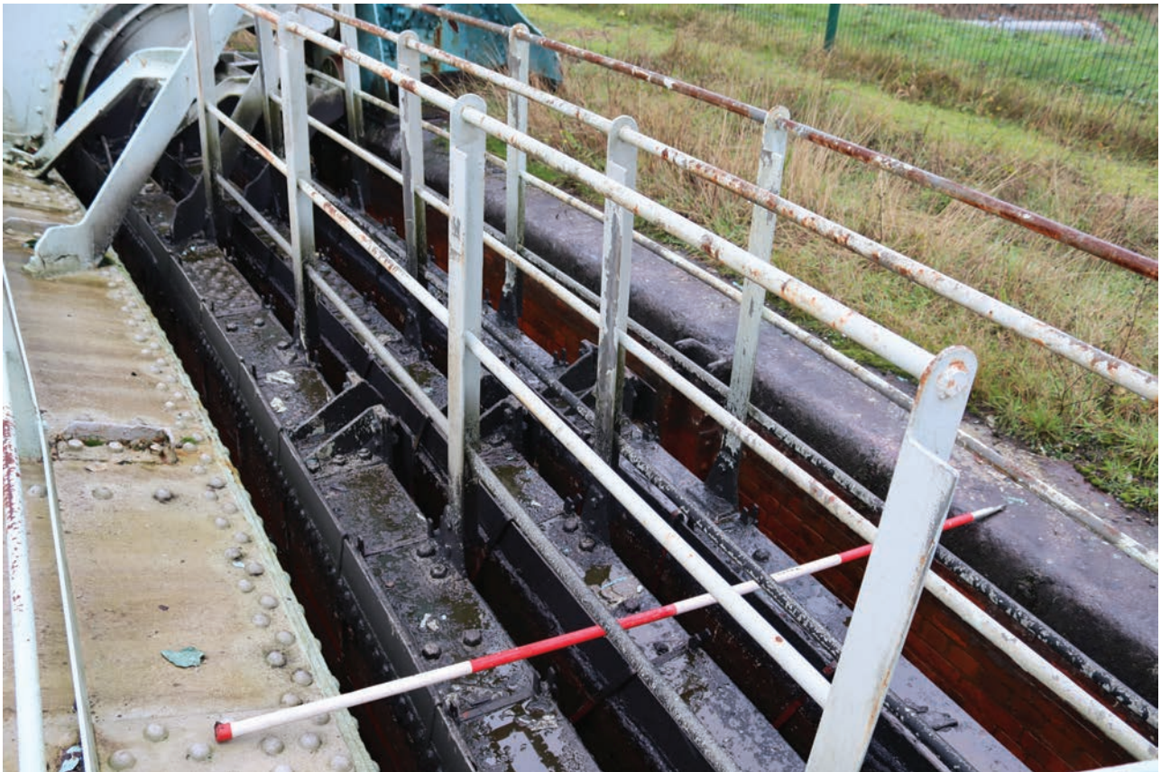
Plate 112: Gasholder No 5, general view of lift tops showing square grips, from the ENE
