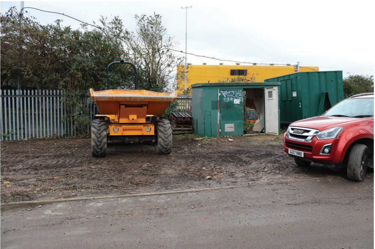
Plate 186: Structures 10c and 10d, general view of disused governor houses, from the north-west
