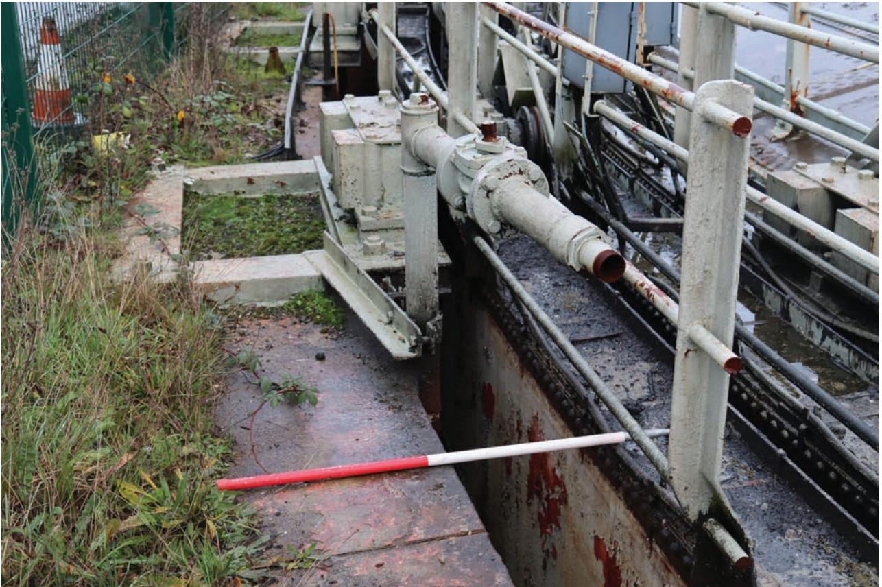
Plate 67: Gasholder No 4, detail view of oil maintenance pipe, from the WSW
