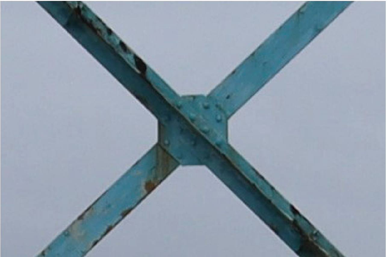
Plate 105: Gasholder No 5, detail view of hexagonal plate riveted at the centre of each strut, from the south
