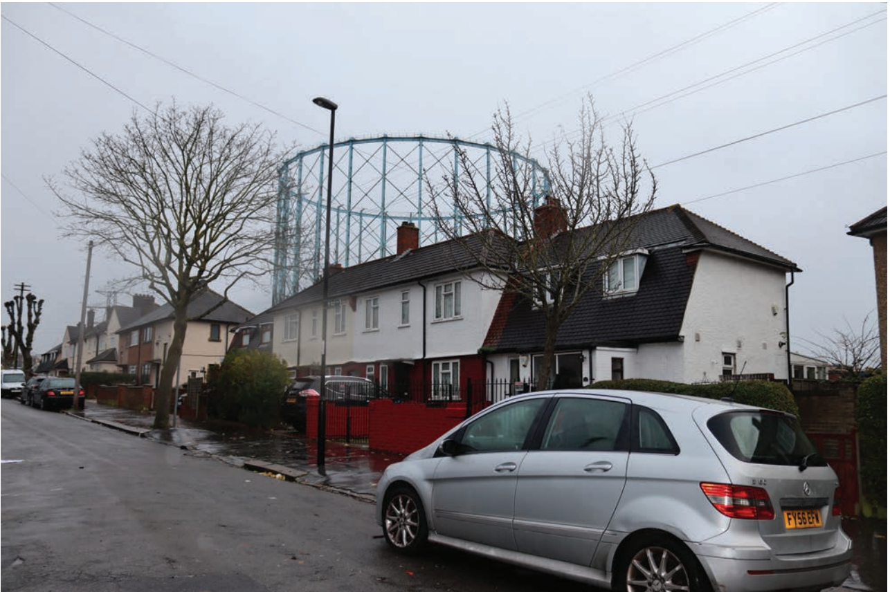
Plate 3: General view of the site from Martin Crescent to the north-west, from the WNW
