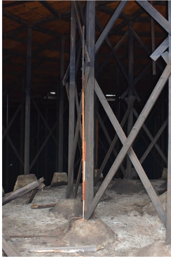
Plate 69: Gasholder No 4, detail view of narrow pipe attached to a vertical post of the crown support frame, from the north-west
