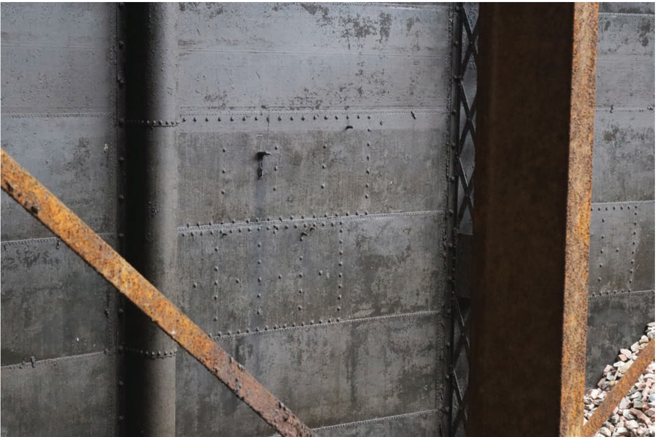
Plate 118: Gasholder No 5, detail view of unidentified use bolt arrangements on the north-east side of the top lift wall interior base, from the WSW
