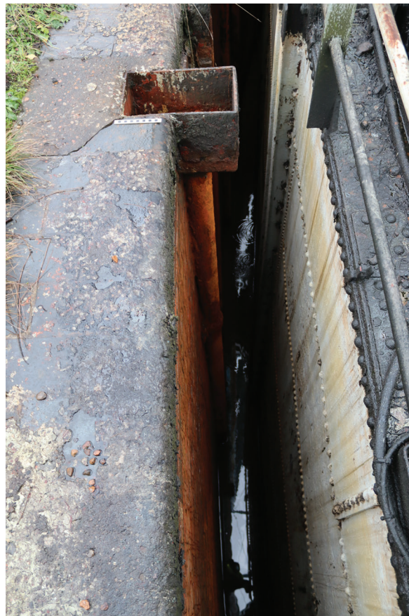
Plate 150: Gasholder No 5, detail view of possible water discharge point between standards 25 and 26, from the ENE
