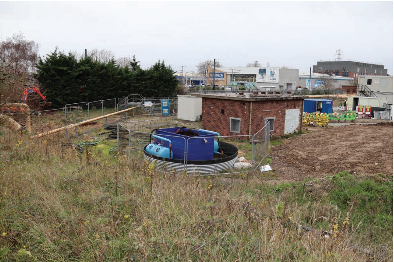
Plate 10: General view of structures on the south-west site boundary, from the ENE
