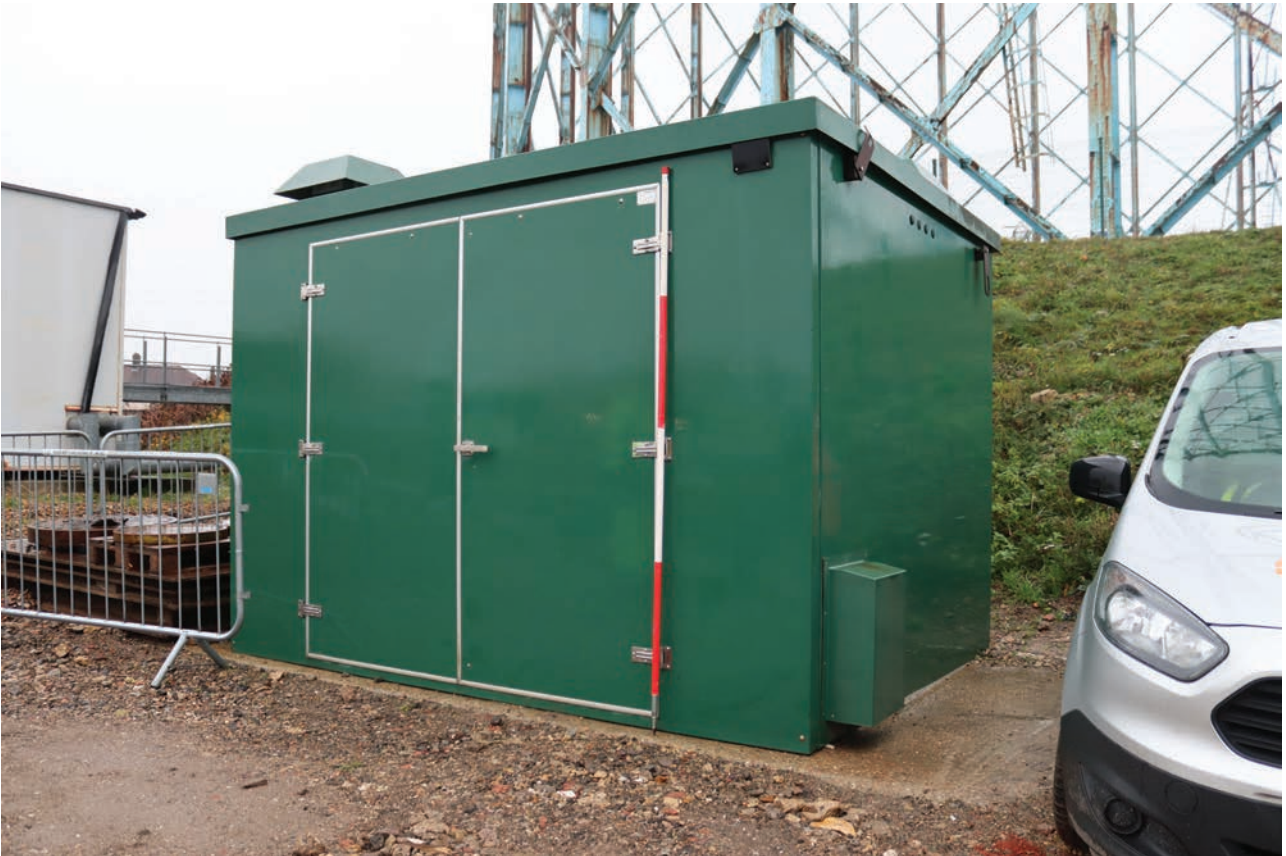
Plate 187: Structure 10e, general view of disused governor house, from the south-east
