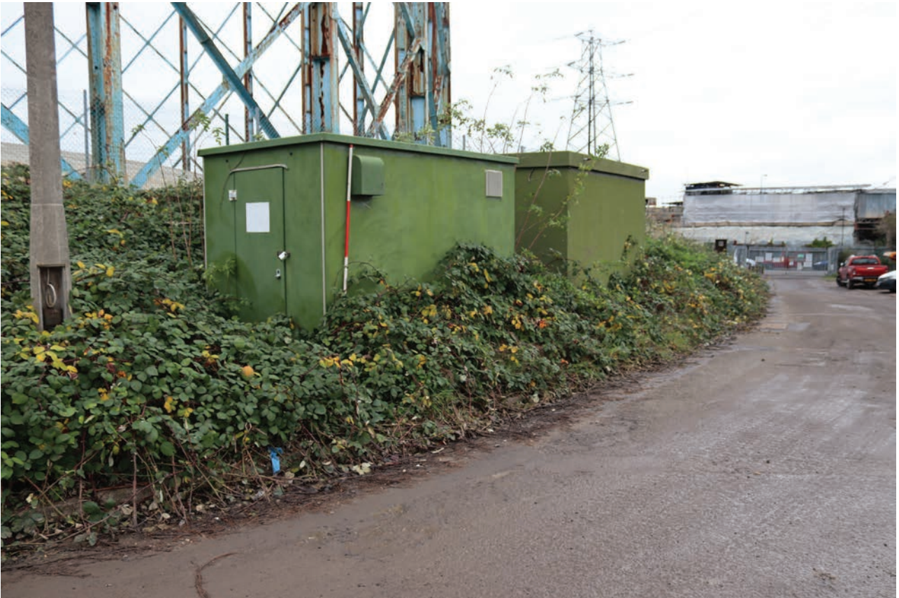
Plate 185: Structures 10a & 10b, general view of disused governor house, from the south
