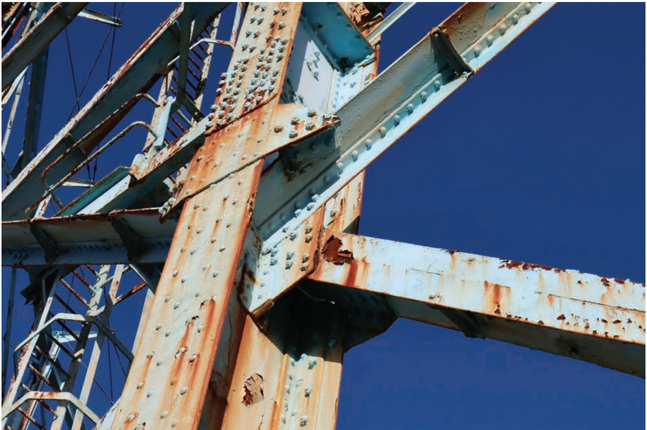
Plate 102: Gasholder No 5, detail view of gusset plates on the exterior side and middle of standard 4, from the south
