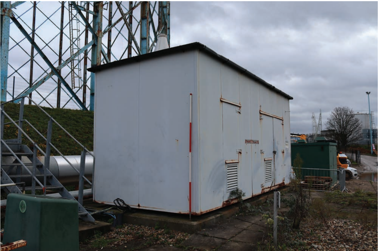
Plate 164: Structure 1, general view of the Boiler House (Structure 2), from the west
