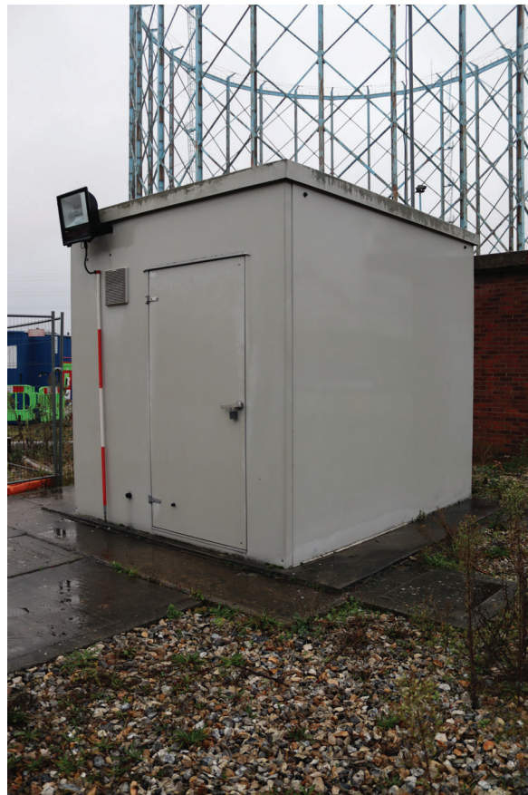
Plate 184: Structure 9, general view of unidentified building, from the south
