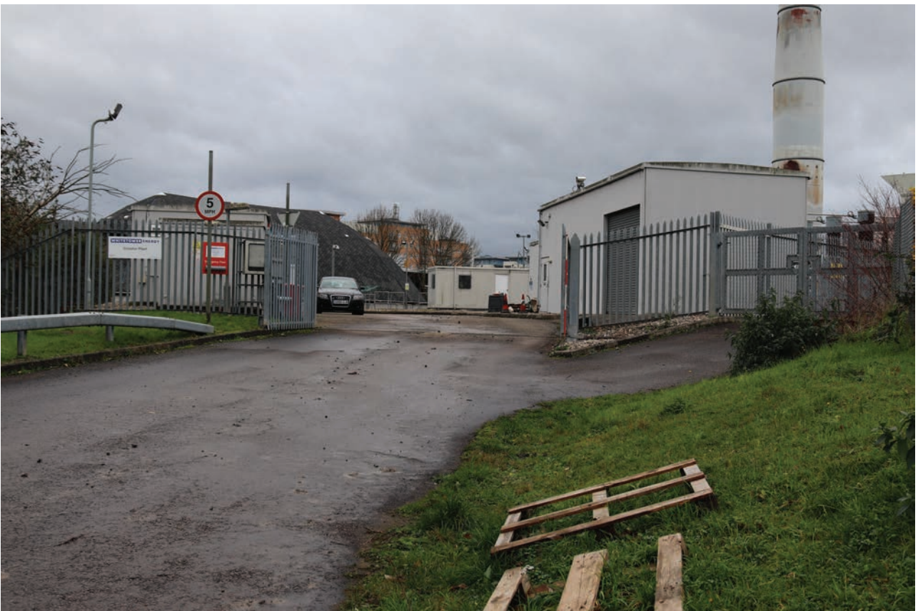
Plate 8: General view of the entrance to Whitetower Energy Croydon Plant in the south-east corner of the site, from the NNW
