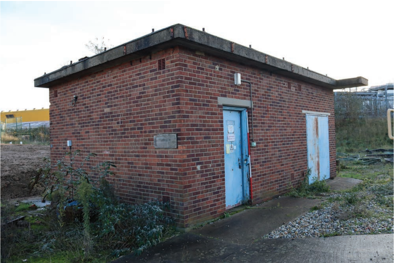
Plate 173: Structure 4, general view of the Switch Room exterior, from the west
