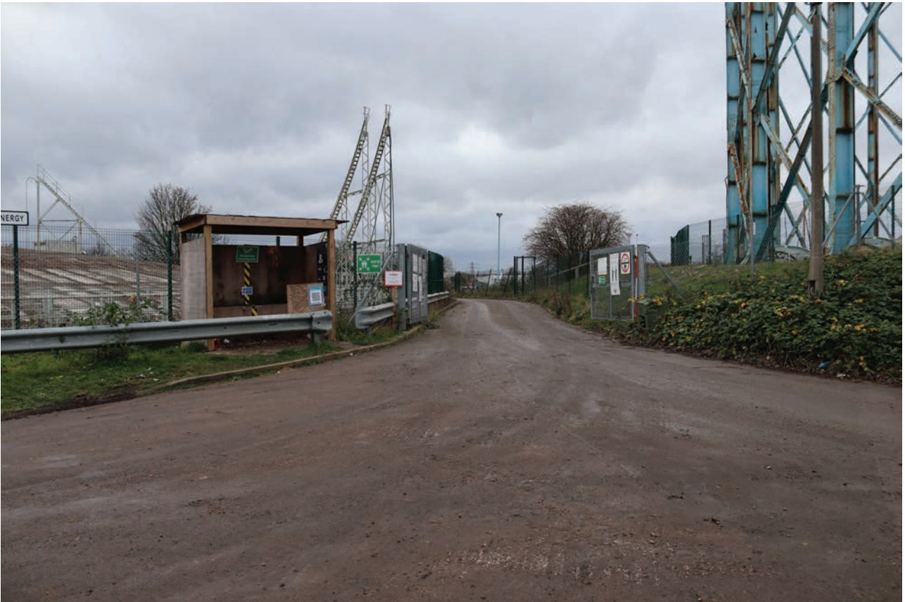
Plate 9: General view of the site road with gate entry between Gasholders Nos 4 and 5, from the north-east
