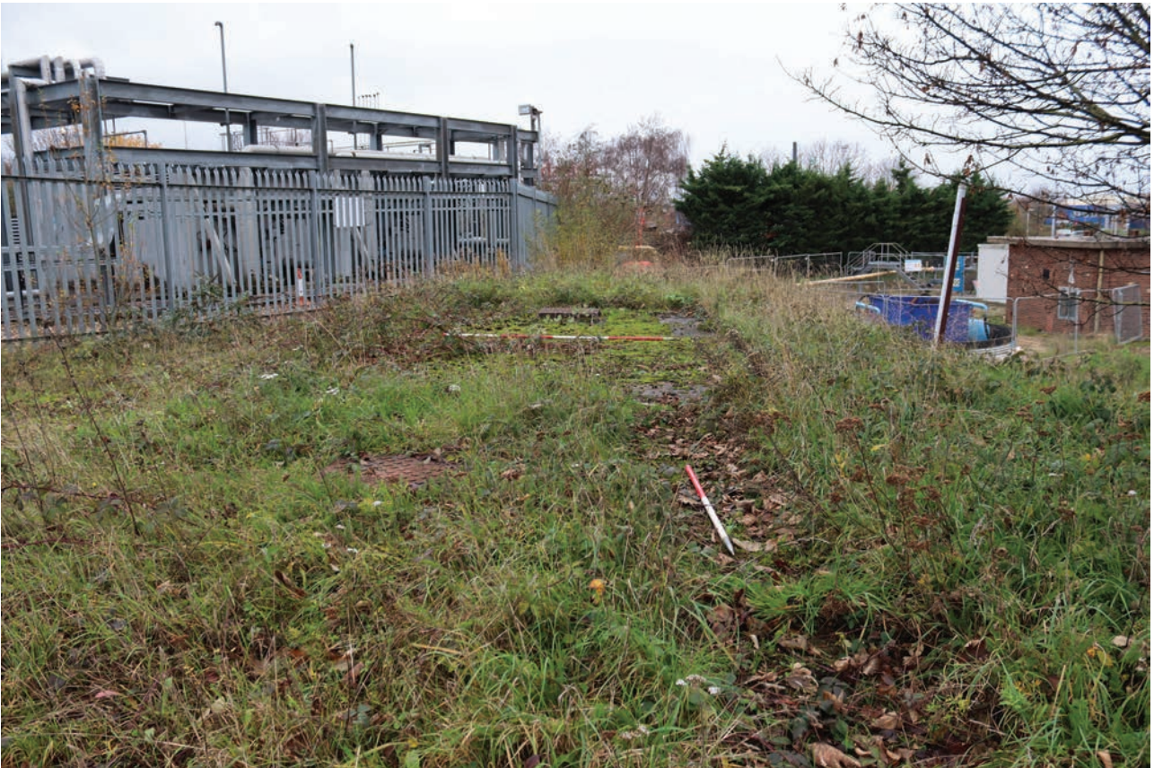
Plate 71: Gasholder No 4, detail view of interceptor tank, from the north-east
