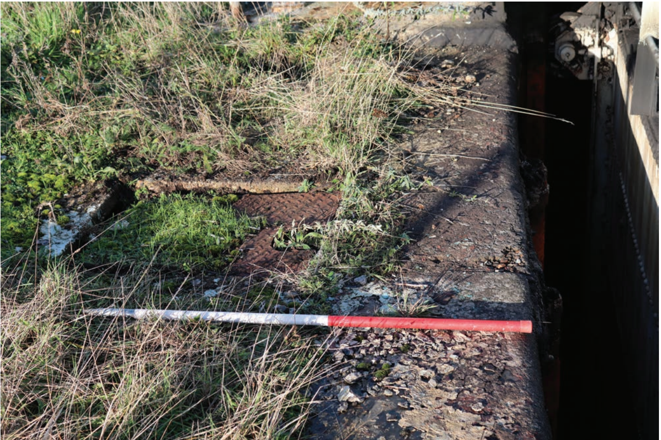
Plate 151: Gasholder No 5, detail view of valve pit between standards 6 and 7, from the south
