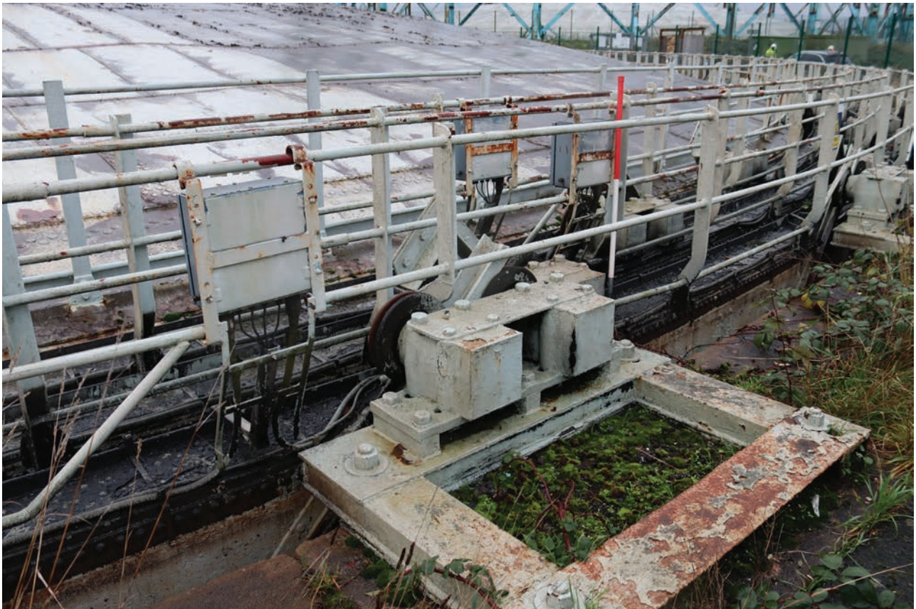
Plate 64: Gasholder No 4, detail view of electrical boxes attached to the handrails, from the ESE
