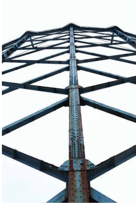
Plate 101: Gasholder No 5, detail view of bolted flange plates and riveted gusset plates on the entire exterior side of standard 12, from the NNW
