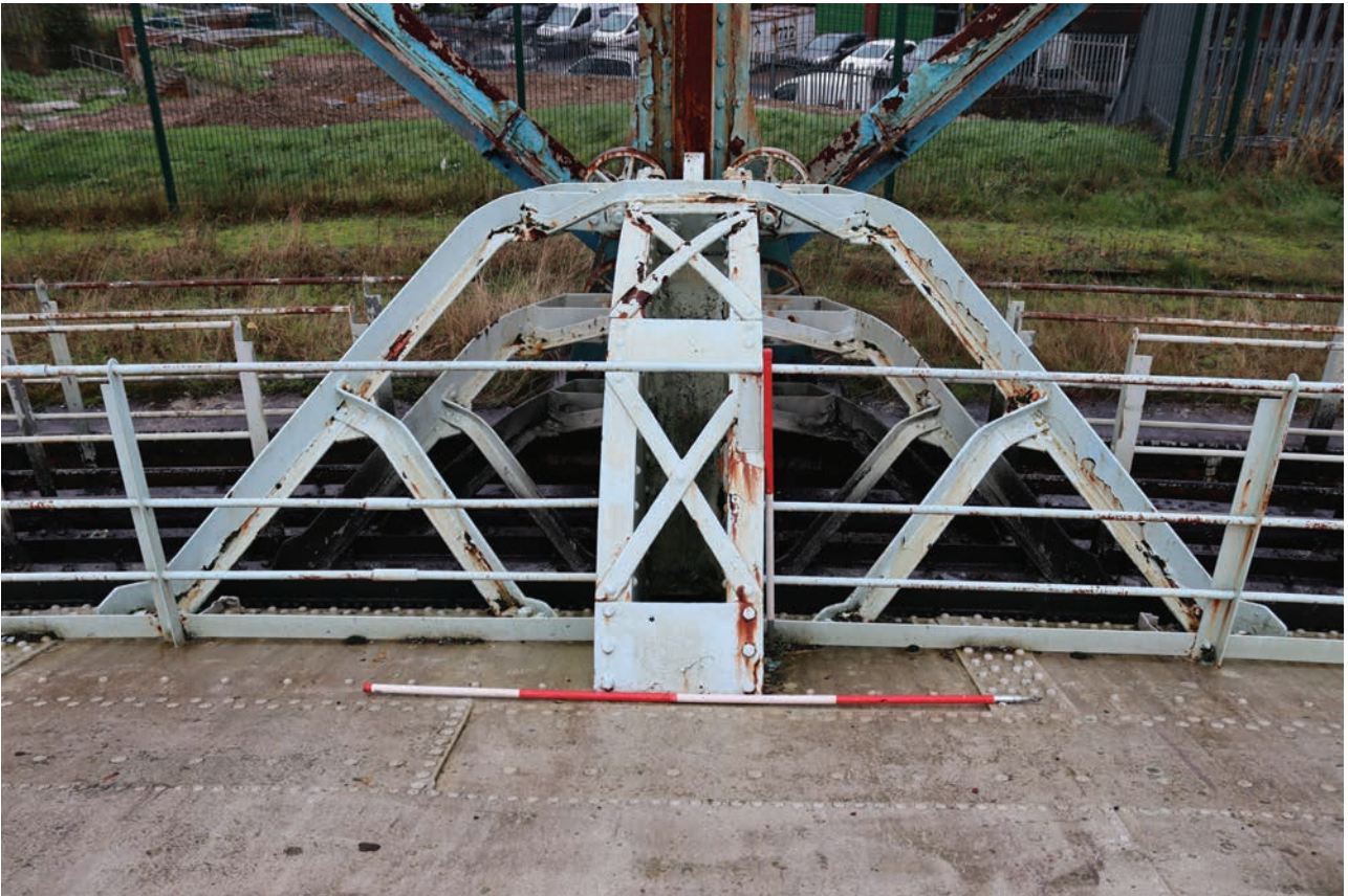
Plate 109: Gasholder No 5, detail view of the roller carriages with cross braces and splaying arms at standard 11, from the south-east
