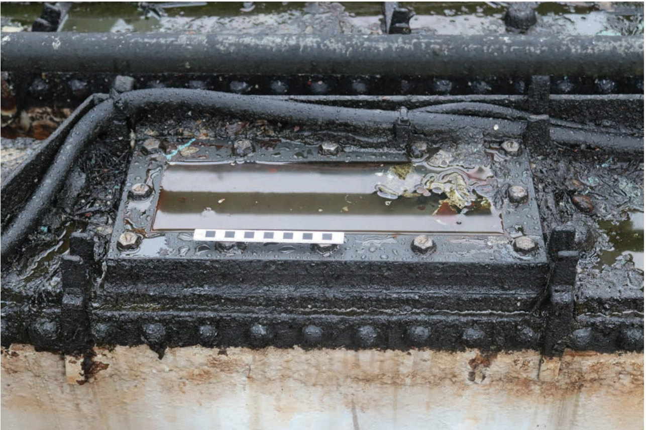
Plate 121: Gasholder No 5, detail view of cup-and-grip viewing window, from the east
