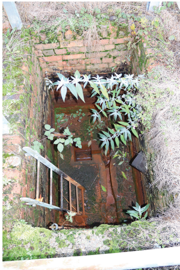
Plate 214: Interceptor tank, detail view, from the south-east
