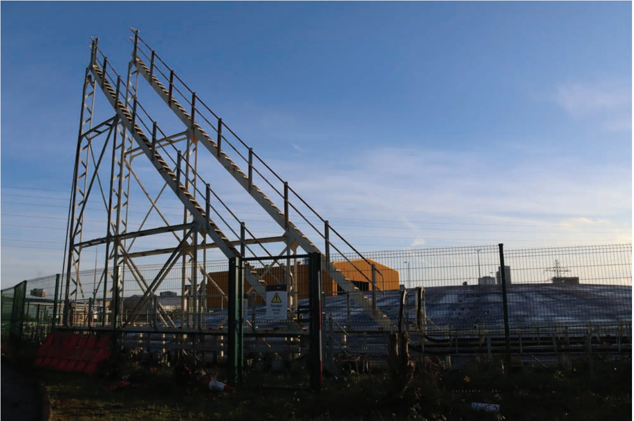
Plate 17: Gasholder No 4, general view of spiral guide rail structures on the north-west side of the holder, from the WSW
