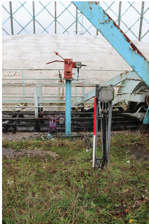
Plate 140: Gasholder No 5, detail view of extra low and extra high knock-off switches between standards 16 and 17, from the NNE
