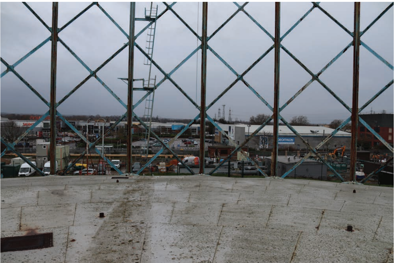
Plate 2: General view of the retail park to the south-west of the site, from the north-east
