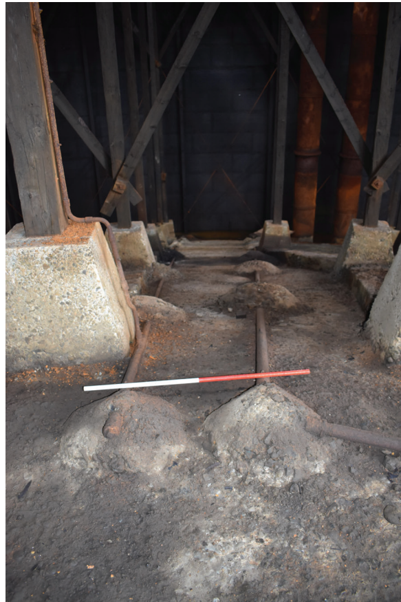
Plate 70: Gasholder No 4, detail view of two narrow pipes secured to the dumpling via concrete mounds, from the ENE
