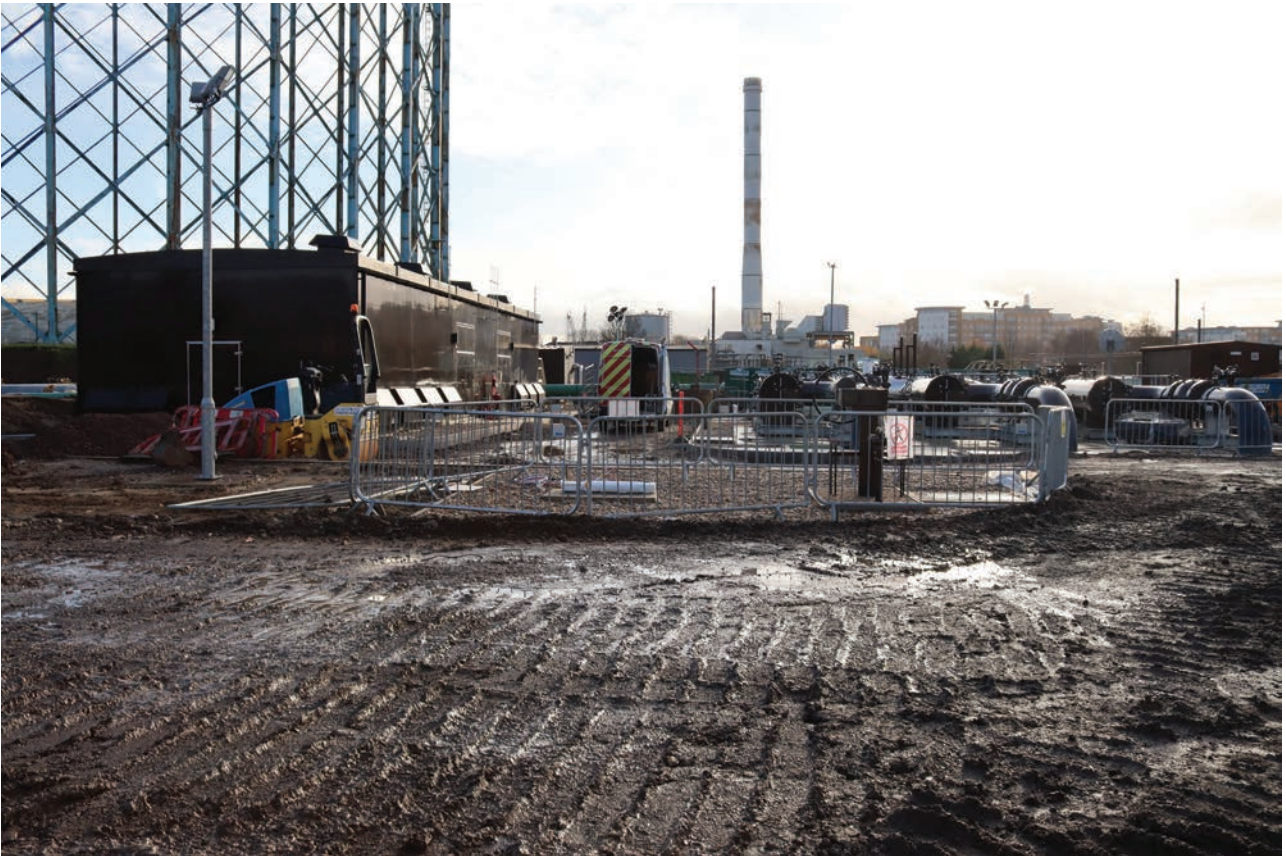
Plate 13: General view of modern high-pressure works, from the north-west
