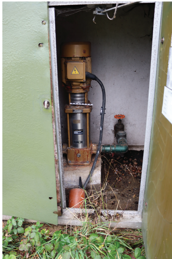
Plate 154: Gasholder No 5, detail view of the top up pump, from the south
