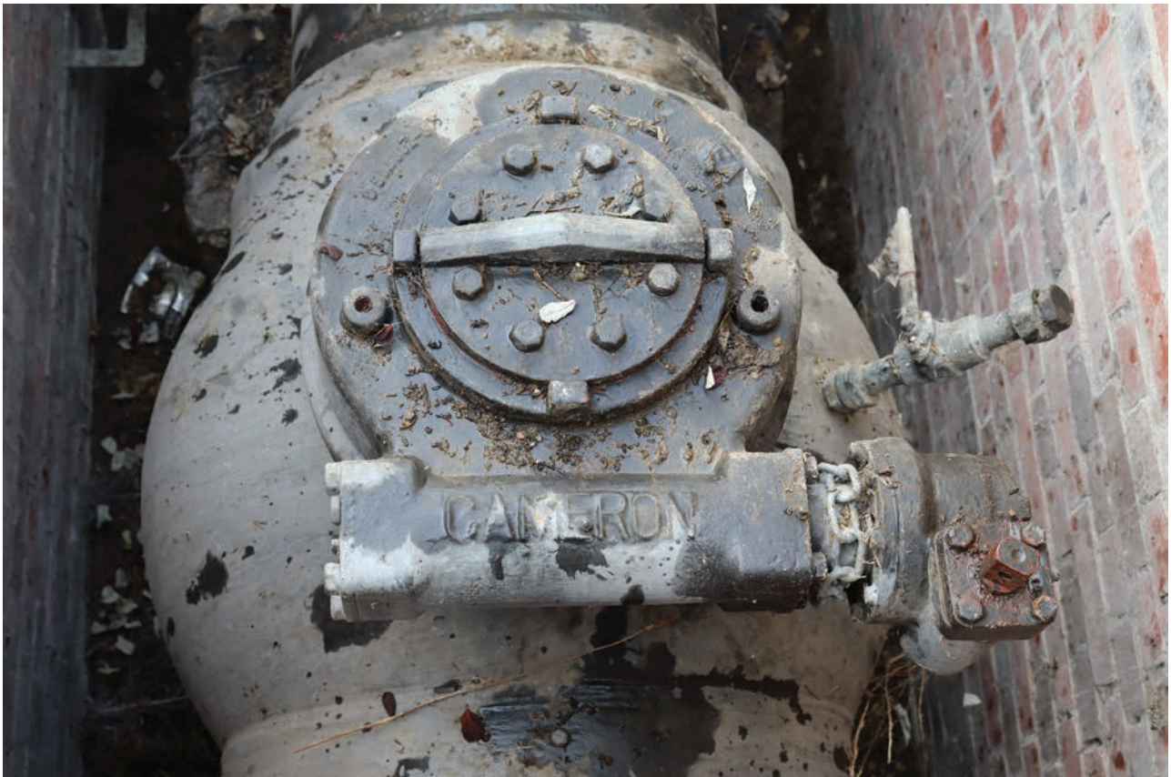
Plate 208: Valve pits, detail view of Cameron ball valve, from the north-east
