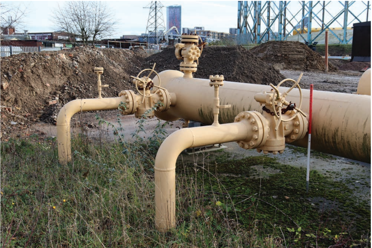
Plate 193: Pipework, general view of AUDCO valve, from the north-west
