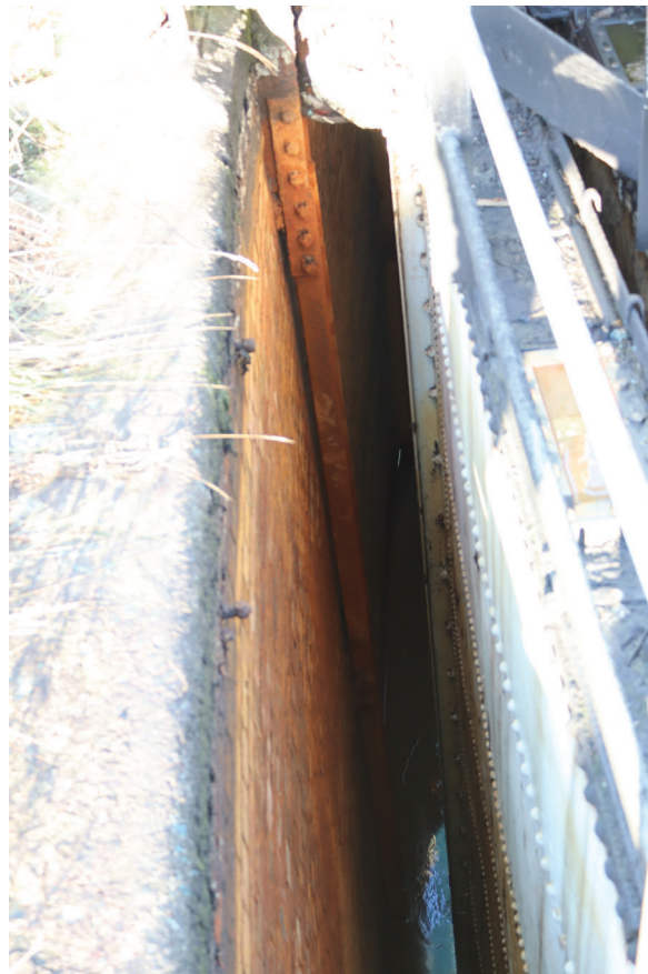
Plate 80: Gasholder No 5, detail view of guide rail set within the tank wall beneath standard 8, from the south
