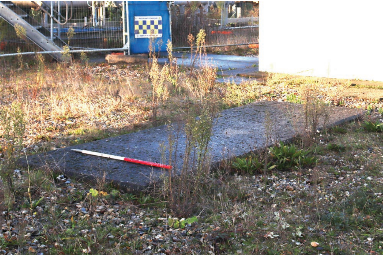
Plate 188: Structure 11b, detail view of concrete footing, from the north-east
