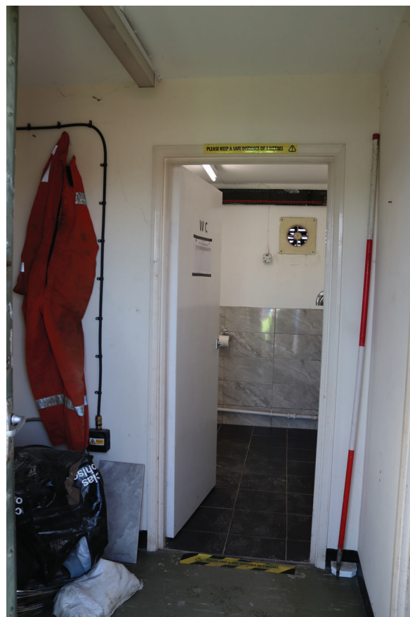
Plate 170: Structure 3, general view from the entrance of the Control Room across the hallway into the toilet, from the north-east
