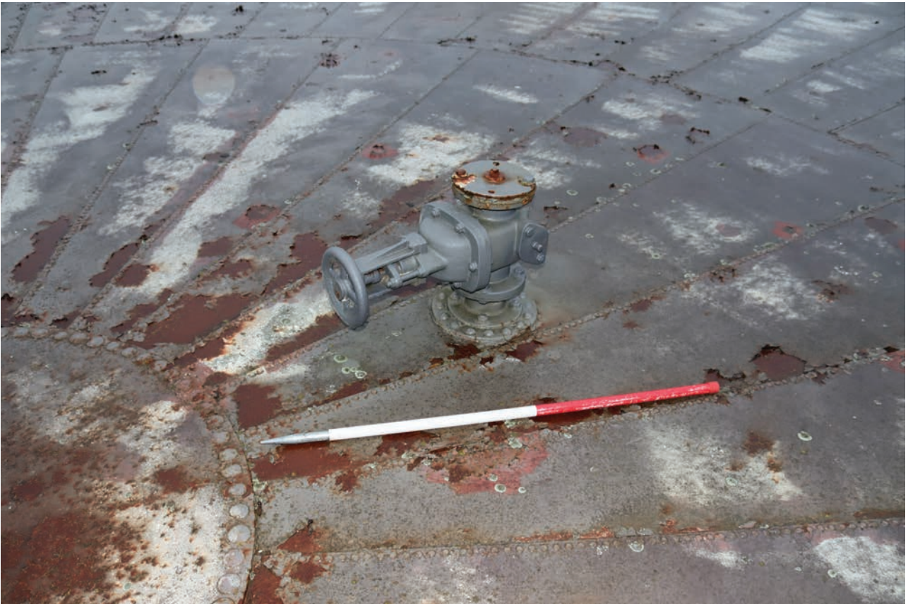
Plate 51: Gasholder No 4, detail view of the crown vent to the south-west of the centre of the crown, from the west
