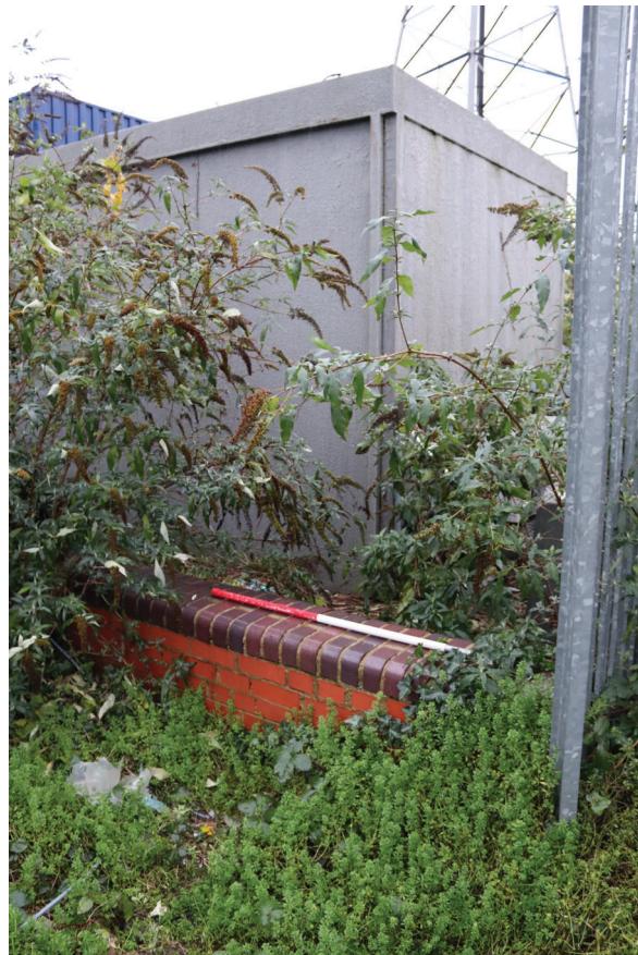
Plate 182: Structure 8, general view of the electrical building, from the south
