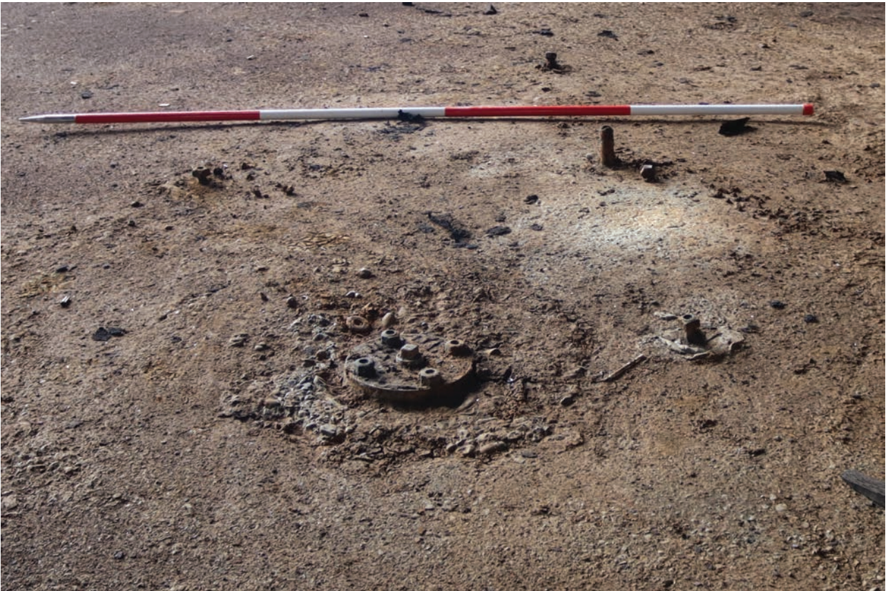
Plate 93: Gasholder No 5, general view of disused iron fixtures set within the centre of the dumpling, from the NNW
