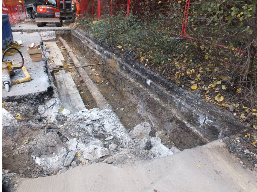
Plate 3: Overview of Trench 1c, looking east
