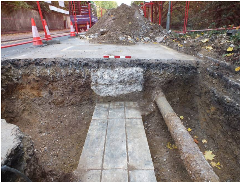
Plate 4: Overview of Trench 1c, looking east
