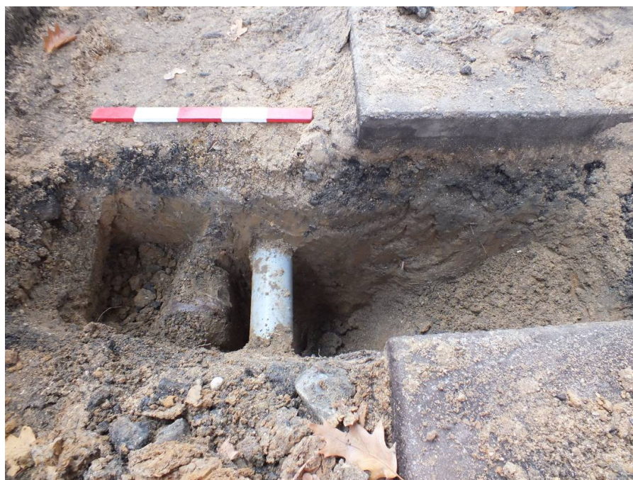
Plate 7: Trench 3 looking southwest
