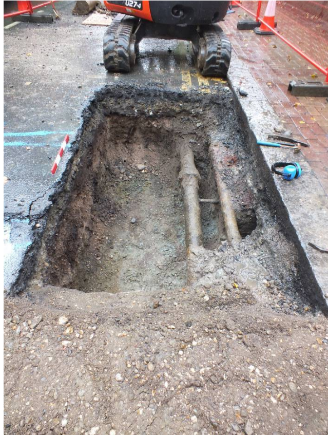
Plate 1: Trench 1a overview prior to extension, looking southwest
