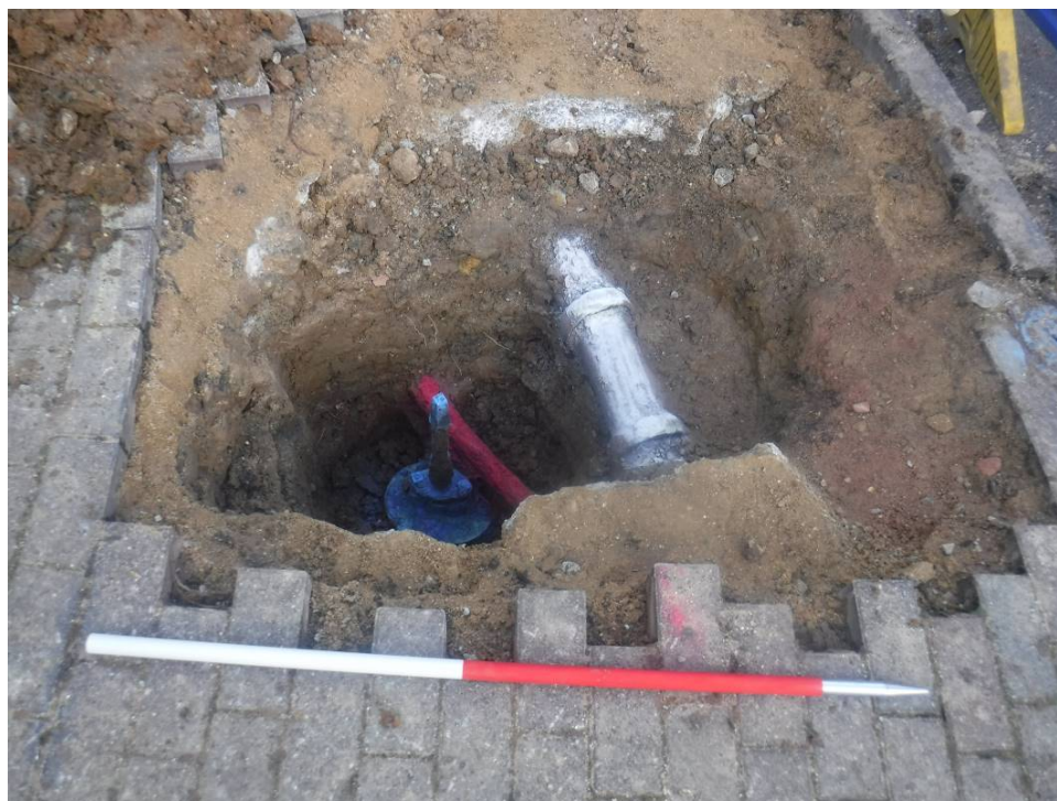
Plate 8: Trench 4 section, looking west, with services painted
