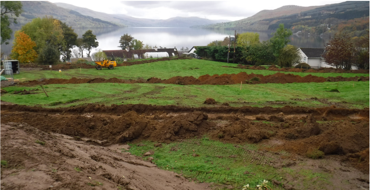
Plate 10: Site from the North – Post Excavation
