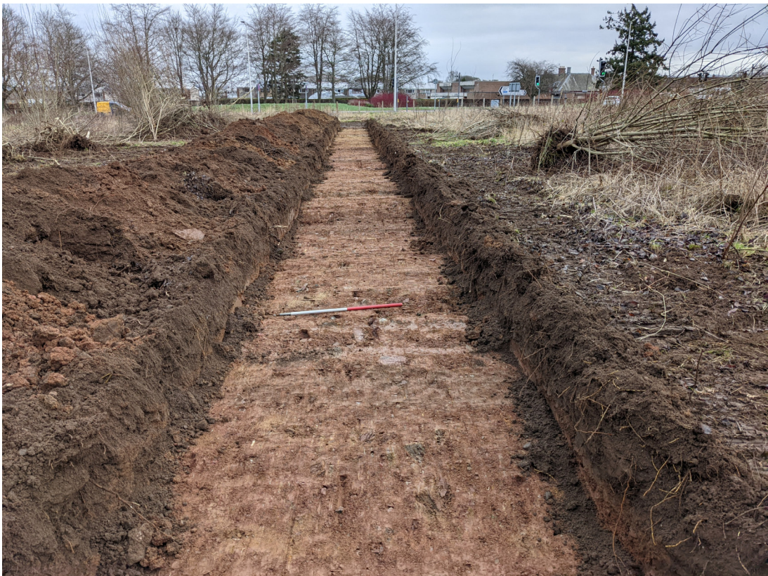
Plate 1 Typical post-excavation view of trench
