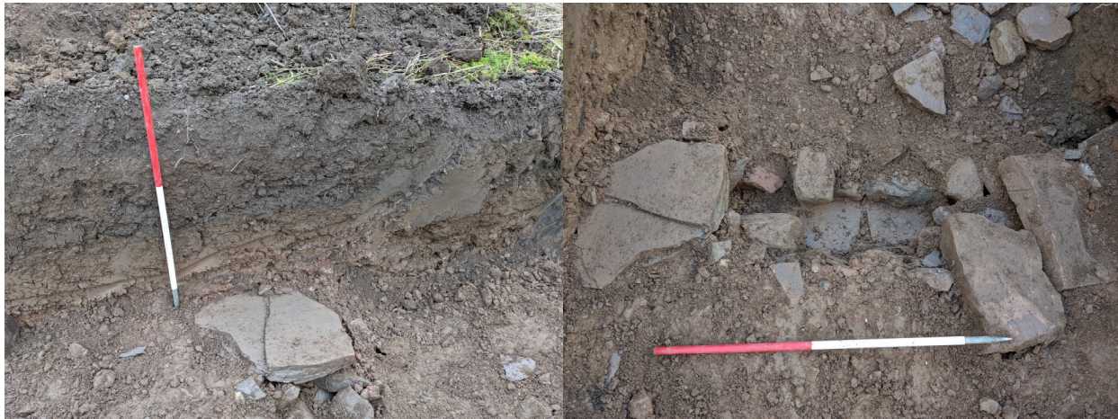
Plate 3 View of Culvert in Trench 2
