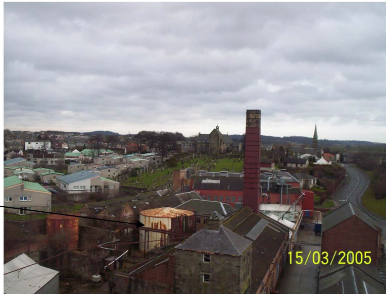
Plate 10: General view Distillery prior to Demolition from west
