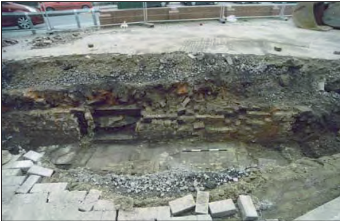
Plate 6: North-facing section of Trench 5 (west end), showing wall [507]
