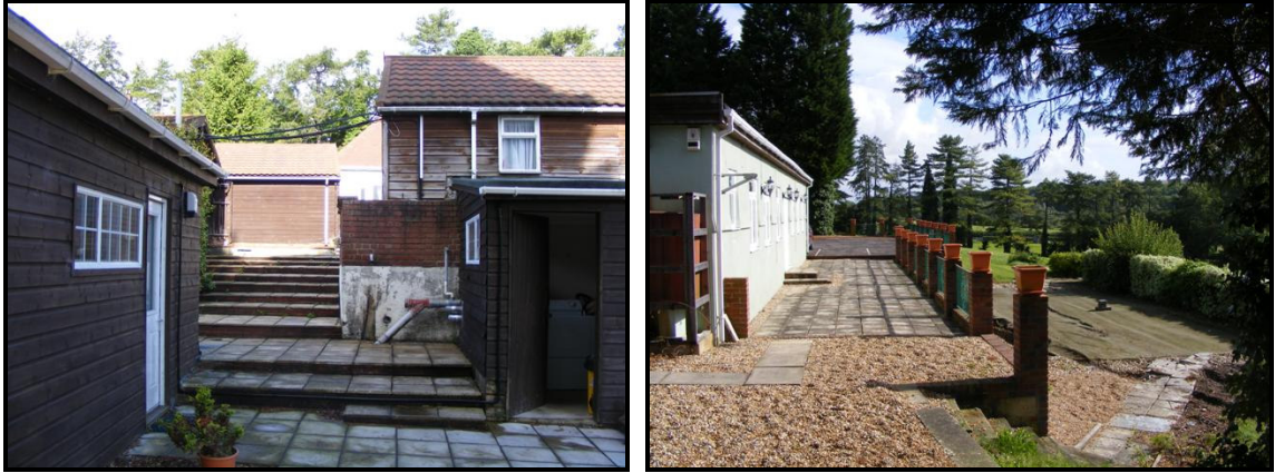
Plate E: View showing difference in level and stairs between terraces amongst the buildings to the south of the conference centre (left) and the difference between the rear of the conference centre and the area of the artificial mini golf green (right);
