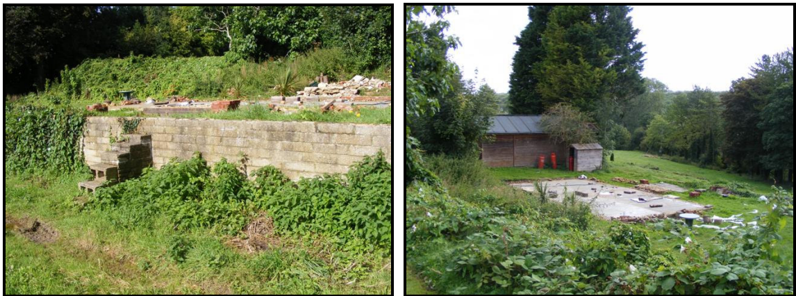
Plate G: View looking east from the eastern section of the development site showing difference in ground level between the lowest two terraces (left) and looking north-east from the 'garden' area showing the demolished building (right)
