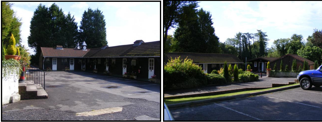
Plate C: Views of the accommodation / conference centre building in the north-east of the site; looking north-east from the area of hardstanding outside the building (top left), and looking south-east from the main car park (top right) - showing the difference in ground level
