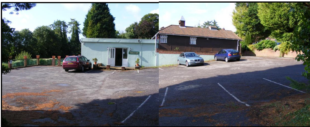
Plate D: Composite picture looking south towards the accommodation / conference centre building from the car park to the north; showing the sloping nature of the site
