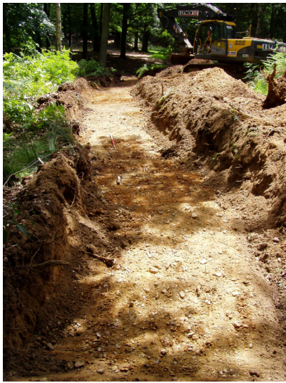
Plate 4: Drainage Excavation
