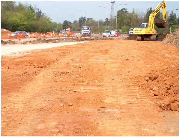
Plate 2: Ground Reduction Access Road
