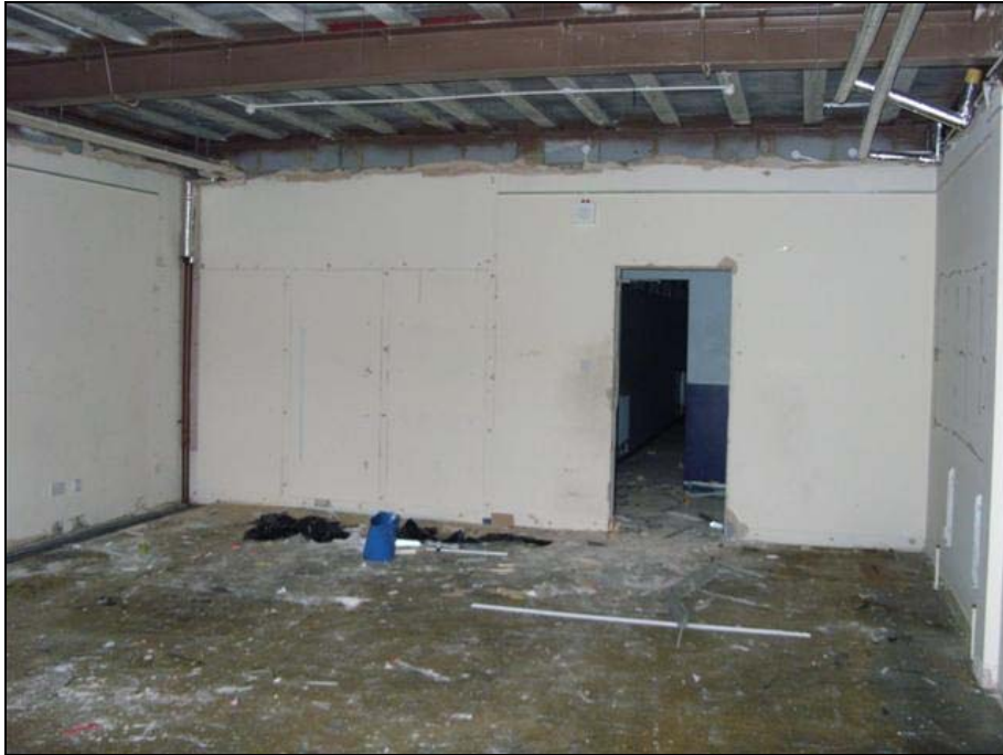
Plate 9: Ground Floor History Classroom looking north
