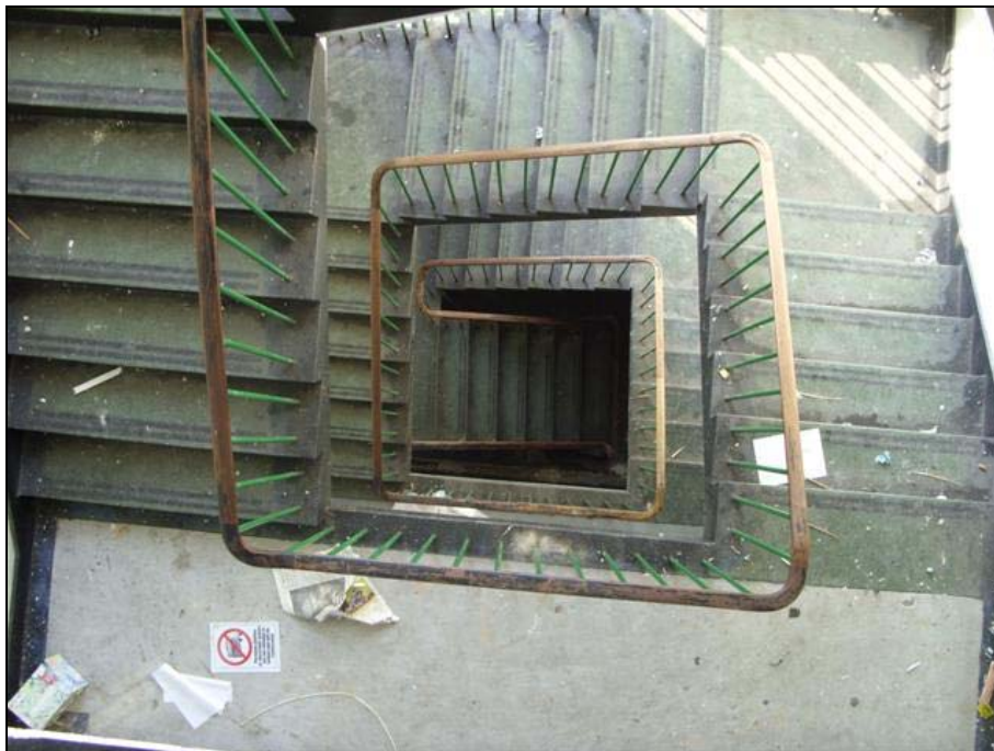
Plate 20: Third Floor Main south stairwell
