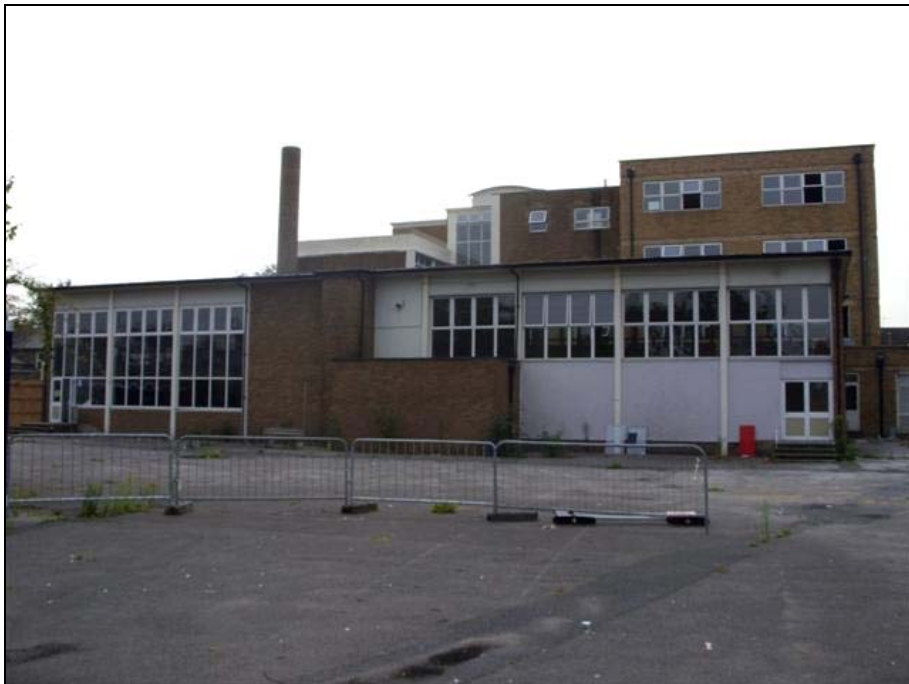
Plate 2: School exterior looking south
