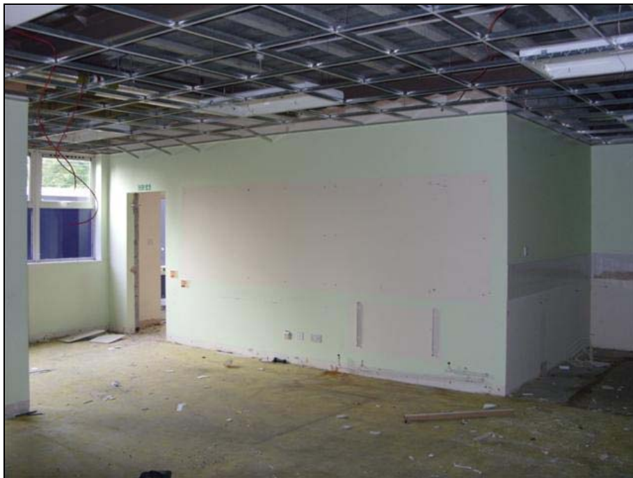
Plate 8: Ground Floor Staffroom, looking northwest
