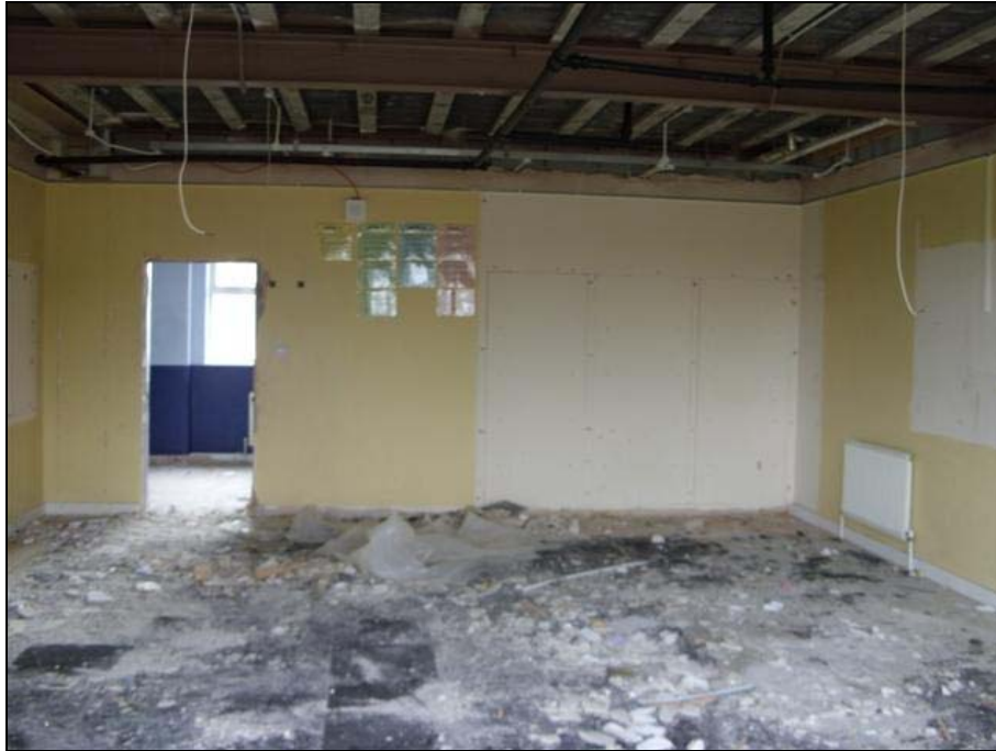
Plate 15: Second Floor English Classroom looking south
