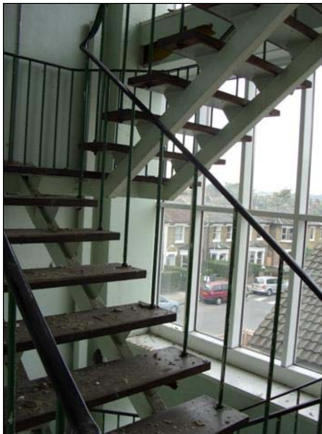
Plate 14: Second Floor Extension Stairwell, looking southwest
