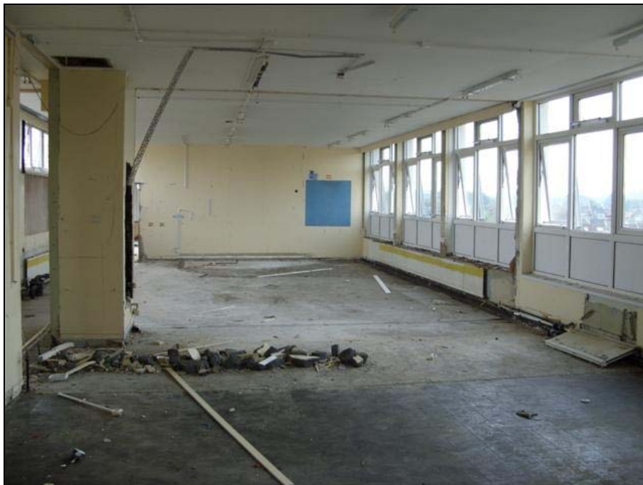
Plate 18: Third Floor Science Classrooms looking south
