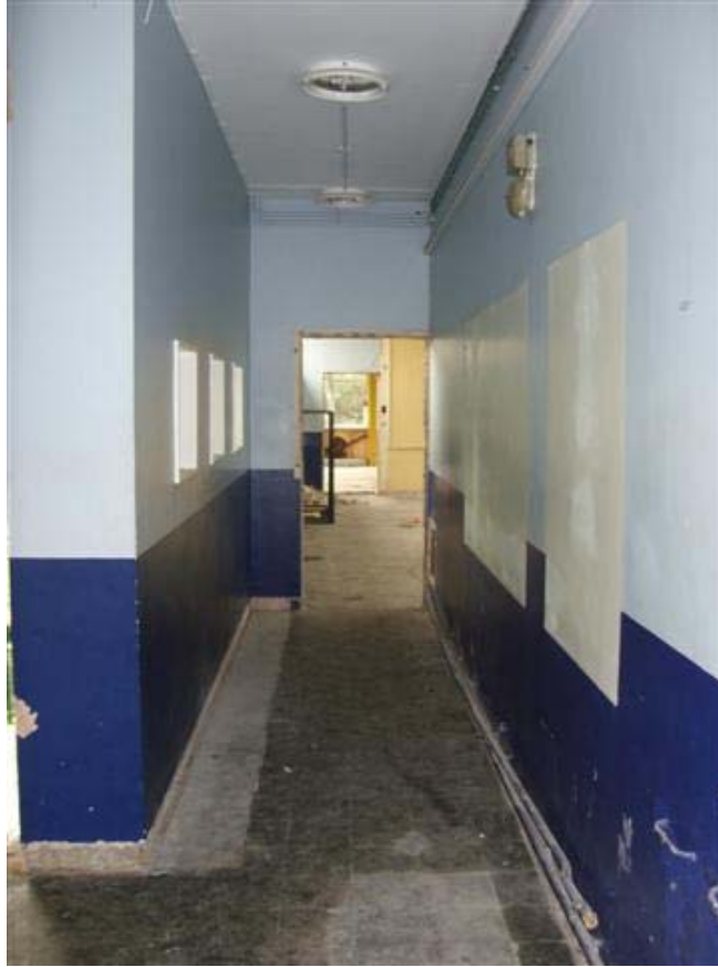
Plate 11: First Floor Corridor looking south
