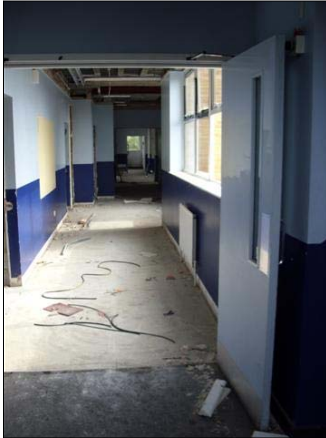
Plate 19: Third Floor Block B corridor
