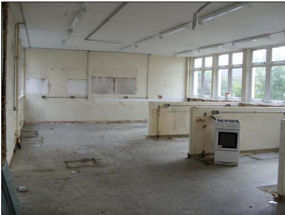
Plate 10: First Floor Technology Classroom, looking southeast
