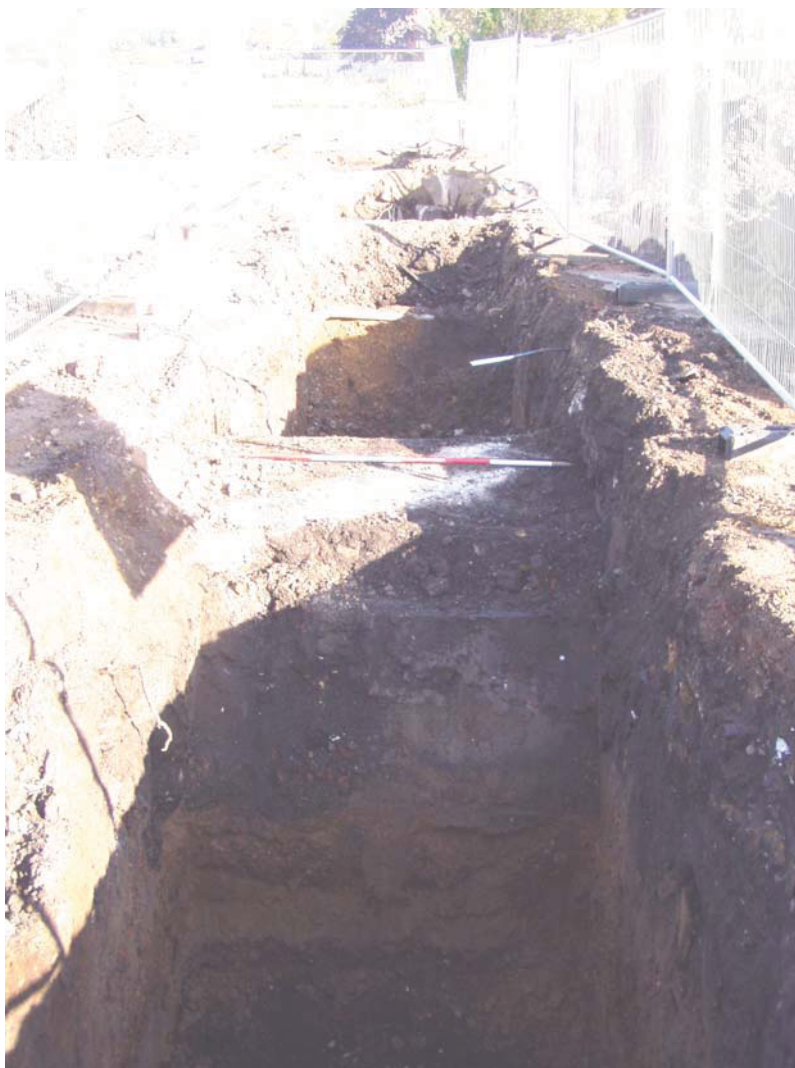
Plate 2. Trench 2 from south.
