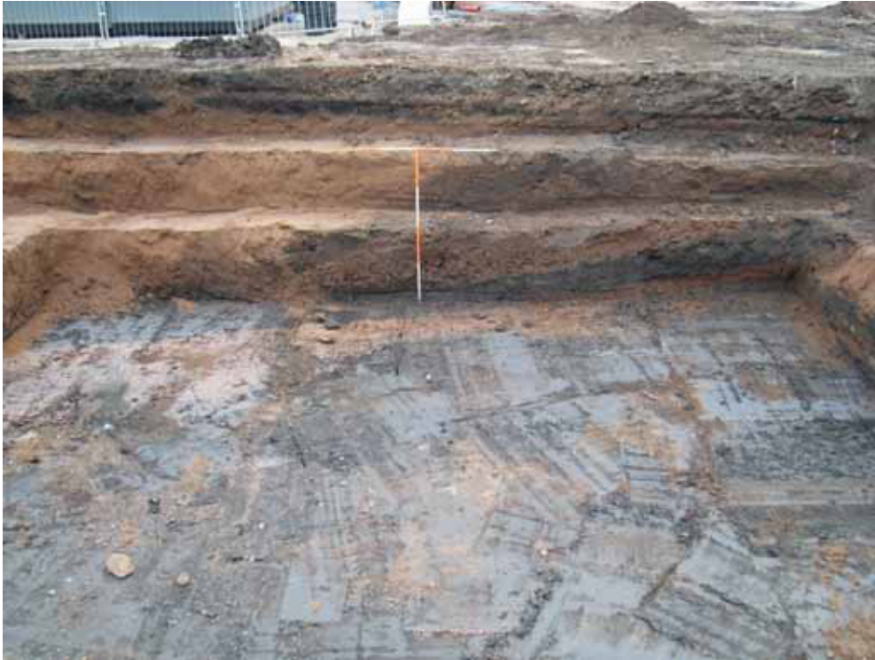
Plate 7: Attenuation tank, showing sloping nature of made ground deposits
