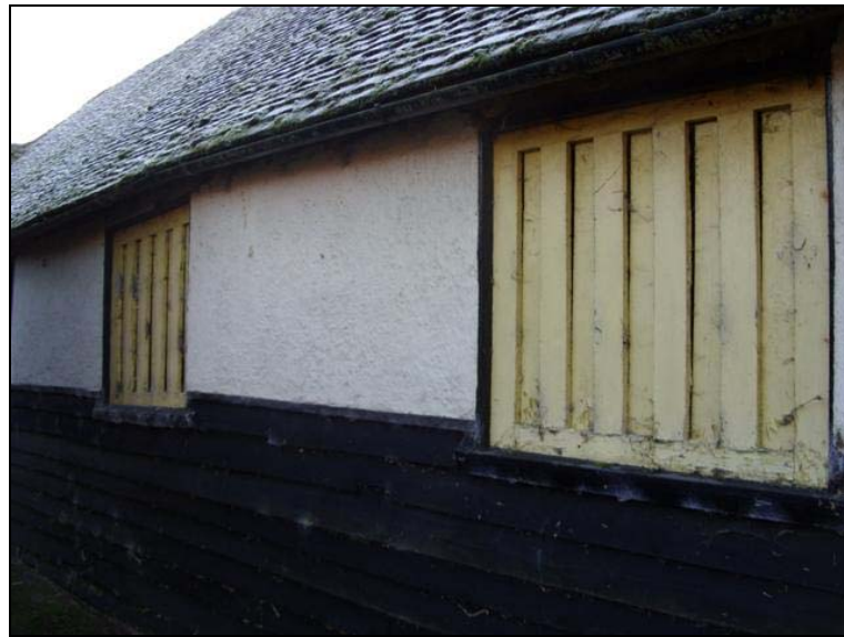
Plate 2: Rendered and boarded north wall
