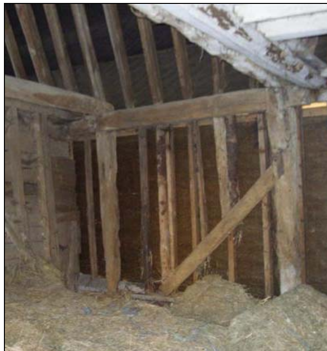
Plate 3, sample of south wall framing, Room 7
