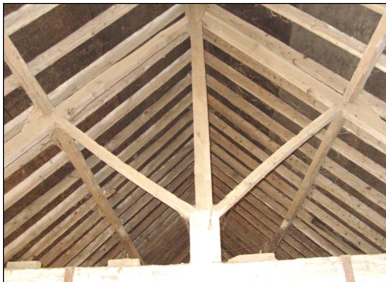
Plate 10: Stable King Post roof
