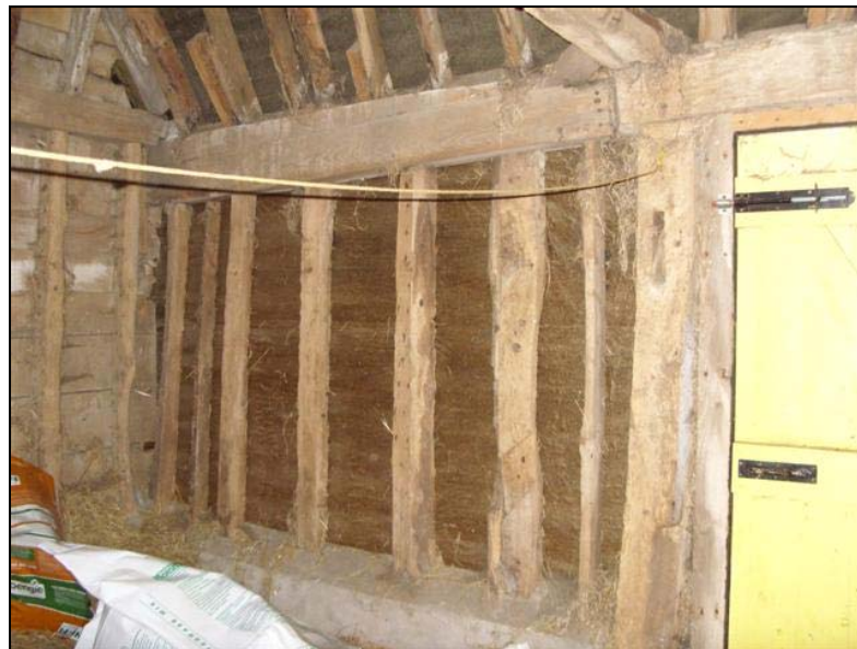
Plate 4, wall framing, Room 6
