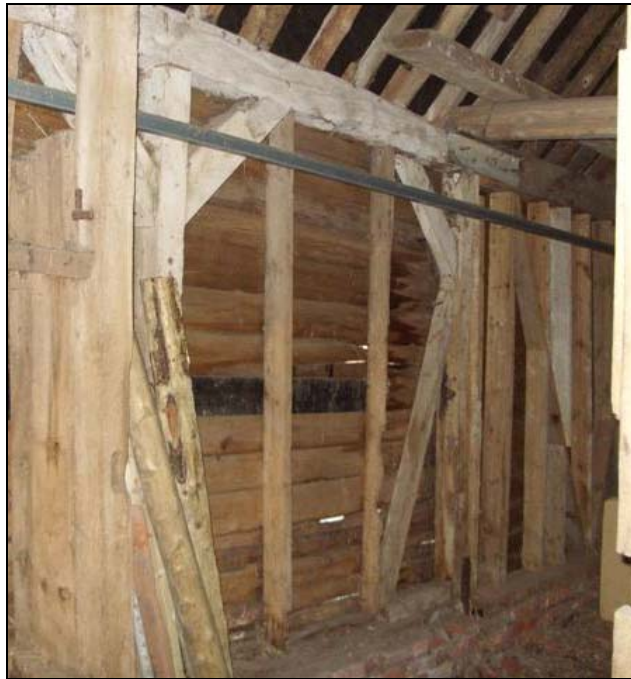
Plate 7: Framing of western extension
