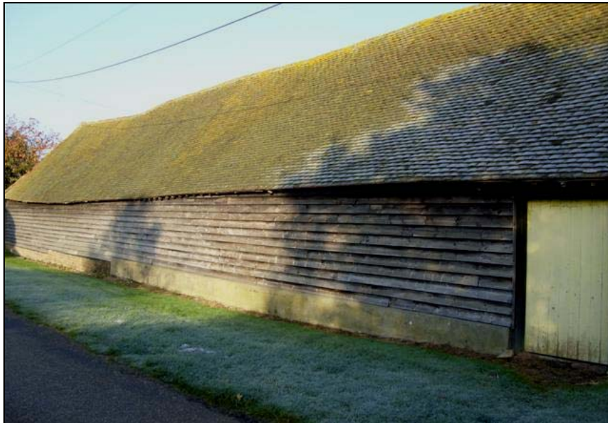
Plate 1, south side of southern block
