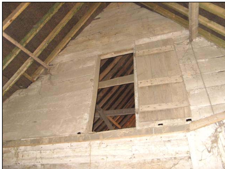
Plate 5: Gable end of early phase.
