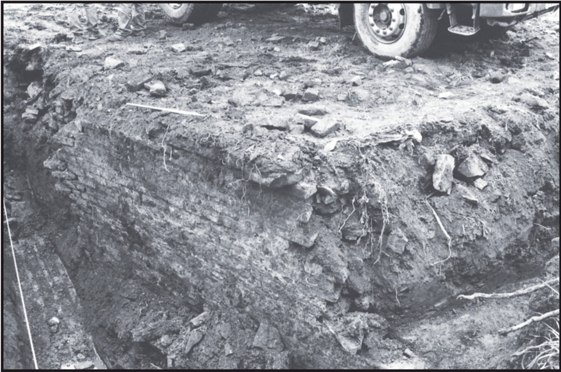
Plate 1: Boilerhouse Wall from NW
