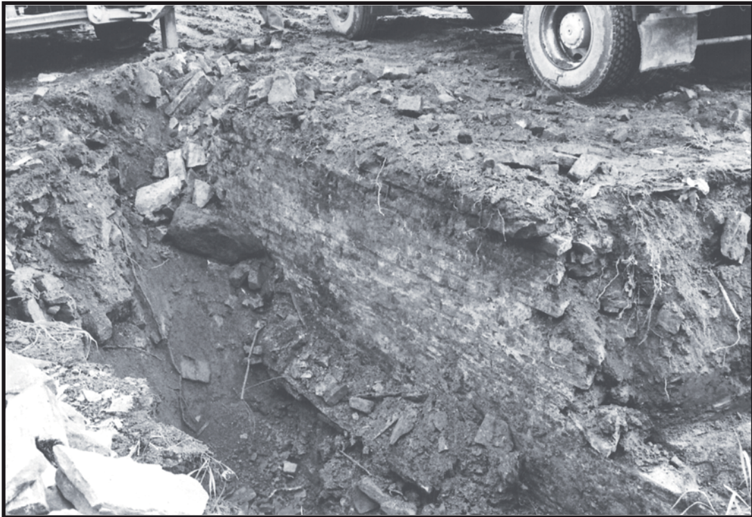
Plate 2: Boilerhouse Wall from NW
