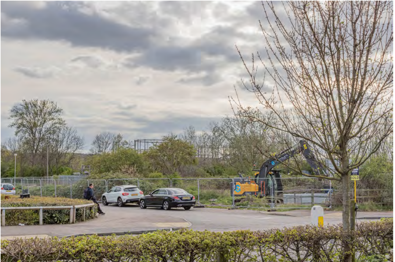
Plate 3 (BEL096): General view of the gasholders from Clydesdale Way from the north-east
