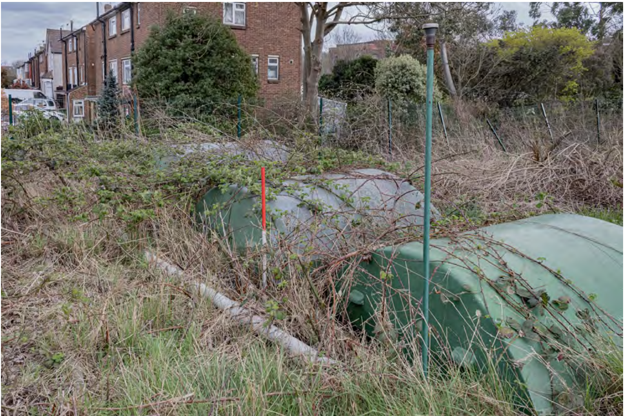
Plate 66 (BEL077): General view of steel covers from the north-west
