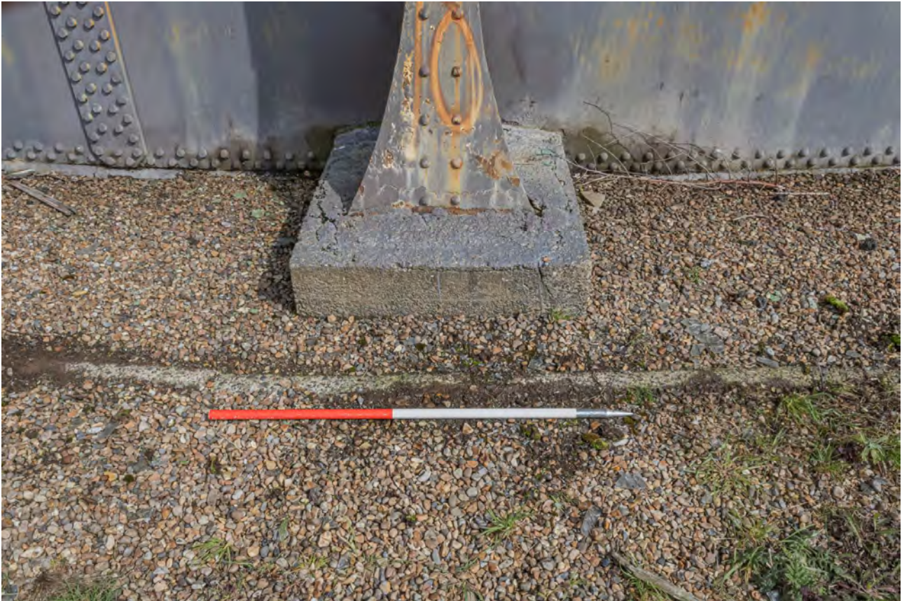
Plate 39 (BEL059): Gasholder No 2, detail of base of standard 10, from the south-west
