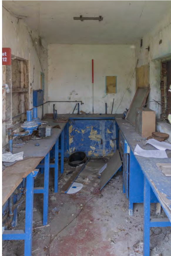
Plate 65 (BEL080): Building B, general view of the interior from the east
