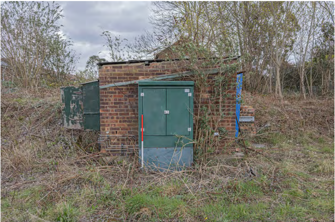
Plate 72 (BEL087): Building C, general view from the west
