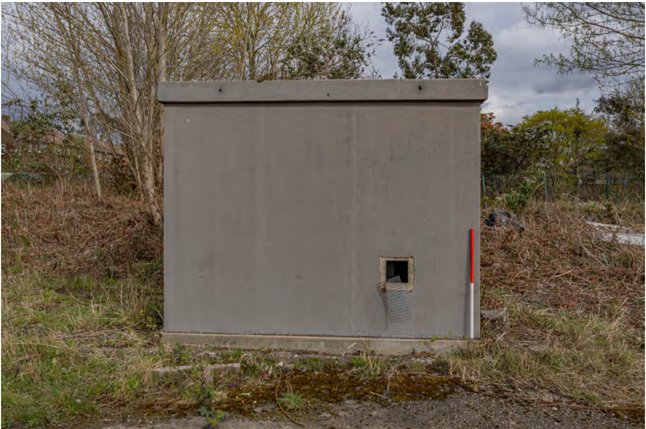
Plate 76 (BEL090): Building D, general view of the Instrument Room from the west
