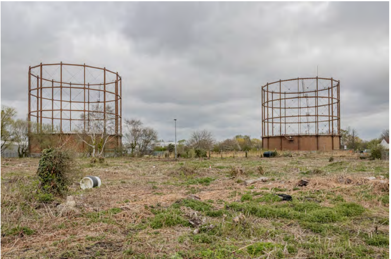
Plate 4 (004): General view of the gasholders within the compound from the south
