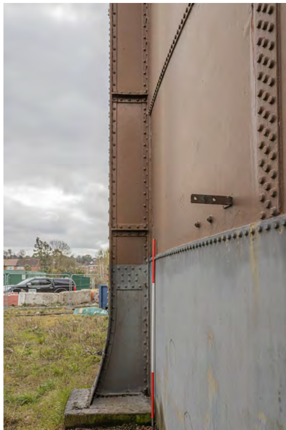
Plate 36 (BEL045): Gasholder No 2, detail of standard 3 from the north
