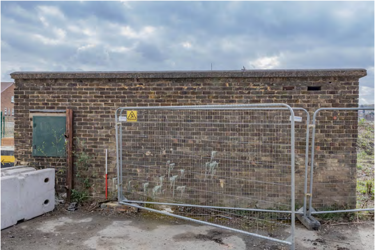
Plate 57 (BEL070): Building A, general view from the north
