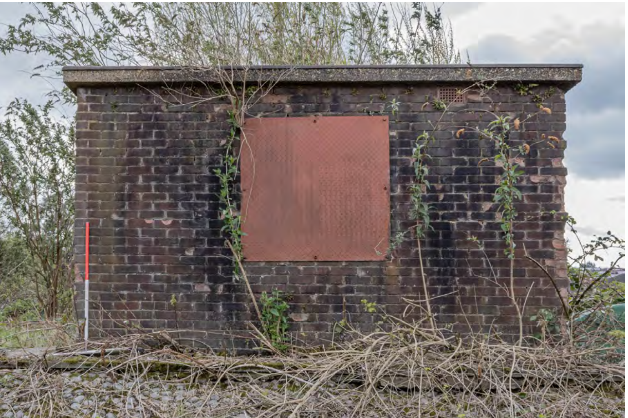
Plate 62 (BEL074): Building B, general view from the north
