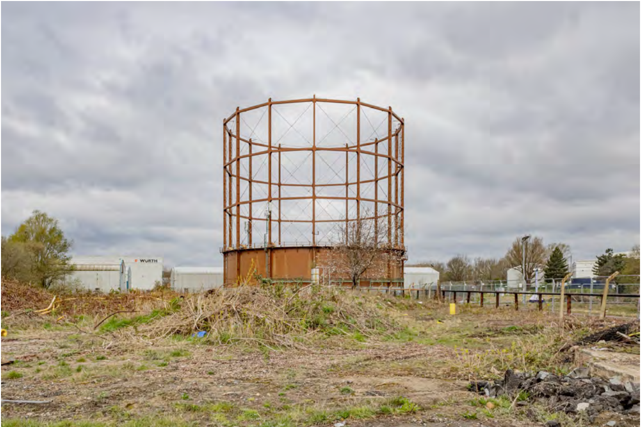
Plate 5 (BEL001): Gasholder No 1, general view from the WSW
