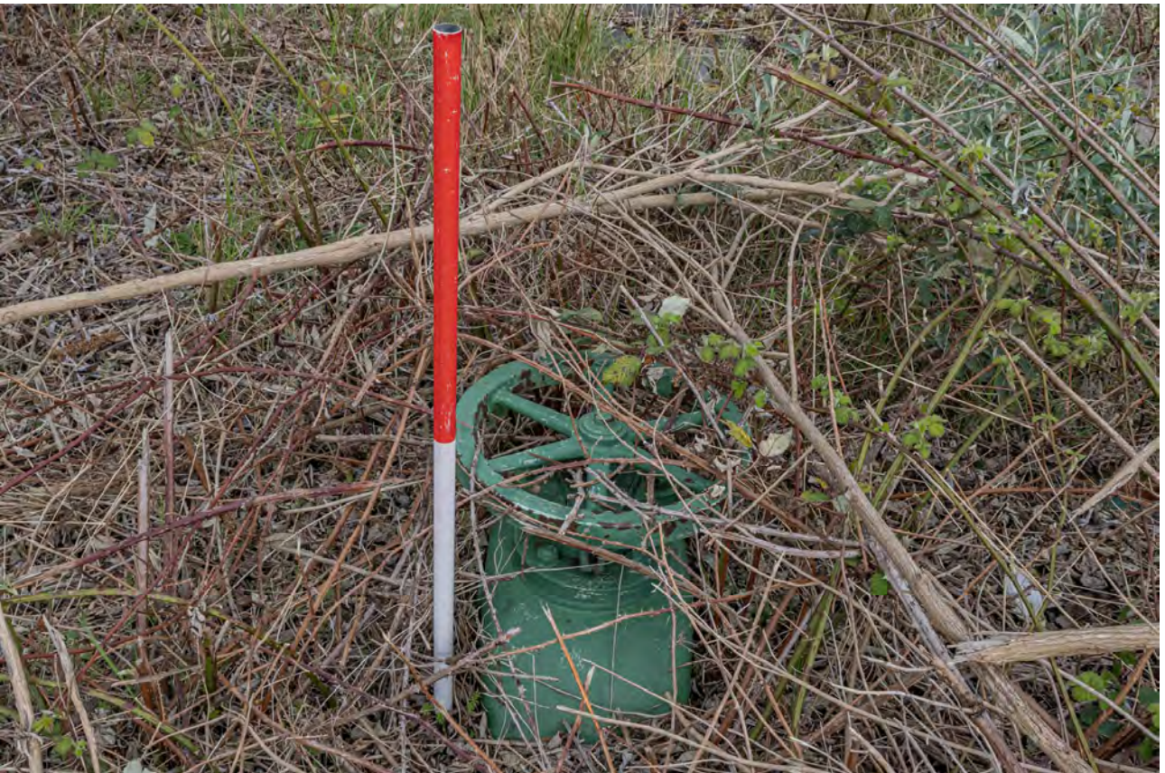
Plate 70 (BEL076): Detail of valve wheel from the SSW
