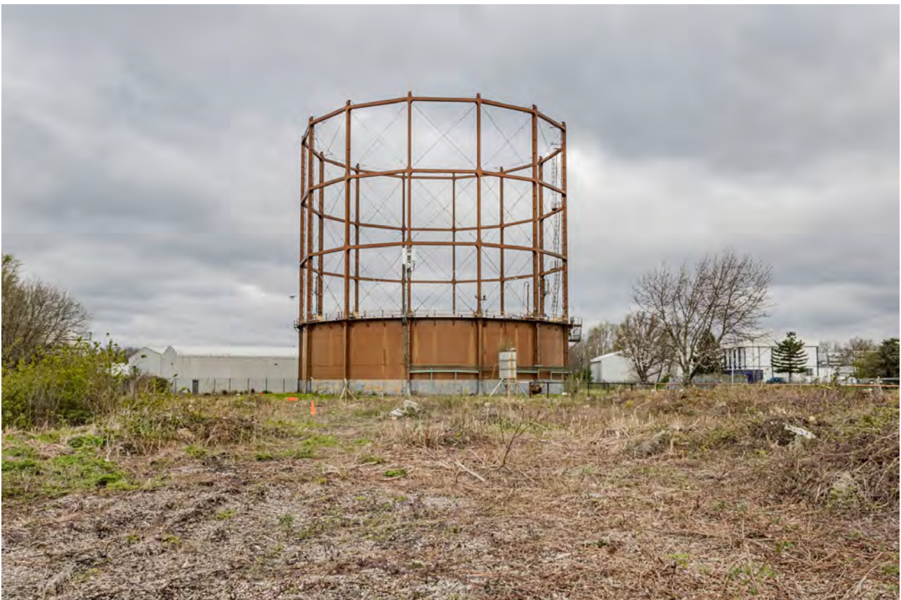
Plate 6 (BEL003): Gasholder No 1, general view from the WNW
