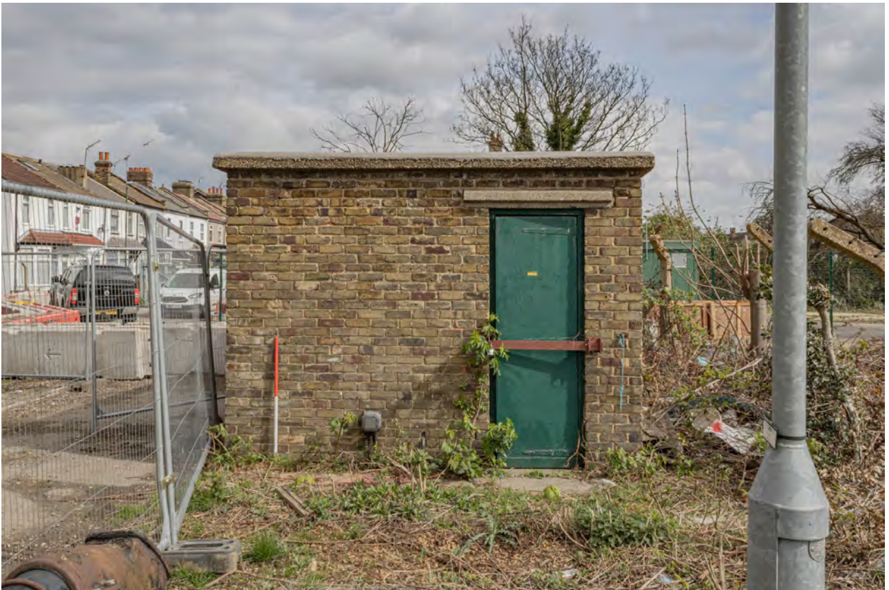
Plate 60 (BEL073): Building A, general view from the west
