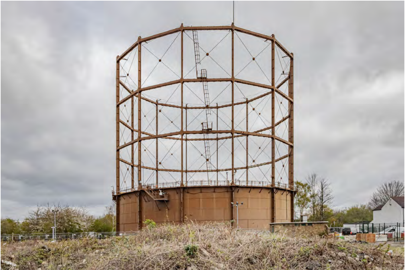
Plate 7 (BEL002): Gasholder No 1, general view from the NNE
