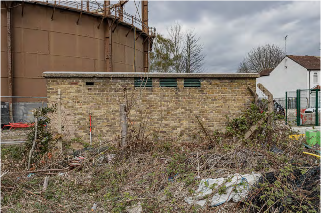
Plate 59 (BEL072): Building A, general view from the south
