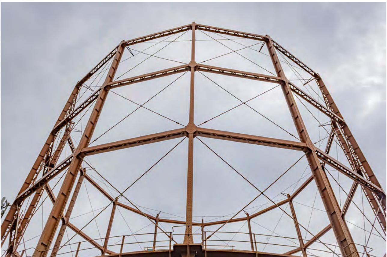
Plate 8 (BEL007): Gasholder No 1, general view of guide framing from the north-west
