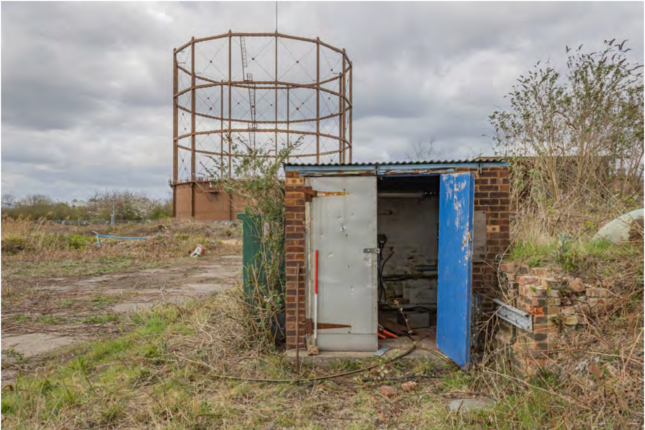
Plate 73 (BEL088): Building C, general view from the south
