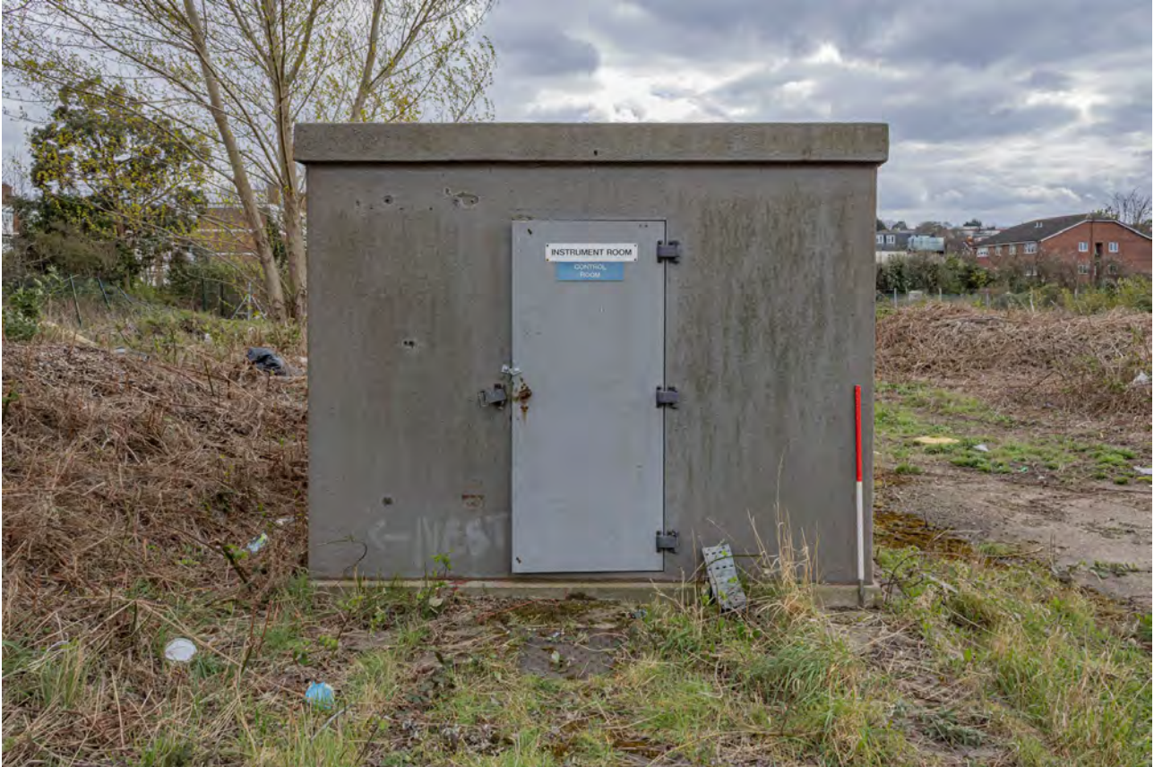
Plate 75 (BEL089): Building D, general view of the Instrument Room from the north
