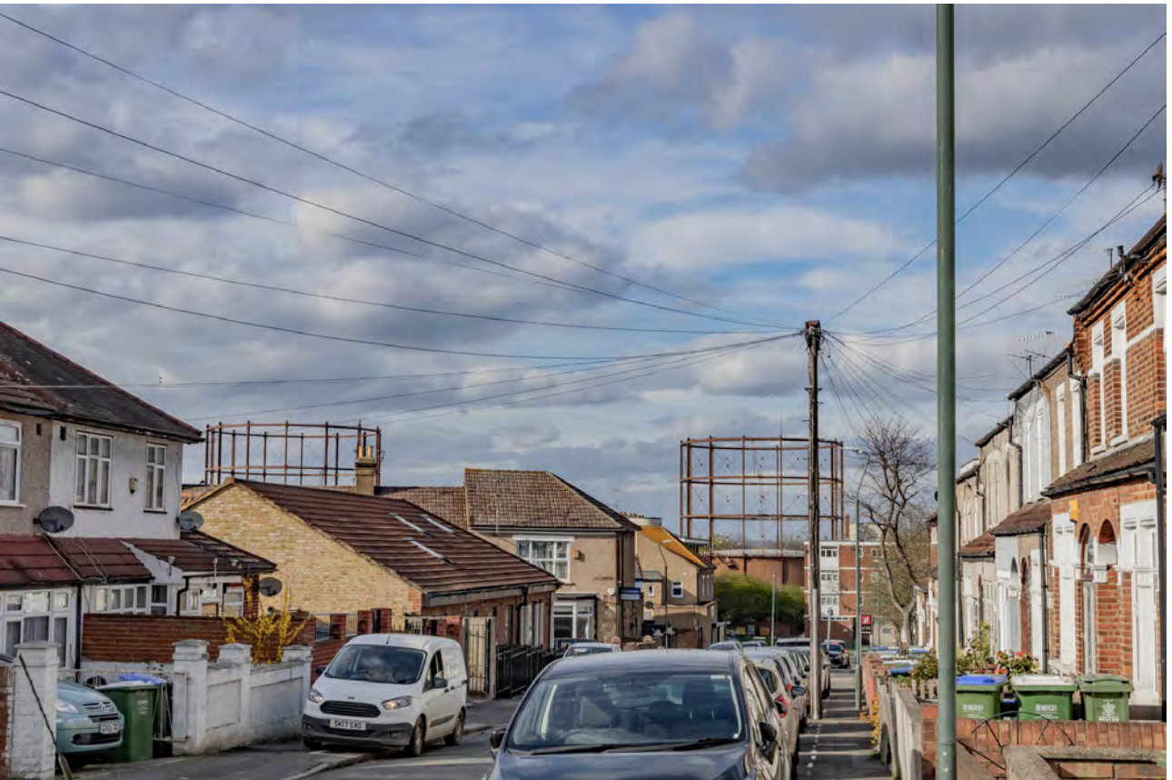
Plate 2 (BEL095): General view of gasholders from Edwards Road from the south
