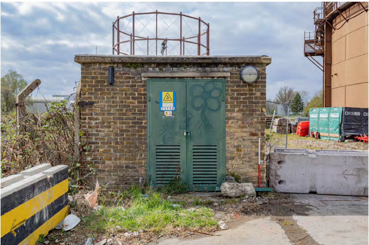
Plate 58 (BEL071): Building A, general view from the east
