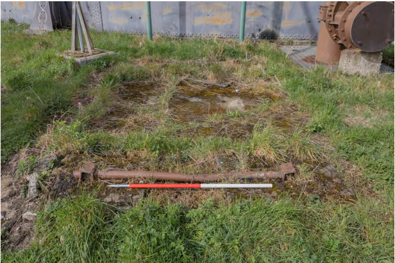
Plate 28 (BEL021): Gasholder No 1, detail of concrete platform between standards 7 and 8 from the east
