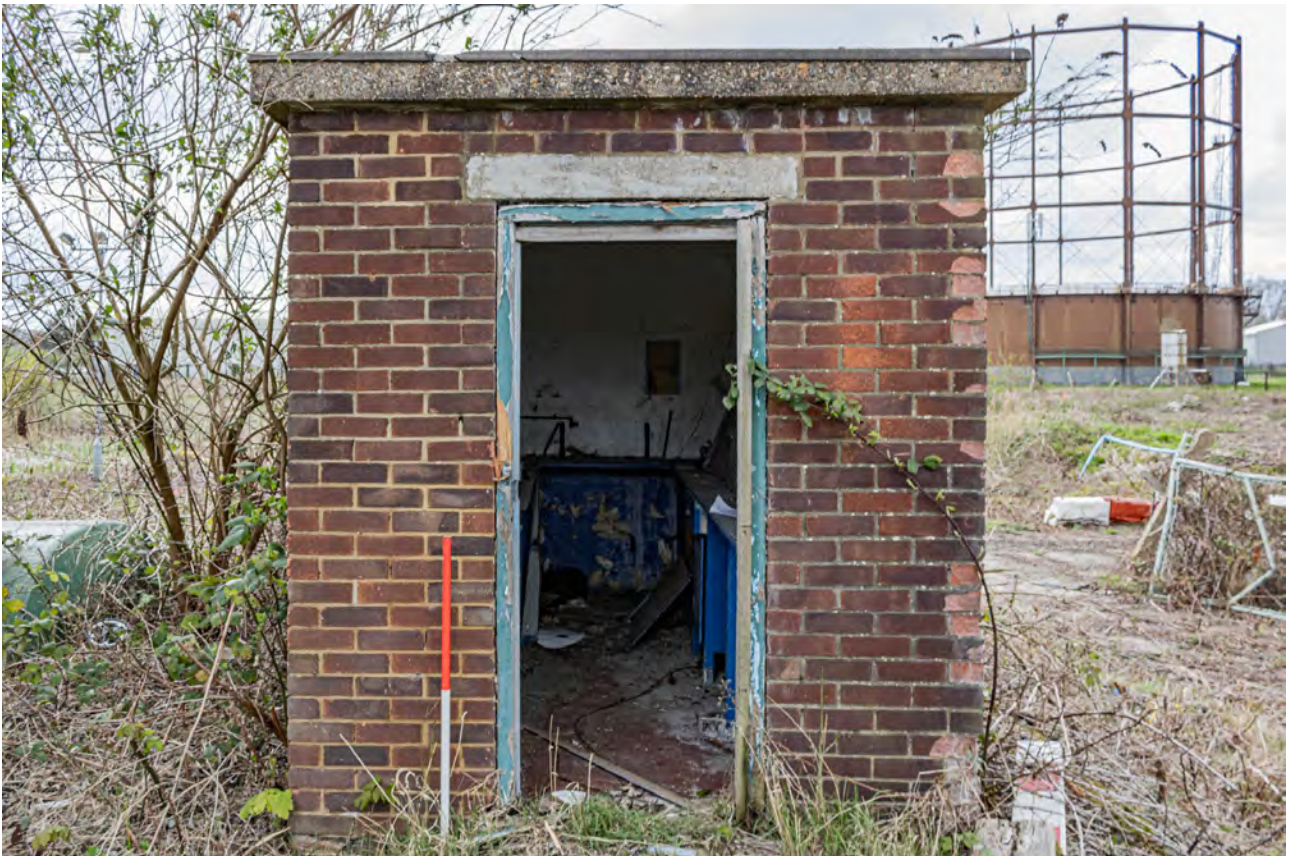
Plate 64 (BEL079): Building B, general view from the east
