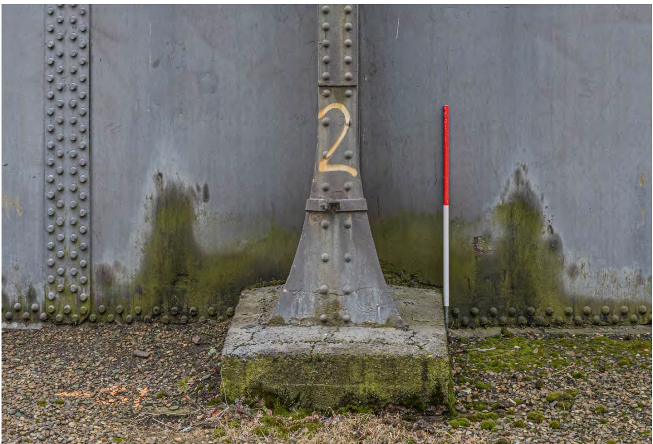
Plate 38 (BEL082): Gasholder No 2, detail of standard 2 from the north-east
