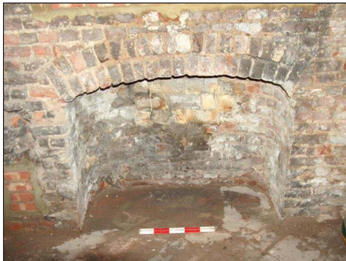
Plate 4: Fireplace, Room B5
