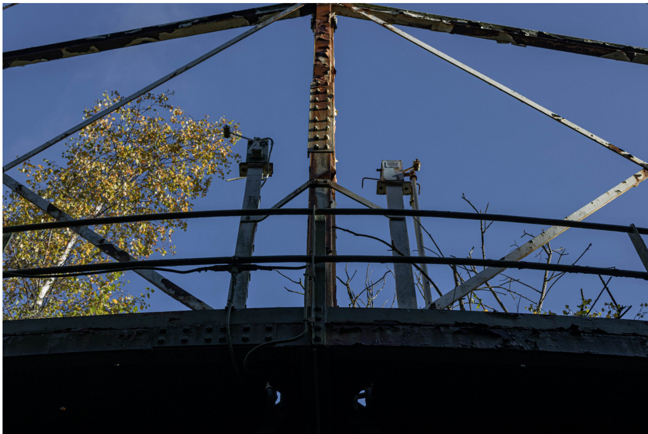
Plate 20: Gasholder No 3, detail of knock-off switches to the south-west of the holder from the south-west
