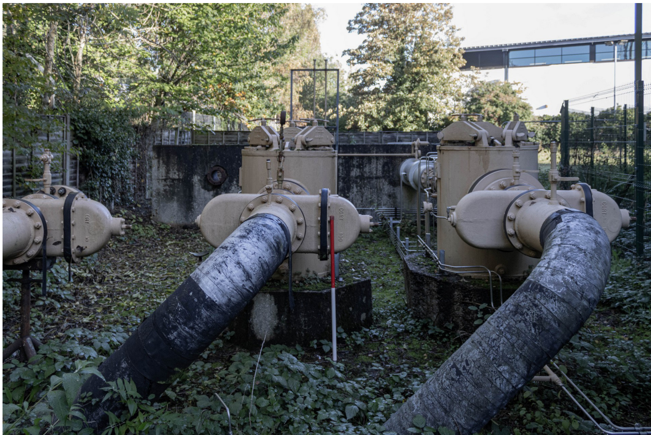
Plate 26: Gasholder No 3, detail of pipework from the SSW
