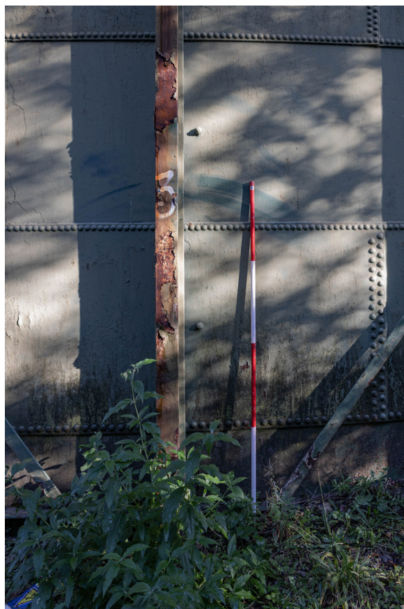
Plate 14: Gasholder No 3, detail of Standard 3 from the SSW
