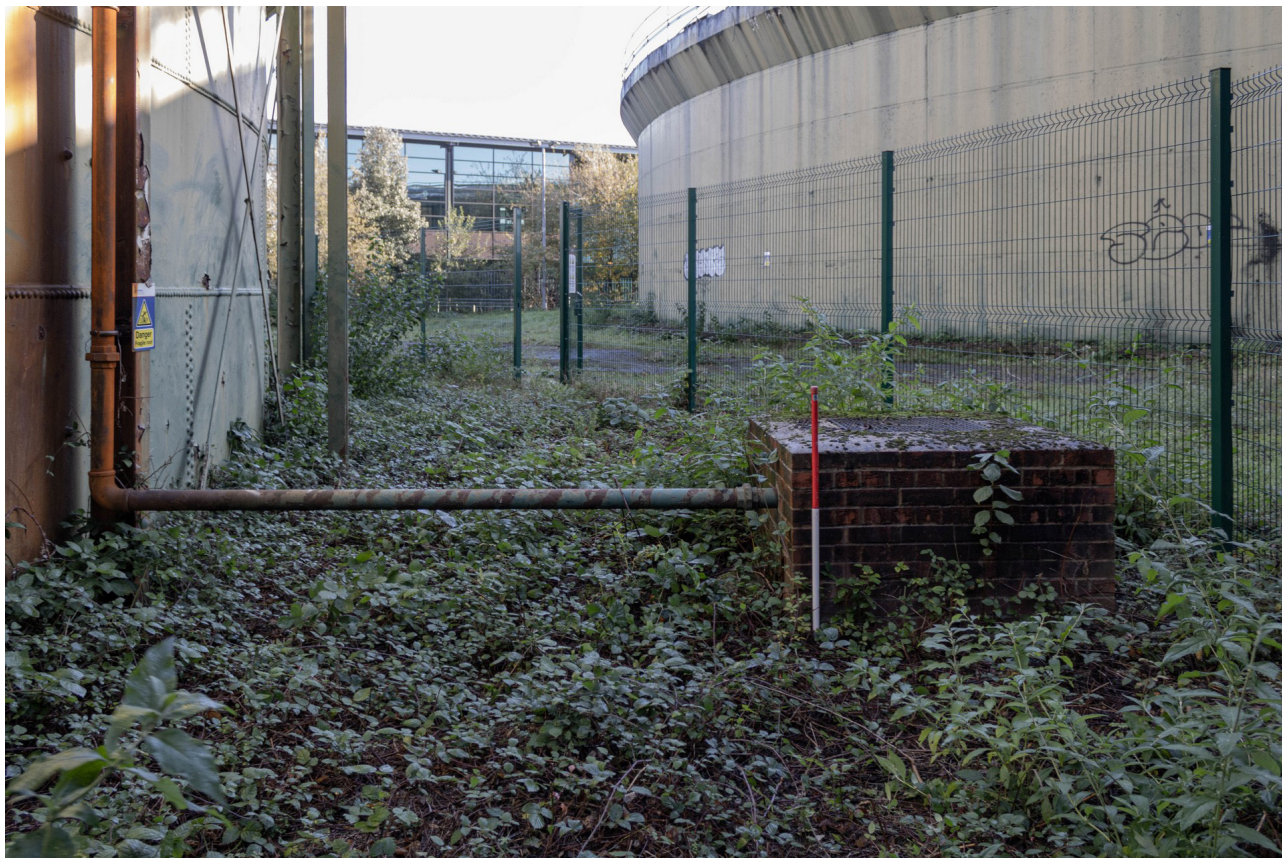
Plate 24: Gasholder No 3, detail of brick tank to the SSE side of the holder from the west
