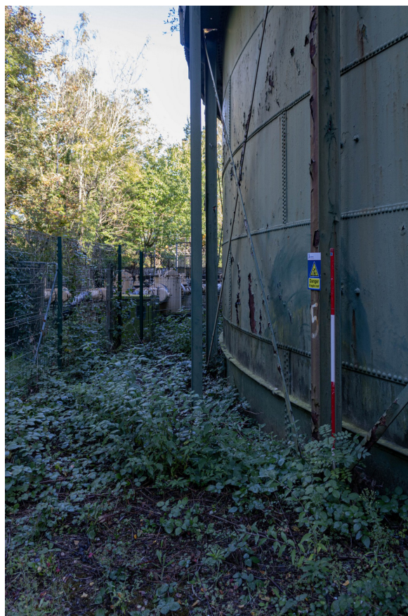
Plate 11: Gasholder No 3, detail of tank at Standard 5 from the SSE
