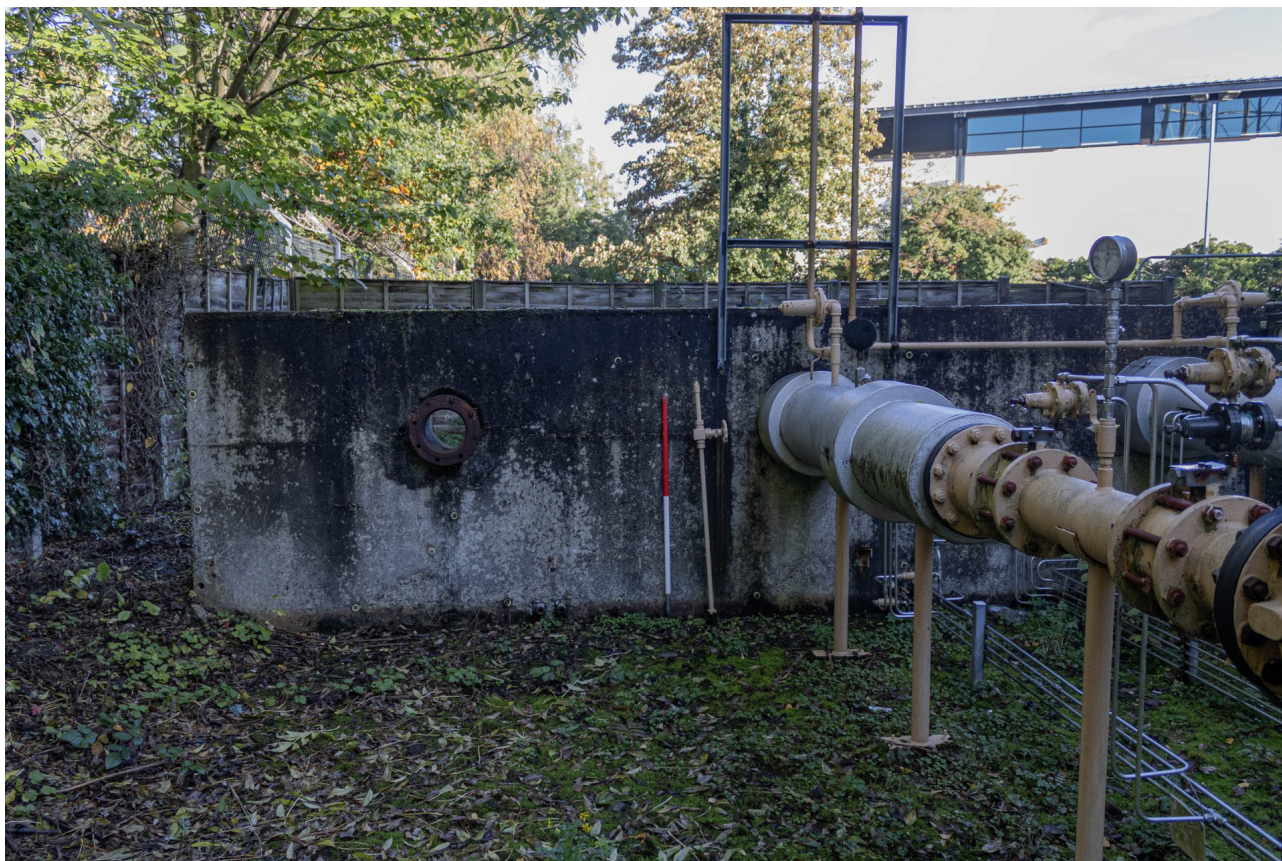
Plate 27: Gasholder No 3, detail of pipework from the SSW
