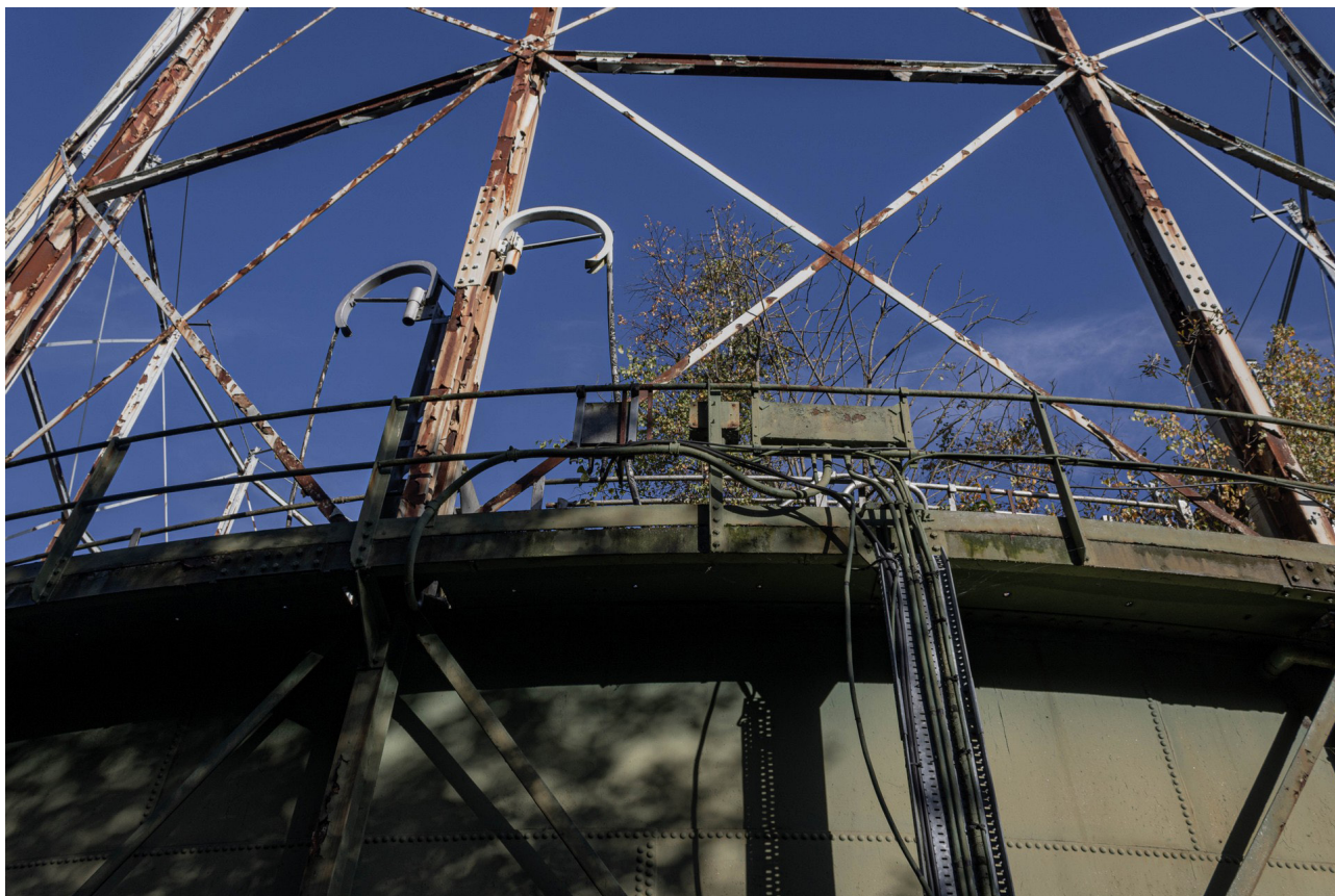
Plate 23: Gasholder No 3, detail of hose supports to the south side of the holder, from the south
