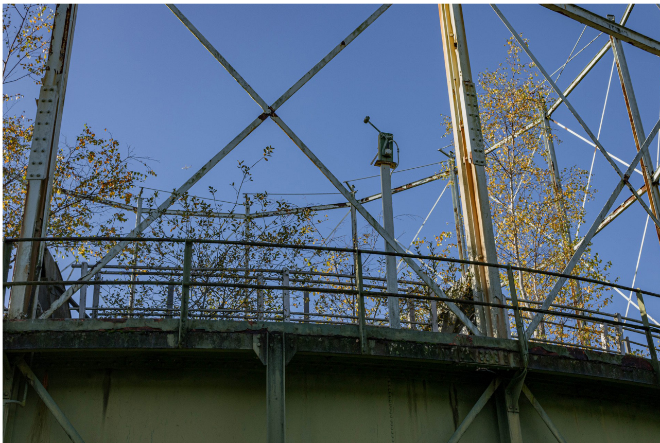
Plate 21: Gasholder No 3, detail of knock-off switch to the north of the holder from the NNW
