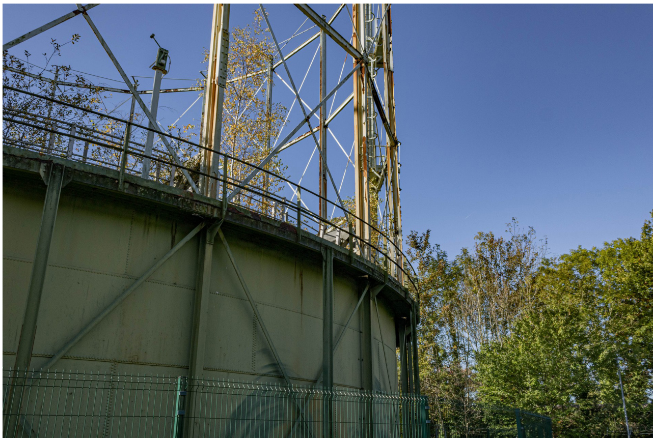
Plate 17: Gasholder No 3, detail of upper walkway from the ENE
