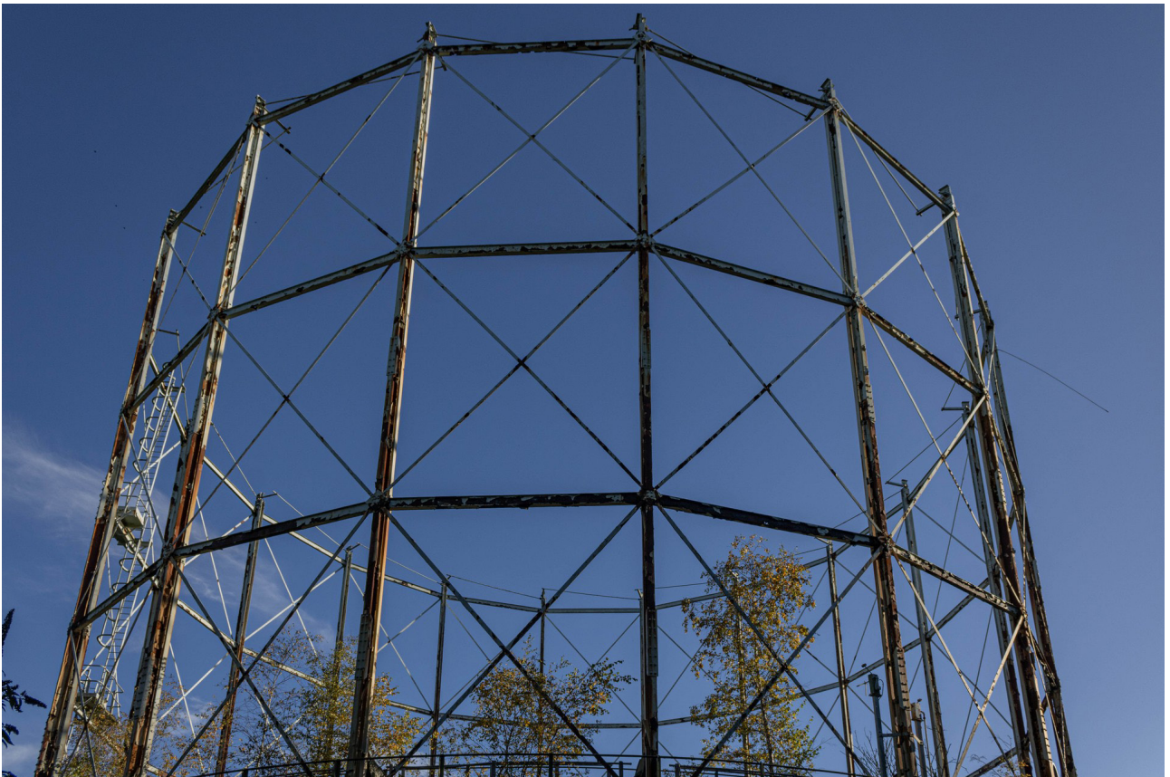
Plate 6: Gasholder No 3, general view of guide framing from the south-west
