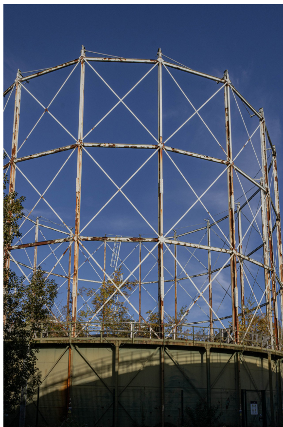
Plate 4: Gasholder No 3, general view of guide framing from the south-east
