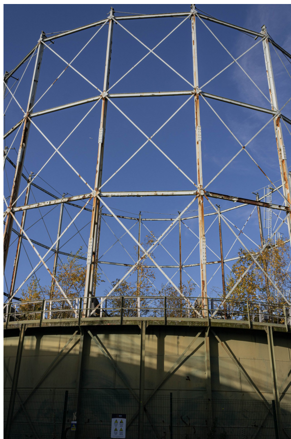
Plate 3: Gasholder No 3, general view of guide framing from the east
