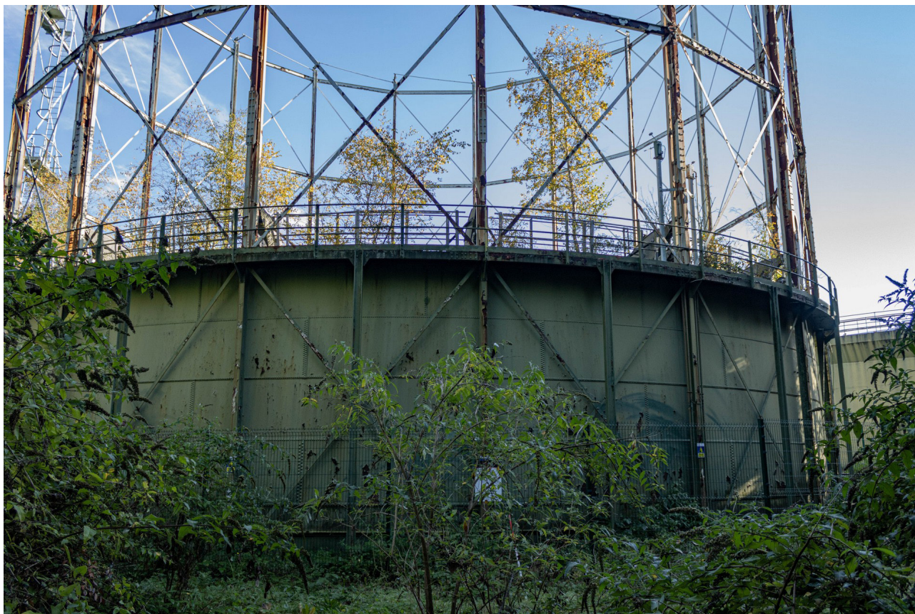
Plate 7: Gasholder No 3, general view from the south-west
