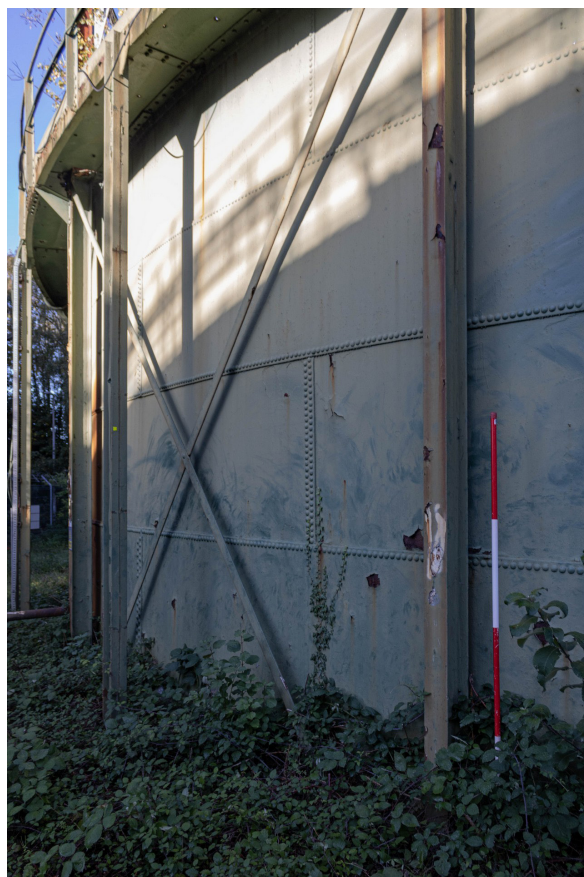
Plate 10: Gasholder No 3, detail of tank from the ESE
