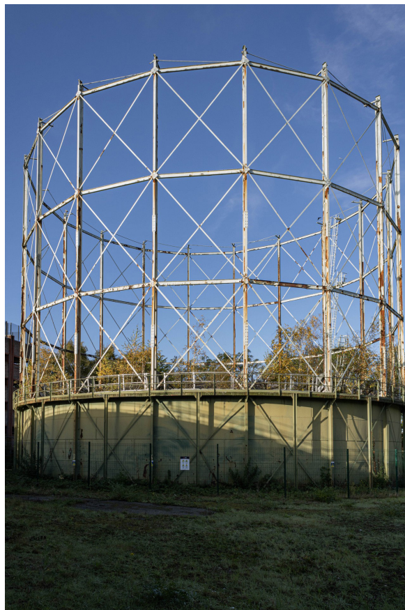
Plate 2: Gasholder No 3, general view from the east
