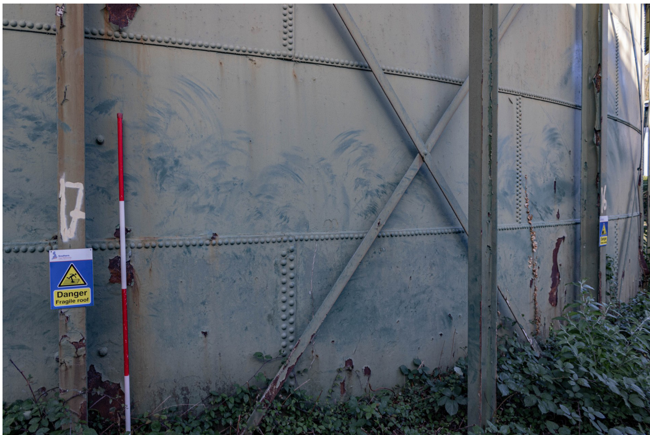
Plate 9: Gasholder No 3, detail of tank at Standard 17 from the south-west
