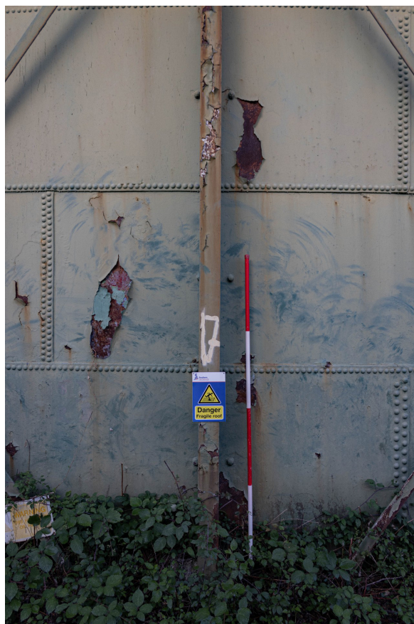
Plate 13: Gasholder No 3, detail of Standard 17 from the south-east
