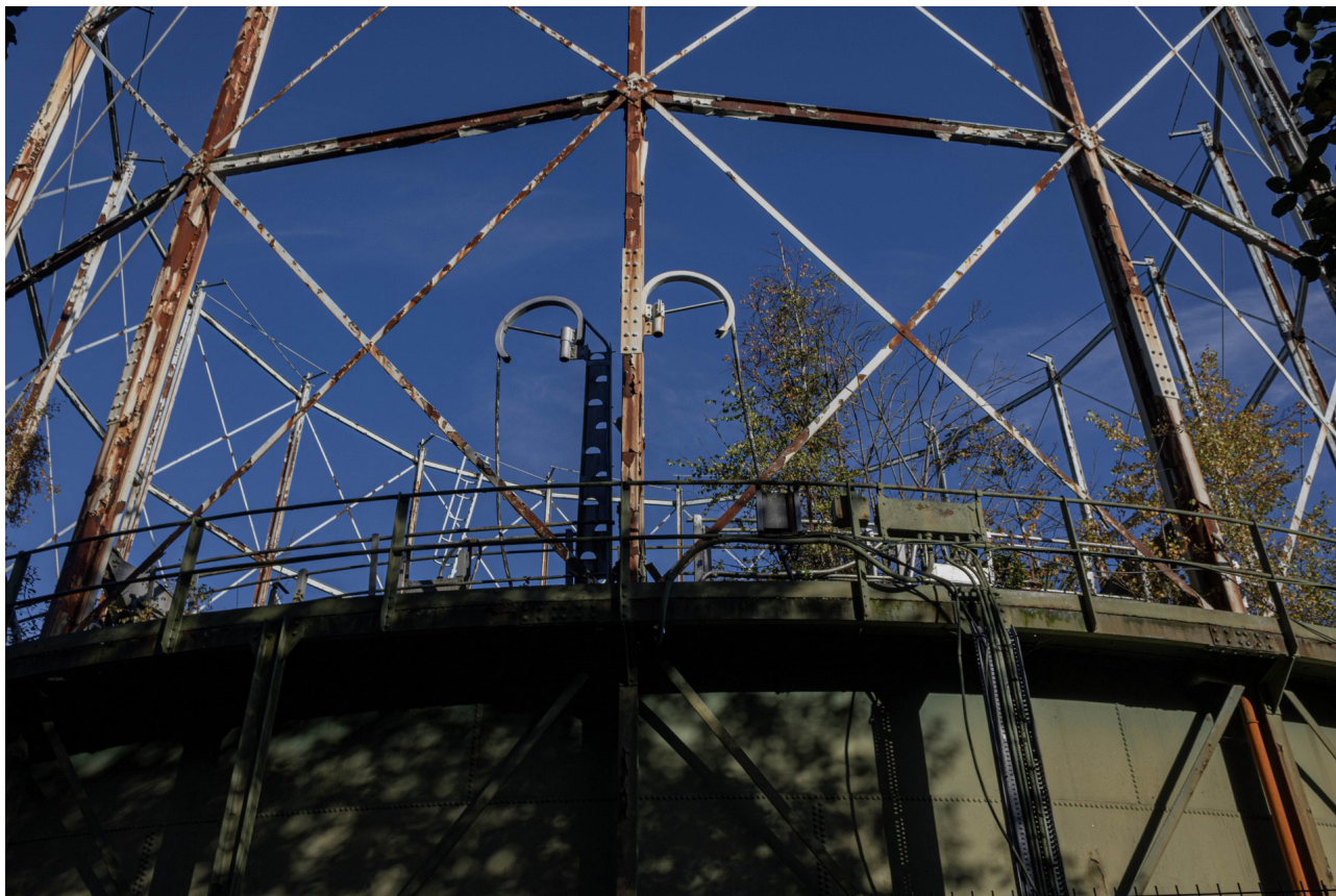
Plate 22: Gasholder No 3, detail of hose supports to the south side of the holder, from the south
