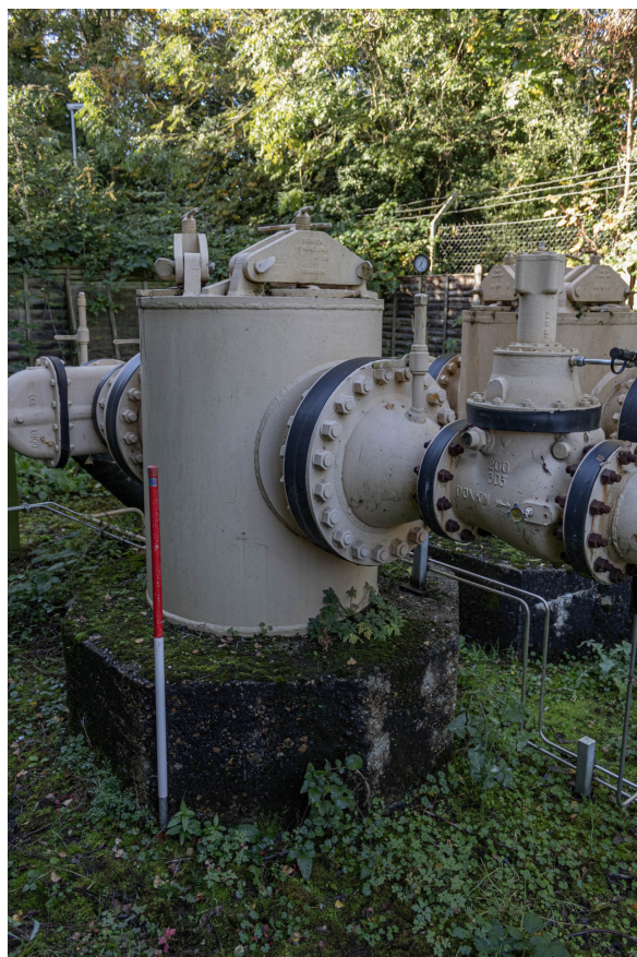
Plate 28: Gasholder No 3, detail of pipework from the NNW
