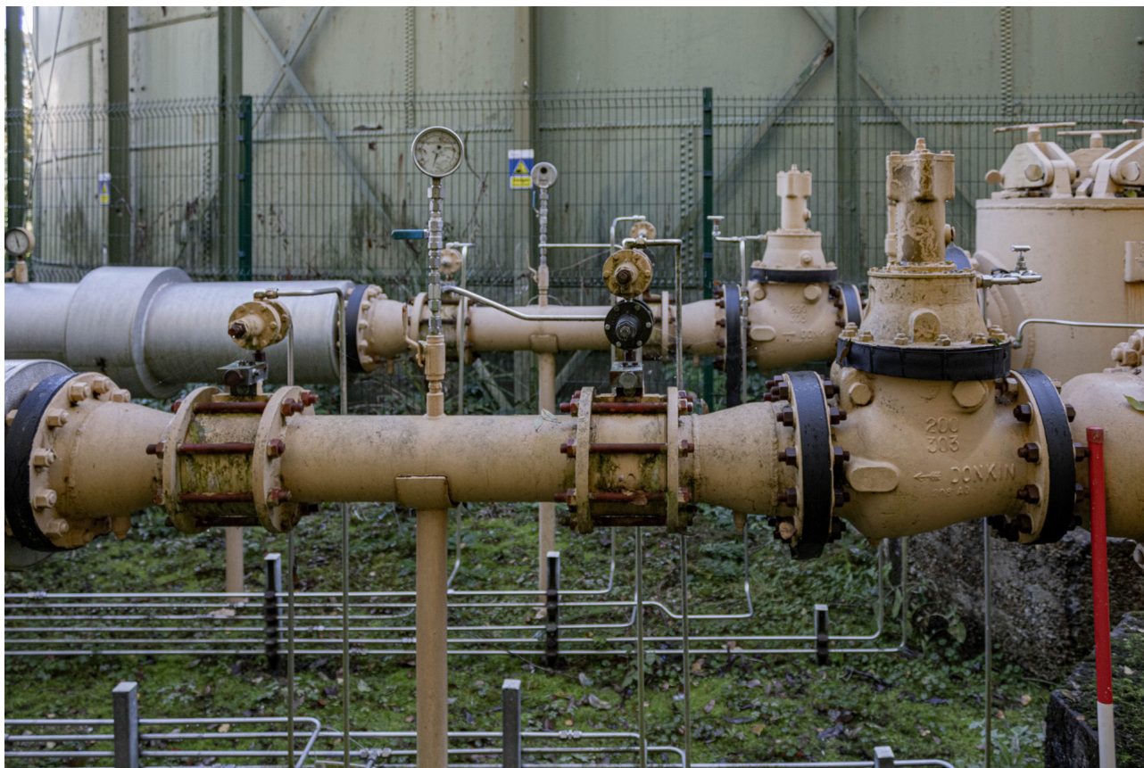
Plate 25: Gasholder No 3, detail of pipework from the north-west
