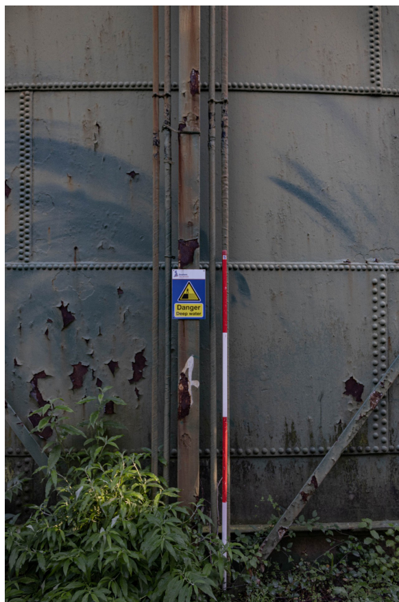
Plate 15: Gasholder No 3, detail of Standard 4 from the south-west
