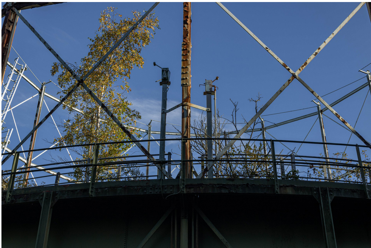
Plate 19: Gasholder No 3, detail of knock-off switches to the south-west of the holder from the south-west
