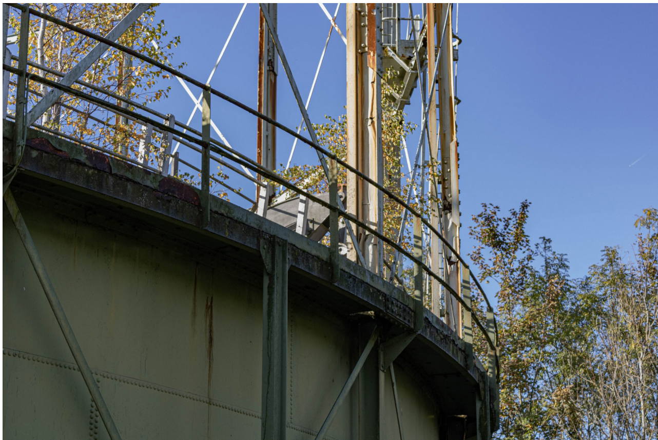
Plate 18: Gasholder No 3, detail of upper walkway from the ENE
