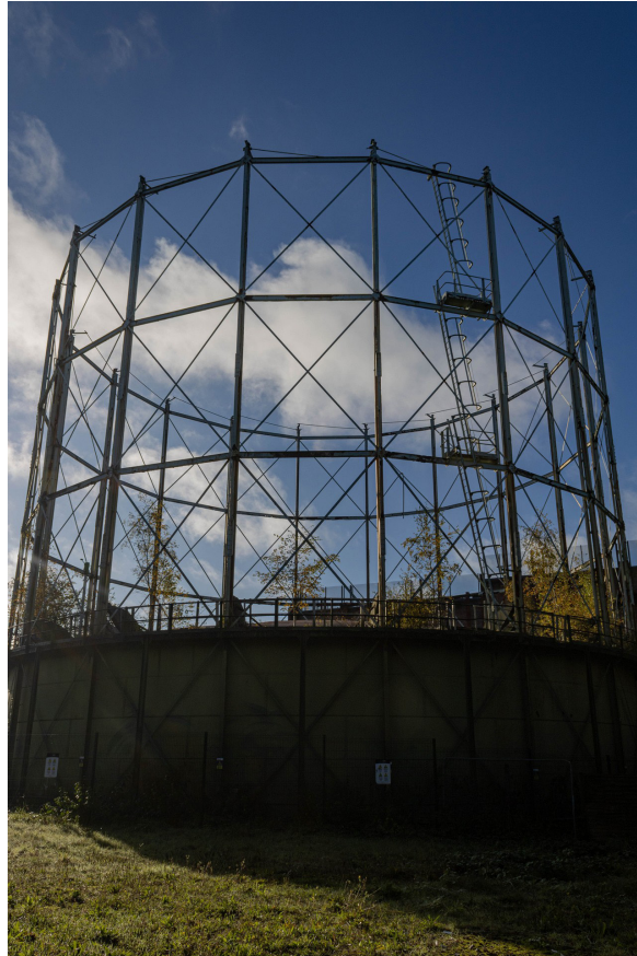
Plate 5: Gasholder No 3, general view from the north-east
