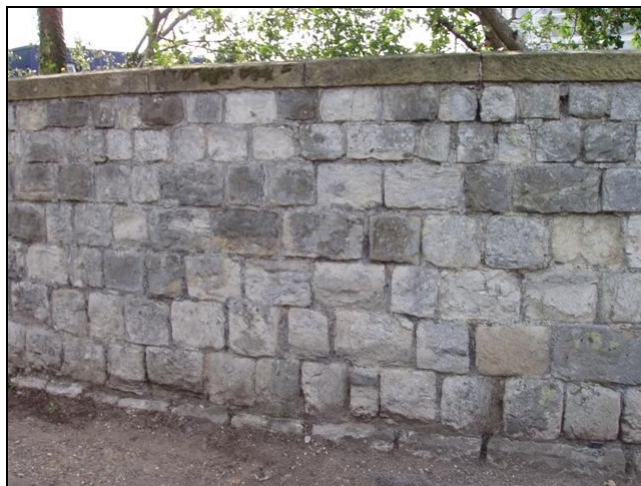
Plate 2: Stone section of wall
