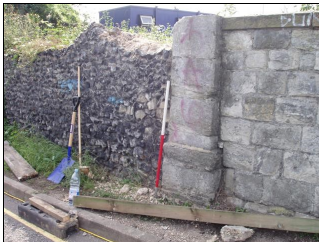
Plate 1: Flint area of wall, with stone pier
