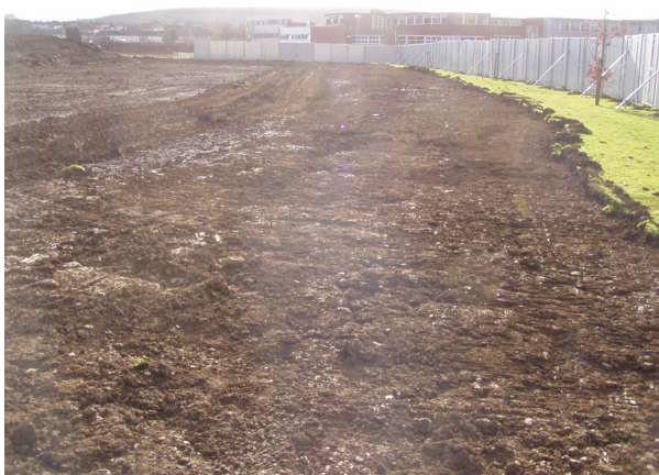
Plate 1: Topsoil Strip
