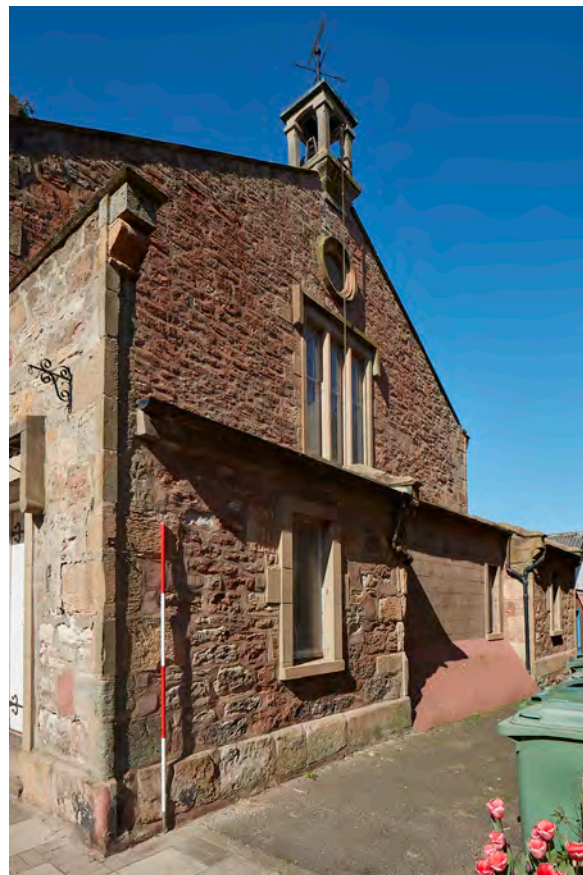
Plate 10: Cockenzie Old Parish Church, East Elevation, oblique view
