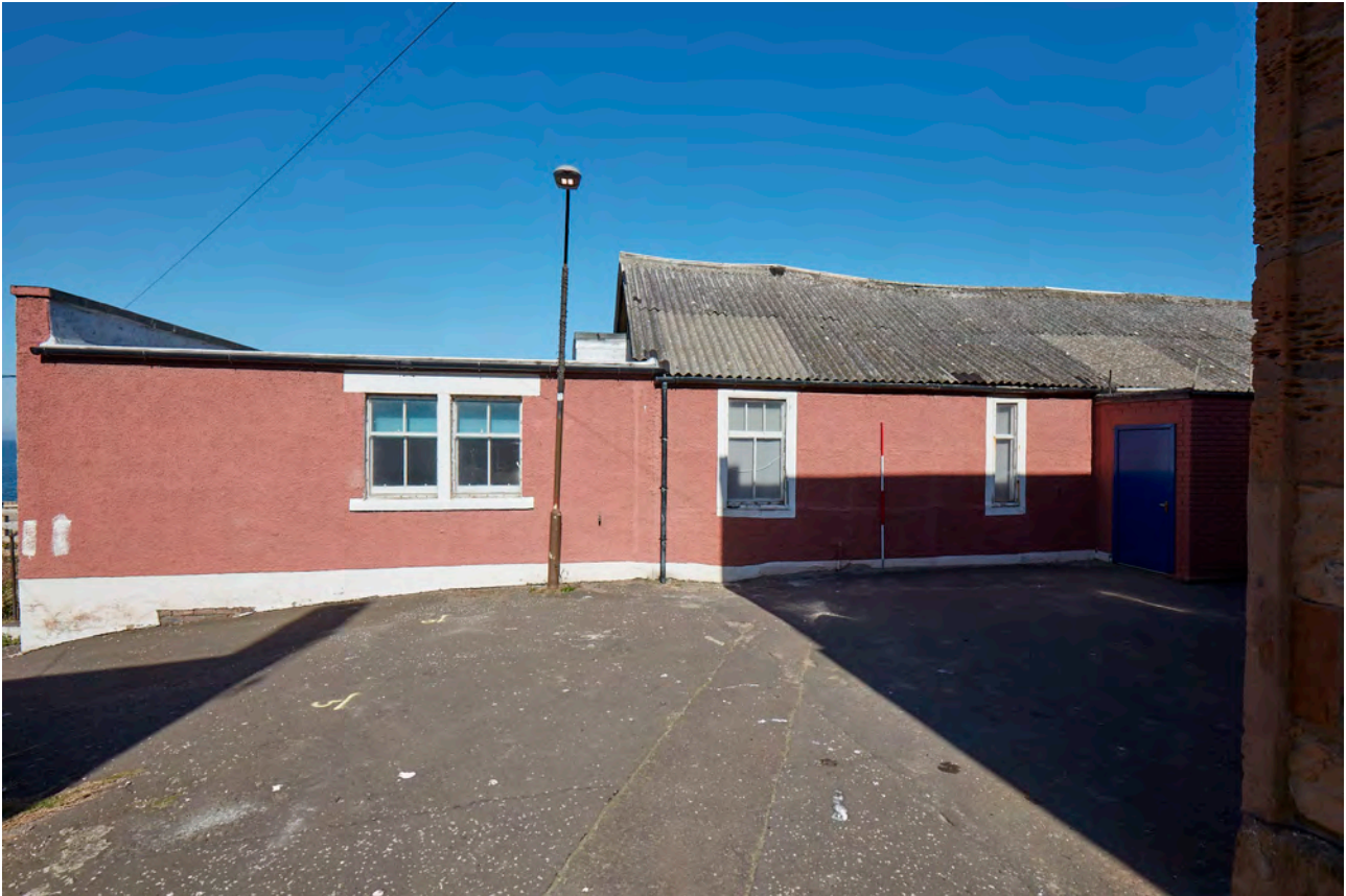
Plate 81: Cockenzie Church Hall, South Elevation, general view of west end
