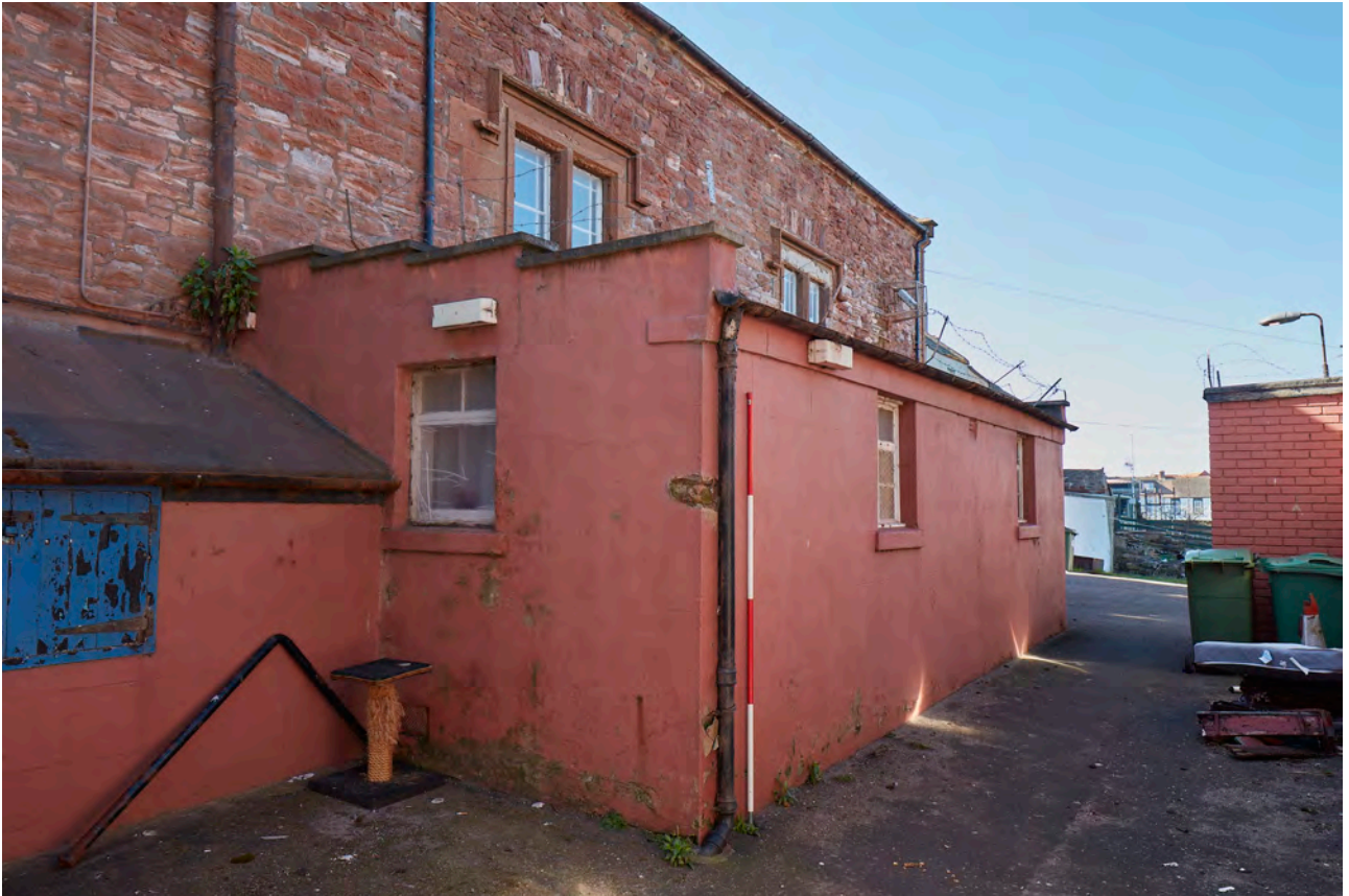
Plate 25: Cockenzie Old Parish Church, North Elevation, oblique view of lean-to vestry
