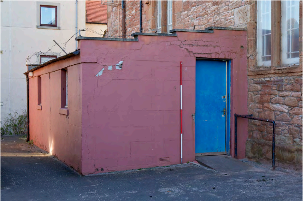
Plate 23: Cockenzie Old Parish Church, North Elevation, general view
