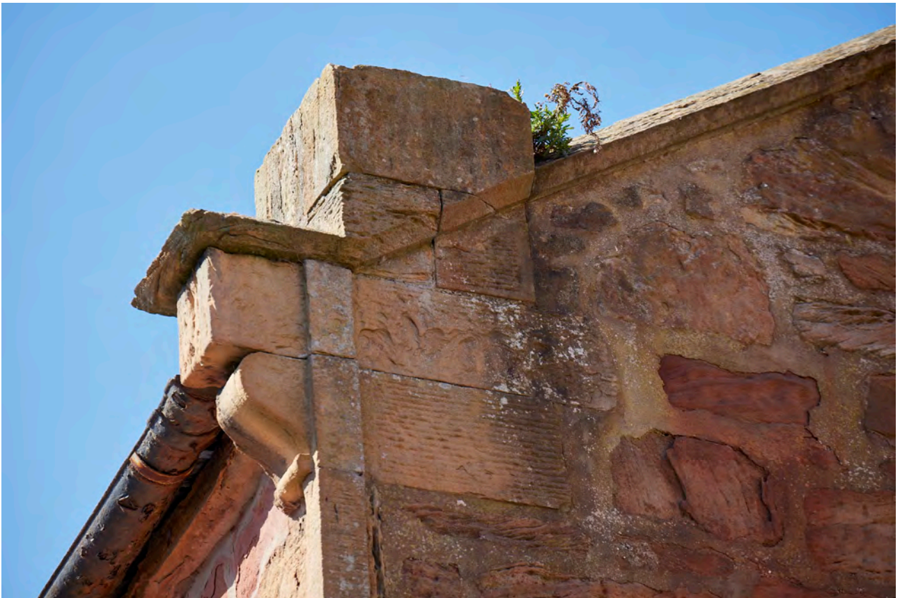
Plate 34: Cockenzie Old Parish Church, East Elevation, detail of skew putt
