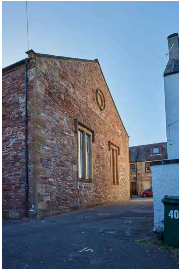
Plate 29: Cockenzie Old Parish Church, West Elevation, oblique view
