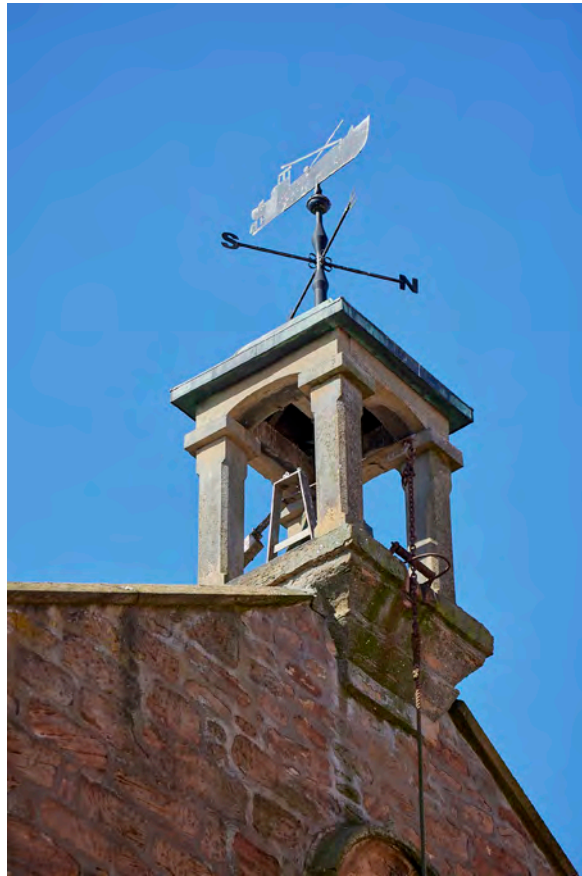
Plate 13: Cockenzie Old Parish Church, East Elevation, detail of bellcote
