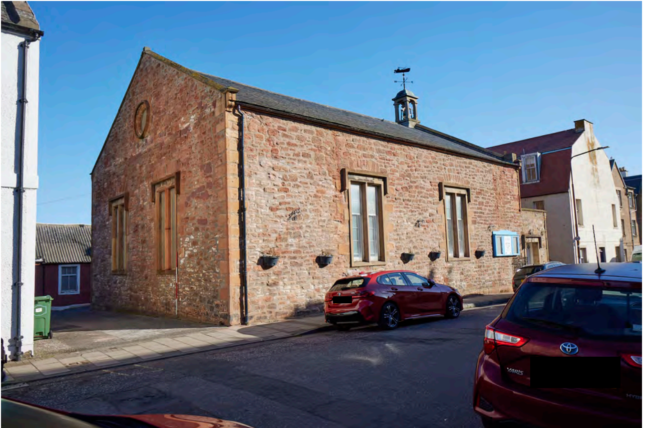
Plate 1: Cockenzie Old Parish Church, South Elevation, oblique view
