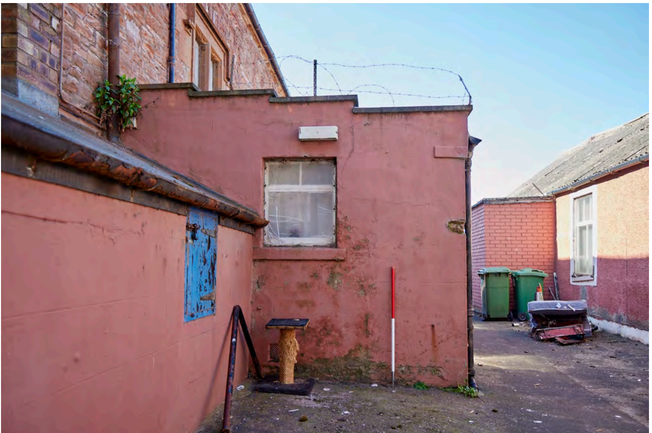
Plate 26: Cockenzie Old Parish Church, North Elevation, general view of lean-to
