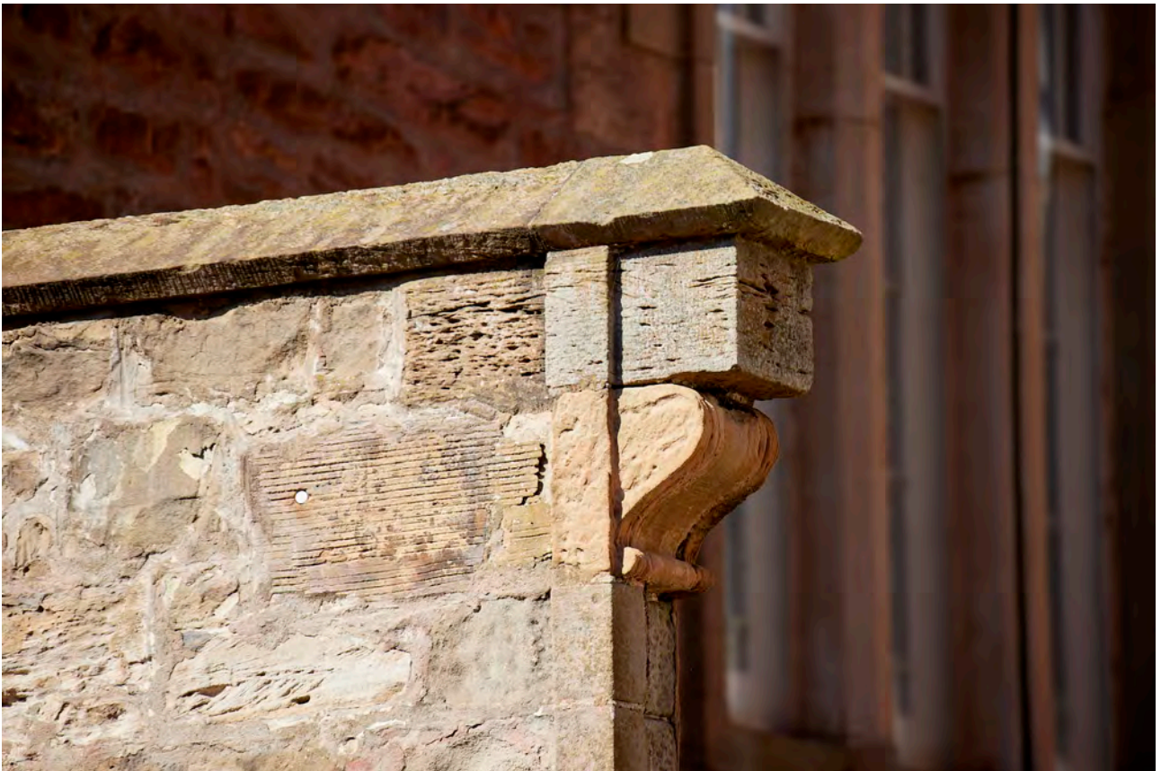
Plate 6: Cockenzie Old Parish Church, South Elevation, detail of consoled skew putt
