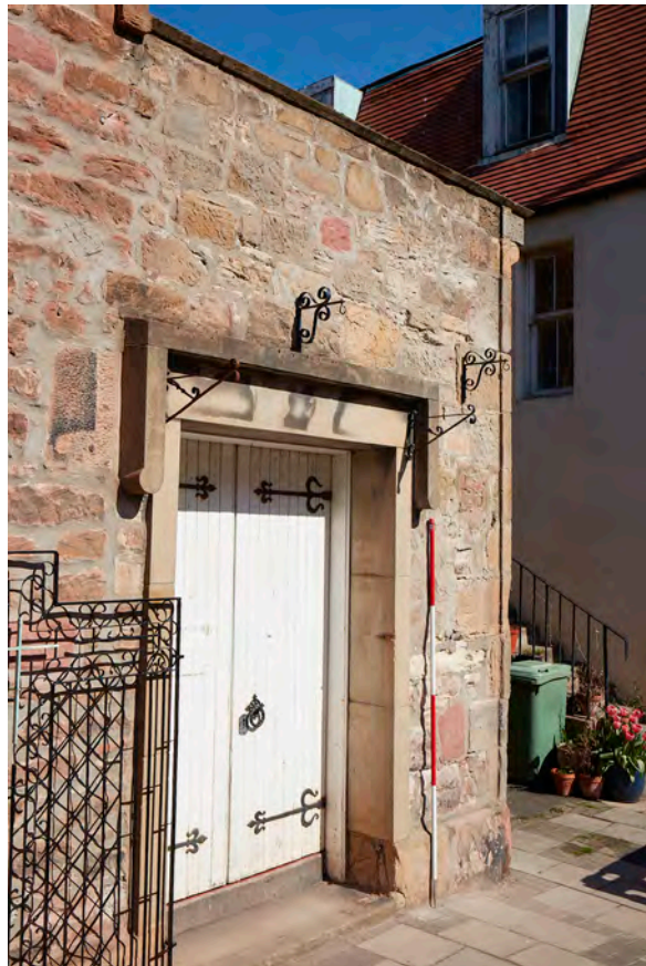
Plate 4: Cockenzie Old Parish Church, South Elevation, detail of eastern main entrance doorway
