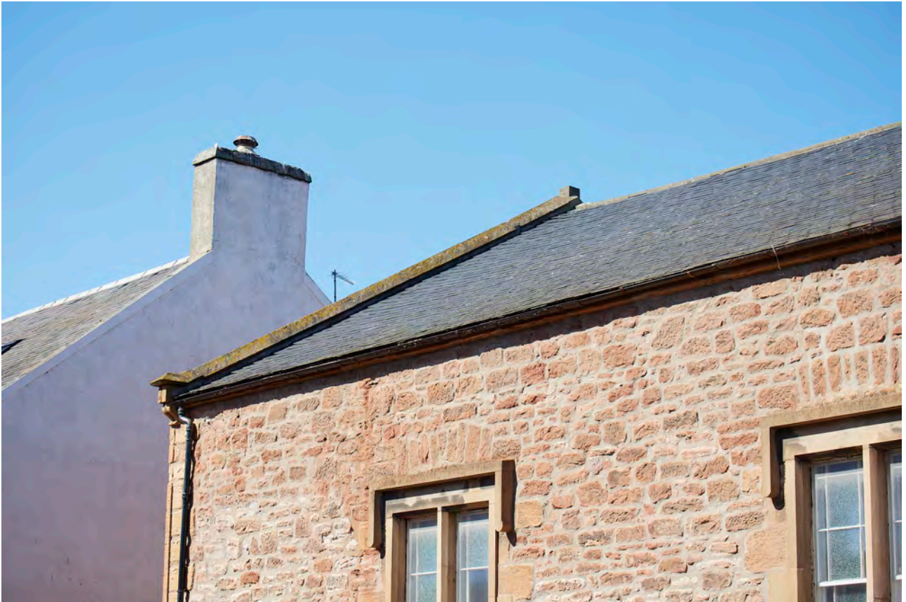
Plate 33: Cockenzie Old Parish Church, Roof, oblique view of skews
