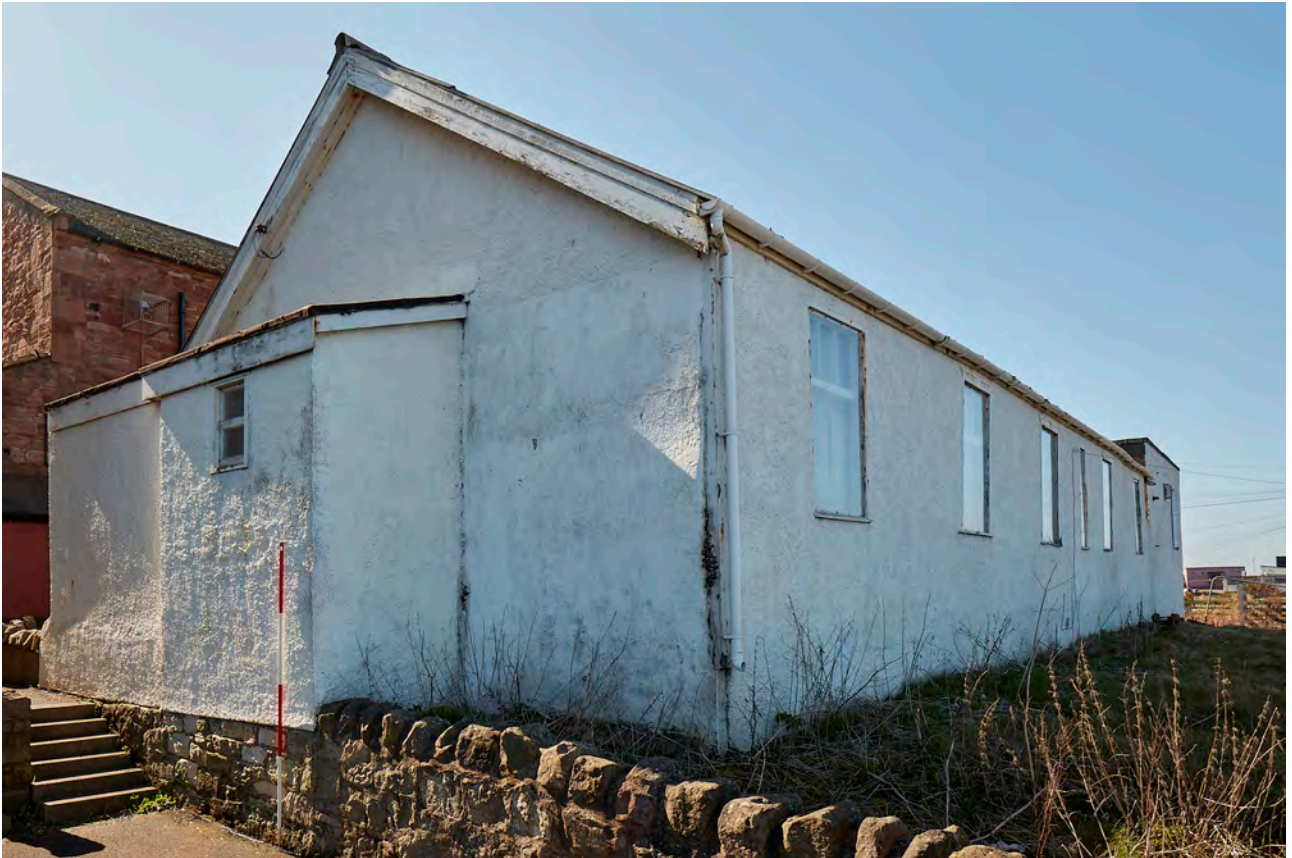
Plate 77: Cockenzie Church Hall, East Elevation, oblique view
