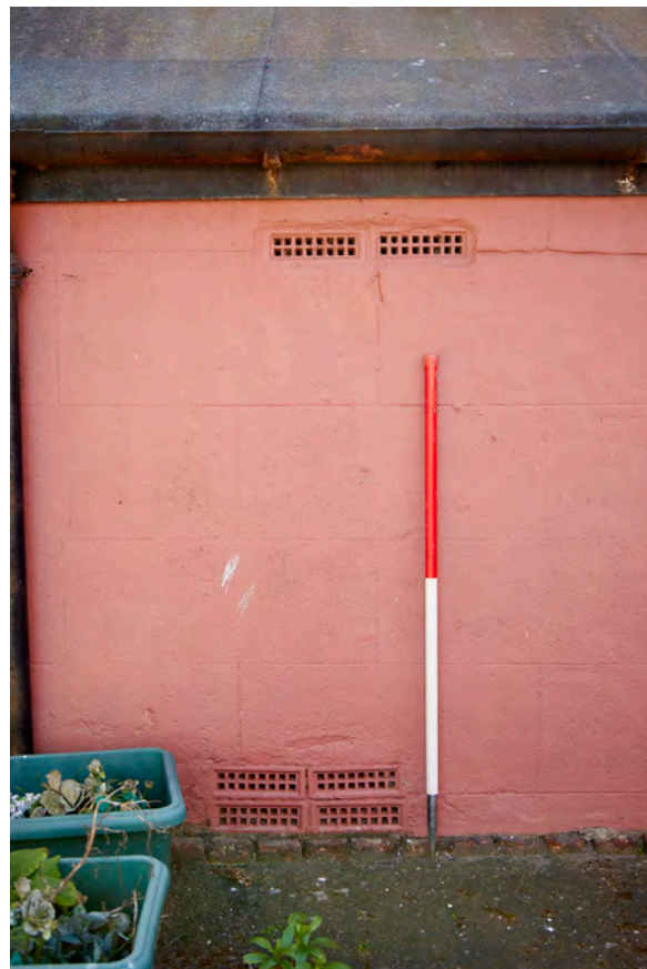
Plate 24: Cockenzie Old Parish Church, North Elevation, detail of vents in the lean-to elevation
