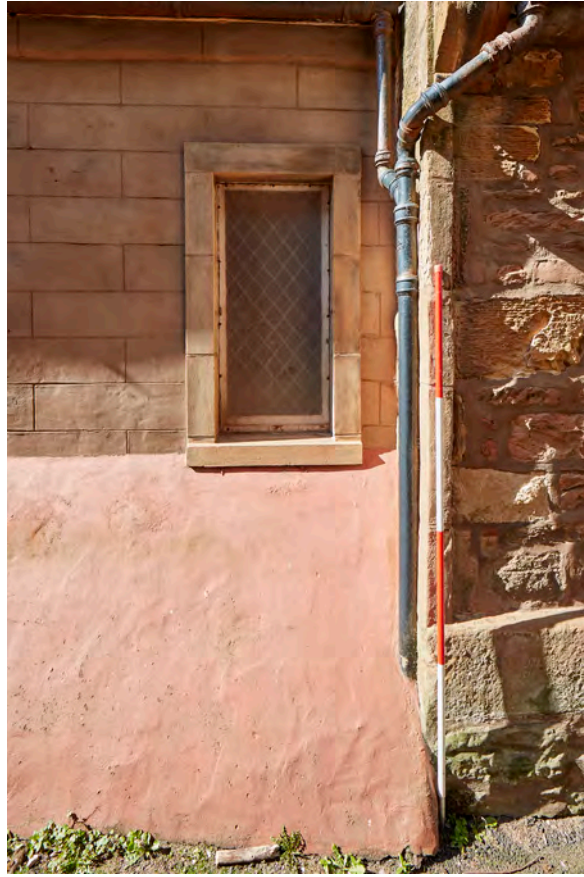
Plate 17: Cockenzie Old Parish Church, East Elevation, detail of batter and window
