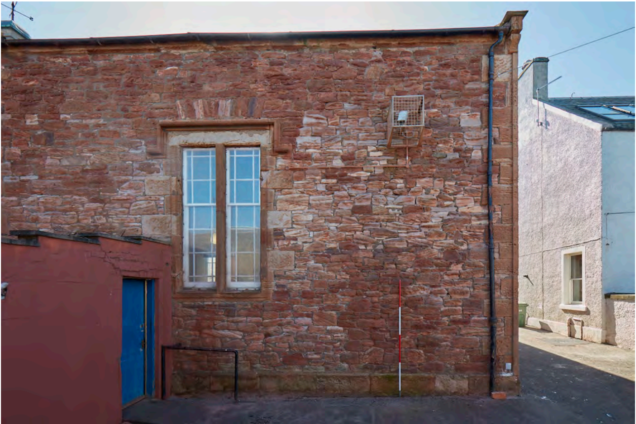
Plate 21: Cockenzie Old Parish Church, North Elevation, general view of west end
