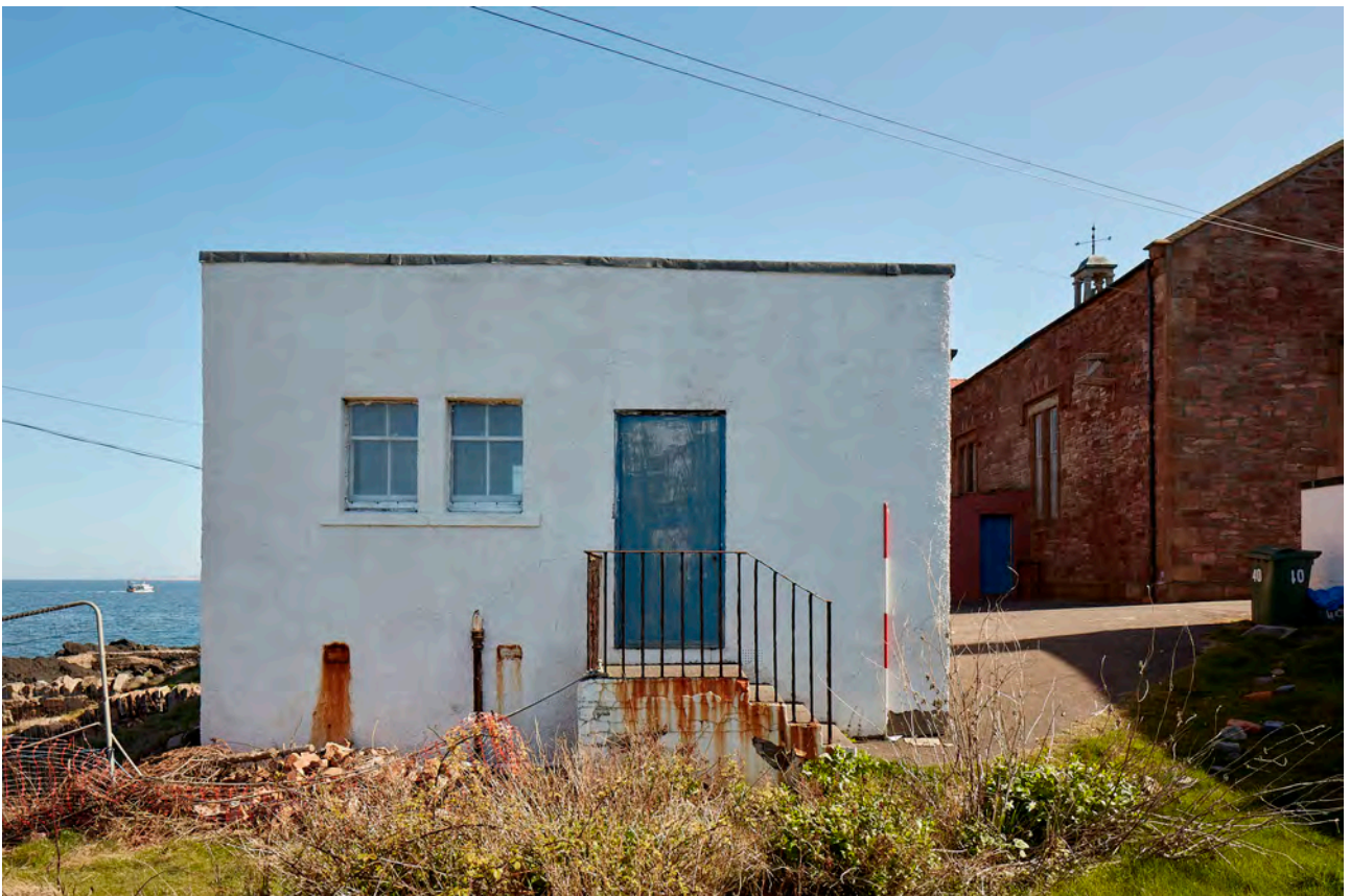
Plate 78: Cockenzie Church Hall, West Elevation, general view
