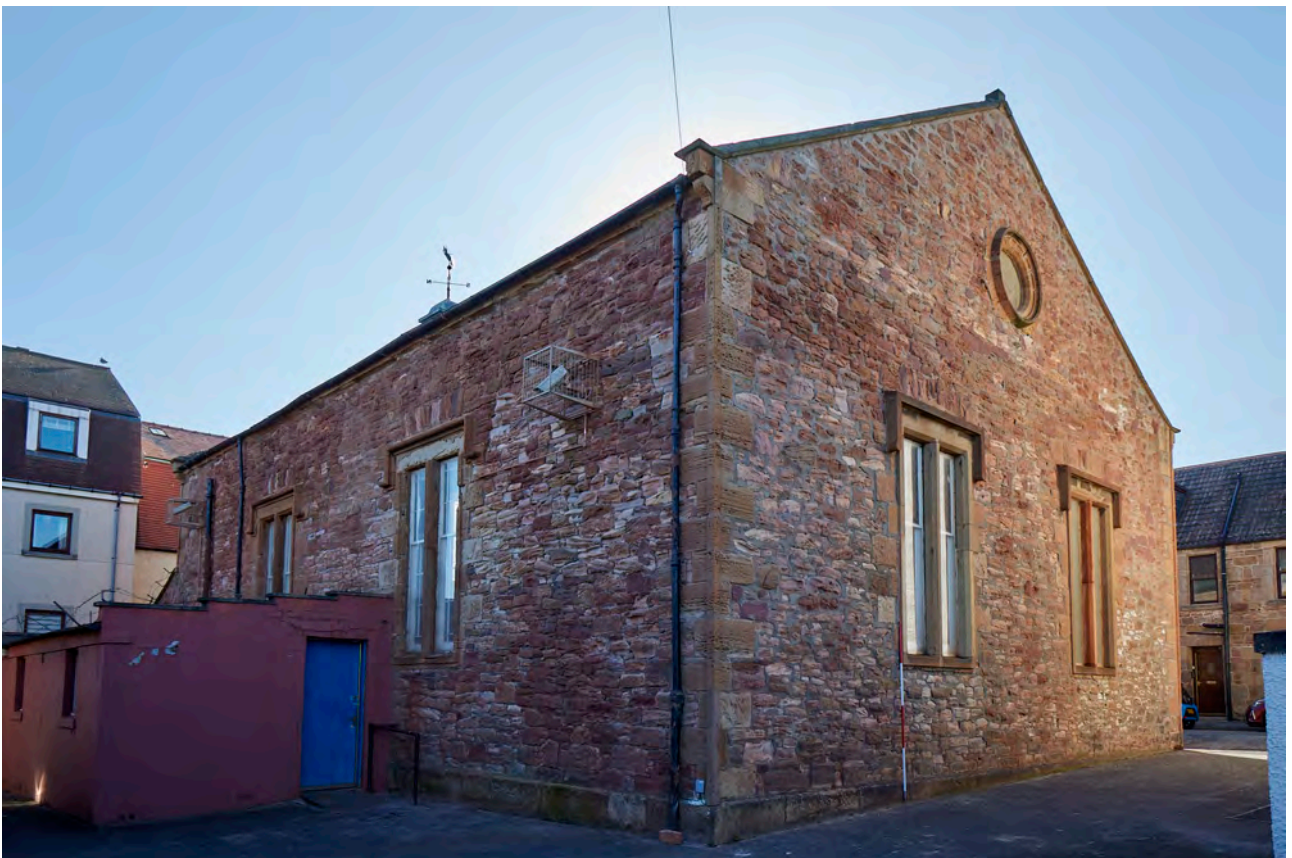
Plate 20: Cockenzie Old Parish Church, West and North Elevations, oblique view
