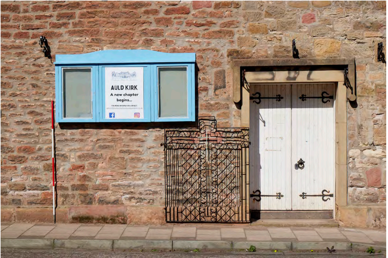
Plate 5: Cockenzie Old Parish Church, South Elevation, general view of eastern main entrance doorway, gate and sign
