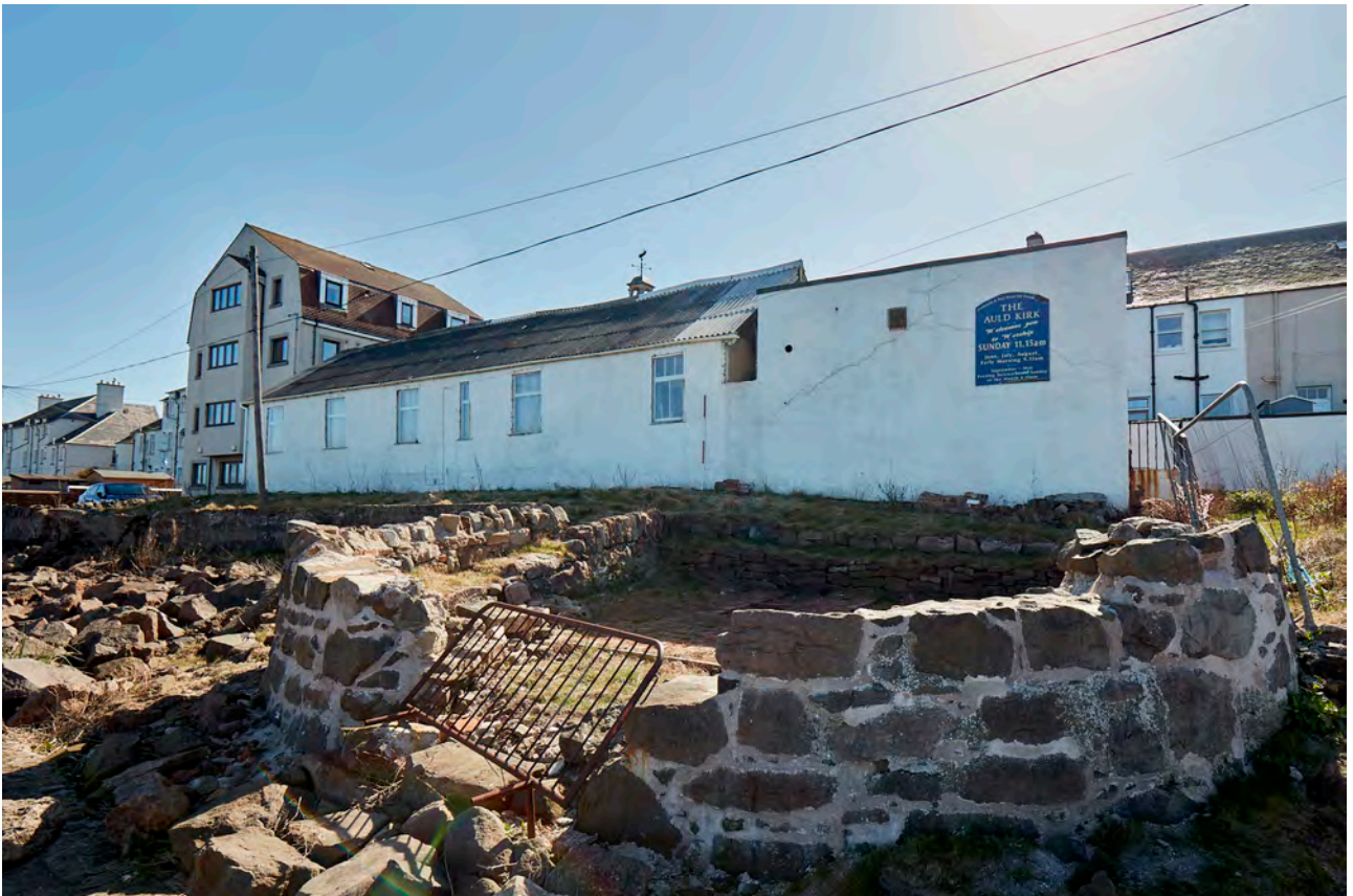
Plate 76: Cockenzie Church Hall, North Elevation, oblique view
