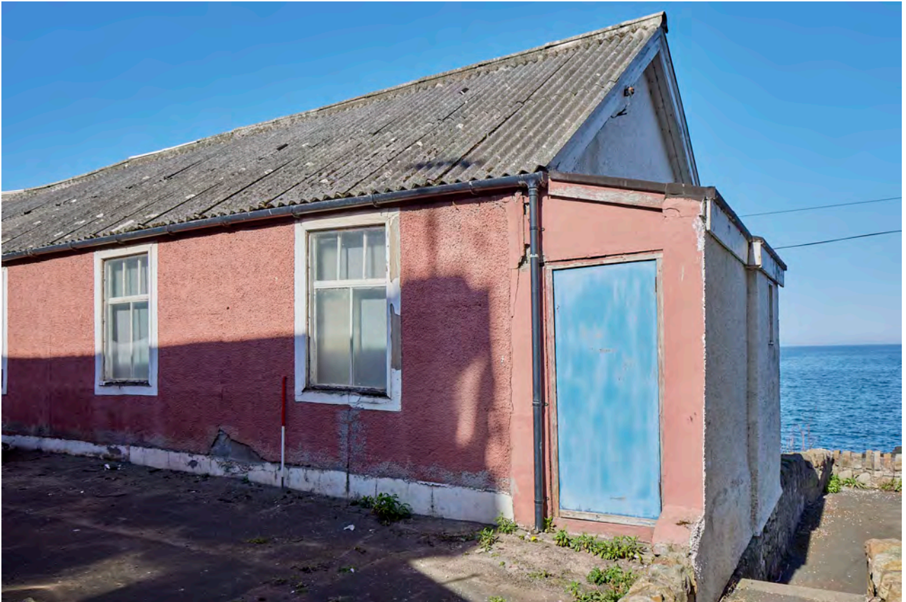
Plate 79: Cockenzie Church Hall, South Elevation, general view of east end
