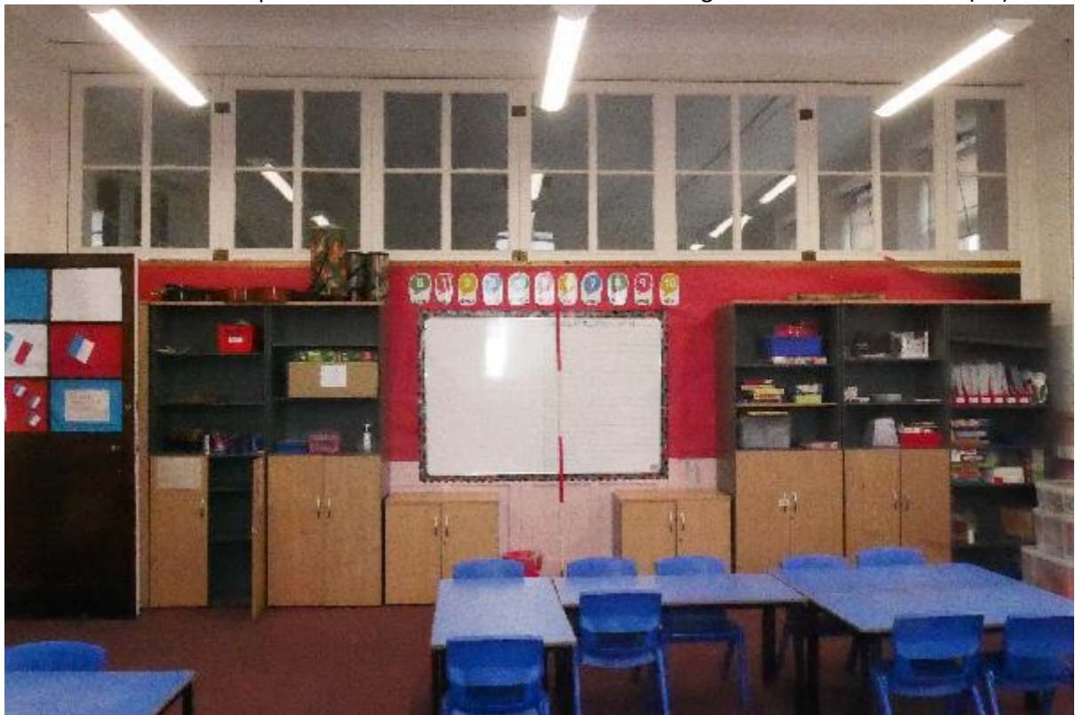
Illustration 80- Internal North facing elevation of Classroom (18) showing original folding dividing wall.
