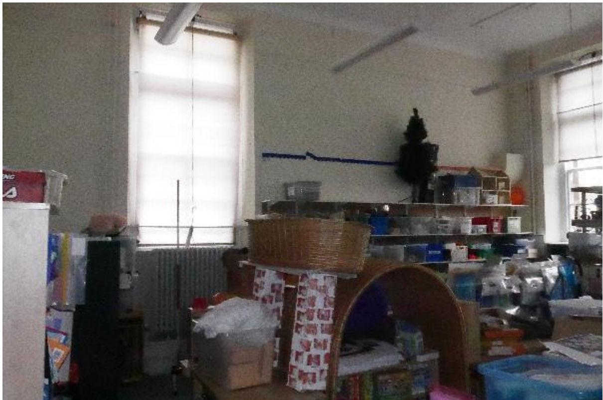
Illustration 59- Glazed window in internal West facing elevation of Classroom (13).
