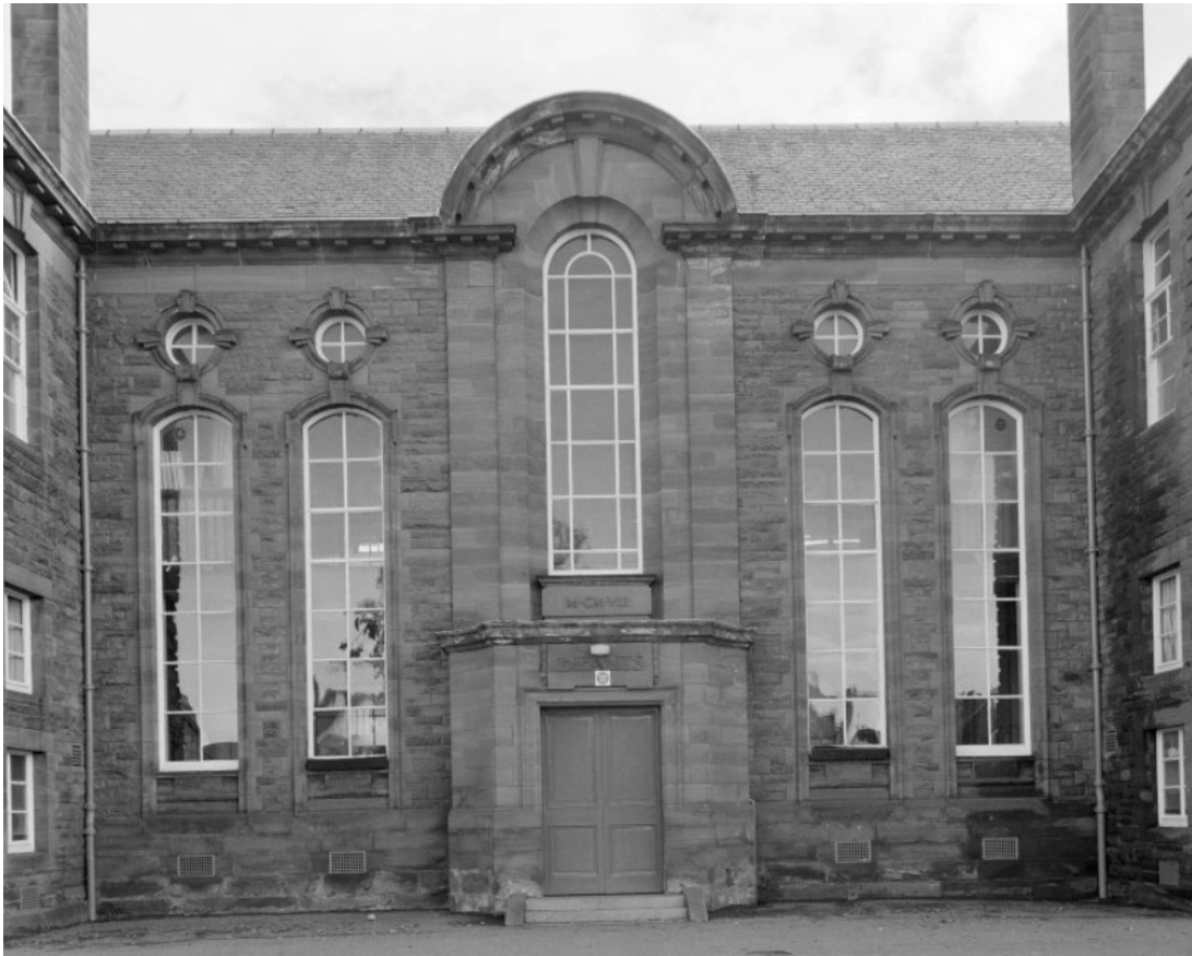
Plate 11: Detailed view of the stonework of the central bay on the north-west facing elevation pre-demolition (© Crown Copyright: HES)
