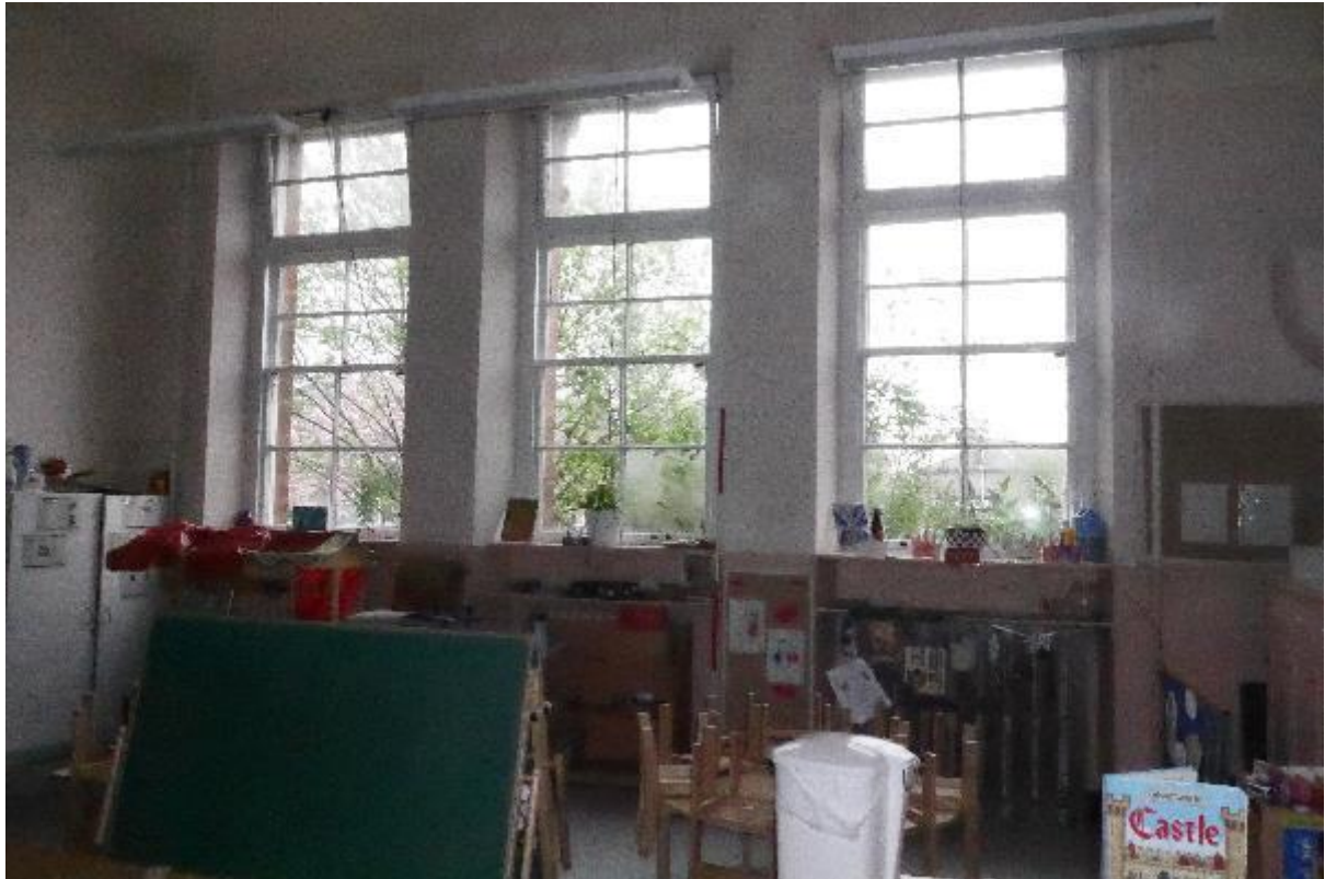
Illustration 62- Glazed windows in internal West facing elevation of Classroom (14).
