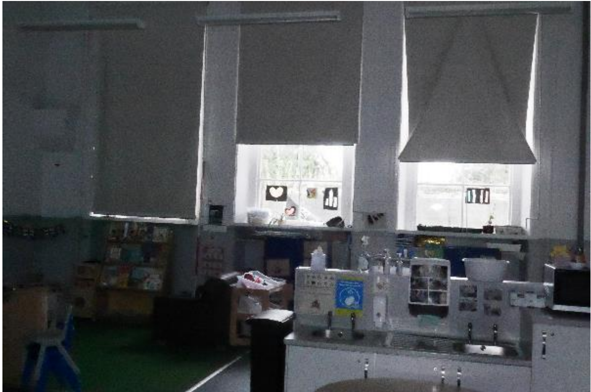
Illustration 47- North facing elevation of Classroom (10) showing glazed windows.
