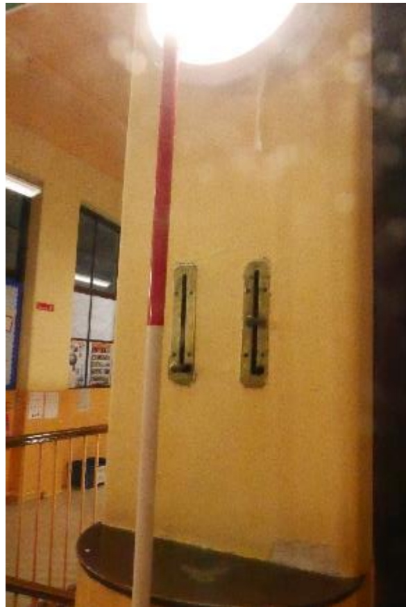
Illustration 91 - Ventilation controls (brass) in lobby (21).
