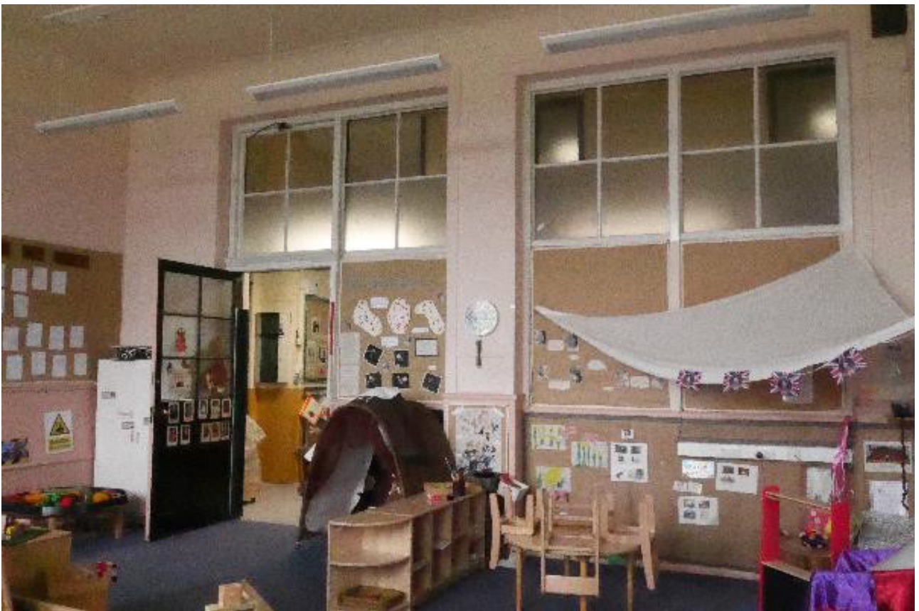
Plate 66: General view of the south-west wall in Room 0/18, looking south-west (© Derek Hall 2023)
