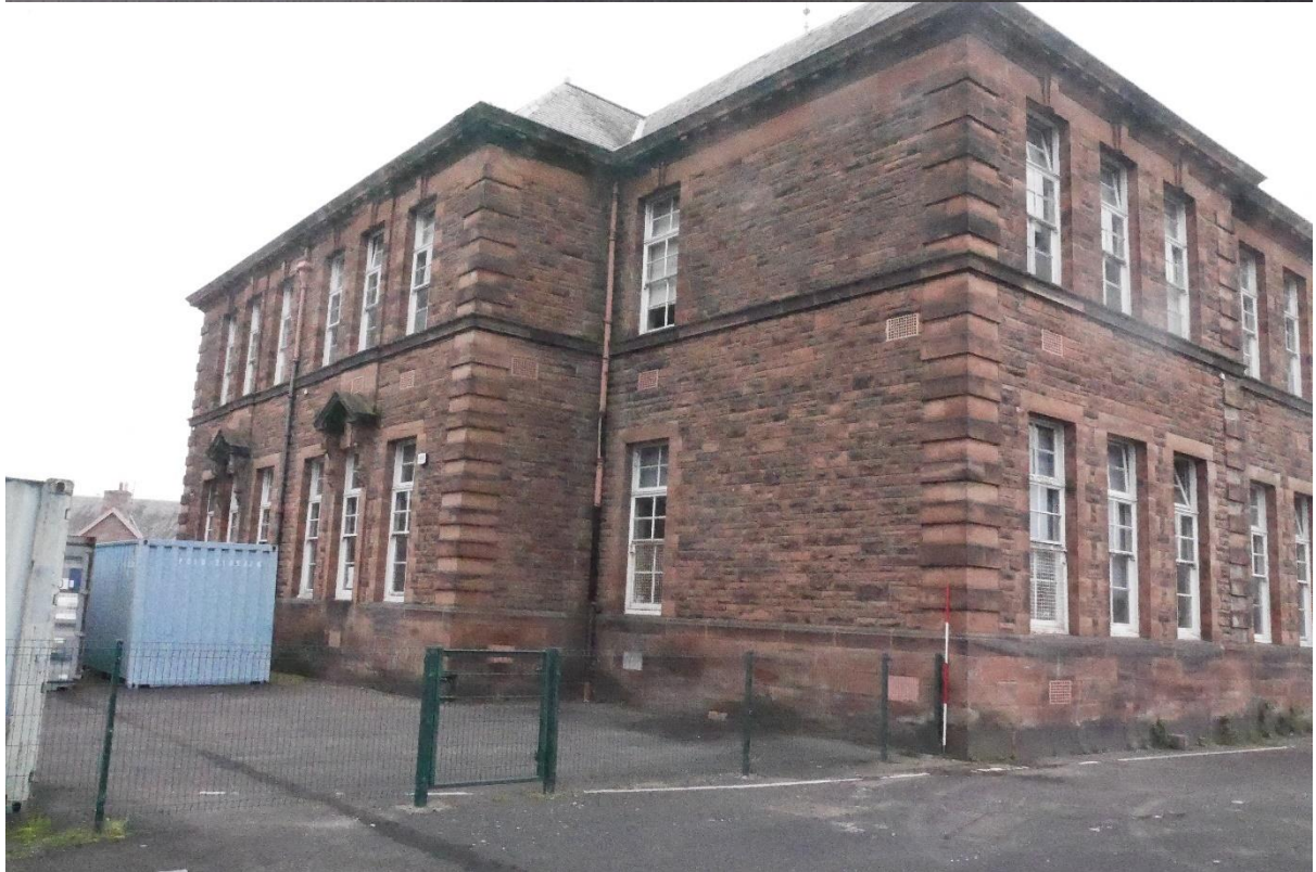
Illustration 7 – West facing external elevation of Balhousie Primary School, top looking South East bottom looking North East (2023).
