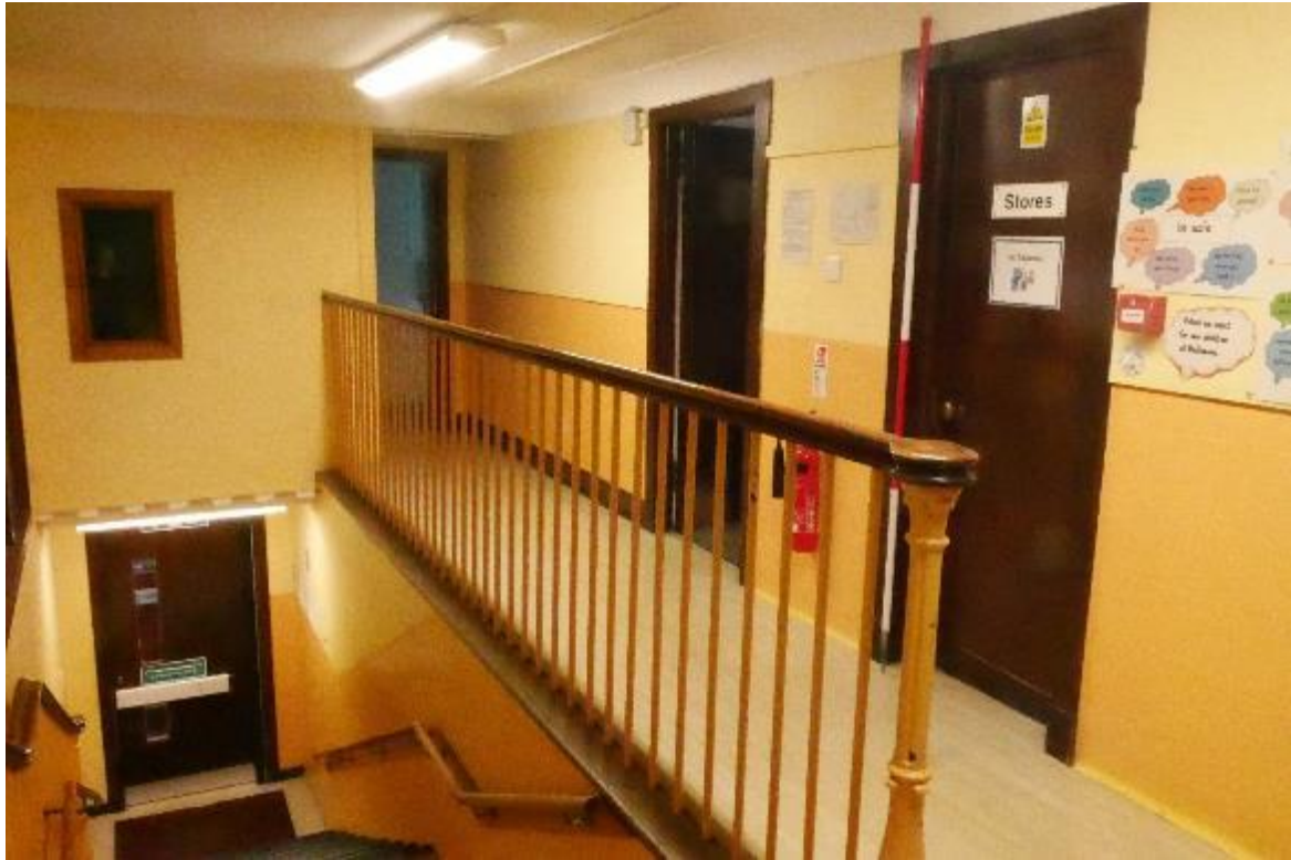
Illustration 71- General view of head teachers' office (a), stores (b) and toilets (c) on Mezzanine level at Western end of the building.
