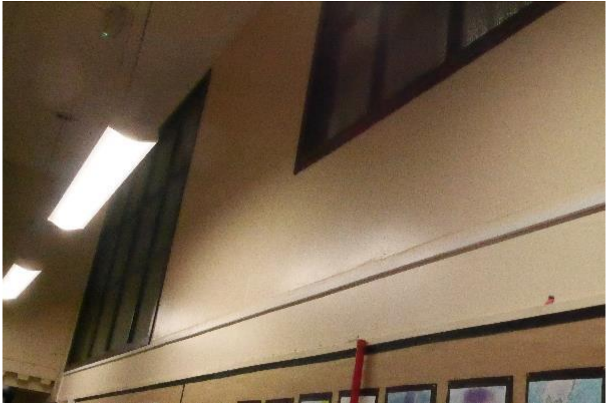
Illustration 16- timber framed windows in West facing internal elevation of corridor (1).
