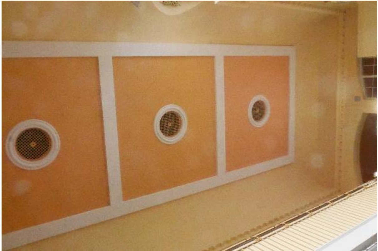
Illustration 42- Ceiling of Hall (7) showing ventilation grilles and moulding.
