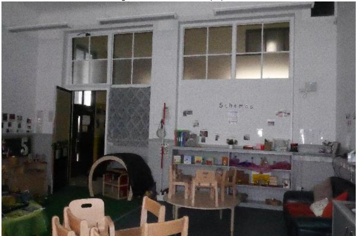
Illustration 55- Internal South facing elevation of Classroom (12) showing glazed windows, doorway, half-timbered panelling and shelving.
