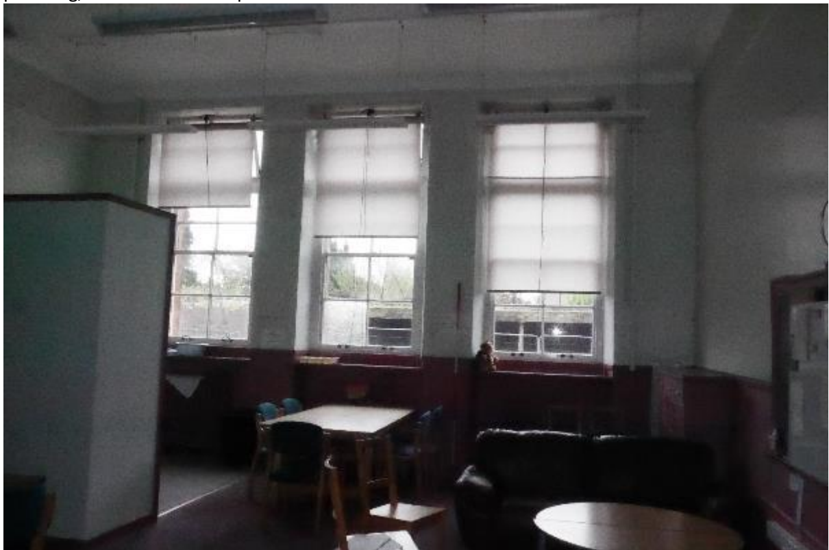
Illustration 34- Glazed windows in North facing elevation of Staff Room (6).
