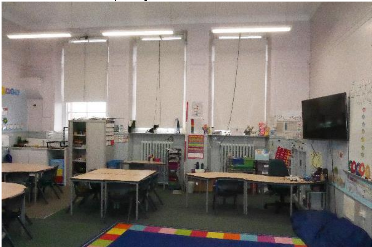
Illustration 97- Internal North facing elevation of Classroom (23) showing glazed windows and half-timbered panelling.
