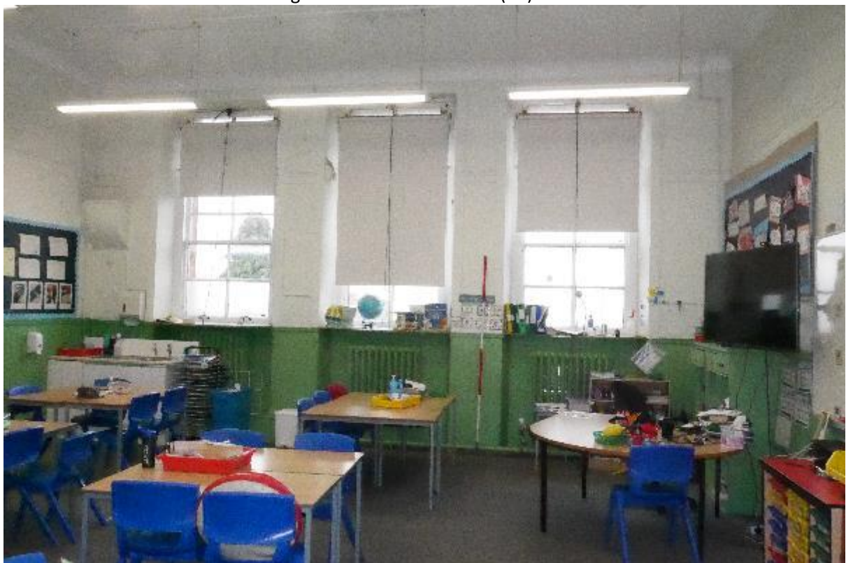
Illustration 107- Internal North facing elevation of Classroom (26) showing glazed windows and half-timbered wall.
