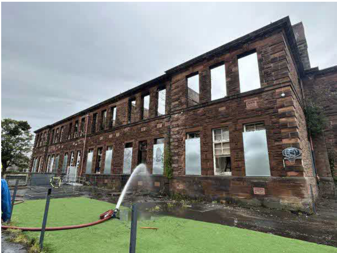
Plate 18: General view of south-east facing elevation pre-demolition, looking west (© G3 Consulting Engineers 2025)
