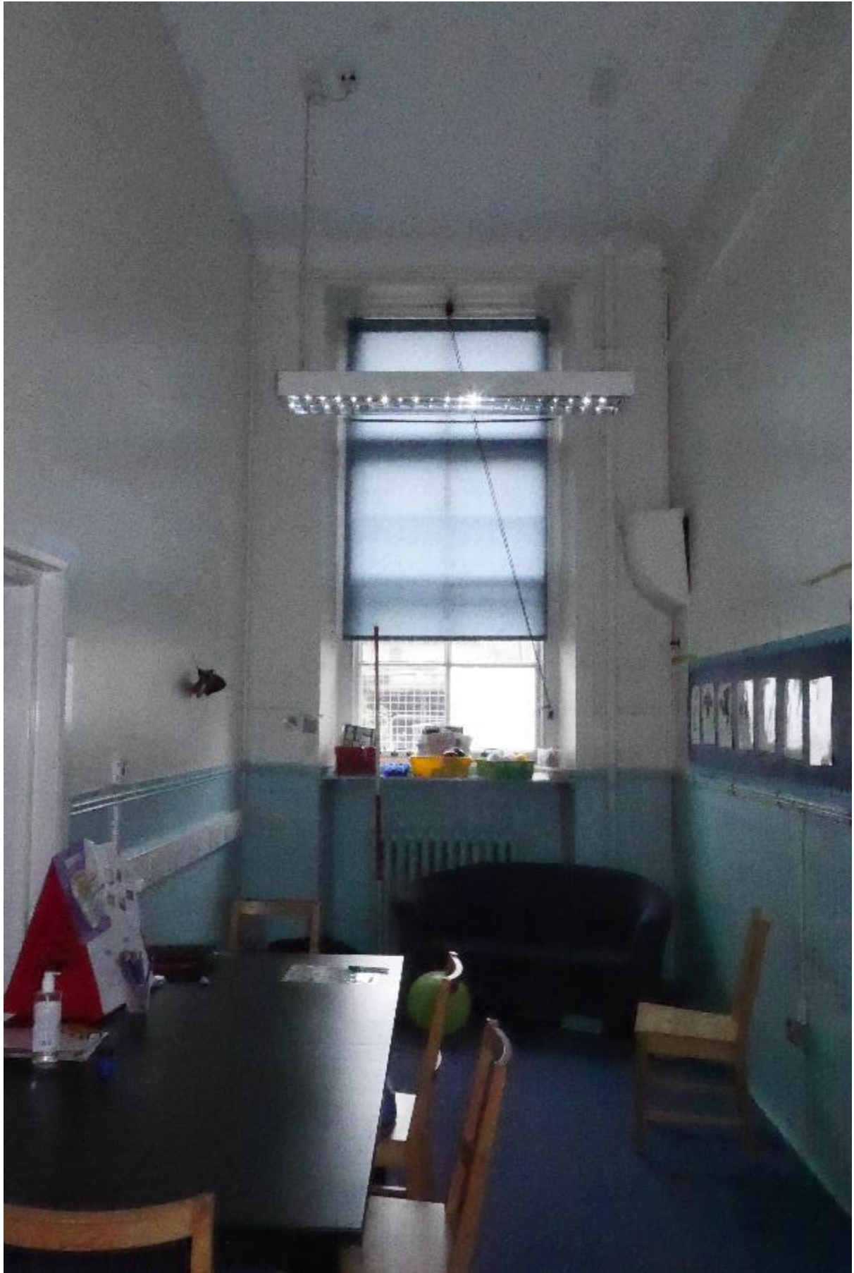
Illustration 25- Glazed window in internal North facing elevation of Meeting Room (4).
