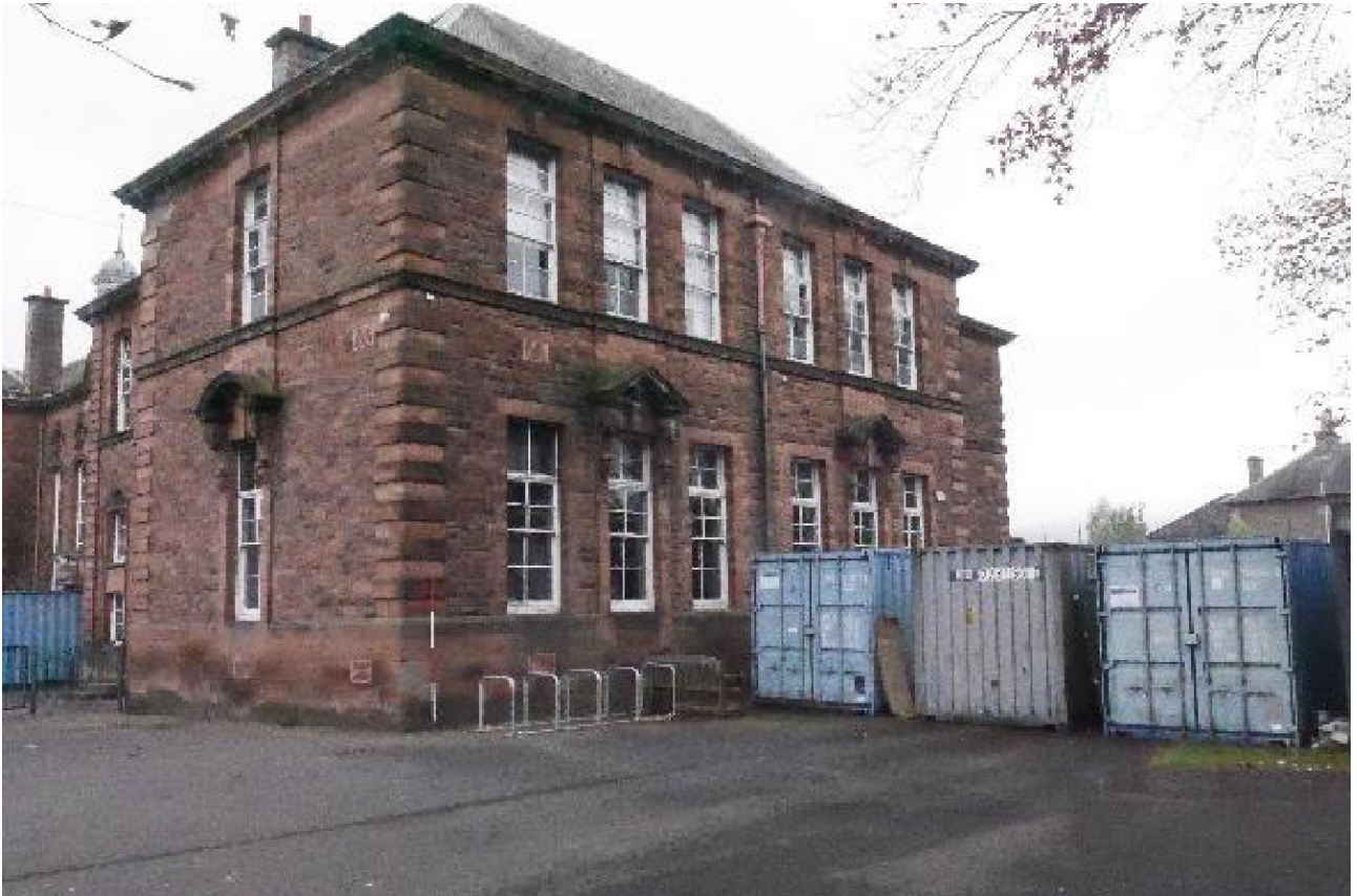
Plate 13: General view of the south-west facing elevation, looking south-east (© Derek Hall 2023)
