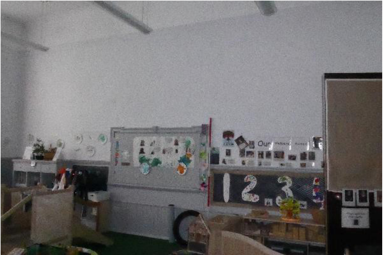
Plate 63: General view of the south-west wall in Room 0/16, looking south-west (© Derek Hall 2023)
