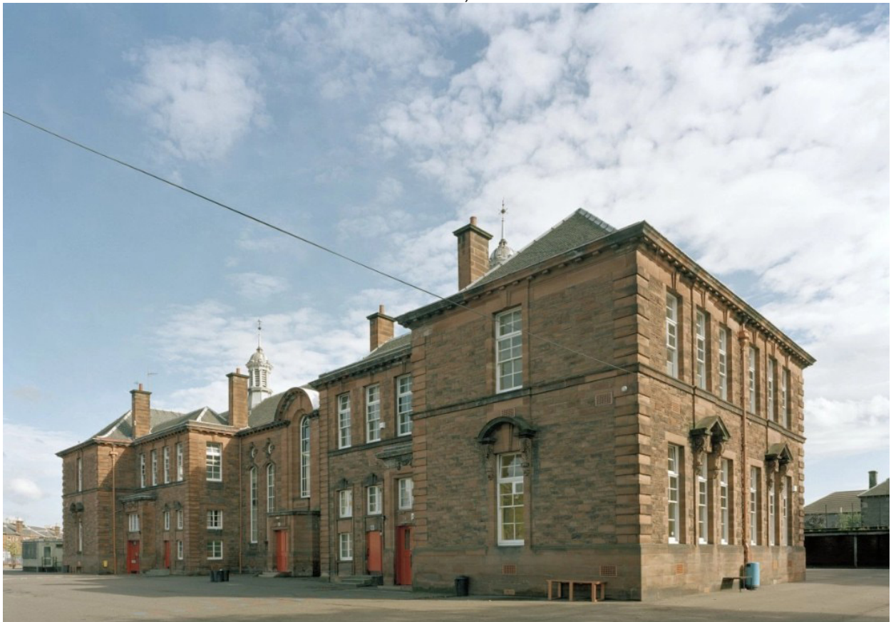
Plate 4: General view of the north-west facing elevation, looking east (©Crown Copyright: HES)
