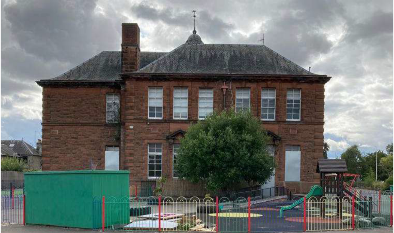
Plate 19: General view of the north-east elevation, looking south-west (© Perth and Kinross Council 2023)
