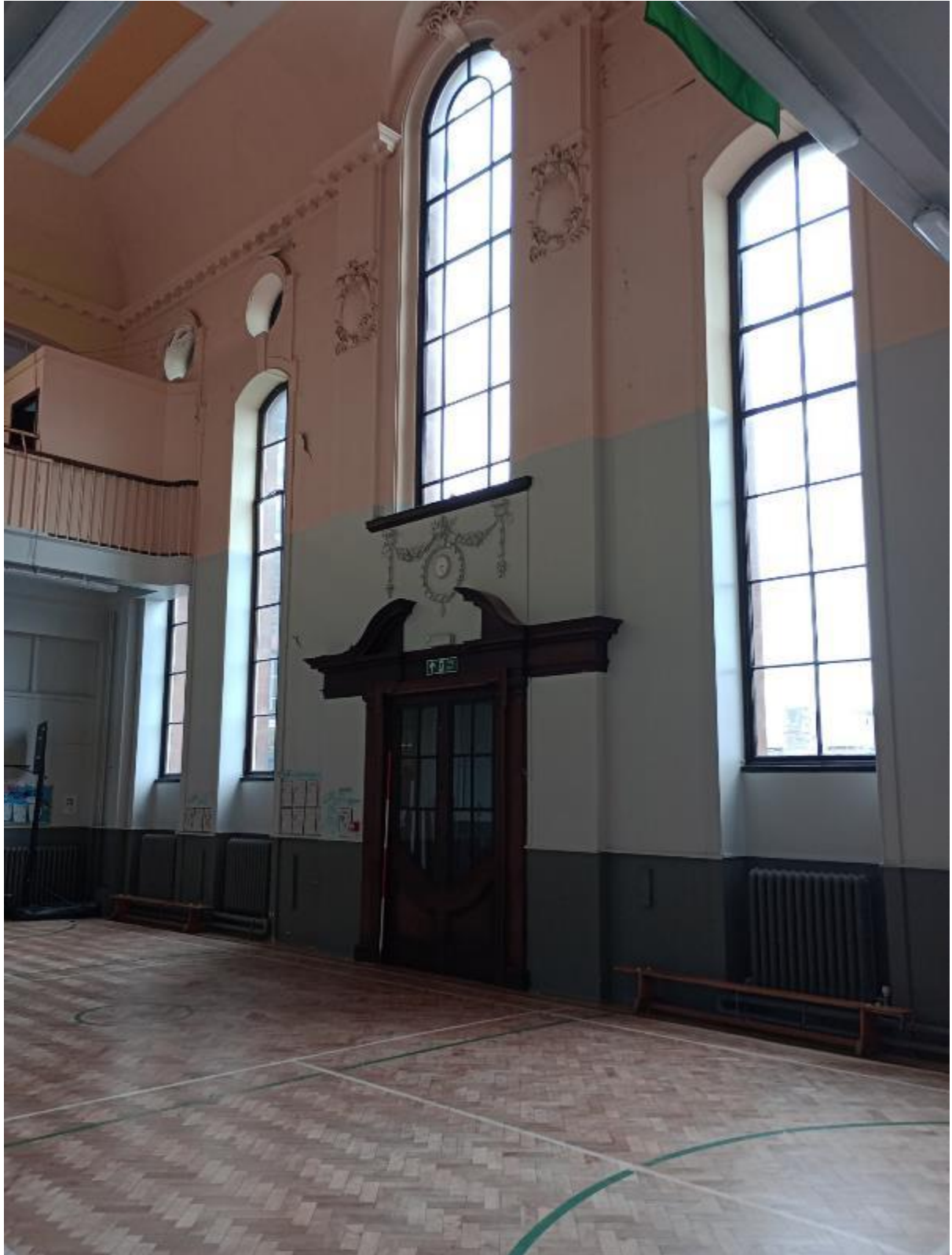
Illustration 39- Internal South facing elevation of Hall (7) showing main door, decorative plasterwork, arched and circular windows.
