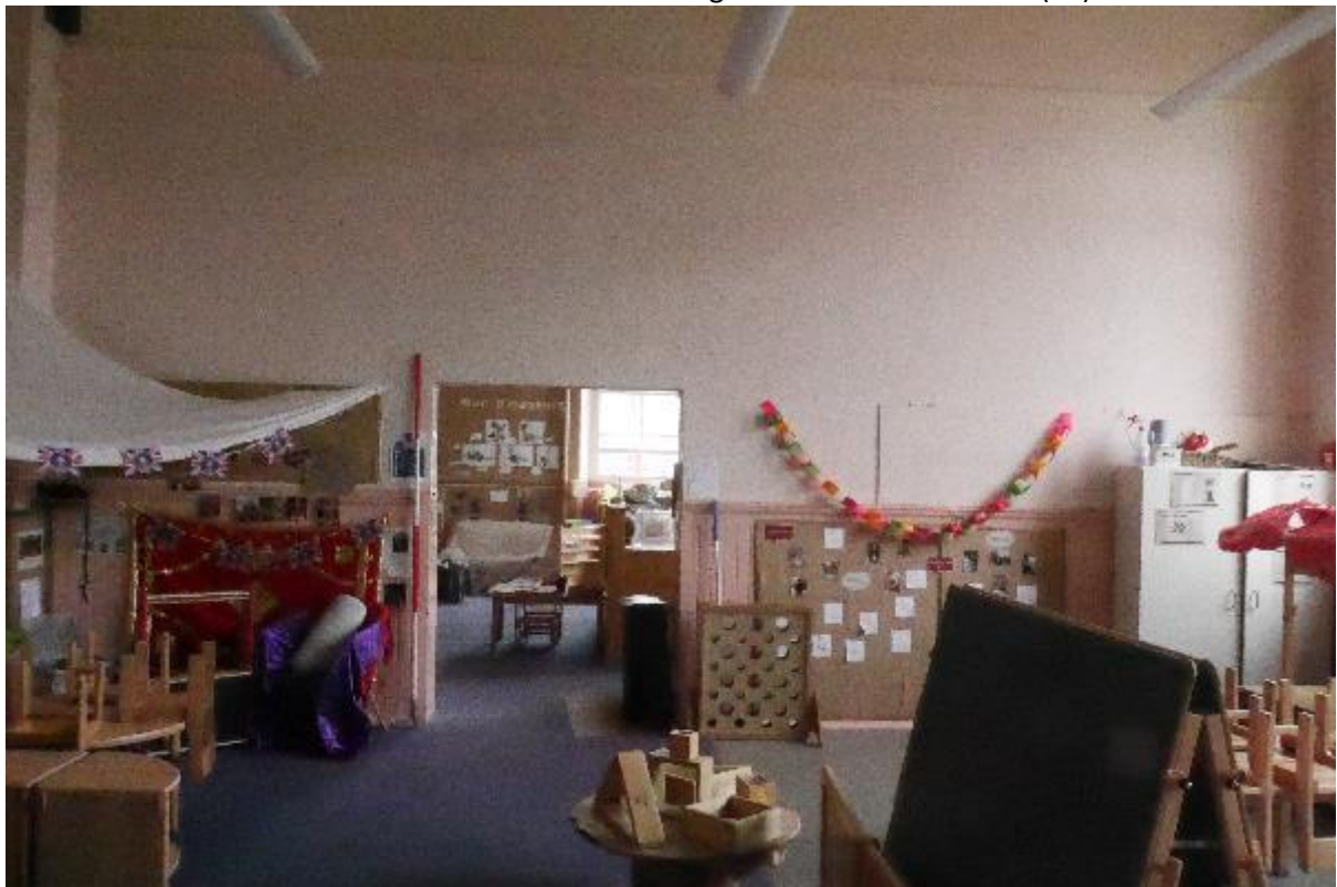
Illustration 63- Internal South facing elevation of Classroom (14) showing doorway into Classroom (15).
