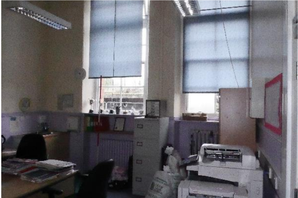
Illustration 24- Glazed windows in internal North facing elevation of Office (3).
