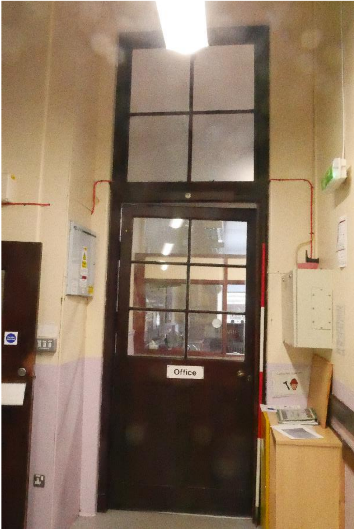
Illustration 23- Entrance door into Office (3)
