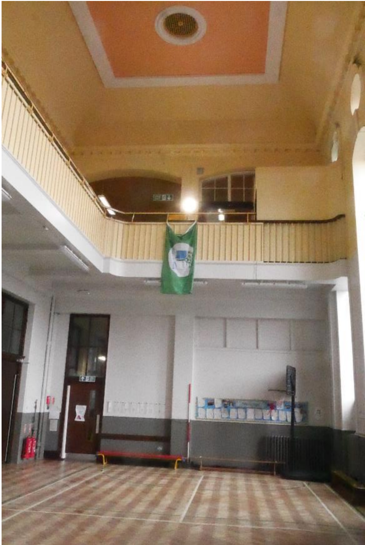
Illustration 40 - Internal West facing elevation of Hall (7) showing balustrade at upper floor level and vaulted ceiling.
