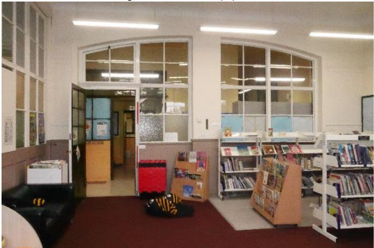
Illustration 95- Internal South facing elevation of Classroom (22) showing low arched glazed windows around doorway.
