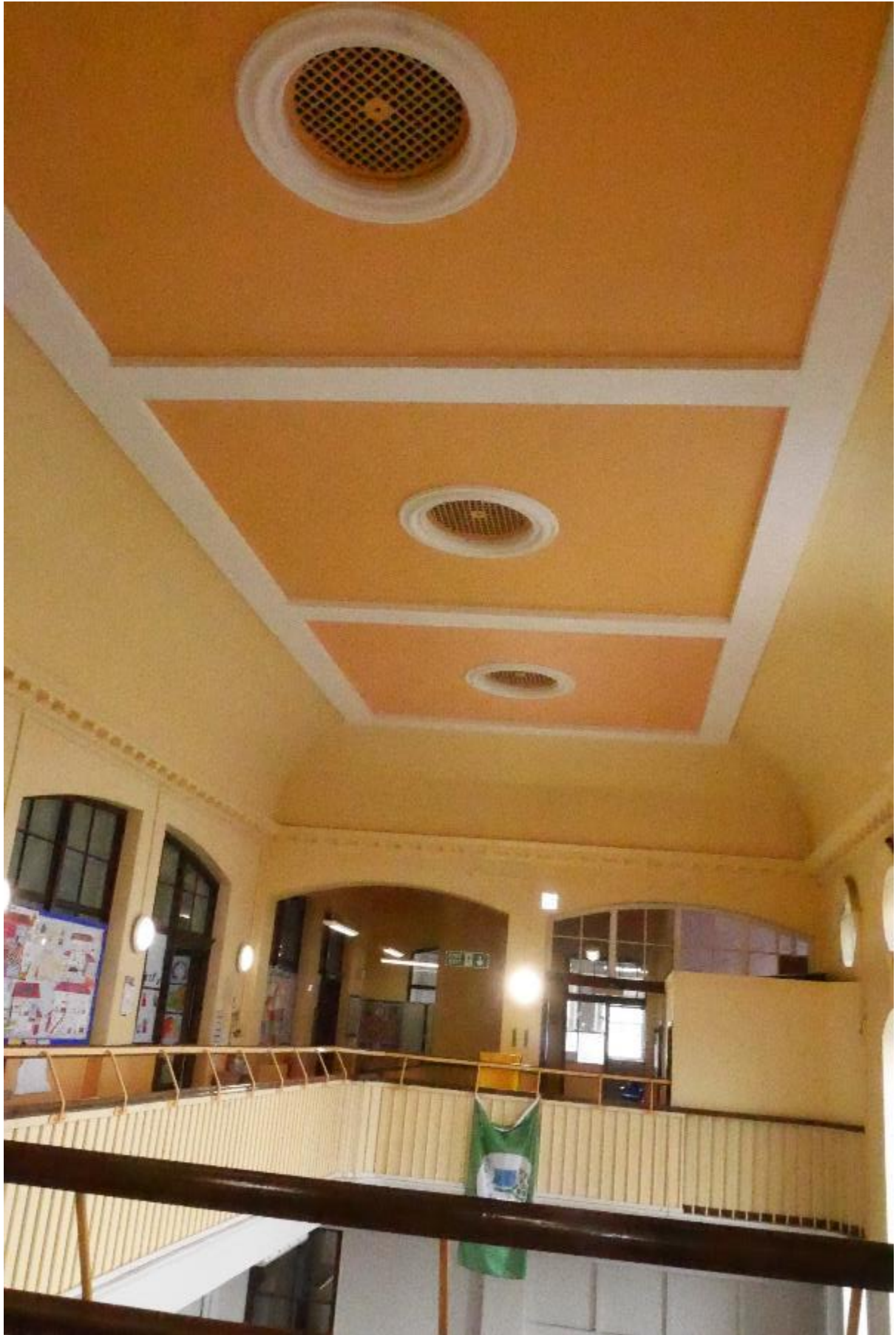
Illustration 101- General view of balustrade for balcony (24) on upper floor above Hall (7).
