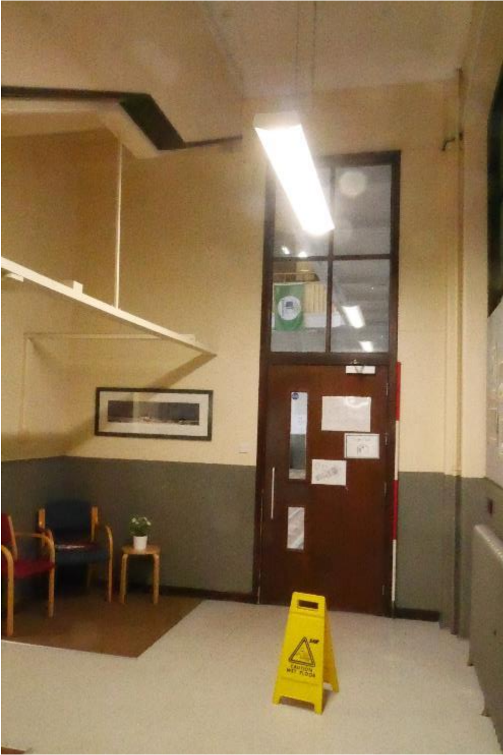
Illustration 32- Doorway from Lobby (5) into Hall (7).
