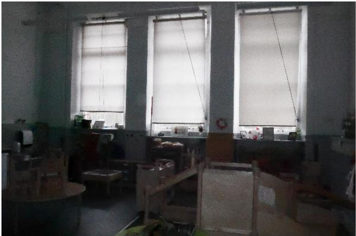
Illustration 53- Glazed windows in internal North facing elevation of Classroom (12).
