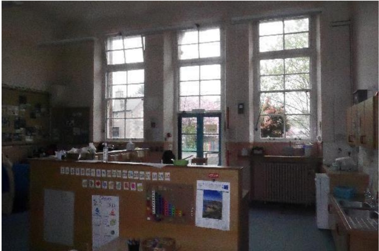
Illustration 66 - Glazed windows in internal West facing elevation of Classroom (15).
