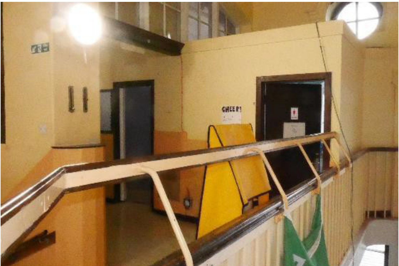
Plate 88: General view showing entrance ways to Rooms 1/20 & 1/21 located to the rear of the south mezzanine stairs, looking WSW (© Derek Hall 2023)
