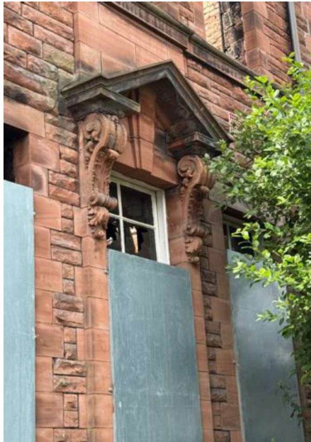
Plate 15: Detailed view of the triangular pediment details as repeated on south-west and north-east elevation (© Graham & Sibbald 2025)
