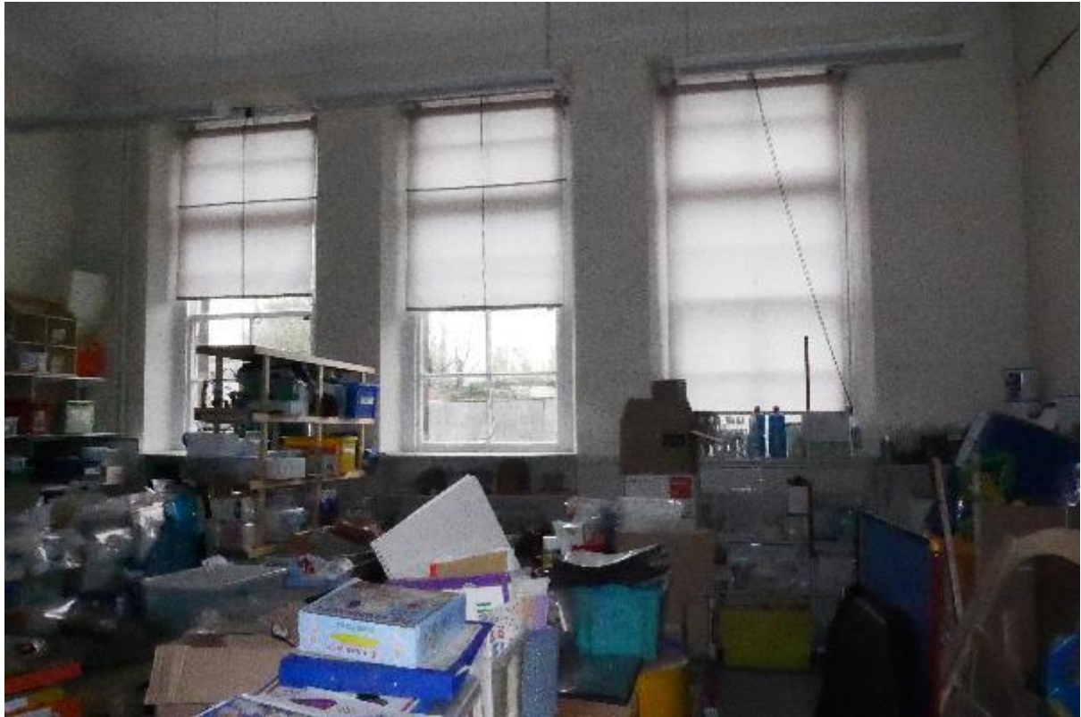
Illustration 58- Glazed windows in internal West facing elevation of Classroom (13).
