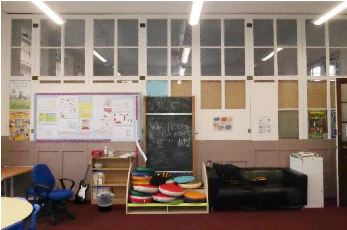
Illustration 92 - Internal West facing elevation of Classroom (22) showing original folding dividing wall.
