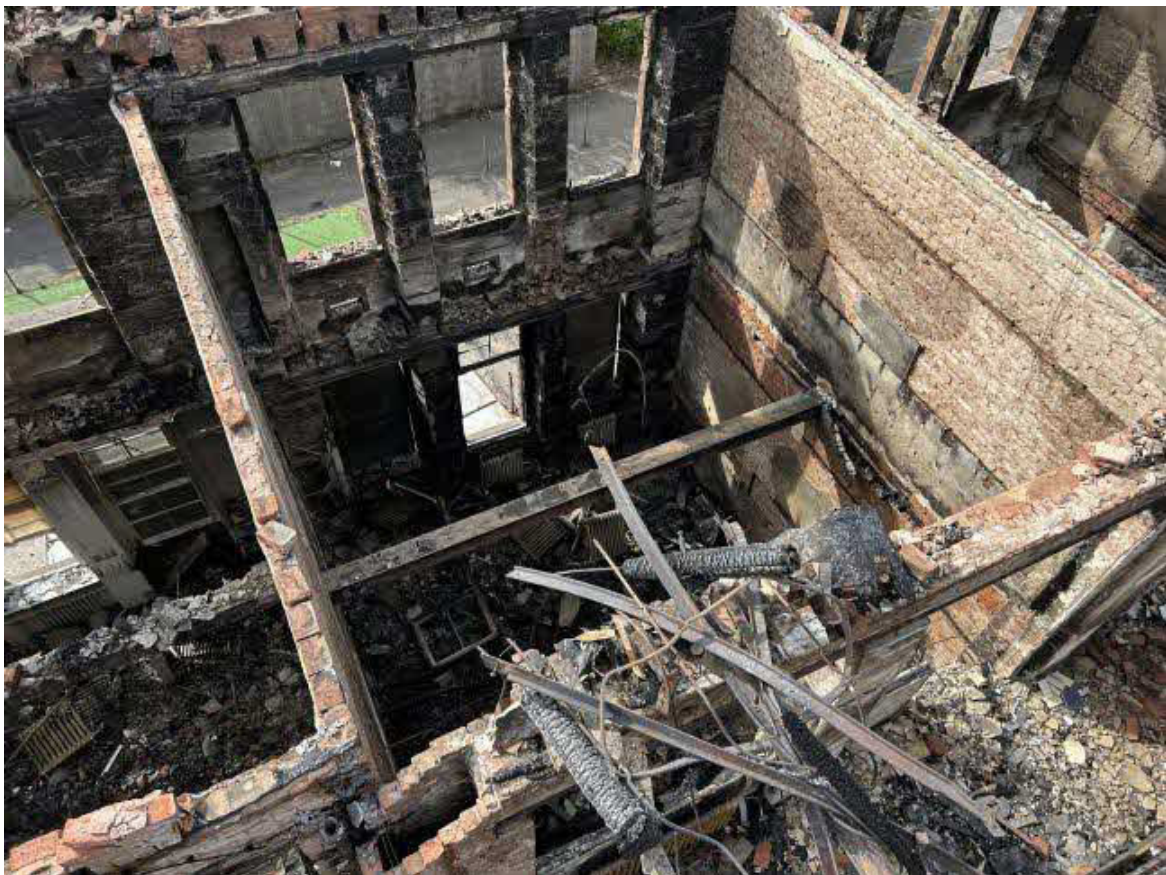
Plate 28: Overview of fire-damaged interior showing construction materials in Rooms 0/16 & 1/9, looking ESE (© G3 Consulting Engineers 2025)
