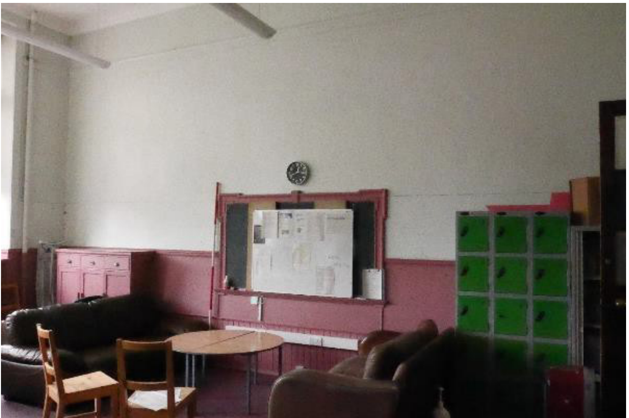
Plate 52: General view of the south-west wall showing the original blackboard, looking south (© Derek Hall 2023)
