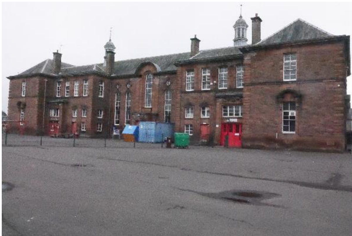
North facing external elevation of Balhousie Primary School looking South East.
