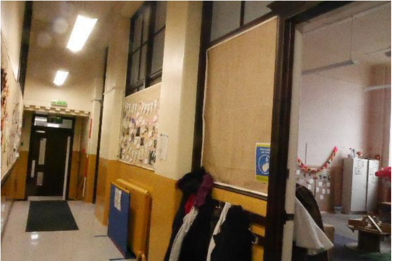
Plate 69: General view of Room 0/22, looking north-west (© Derek Hall 2023)
