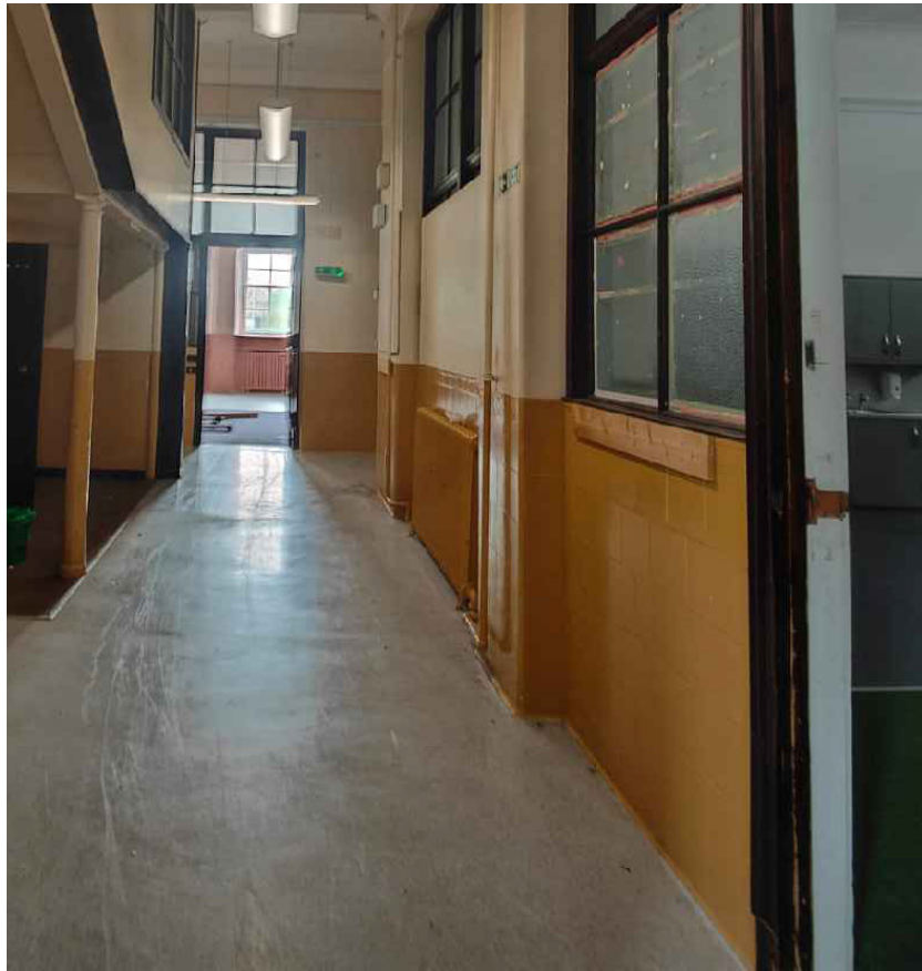
Plate 61: General view of Room 0/15, looking north-east (© Trail Architects 2024)
