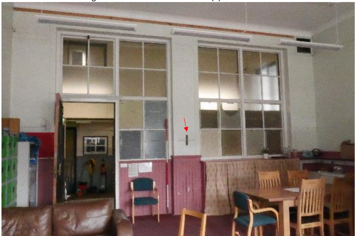
Illustration 36- South facing internal elevation of Staff Room (6) showing entrance door, glazed windows and fitted cupboards. Red arrow indicates location of original control for ventilation system (see next Illustration).
