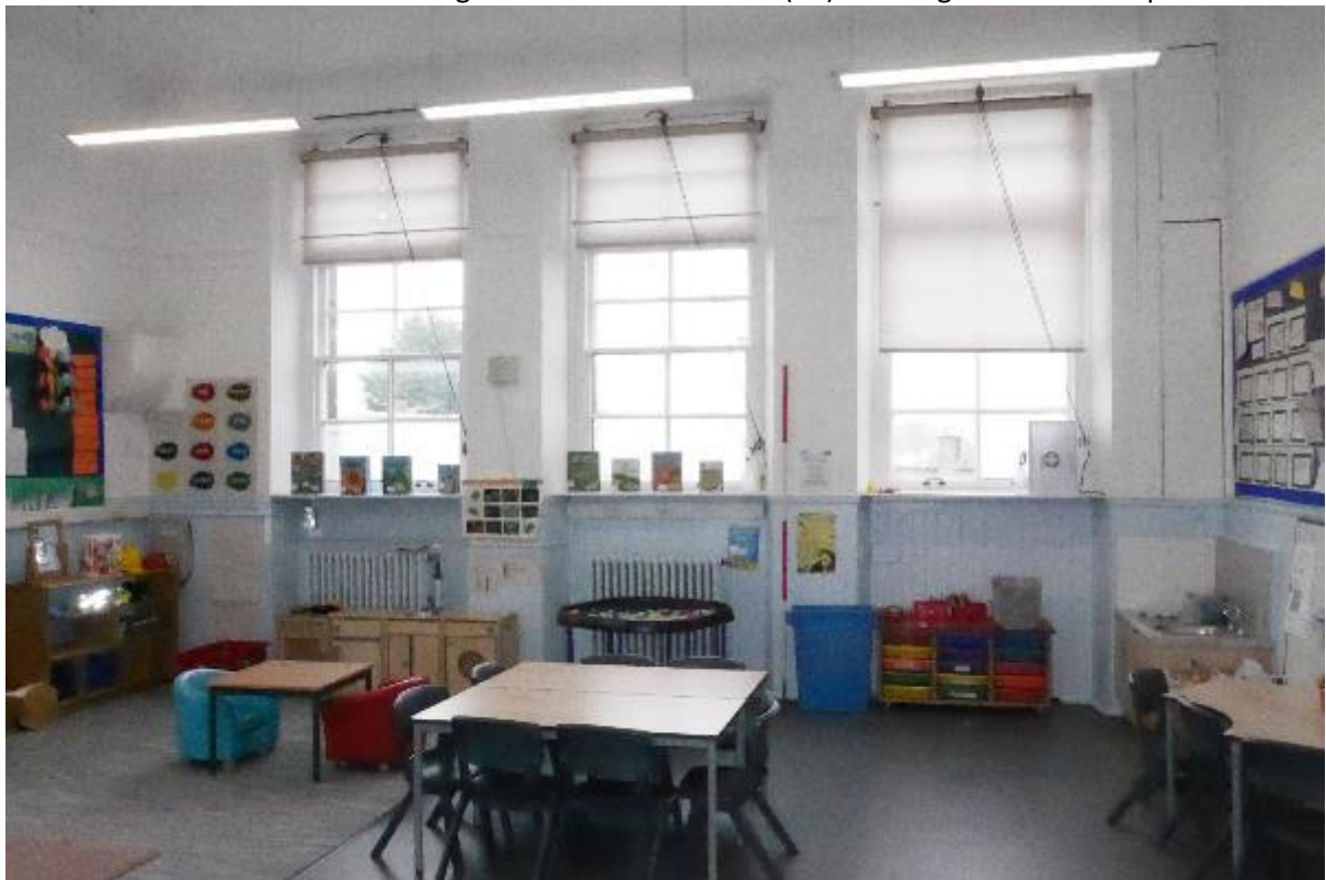
Illustration 111- Internal North facing elevation of Classroom (27) showing glazed windows and half-timbered planked wall.
