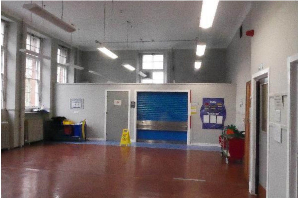
Illustration 18- Interior of Dining Room (2) looking North towards serving area.
