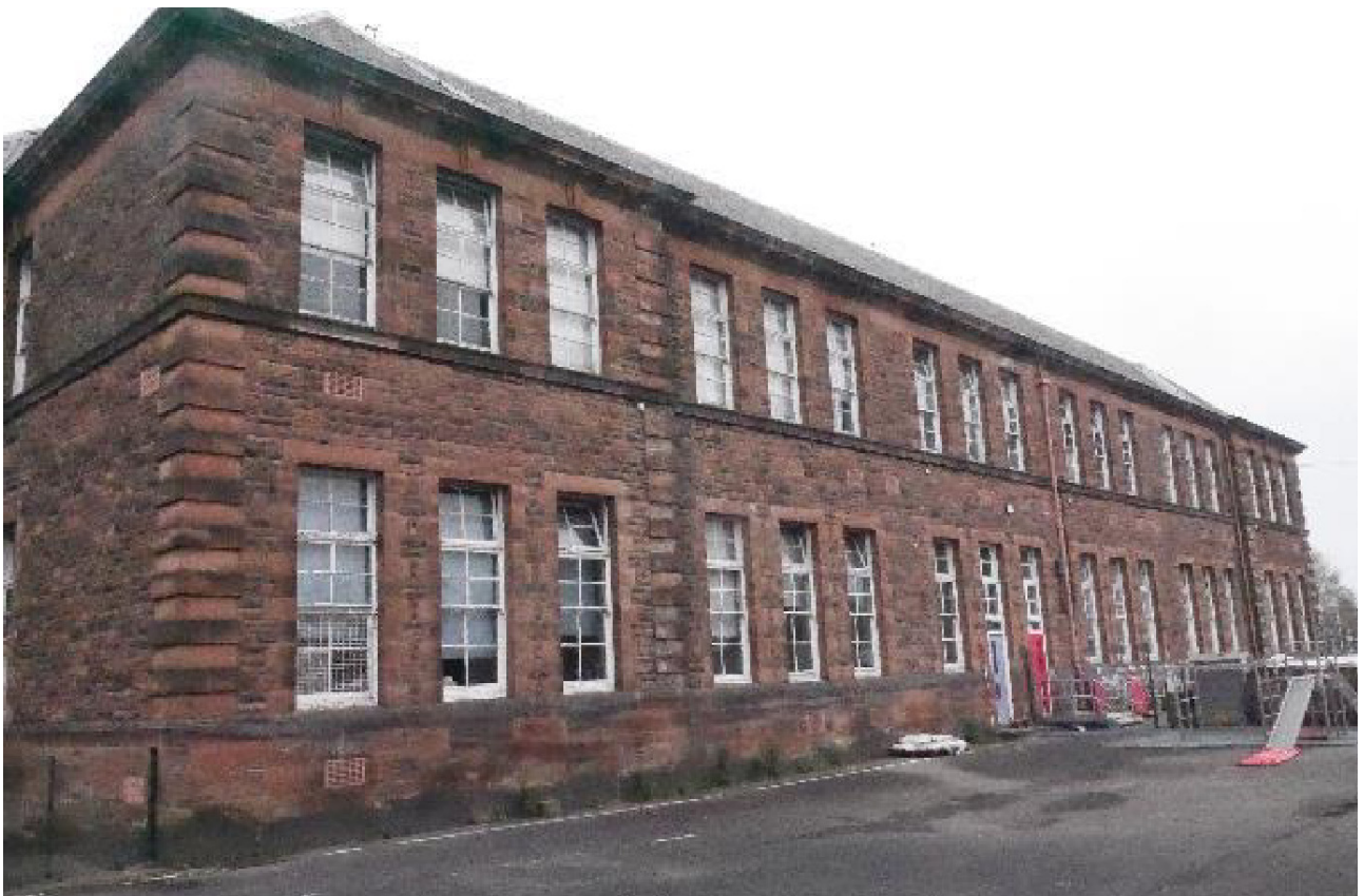
Plate 16: General view of south-east facing elevation, looking north (© Derek Hall 2023)
