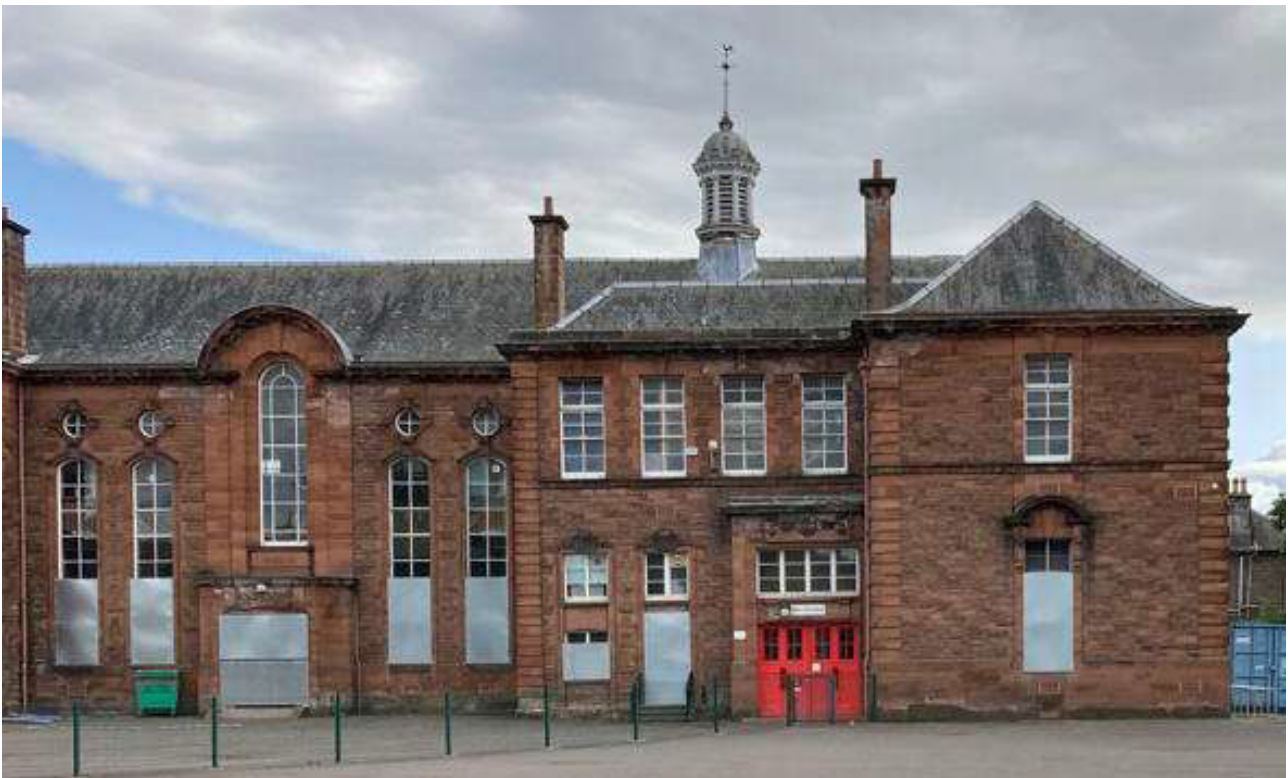
Plate 6: General view of the north-west facing elevation - west extent, looking south-east (© Perth and Kinross Council 2023)
