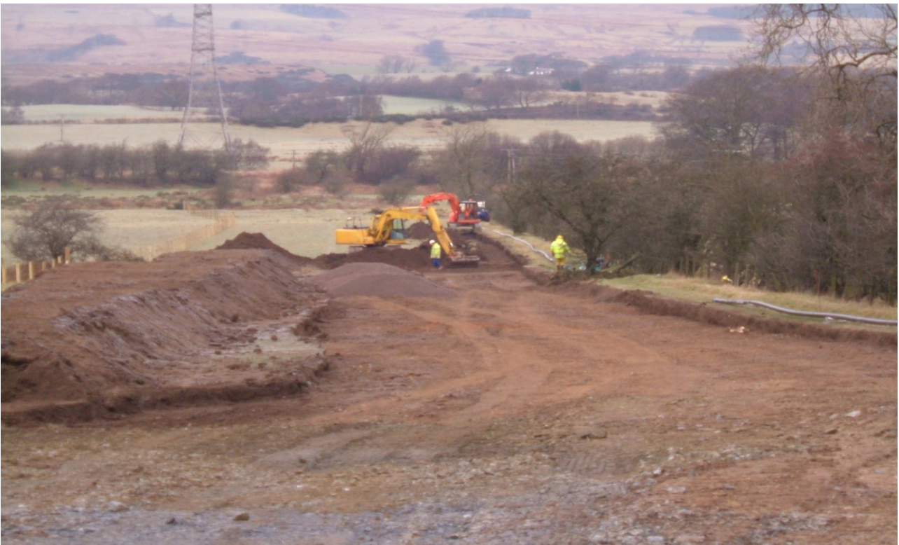
Plate 2 Way-leave top-soil stripping from south
