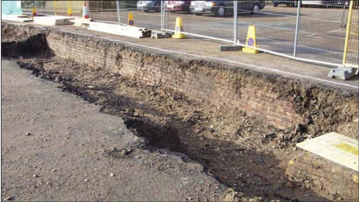
Plate 1: Historic wall, looking West
