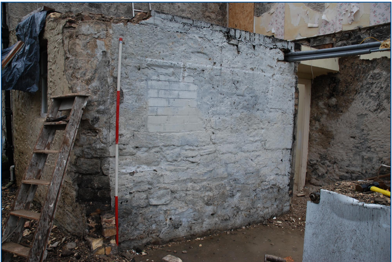
Plate 12: Detail of east wall on Room 0.3 during demolition of Manor House extension from west
