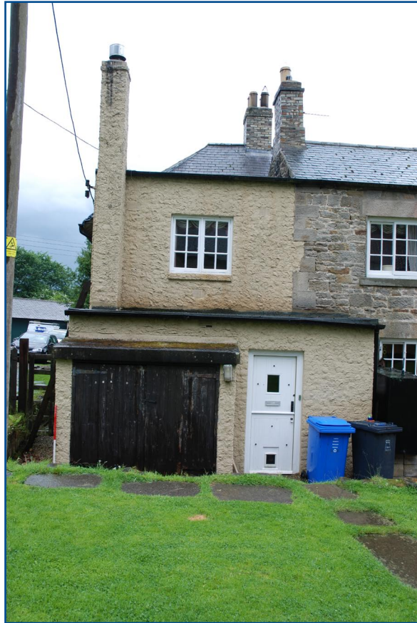
Plate 7: General view of north end of west elevation (later extension, now demolished) of Manor House from west
