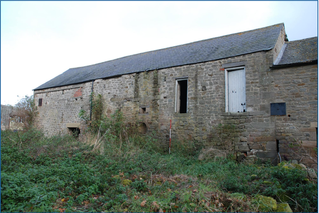
Plate 19: General view of west elevation of barn from south-west
