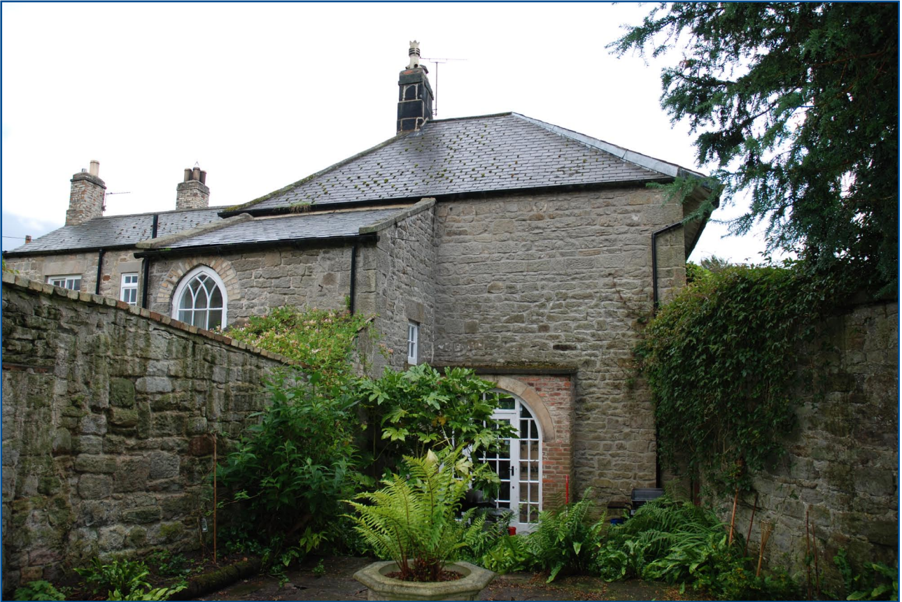
Plate 5: General view of south end of west elevation of Manor House from south-west
