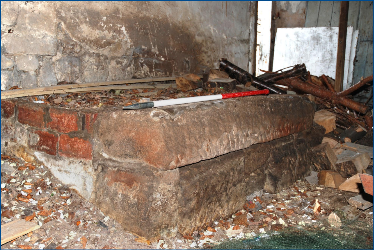
Plate 23: Detail of dressed stones to centre of east wall from north-west
