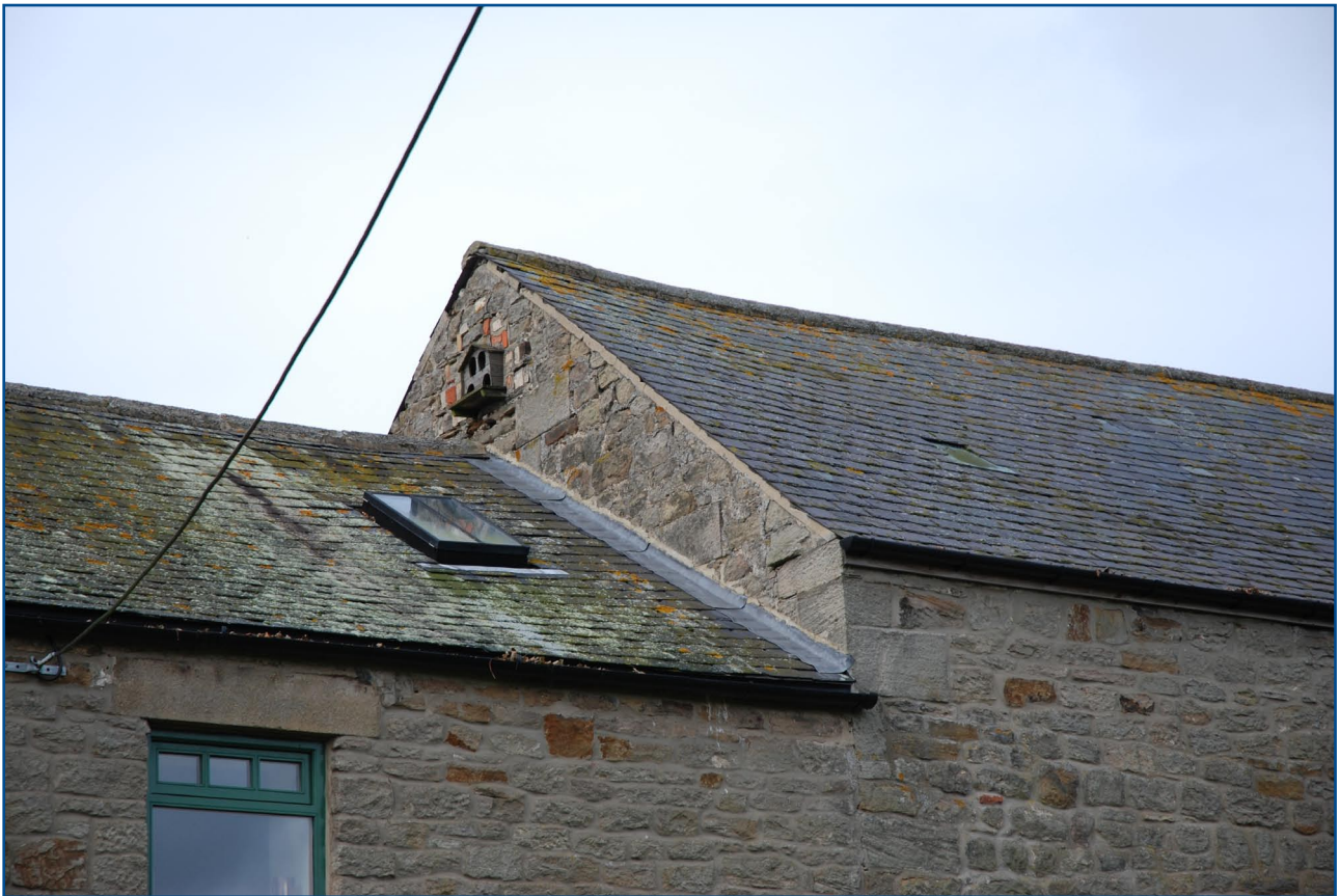
Plate 18: General view of south elevation of barn from south-east
