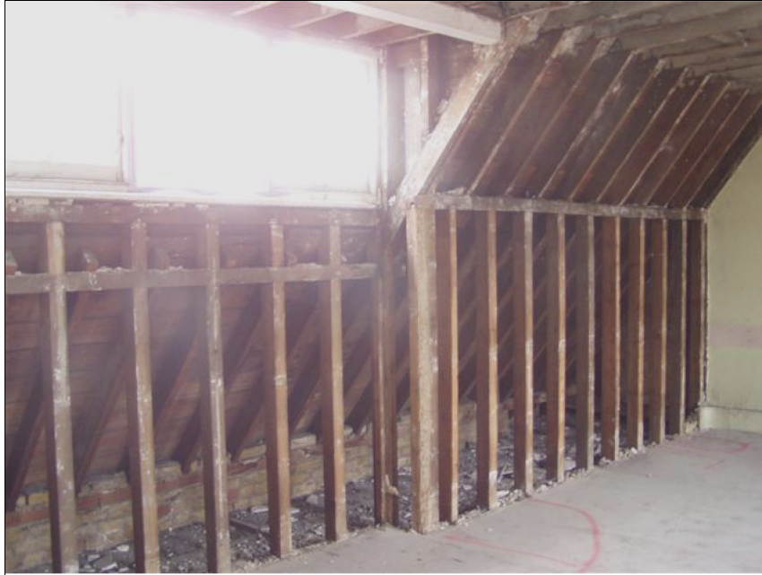
Plate 12: Second floor Room S3 looking northeast
