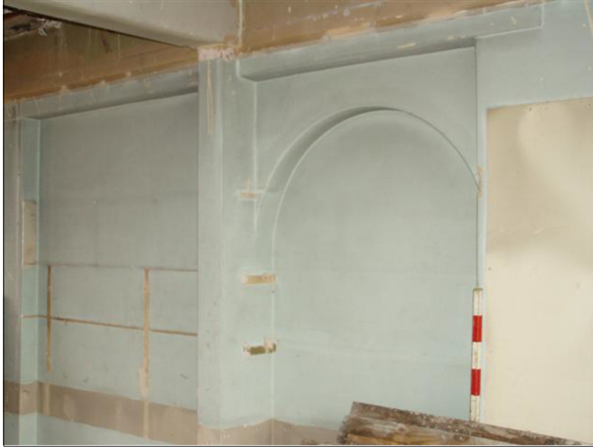
Plate 9: Room F1 arch between chimneybreasts, First Floor Room looking southwest
