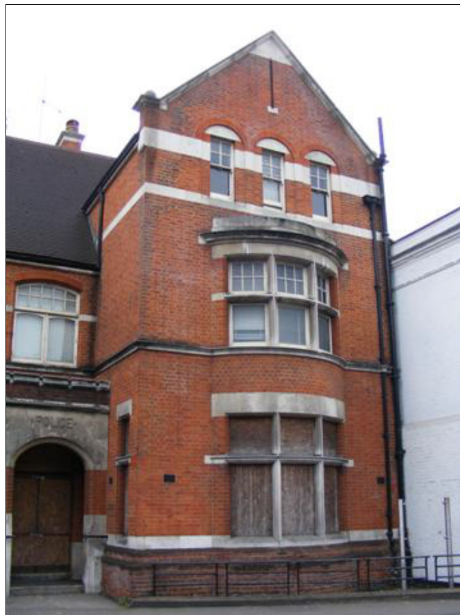
Plate 2: External view of western section and porch entrance looking south
