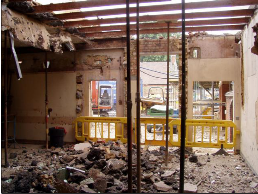
Plate 6: Ground floor Room G1 looking south
