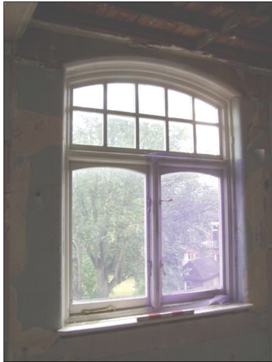
Plate 11: Front window, Room F3
