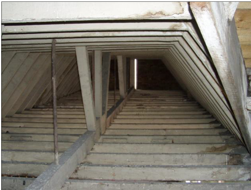
Plate 13: Roof assembly above room S3 looking east
