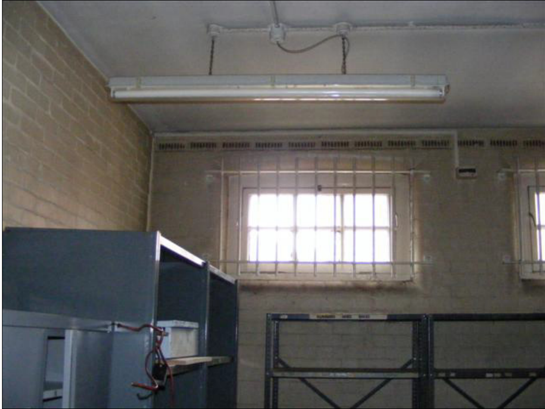
Plate 17: Room A1, including window grill
