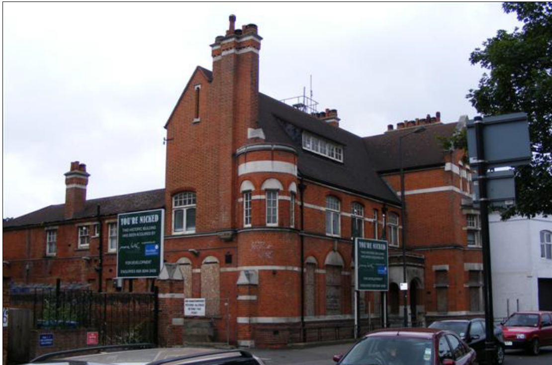
Plate 1: External view of Police Station looking southwest
