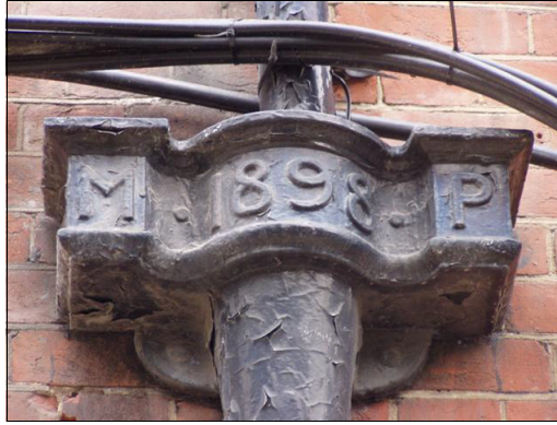
Plate 3: Detail of hopper, east side.
