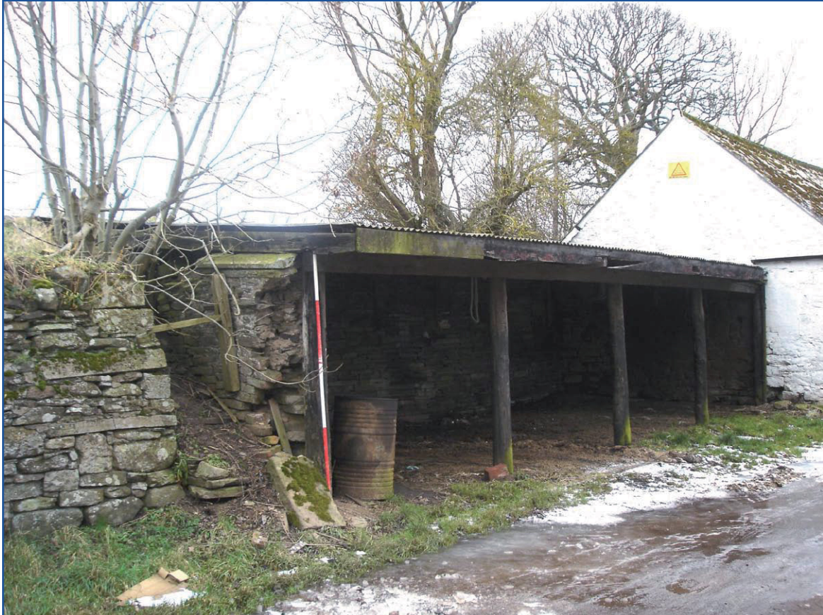
Plate 18: Building E, general view from the east
