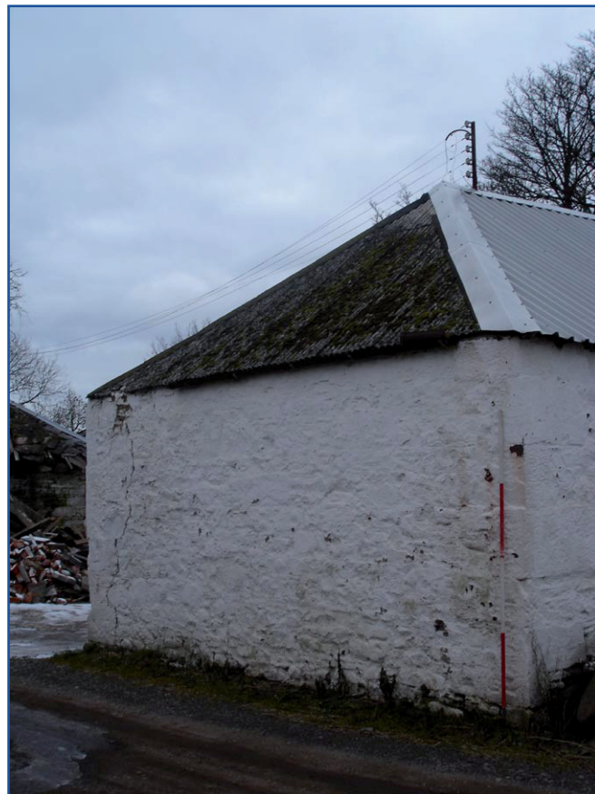
Plate 2: Building A, general view of west elevation
