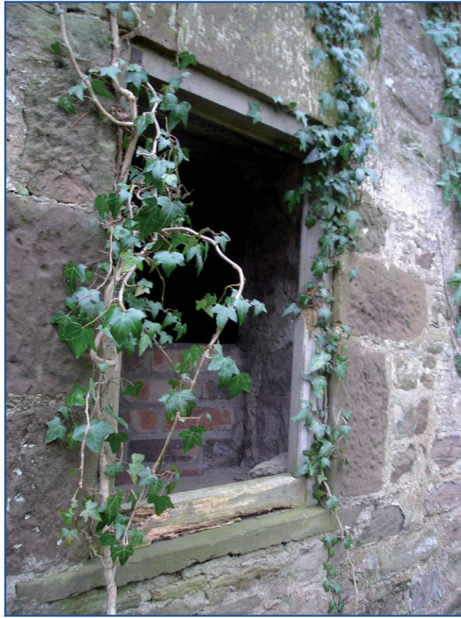
Plate 7: Building A, detail of window in east elevation
