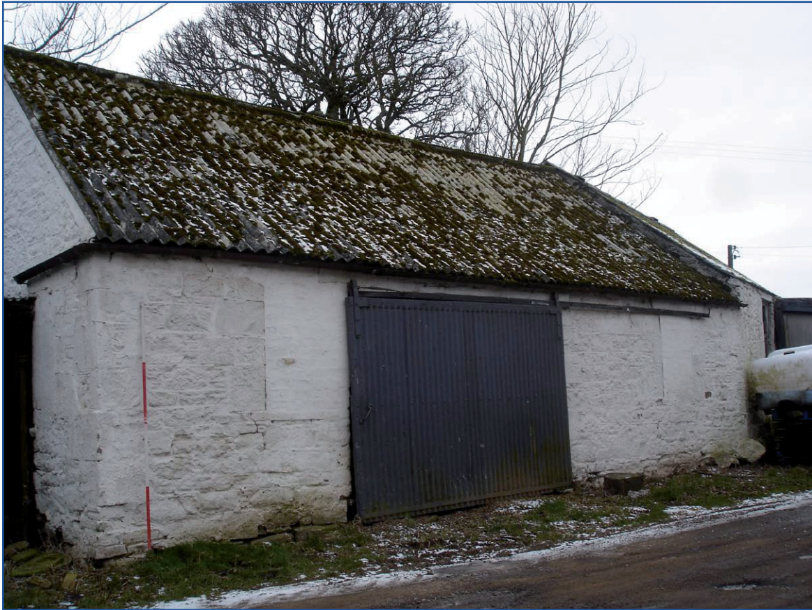
Plate 19: Building F, general view of north-east elevation
