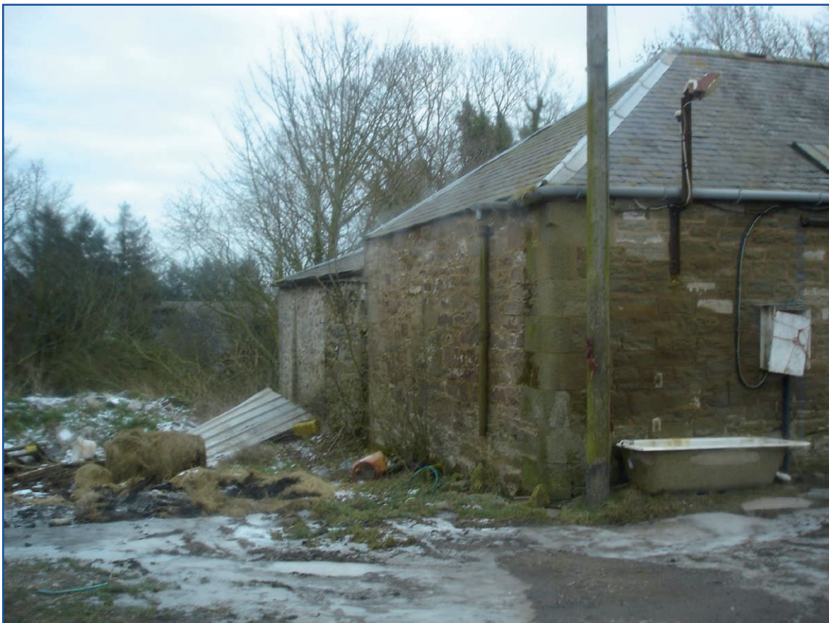
Plate 16: Building D, general view of north elevation
