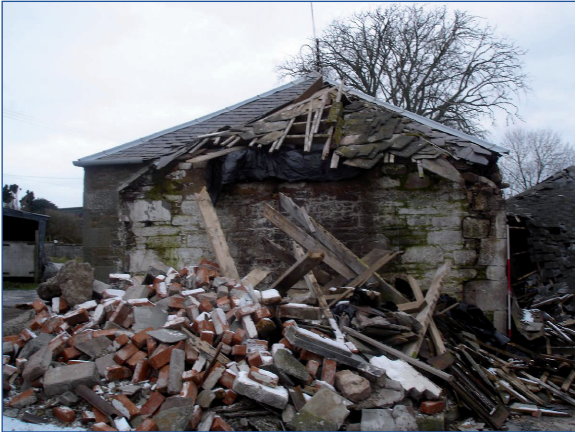
Plate 15: Building D, general view of the north elevation
