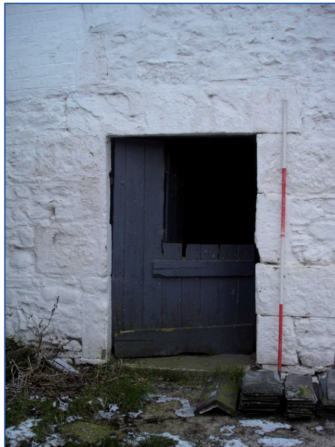
Plate 4: Building A, detail of door in north elevation
