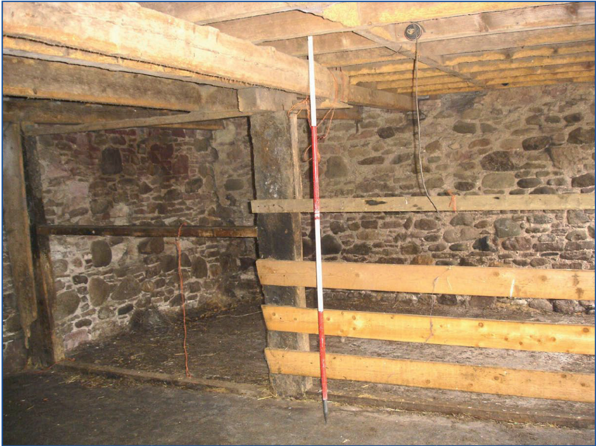
Plate 11: Building B, general view of interior from north-west
