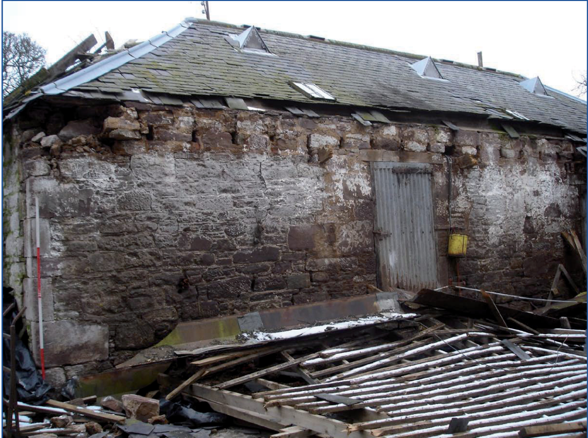
Plate 14: Building D, general view of east elevation
