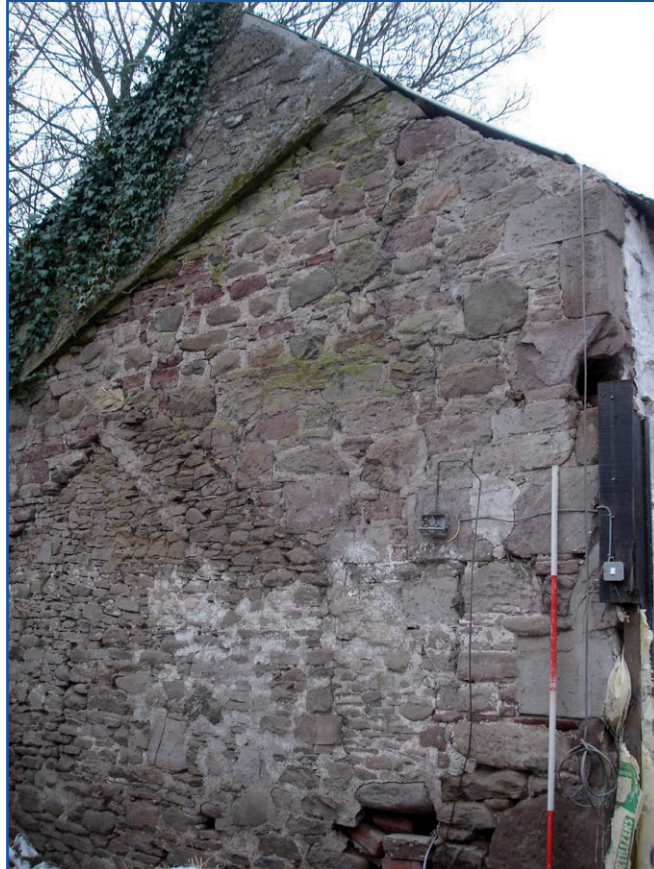
Plate 10: Building B, general view of north gable
