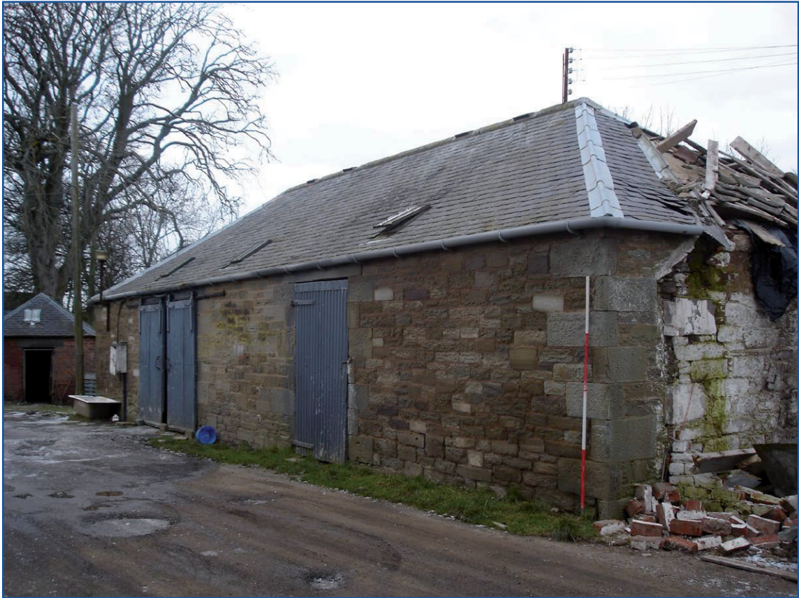
Plate 13: Building D, general view of west elevation
