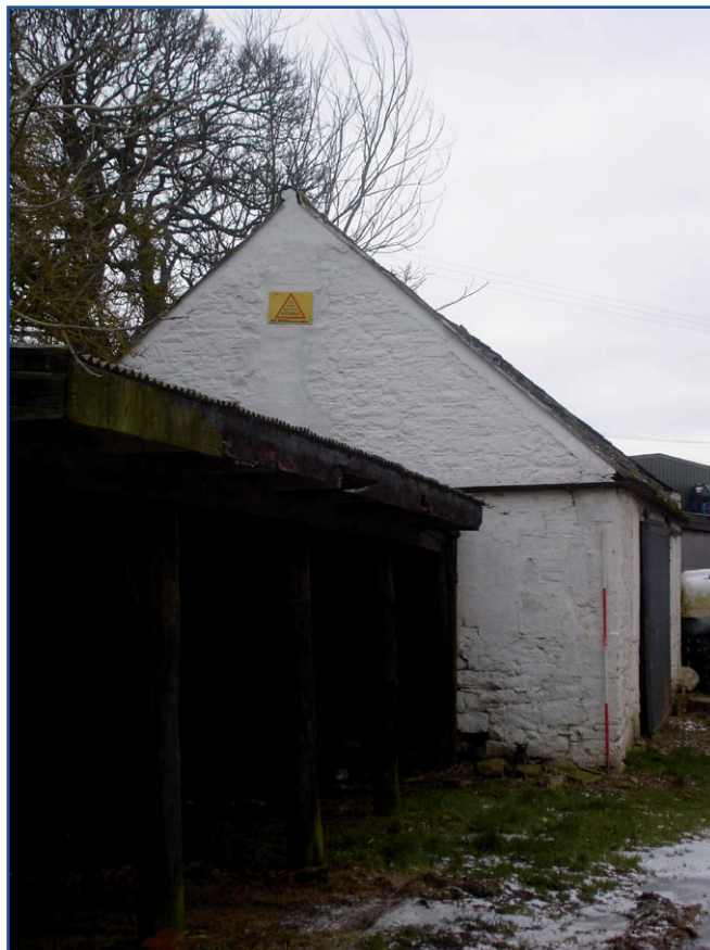
Plate 20: Building F, general view of south-east gable
