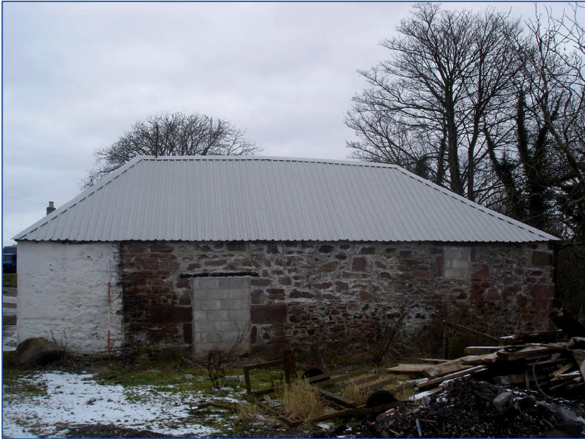
Plate 1: Building A, general view of south elevation
