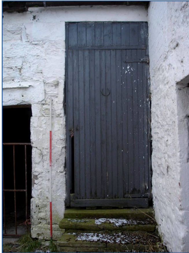
Plate 5: Building A, detail of west-facing door to first floor
