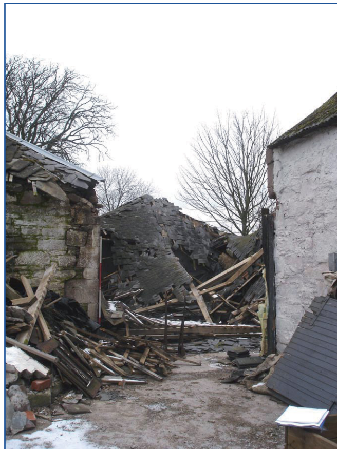
Plate 12: Building C, general view of collapsed building from the south-west
