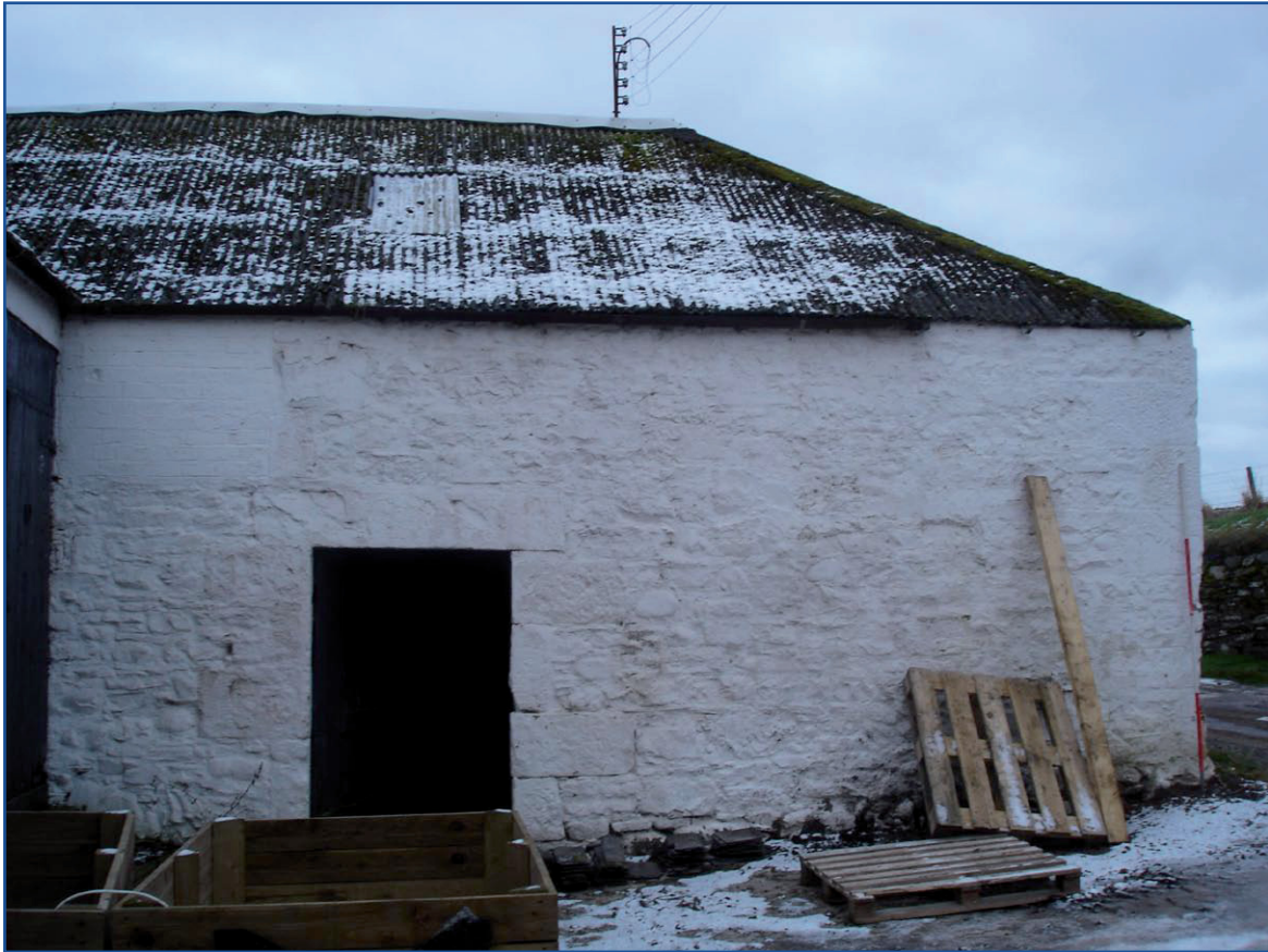
Plate 3: Building A, general view of north elevation
