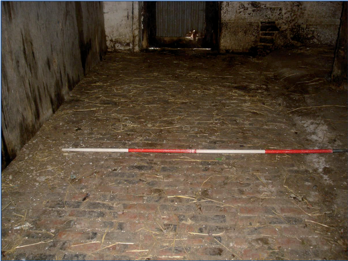
Plate 17: Building D, detail of brick paving to the interior from the west
