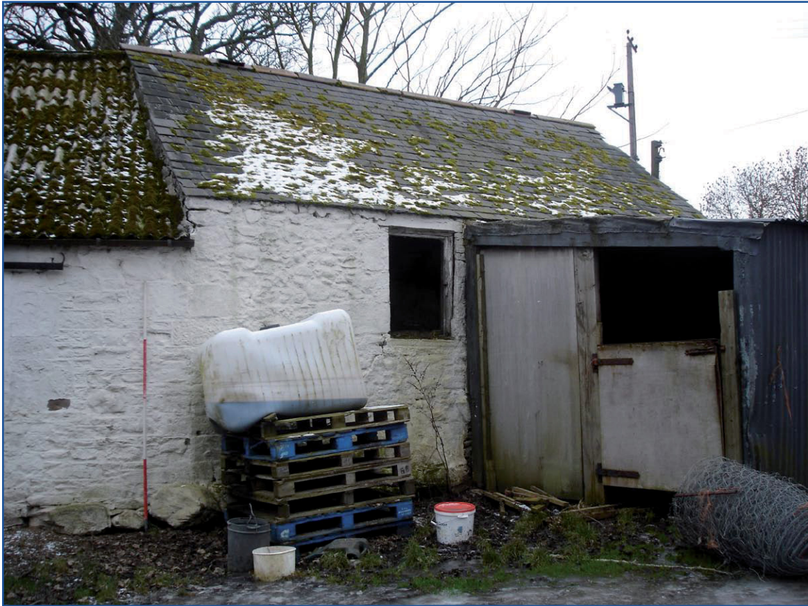
Plate 21: Building G, general view from the east
