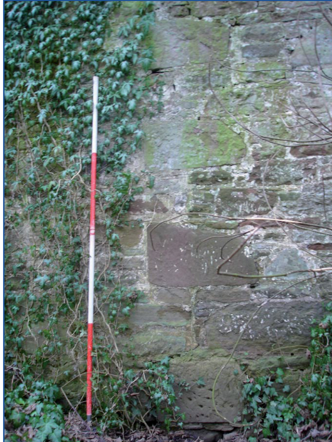
Plate 6: Buildings A & B, detail of phase line in east elevation
