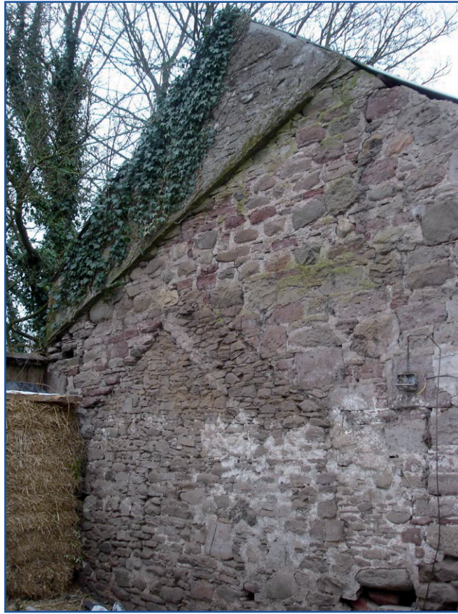
Plate 9: Building B, general view of north gable
