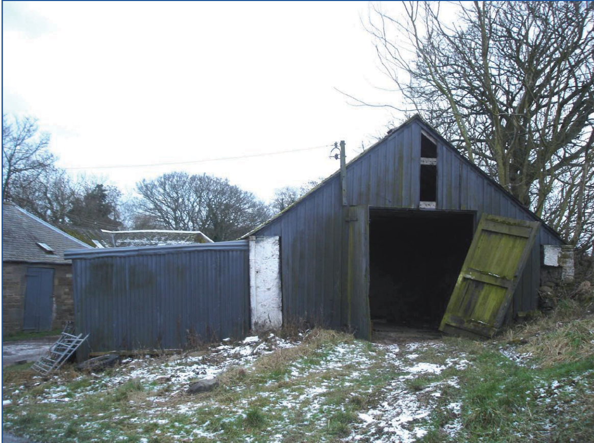
Plate 22: Building G, general view from the north
