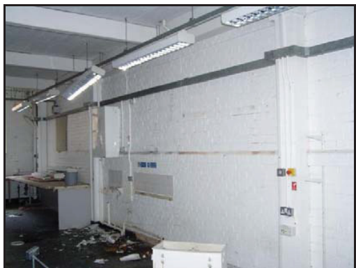
Plate E. View of Ground Floor Room
