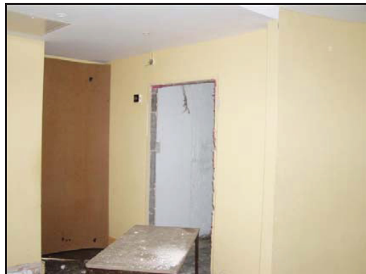
Plate D. View of Foyer
