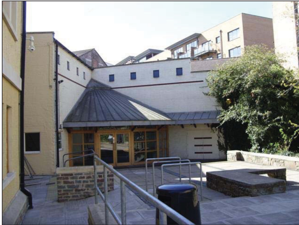
Plate 4: View of east elevation.
