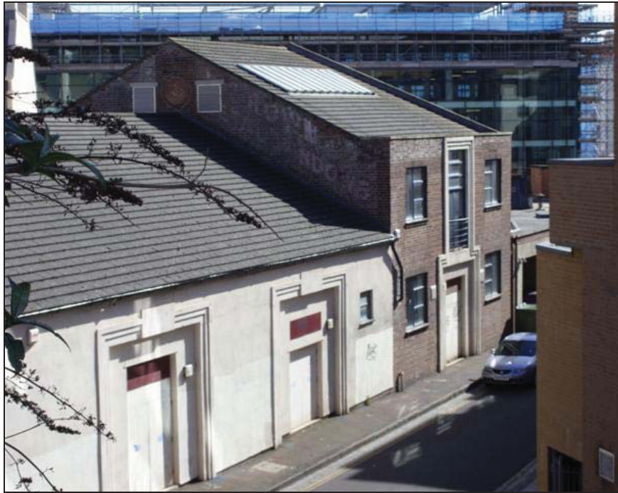
Plate 1: West elevation of Lower Lamb Street entrance
