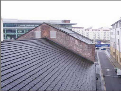
Plate A. View of Roof
