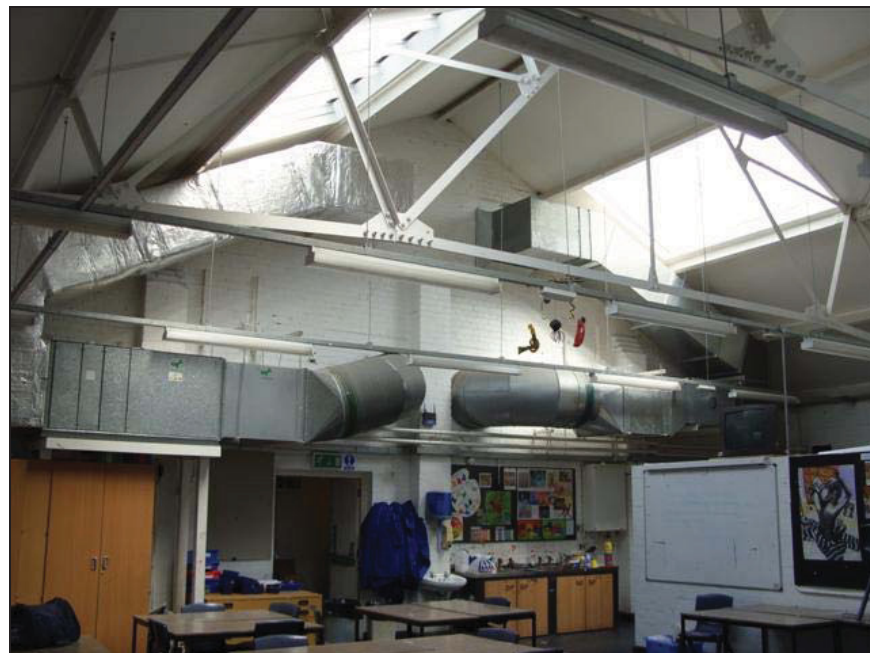
Plate 6: First Floor Room F1 looking north
