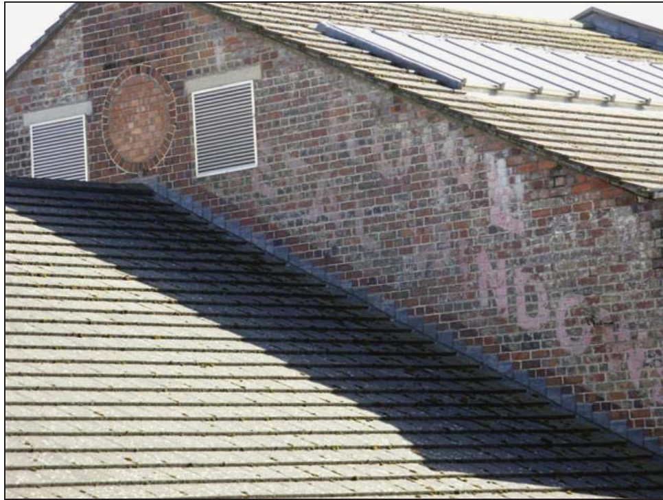
Plate 3: Rowe's Metal Windows and office roofline
