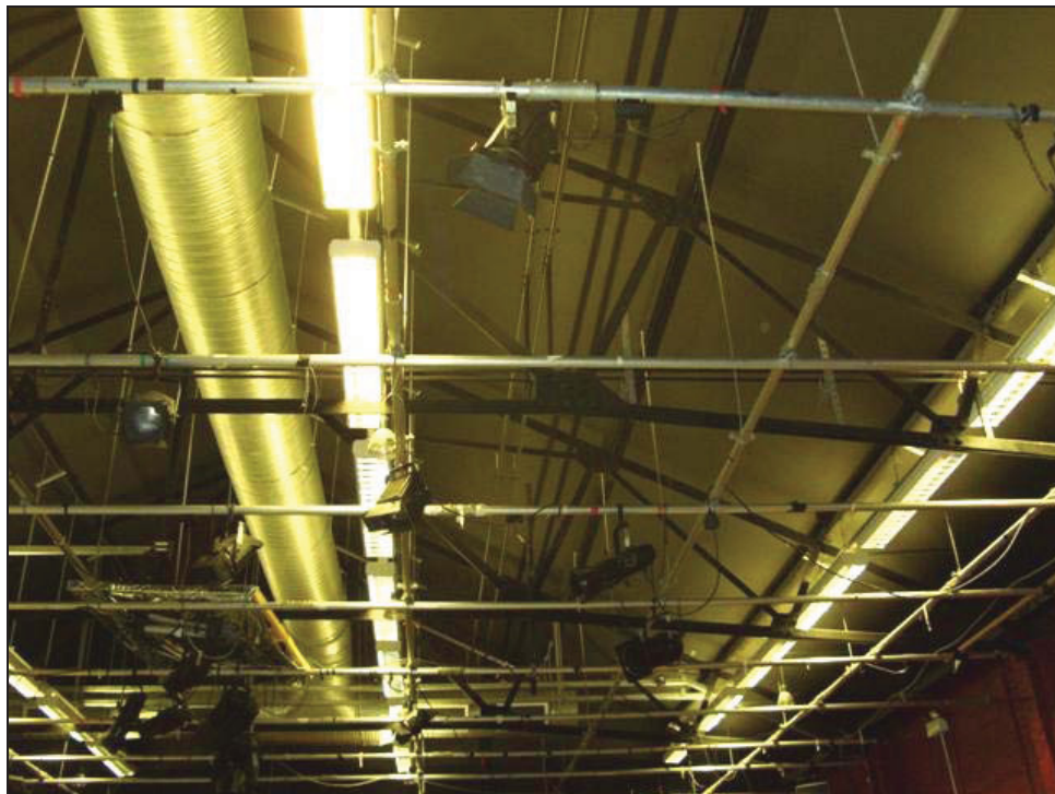
Plate 8: Theatre roof trusses
