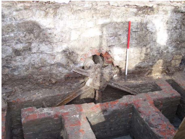
Plate 3: Stone wall [306] with internal walls [305] and the remains of the internal wheel.
