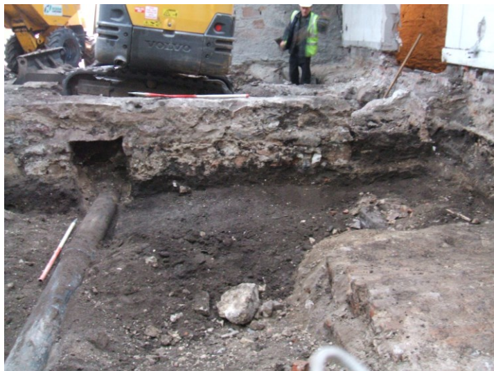
View of wall (143) prior to removal: from north-east
