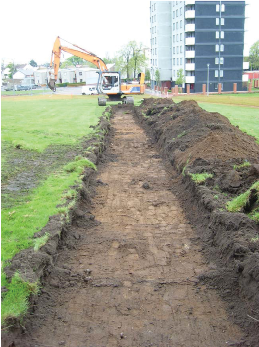
Plate 2: Trench 4 looking north-east
