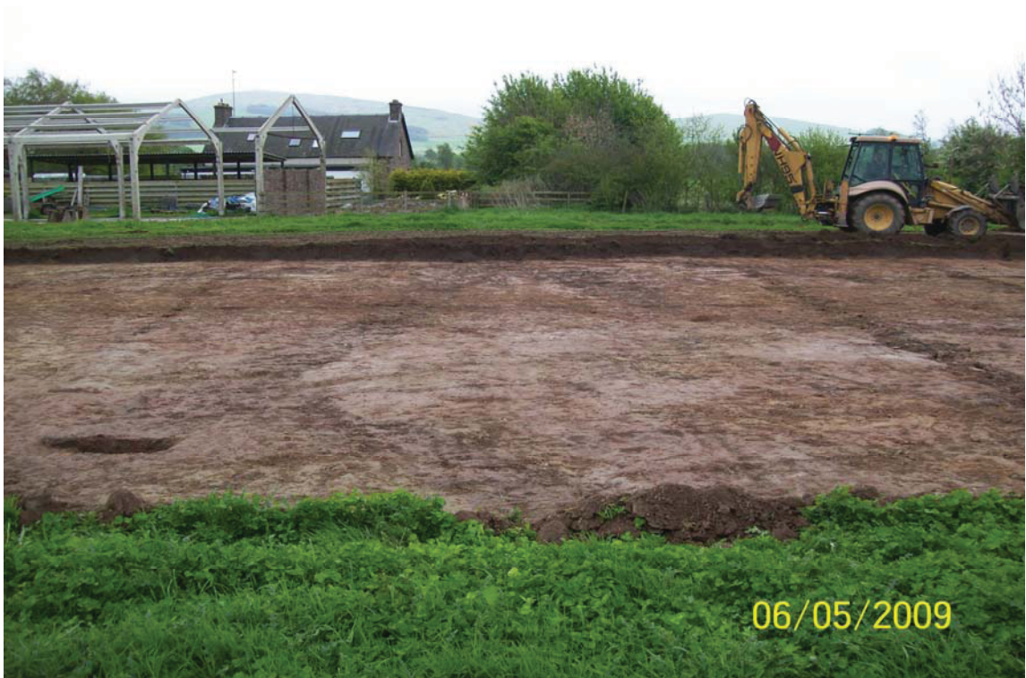
Plate 2 Area Shot Showing Field Drains
