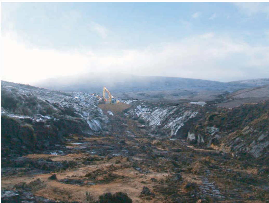
Plate 4: General view after peat stripping access road between turbines 1 and 2, from the north
