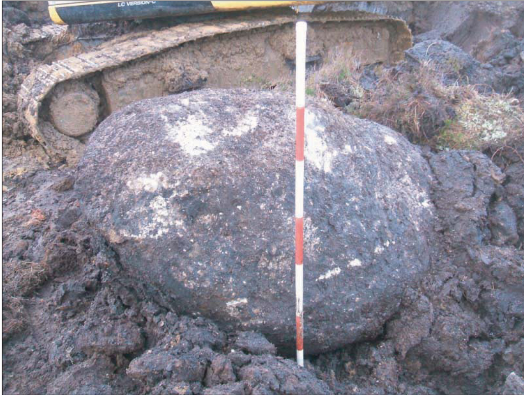
Plate 5: General view of typical glacial erratic encountered along parts of the access road to turbines 1 and 2
