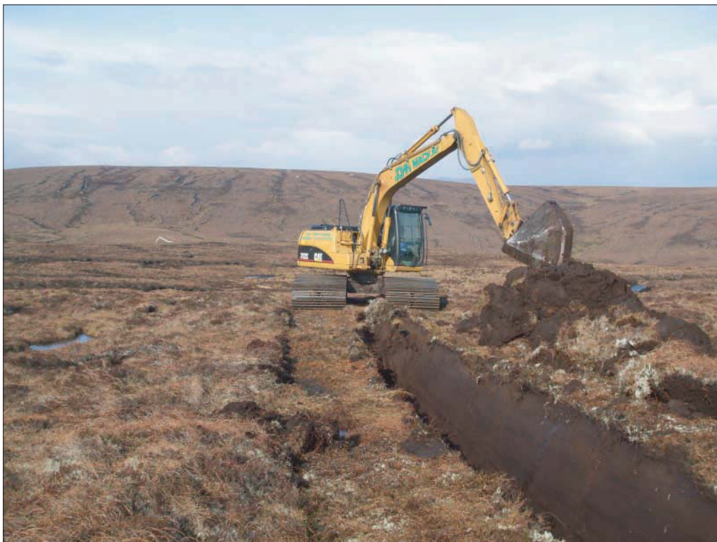
Plate 8: General view during excavation of cable trench, from the east
