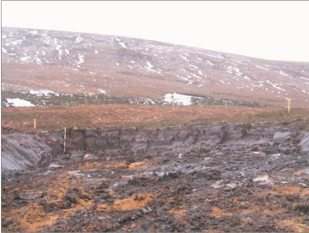
Plate 3: General view during peat stripping along the access road to turbine 1
