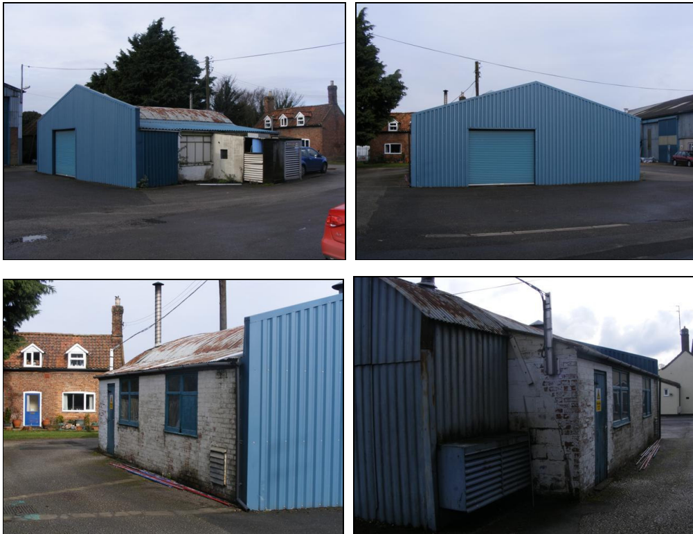
PLATE K: Views of the single storey spray paint shop in the southern section of the proposed development site
