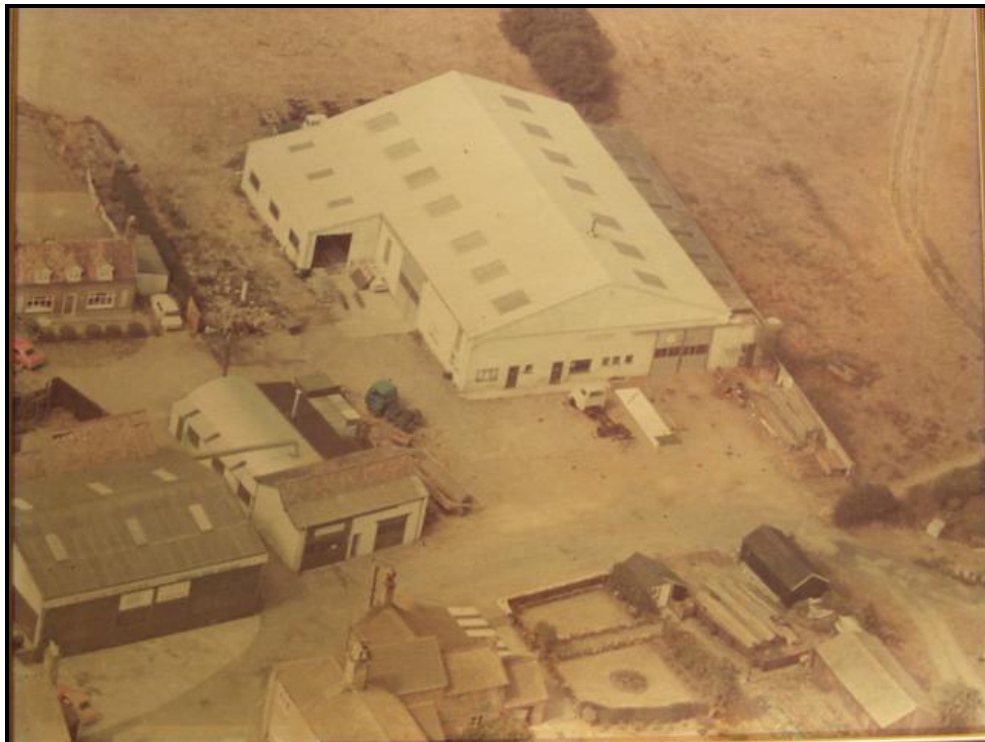
PLATE D: Aerial Photograph (c.1960s) showing proposed development site
