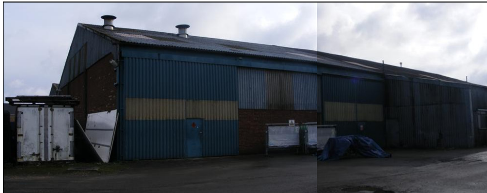
PLATE H: Main warehouse / assembly building in the east of the site, viewed from the west
