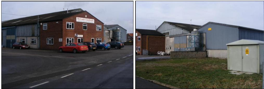
PLATE G: Main warehouse / assembly building in the east of the site, viewed from the south-west (left) and south-east (right)
