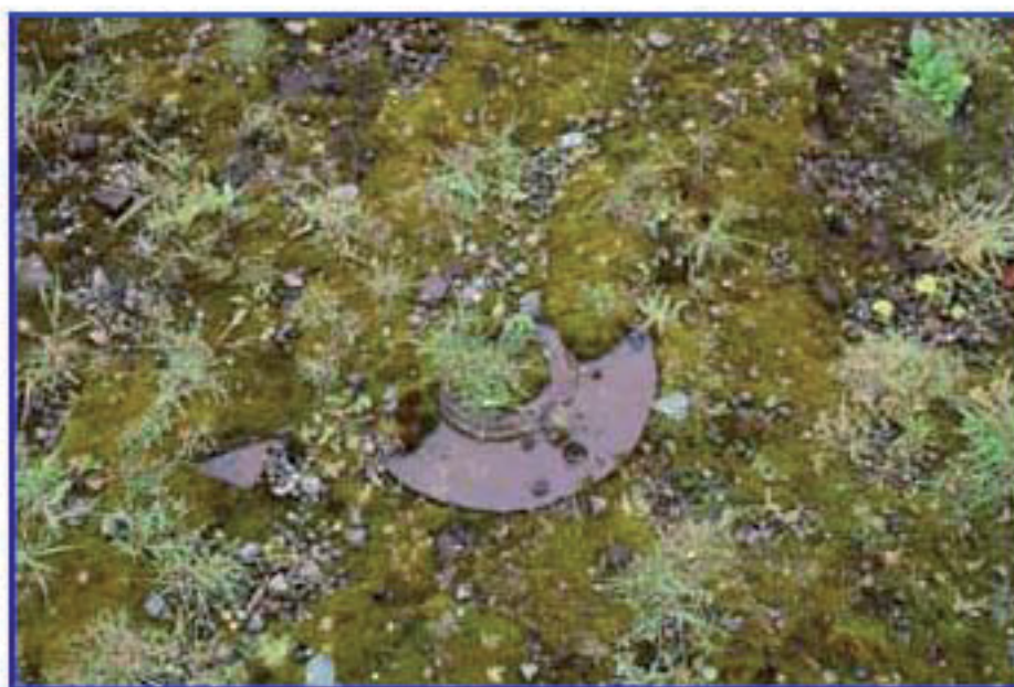
Plate 6: Detail of a circular metal fitting bolted to the concrete floor
