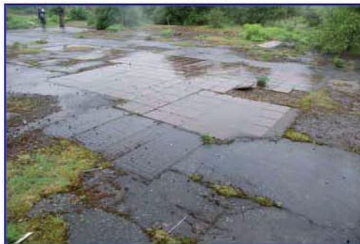
Plate 5: General view of one of the non slip floor surfaces
