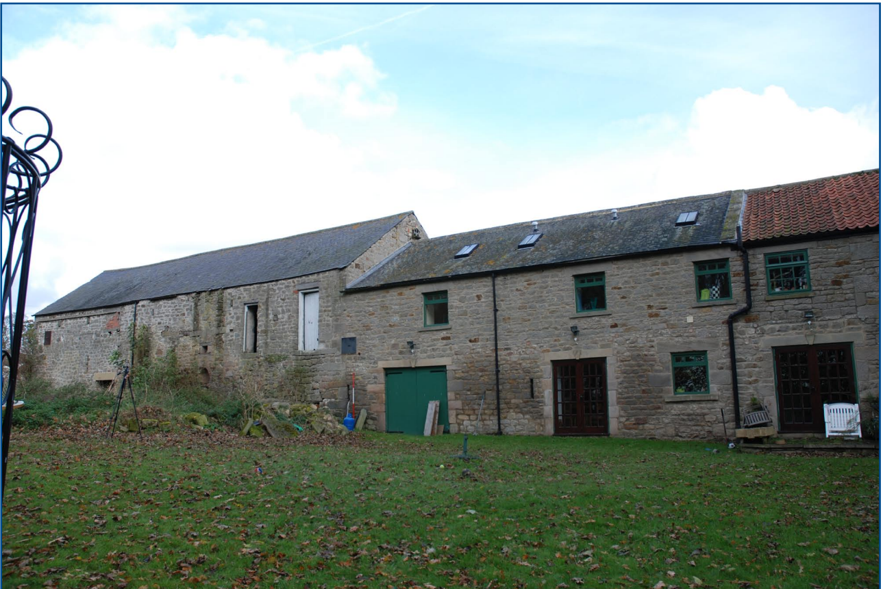
Plate 16: General view of barn from south-west
