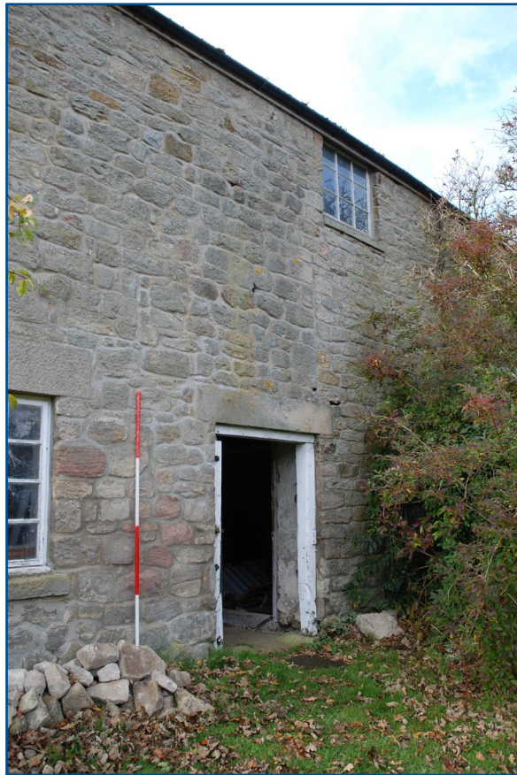
Plate 17: Detail of central door and edge of blocked door in east elevation of barn from east
