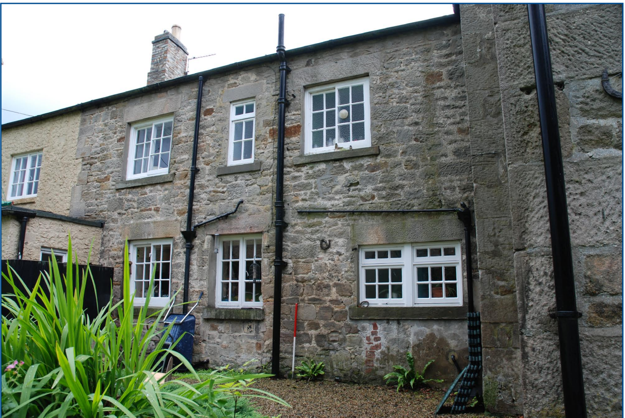
Plate 6: General view of centre of west elevation of Manor House from west
