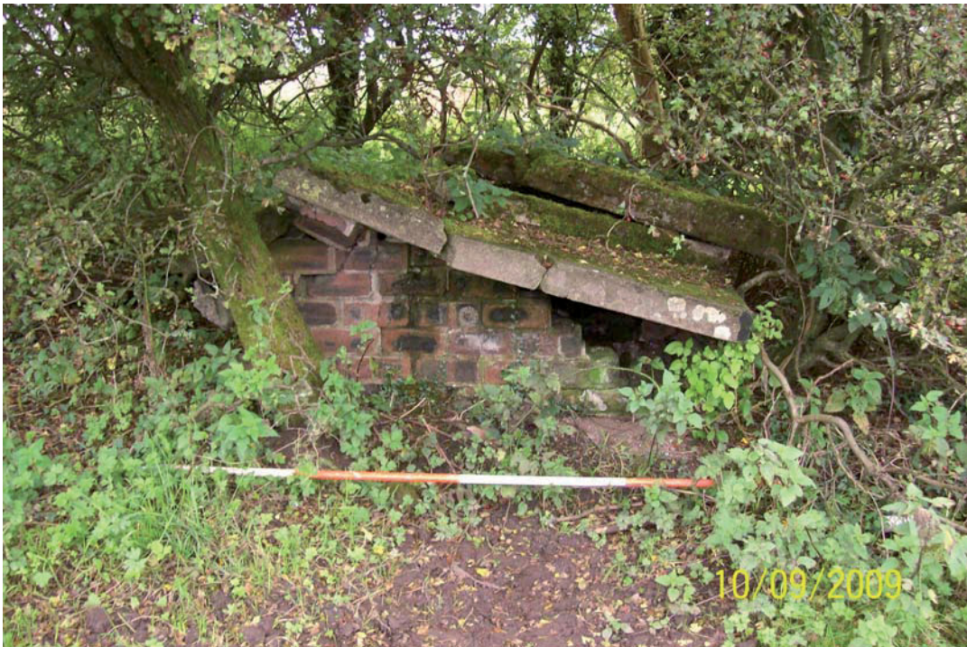
Plate 3: Detail of Structure E
