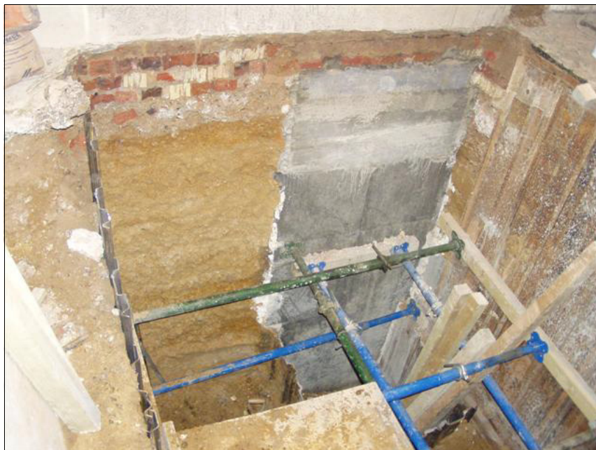
Plate1: Terrace gravels below basement slab.
