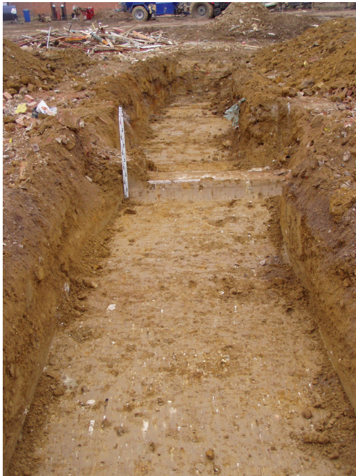
Plate 2. Trench 3 general shot east facing.
